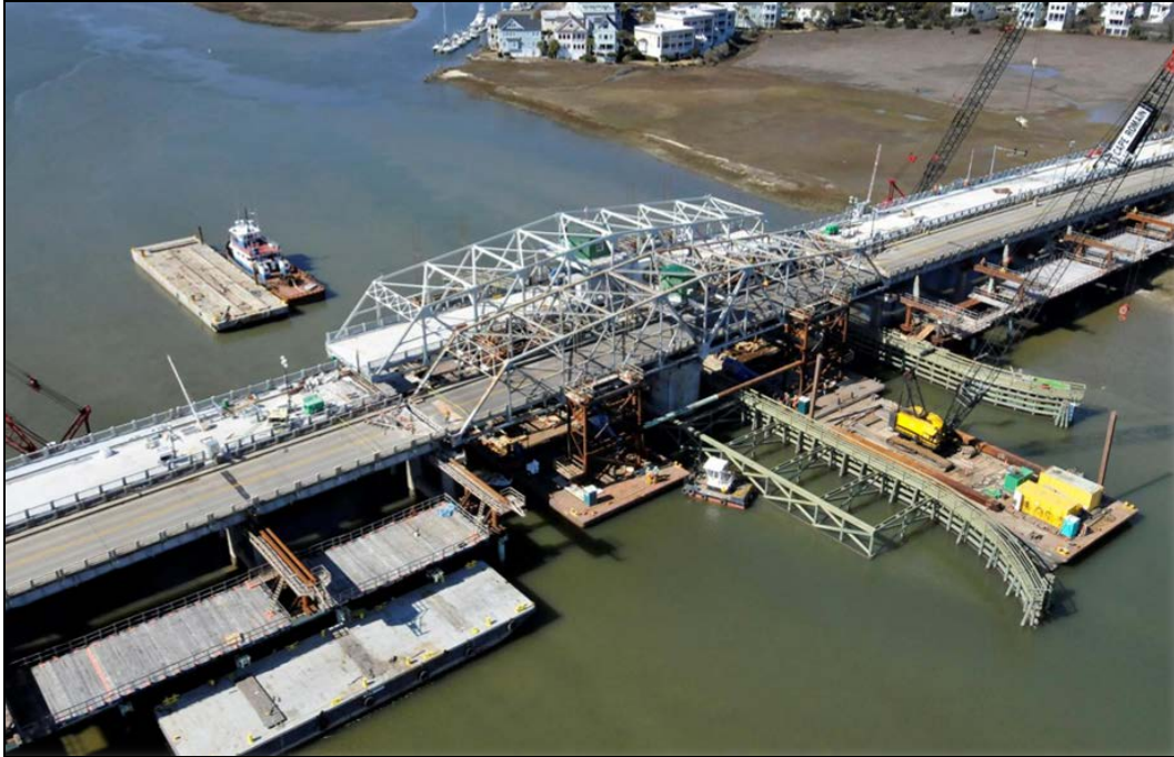
Figure 13. Existing and new bridge elements before bridge closure.
