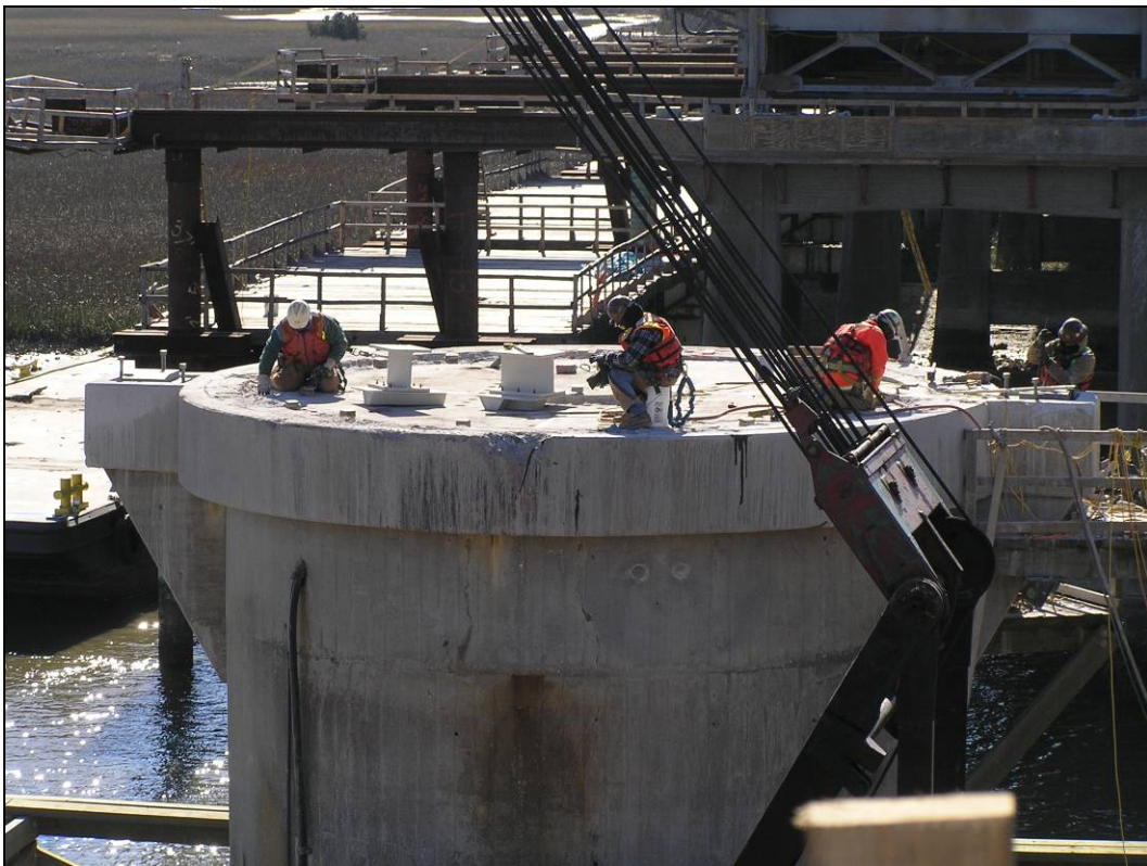
Figure 9. Pivot pier repairs during bridge closure.
