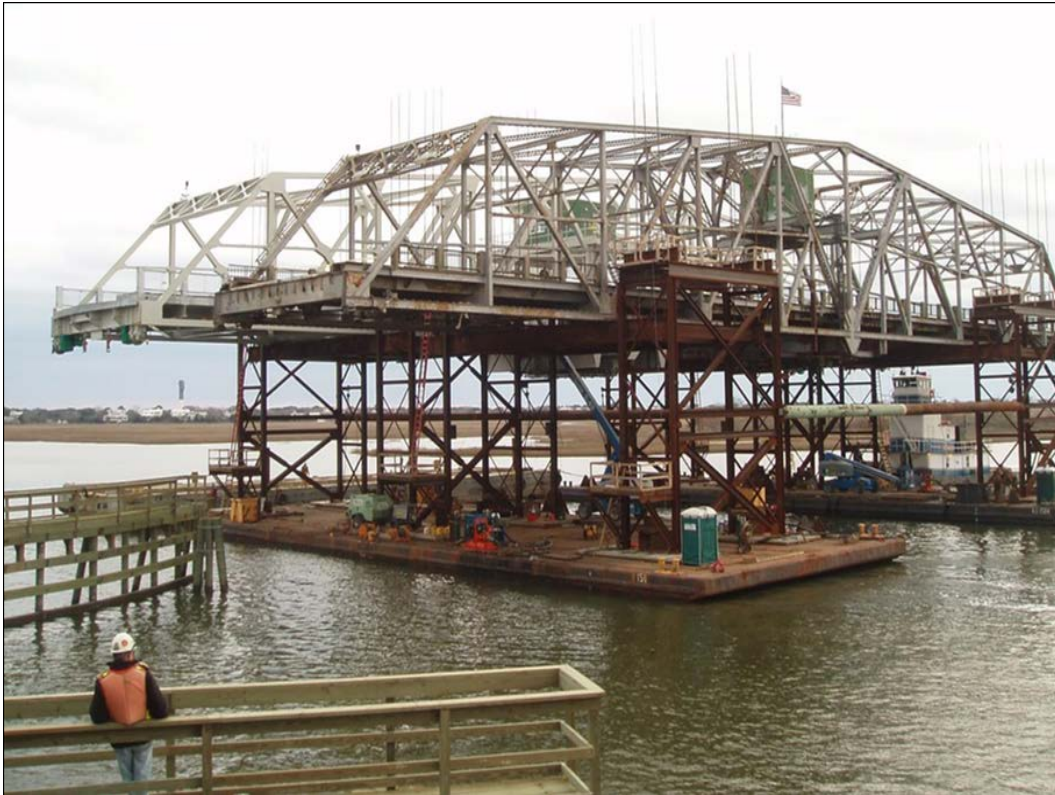
Figure 12. Existing and new swing spans shown side by side on supporting barges.
