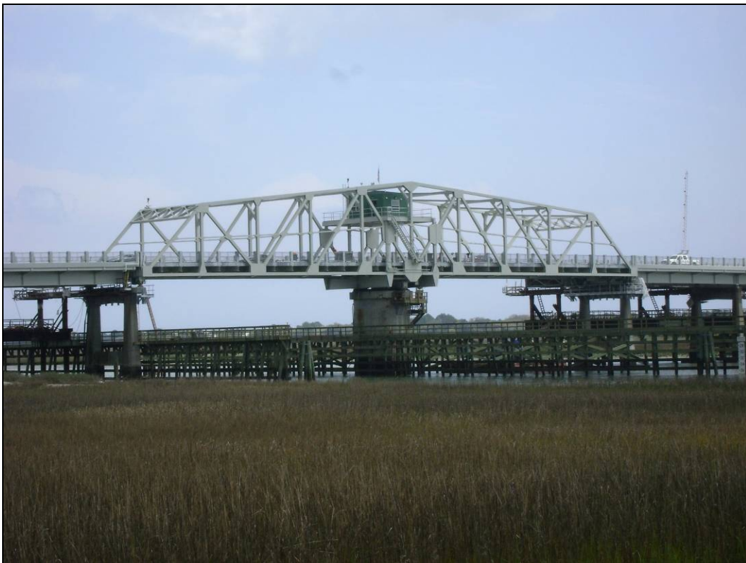
Figure 14. Completed bridge replacement.
