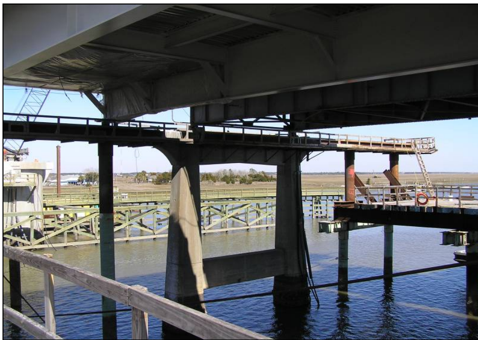
Figure 4. Approach span existing piers.
