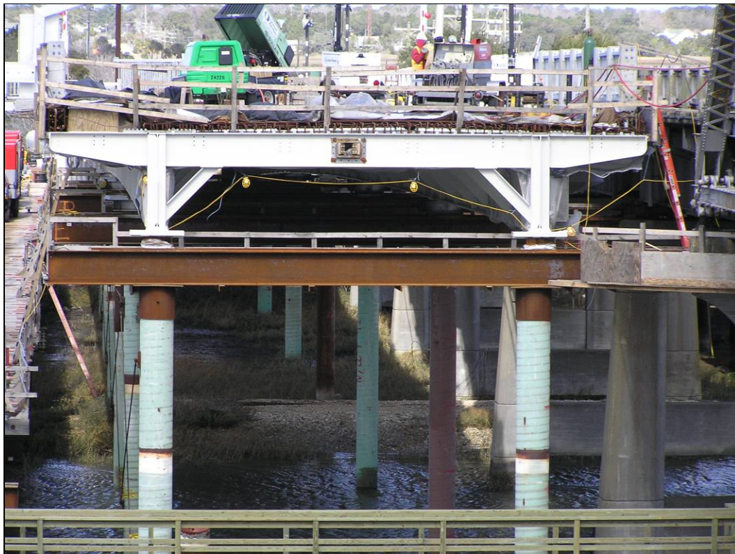
Figure 7. New approach span before sliding into place.
