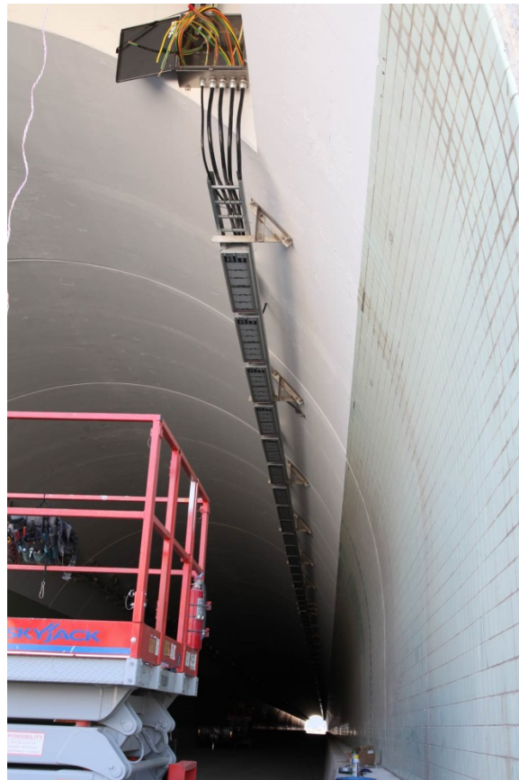
Figure 12. Photo. Installation of LED lighting system.
