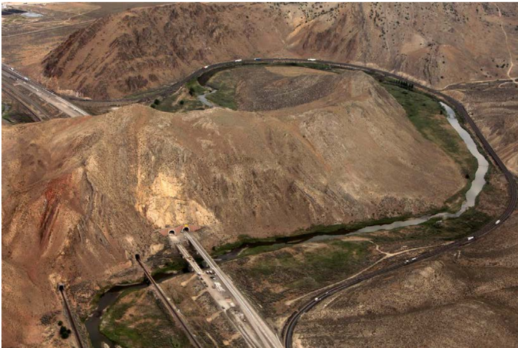
Figure 10. Photo. Bird's eye view of Carlin Tunnels project and detoured traffic.
