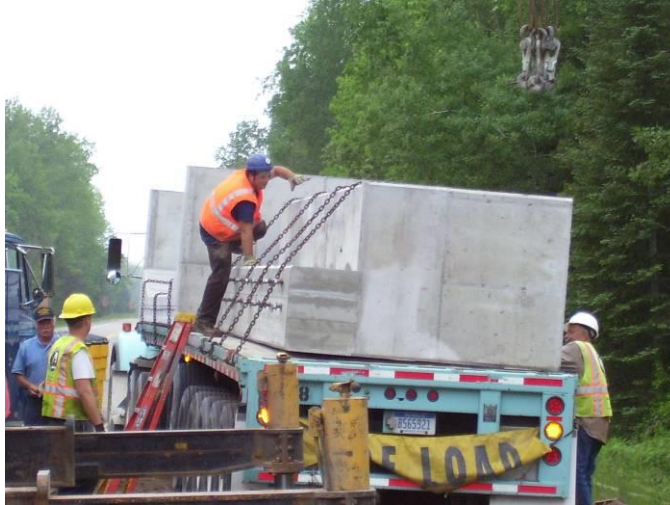
Figure 12. Transporting and unloading the precast bridge elements.
