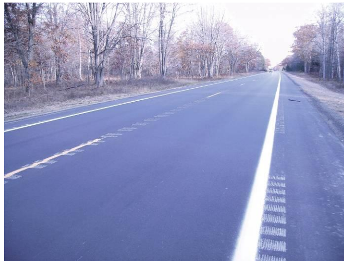
Figure 27. Final pavement surface following application of 5E3 top course.
