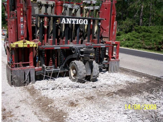
Figure 23. Rubblization of PCC pavement.
