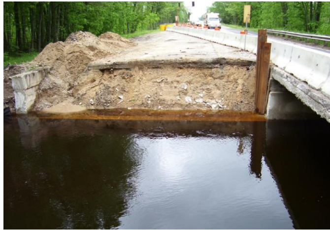
Figure 10. Removal of part of the old bridge with one-lane traffic on the rest of the bridge.
