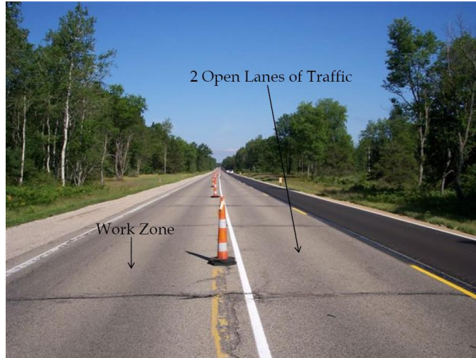
Figure 20. Fully open roadway with two lanes open to traffic.
