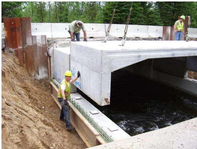
Figure 14. Adjusting the placement of the precast bridge element.
