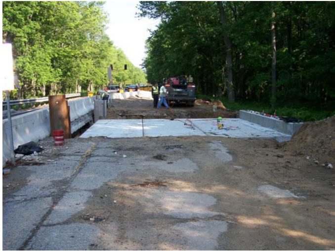
Figure 16. Bridge elements set to grade.
