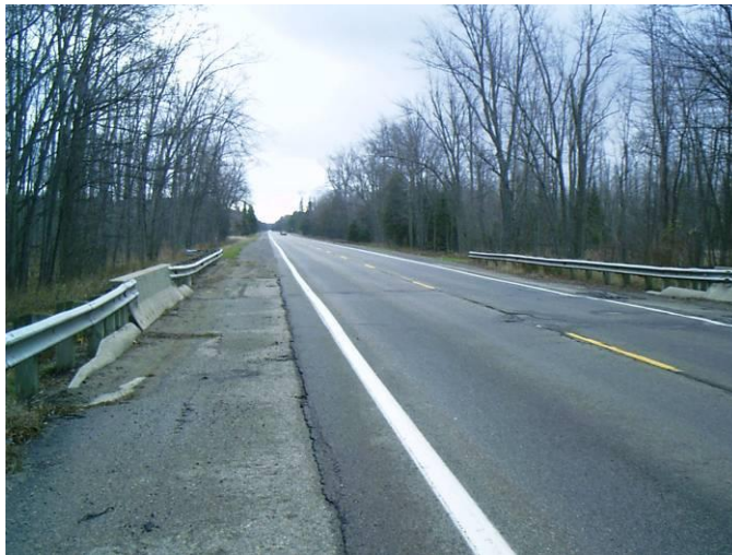
Figure 3. Small bridge over Norway Creek.
