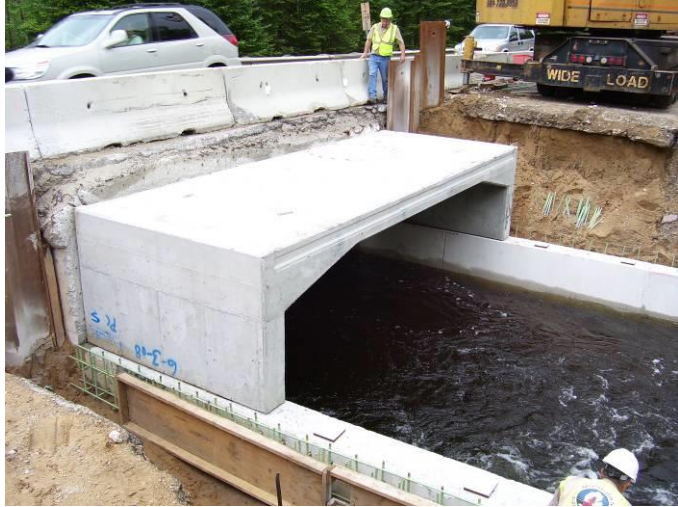
Figure 15. Final placement of a precast bridge element.
