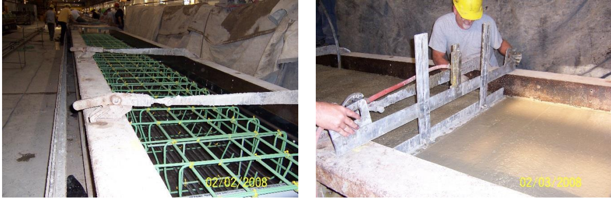
Figure 8. Precasting of MD 28 bridge slabs.
