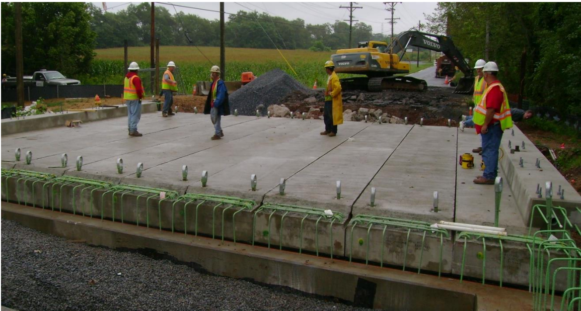
Figure 11. Completion of slab placement at MD 28 project.
