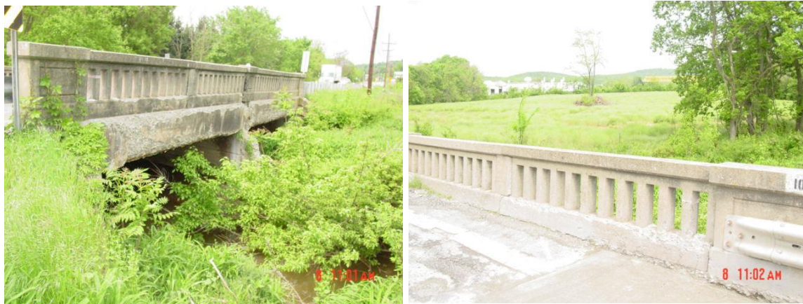
Figure 19. Previous condition of MD 28 bridge over Washington Run.
