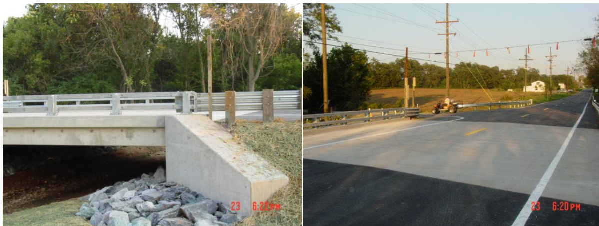
Figure 20. New condition of replaced MD 28 bridge over Washington Run.
