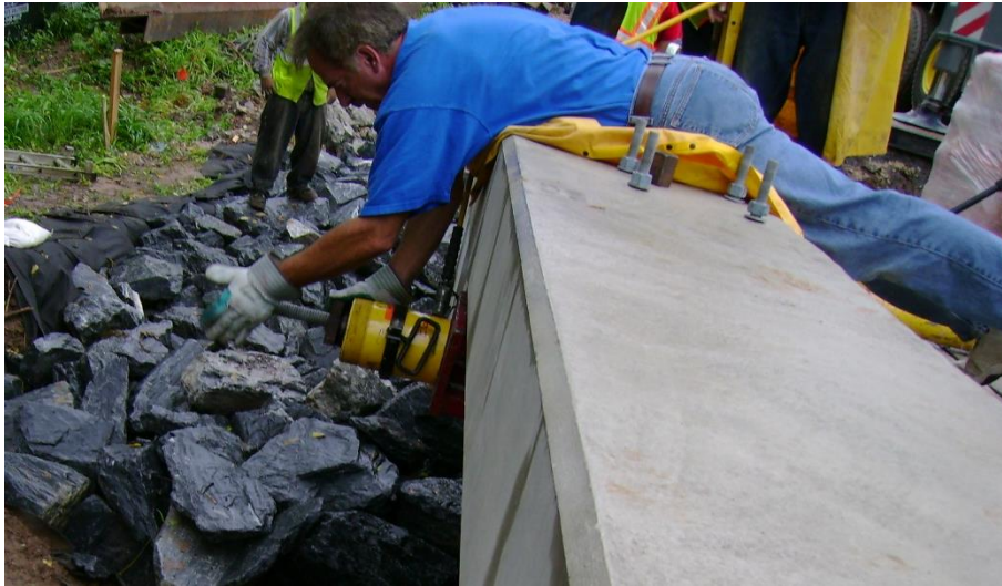
Figure 12. Preparation of post-tensioning on tie rod at MD 28 project.
