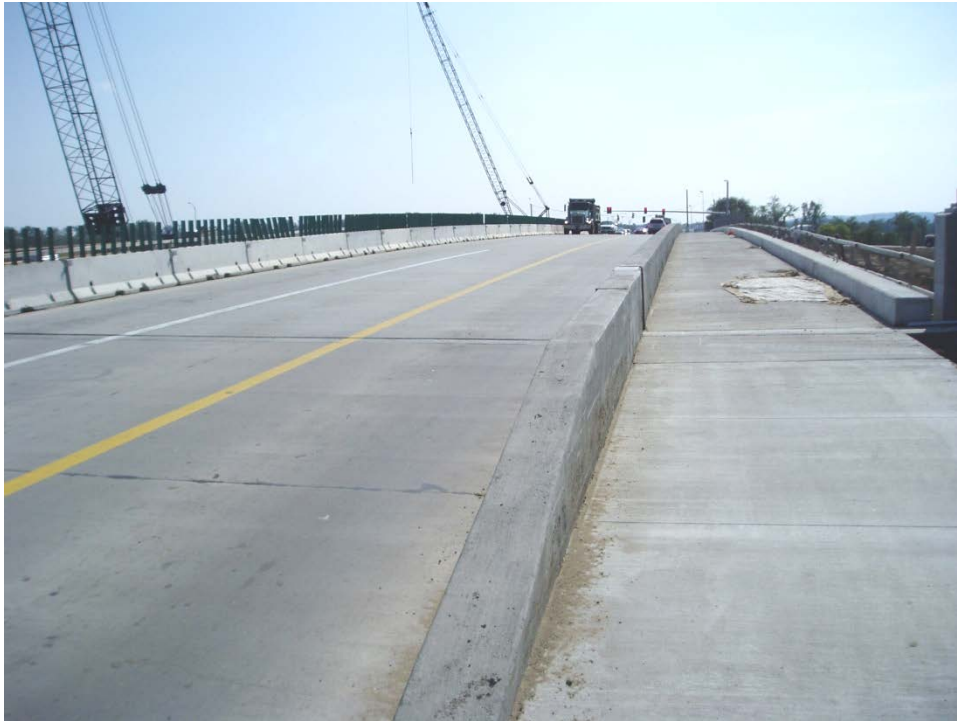
Figure 21. Phase one of the bridge construction open to traffic.
