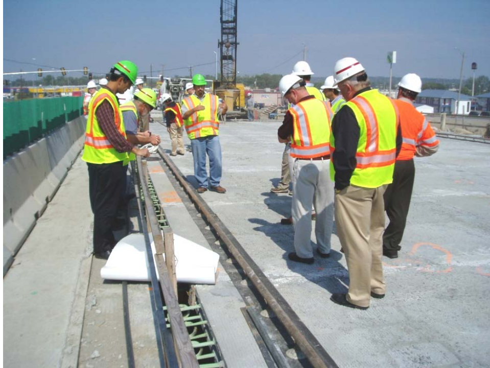
Figure 22. Showcase participants examining the new bridge construction.
