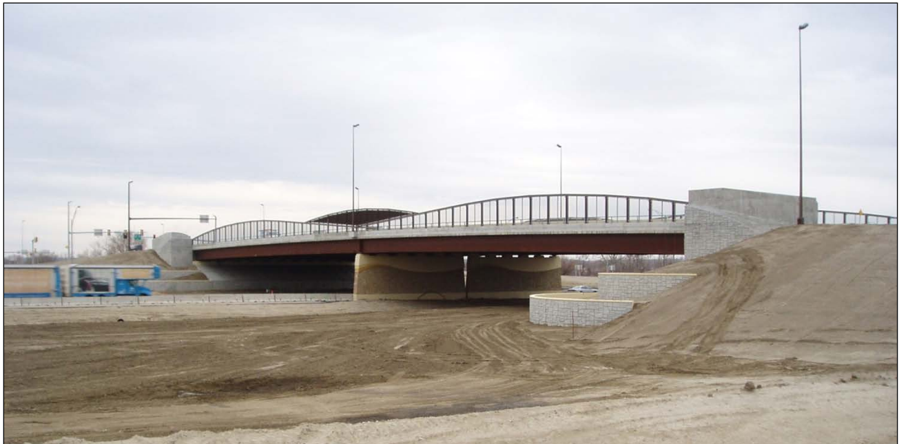
Figure 3. New 24th Street bridge near completion.
