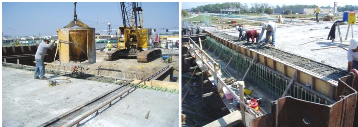
Figure 11. Casting HPC at the bridge abutments.
