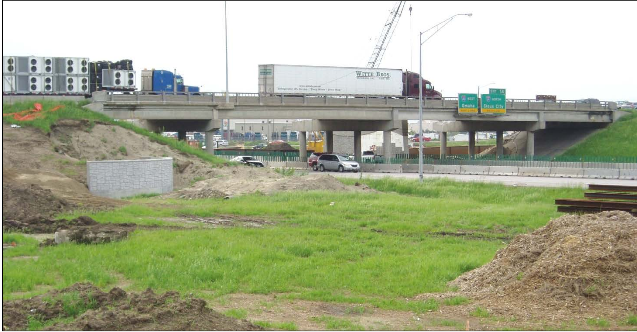
Figure 2. Existing four-span bridge.
