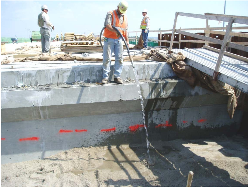
Figure 13. Flooding the self-contained backfill with water to achieve consolidation.
