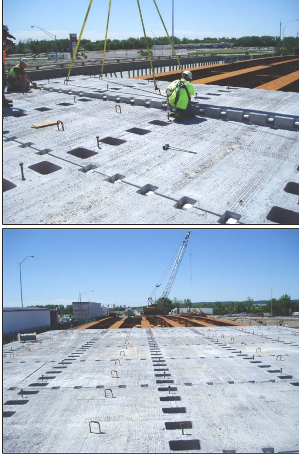
Figure 6. Panel being placed and several panels installed on the new bridge girders.
