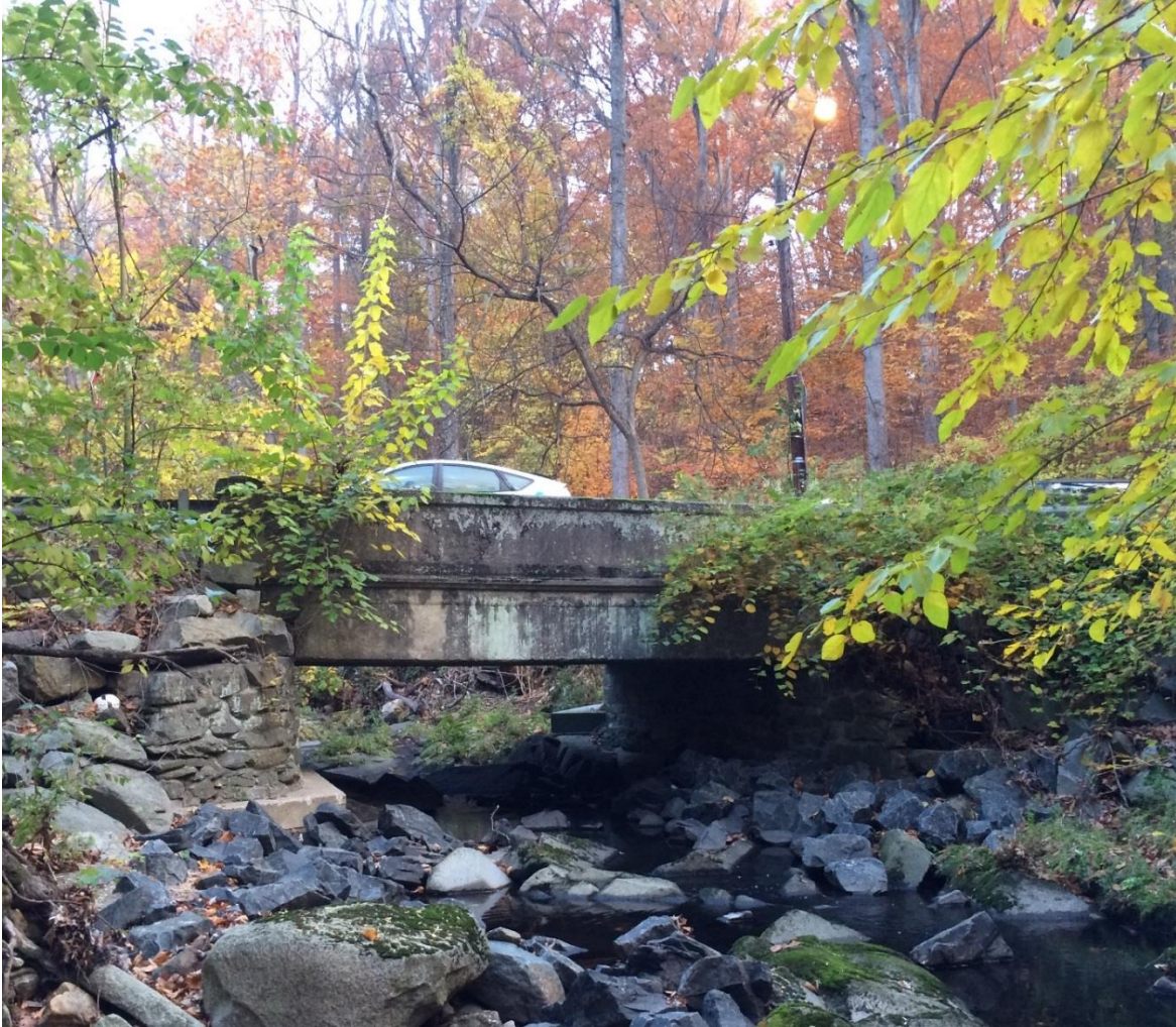
Figure 5. Photo. South face of existing bridge (courtesy: DDOT).
