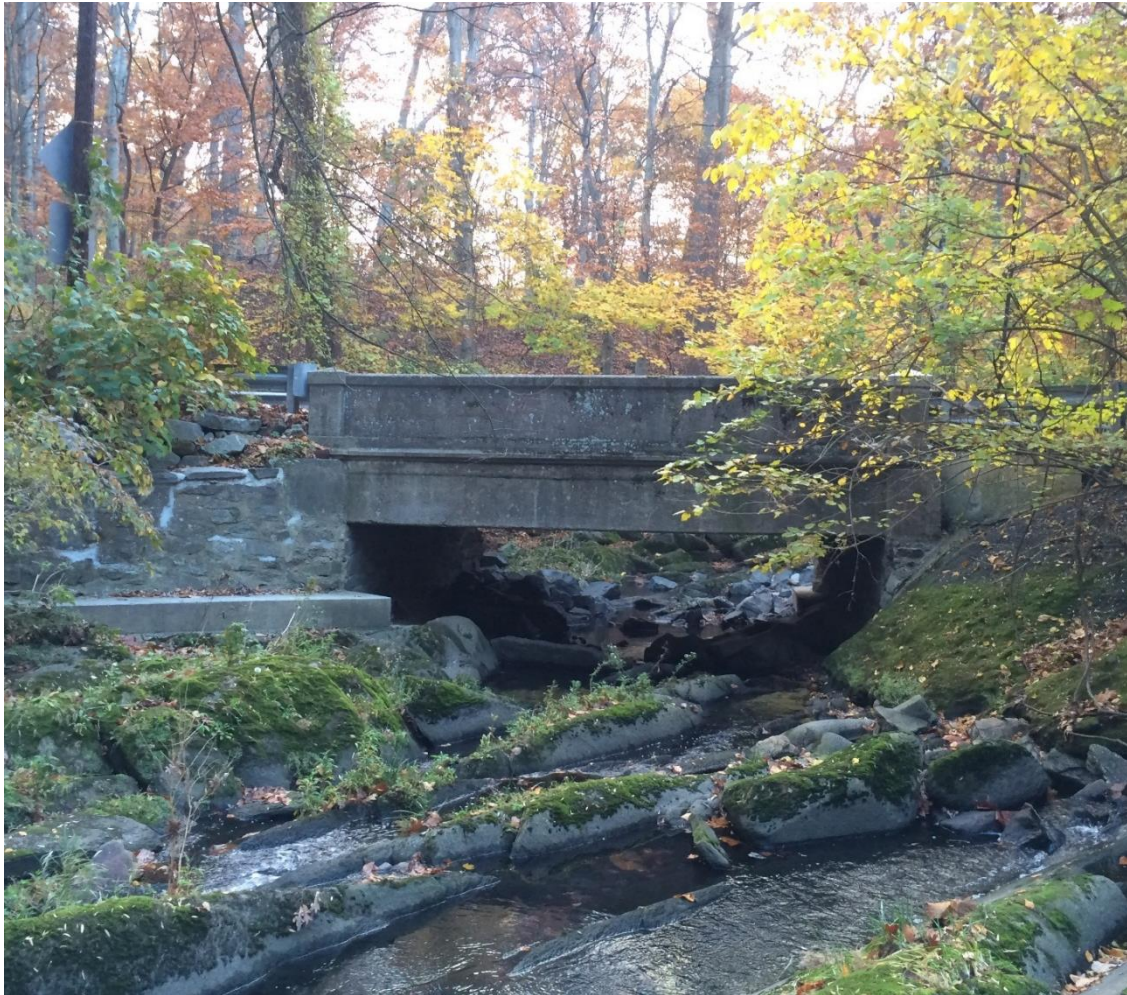
Figure 4. Photo. North face of existing bridge (courtesy: DDOT).
