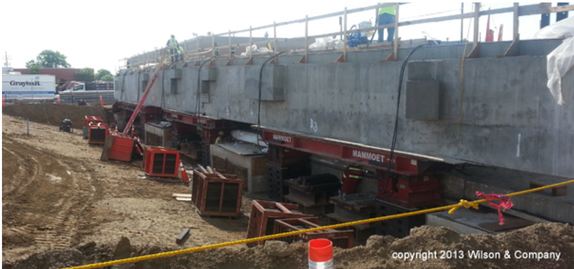
Figure 22. Photo. End diaphragms on temporary support (courtesy: Colorado DOT).
