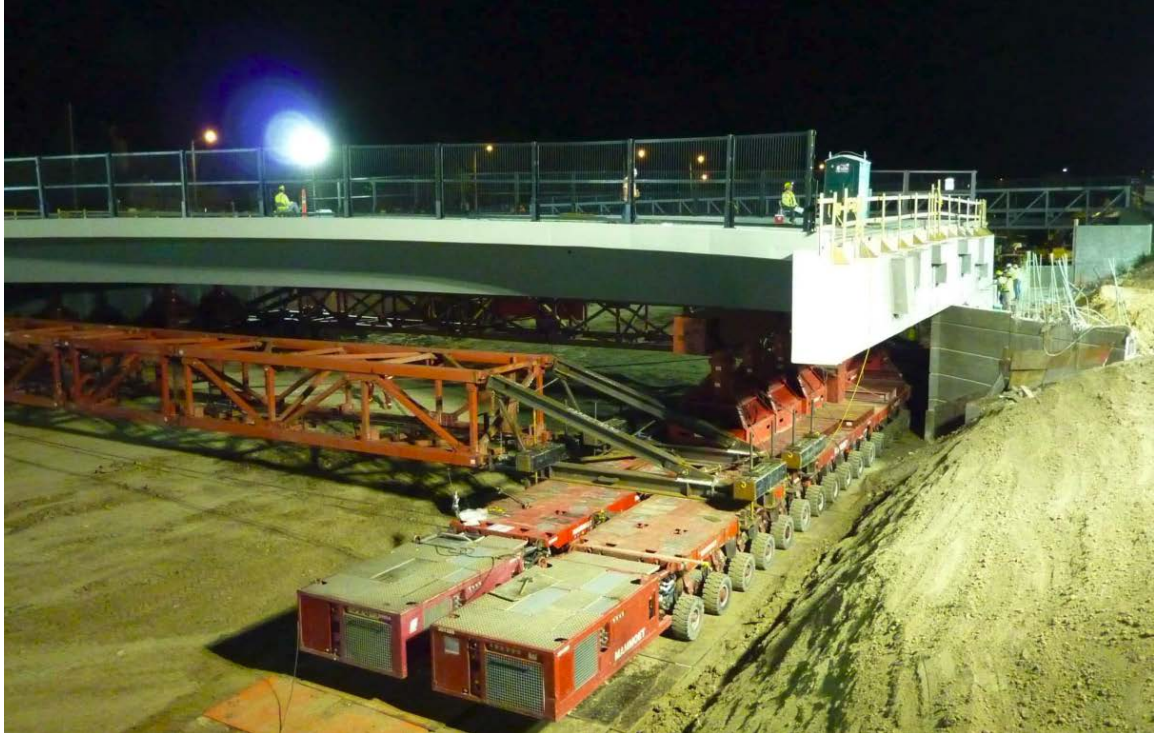
Figure 32. Photo. Superstructure being placed over abutments (courtesy: Colorado DOT).
