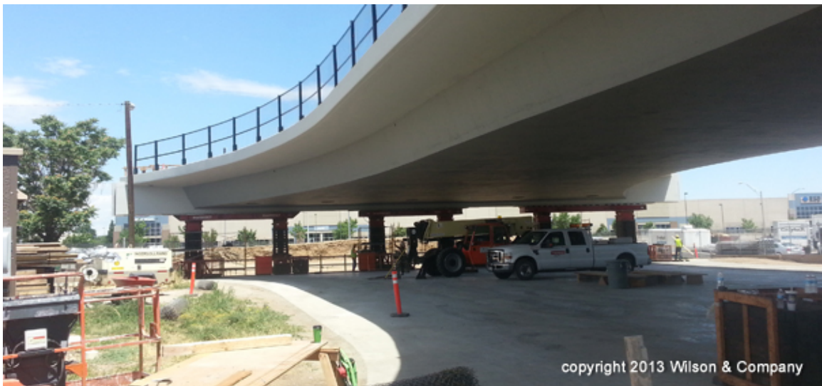
Figure 23. Photo. Superstructure lifted at end diaphragm supports (courtesy: Colorado DOT).
