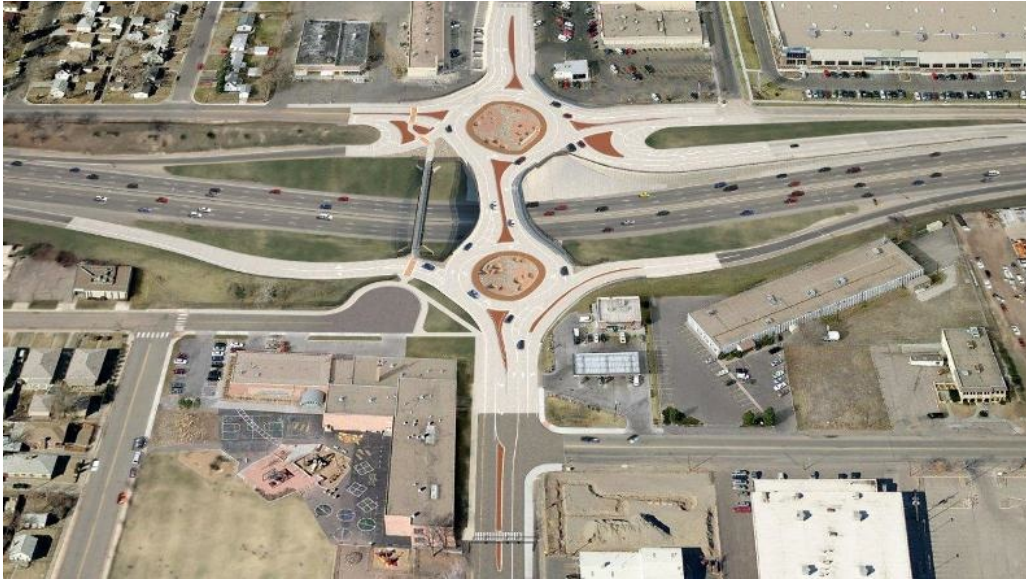
Figure 35. Photo. Plan view of completed project (courtesy: Colorado DOT).
