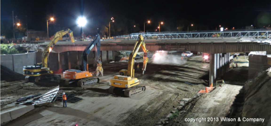
Figure 28. Photo. Demolition of old structure underway (courtesy: Colorado DOT).
