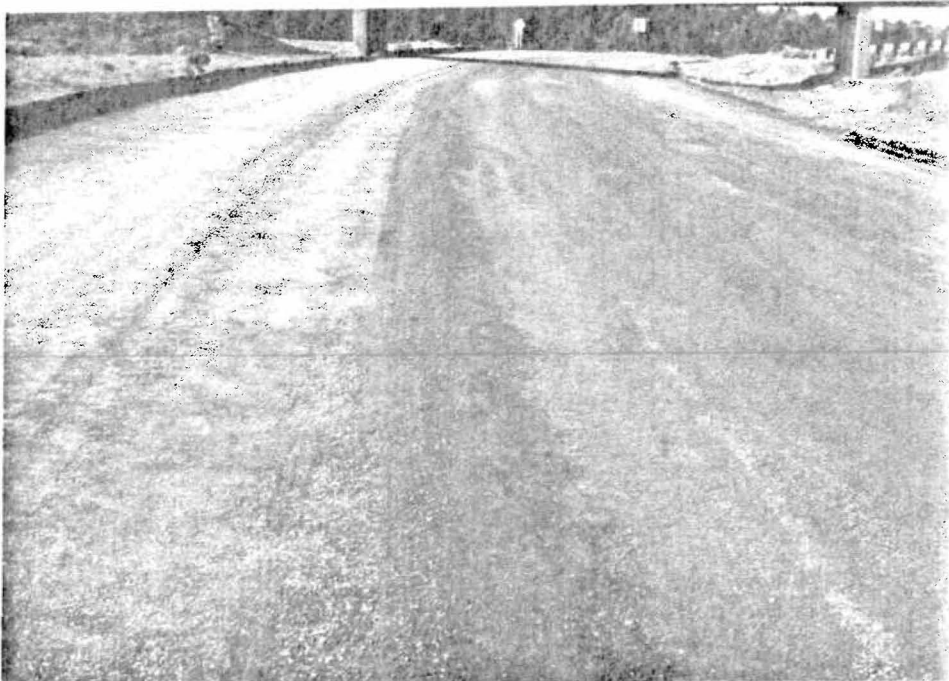
FINISHED BASE GRAVEL
