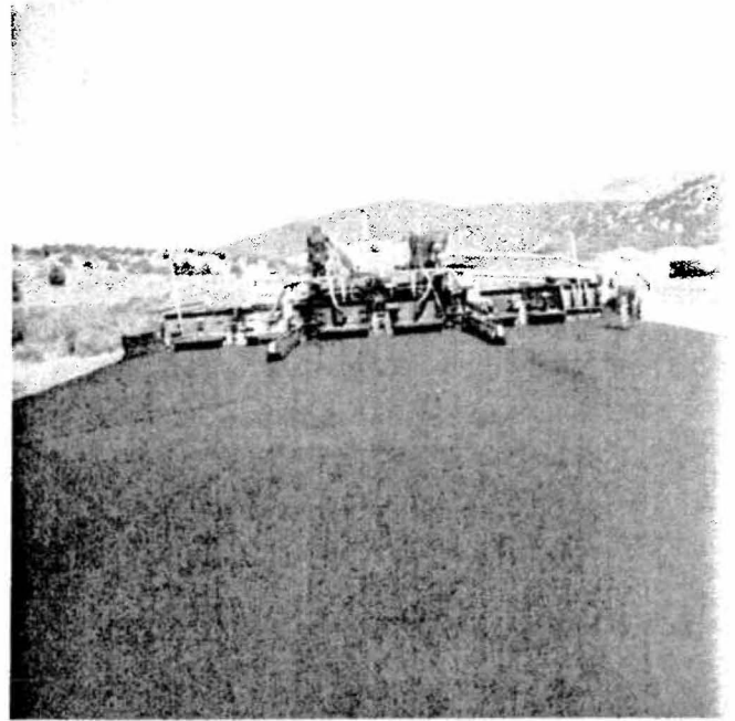
1979 LAYDOWN ON SOUTHBOUND LANES, NOTE FULL WIDTH PAVING
