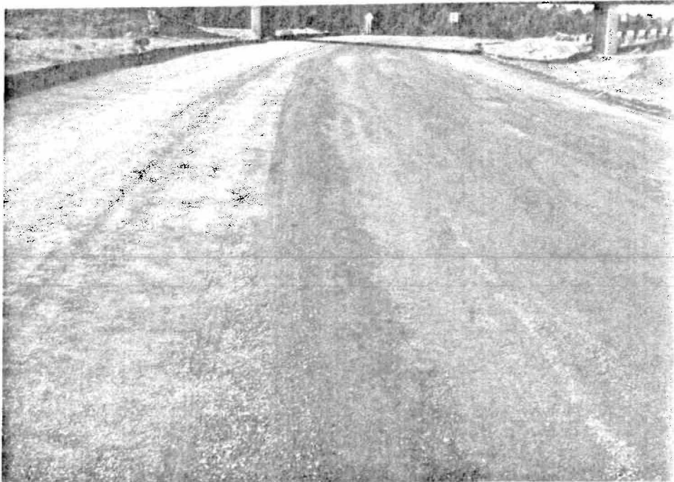
FINISHED BASE GRAVEL
