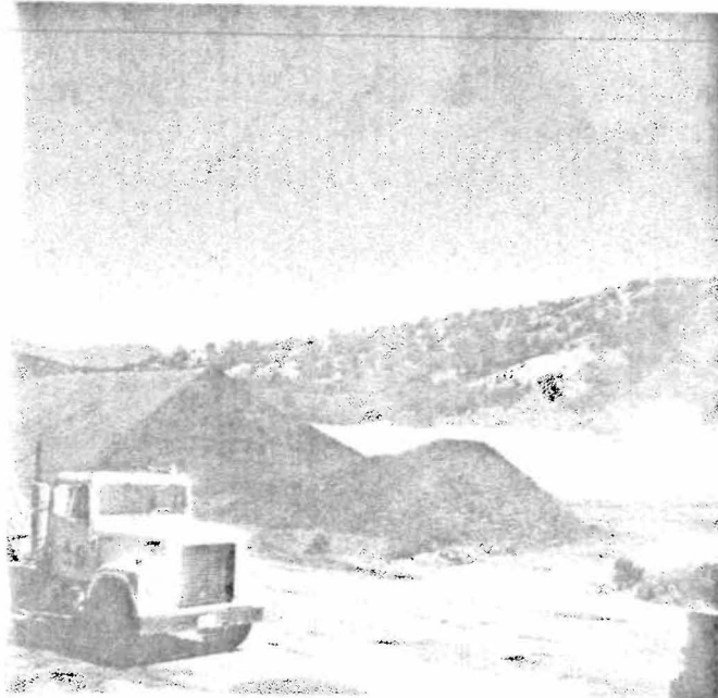
RECLAIMED PAVEMENT STOCKPILE
