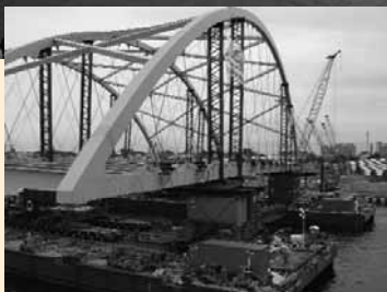
Rhode Island's Providence River Bridge was prefabricated and then transported using two barges to the bridge site in August 2006.
