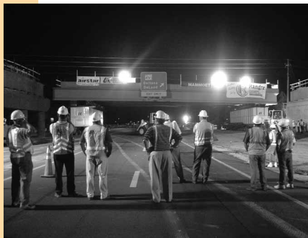
The new Graves Avenue Bridge is installed in Volusia County, FL, in June 2006. The prefabricated bridge spans were lifted and moved using self-propelled modular transporters.
