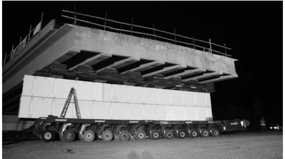
SPMTs are multi-axle computer controlled vehicles that can move in any horizontal direction and also have vertical lift.
