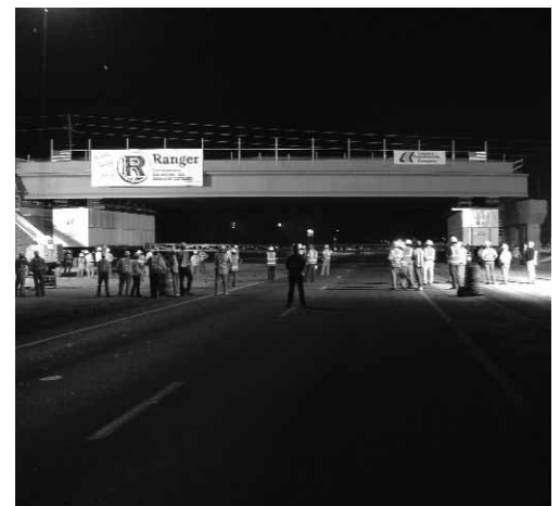
The new Graves Avenue Bridge is installed in Volusia County, FL, in June 2006. The prefabricated bridge spans were lifted and moved using self-propelled modular transporters.
