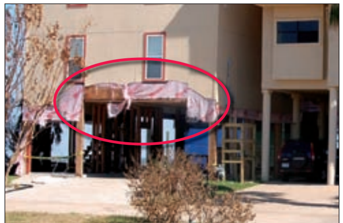
Figure 3. NFIP-compliant breakaway wall construction.
