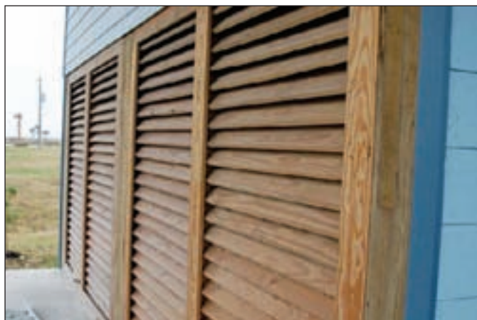
Figure 1. Wood louvers installed beneath an elevated house in a V zone are a good alternative to solid breakaway walls.
