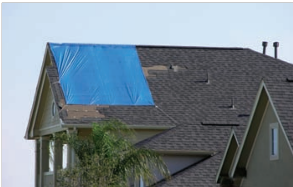
Figure 3-62. Shingle damage at a house near the one shown in Figure 3-61 (Webster, TX)
