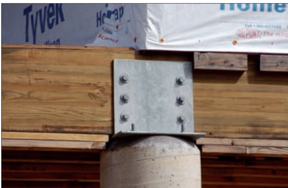
Figure 3-49. Strong concrete column-to-beam steel saddle connector
