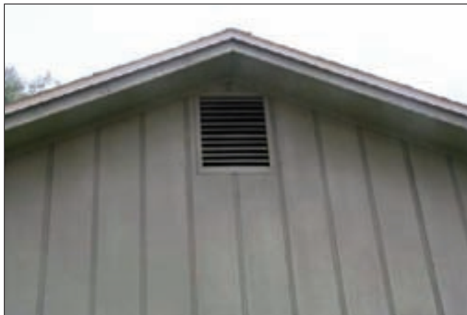
Figure 9. Gable end vent.
