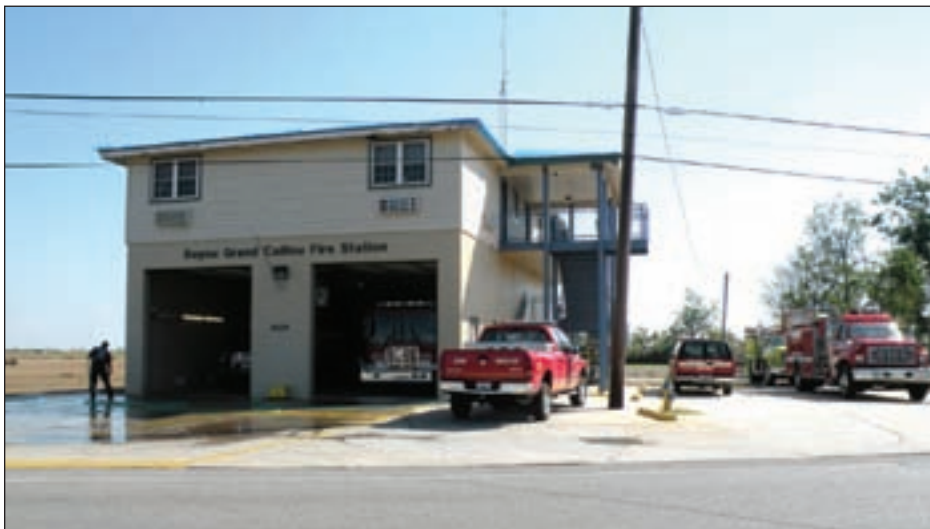
Figure 4-55. The Bayou Grand Caillou Fire Station is elevated above the ABFE and sustained no damage
