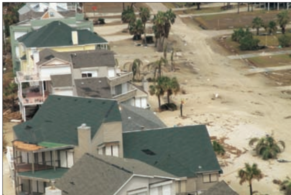
Figure 3-59. A substantial amount of siding (the white lines scattered around the ground), along with roofing materials, blew off these West Galveston, TX, houses (Hurricane Ike estimated wind speed in this area: 90 mph)
