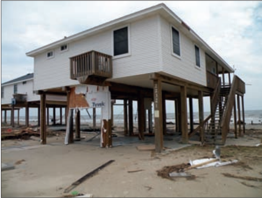
Figure 3-113. Elevated condenser is tightly enclosed, making service access difficult (Bermuda Beach, TX; Hurricane Ike estimated wind speed in this area: 95 mph, Exposure C)
