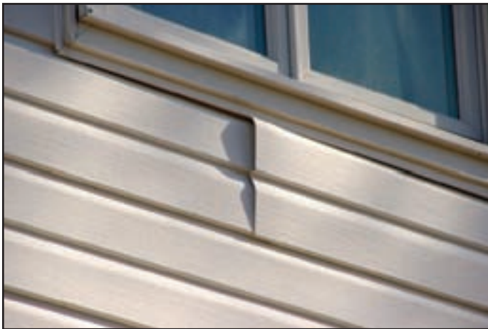
Figure 6. Proper detailing around windows and other obstacles is important. Use utility trim, punch snap-locks into siding, and don't overlap directly beneath a window.
