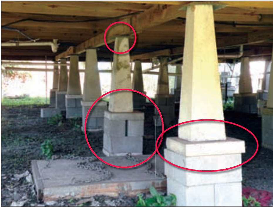
Figure 3-29. House resting (i.e., with no structural connection) on top of precast concrete piers, stacked CMUs, and shallow footing pads (New Iberia, LA)
