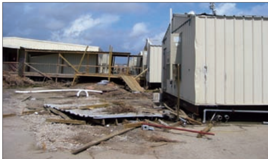
Figure 4-7. Damage to South Cameron Parish School modular units
