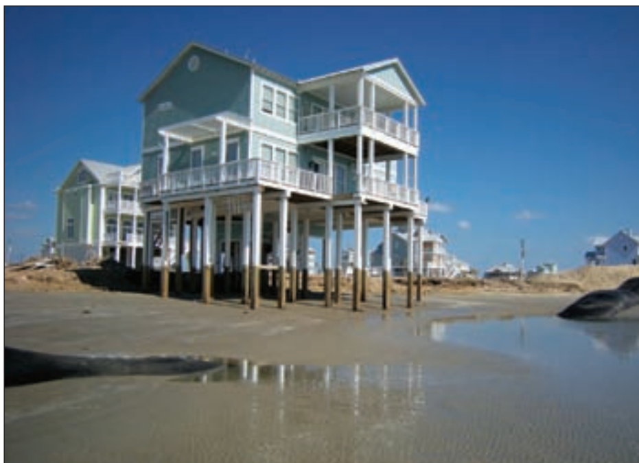
Figure 8-3. Broken geotextile tube at Beachside Drive, Galveston Island, TX
