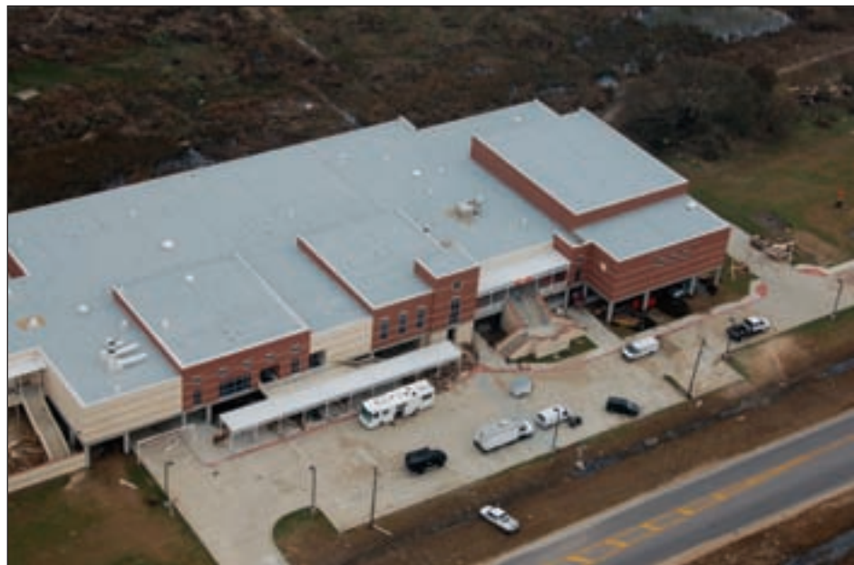
Figure 4-1. September 19, 2008, aerial view of Crenshaw Elementary and Middle School
