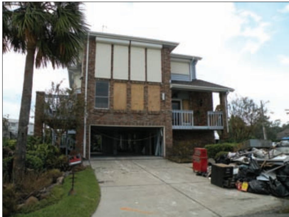
Figure 3-96. Clear Lake, TX, house with plywood shutters installed on the accessible first floor and roll-down shutters installed on the less accessible second floor (Hurricane Ike estimated wind speed in this area: 90 mph, Exposure B)
