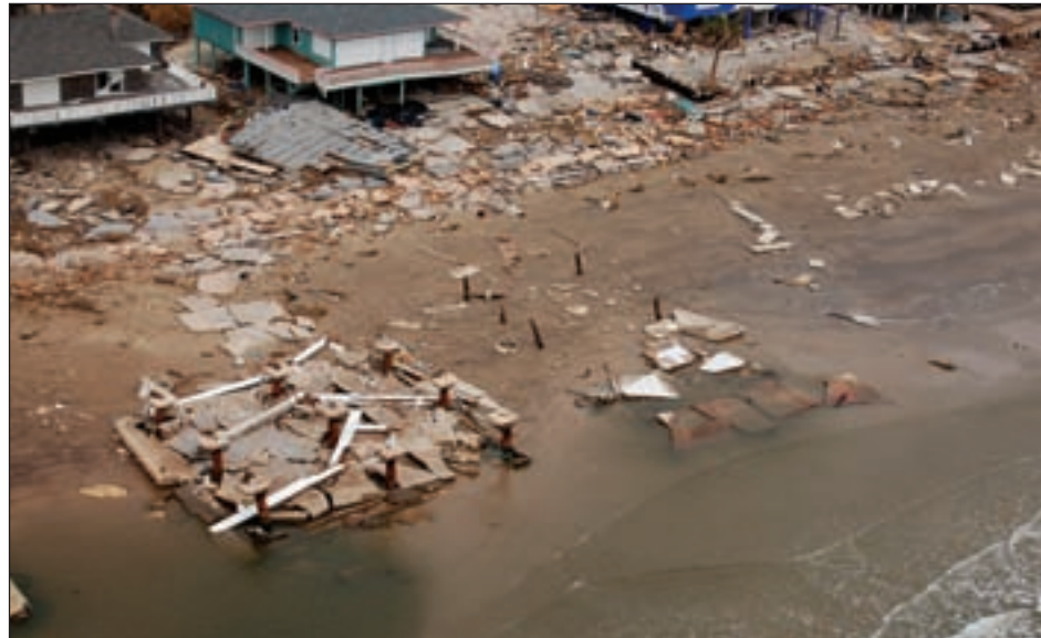
Figure 3-57. Post-Ike photograph of West Galveston Island, TX, illustrating increased severity of flood damage near the shoreline
