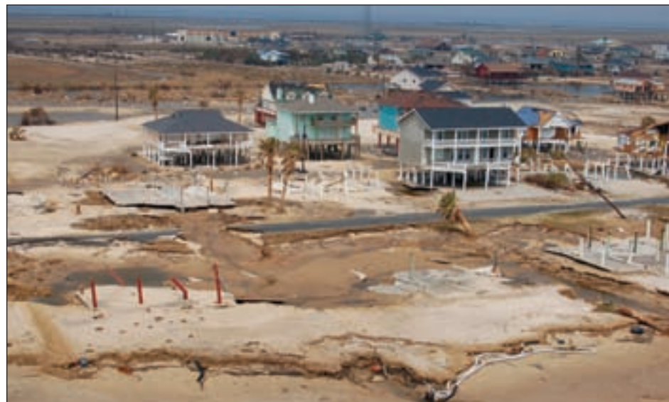
Figure 3-58. Post-Ike photograph of Bolivar Peninsula, TX, illustrating increased severity of flood damage near the shoreline
