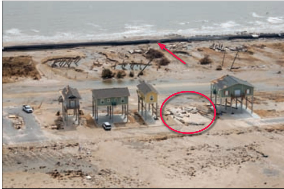
Figure 3-13. Looking toward the Gulf, past Zone V houses on tall concrete column foundations (with the lowest floor 10 feet above the 17-foot BFE). Four of the five tall houses shown in this photograph survived Ike (red circle indicates destroyed house). The red arrow points to exposed geotextile tube (under former dune). Note other destroyed houses (not on tall foundations) seaward of the highway (Bolivar Peninsula, TX).
