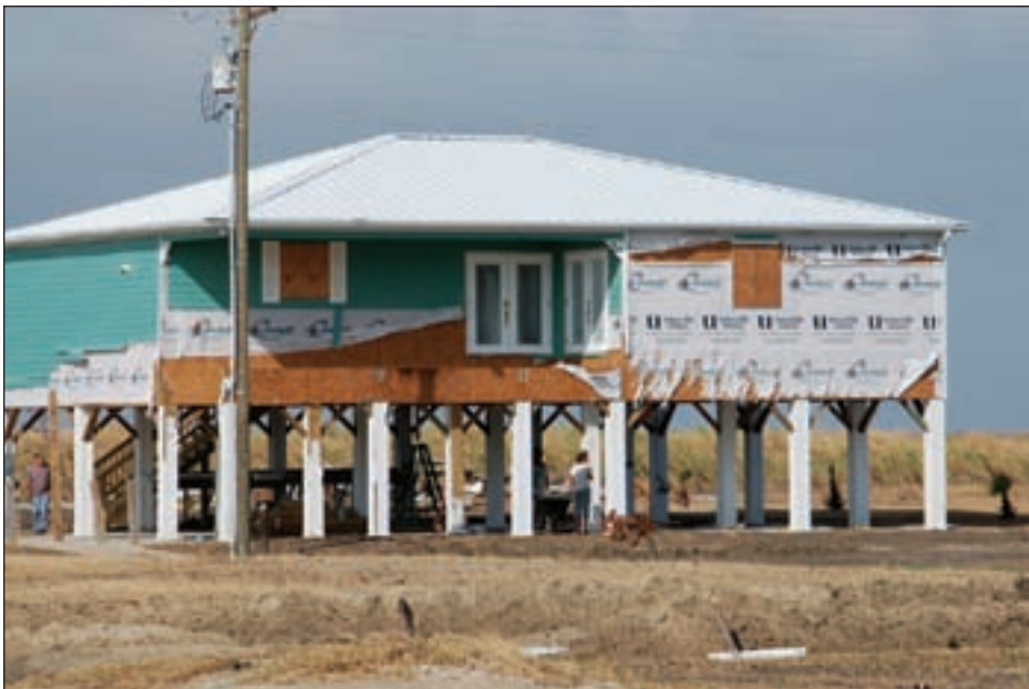
Figure 3-74. Loss of siding at Holly Beach, LA, home (Cameron Parish; Hurricane Ike estimated wind speed in this area 80 mph, Exposure C)
