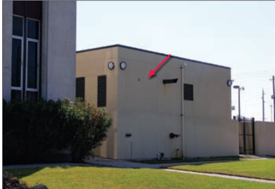
Figure 4-65. The emergency generator is housed in a separate wind- and windborne-debris-resistant building (red arrow)
