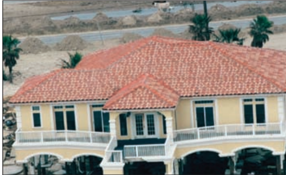
Figure 3-71. This tile roof on Galveston Island, TX, did not experience any wind damage (Hurricane Ike estimated wind speed in this area: 106 mph)
