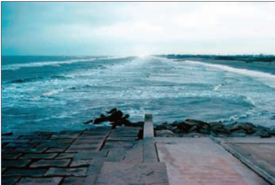
Figure 8-5. West end of the seawall at Galveston, TX. The concrete ramp (right foreground) was the road leading to the beach in the mid-1960s. Since then, the beach has eroded more than 492 feet.
