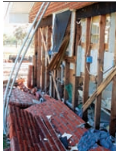
Figure 5. Damage to brick veneer walls due to shallow flooding, floating debris, and small waves. The damaged home was on a sheltered bay shoreline (Baytown, TX, Hurricane Ike).
