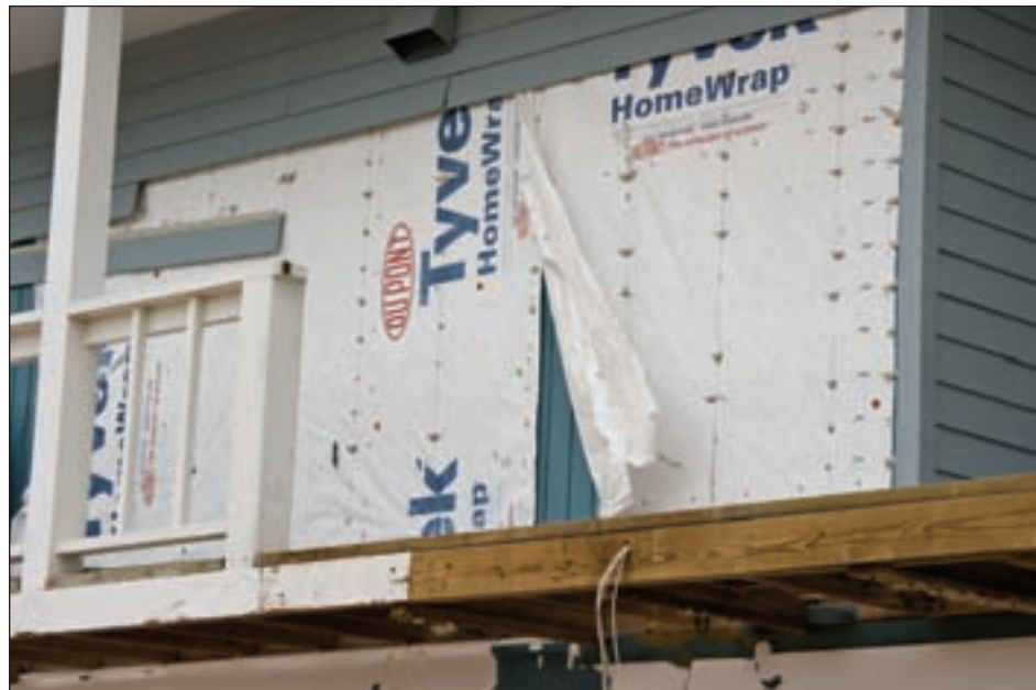
Figure 3-87. Fiber cement plank siding, installed as a reside over the original plywood siding, was torn from this West Bay, Galveston Island, TX, house (Hurricane Ike estimated wind speed in this area: 100 mph, Exposure C)
