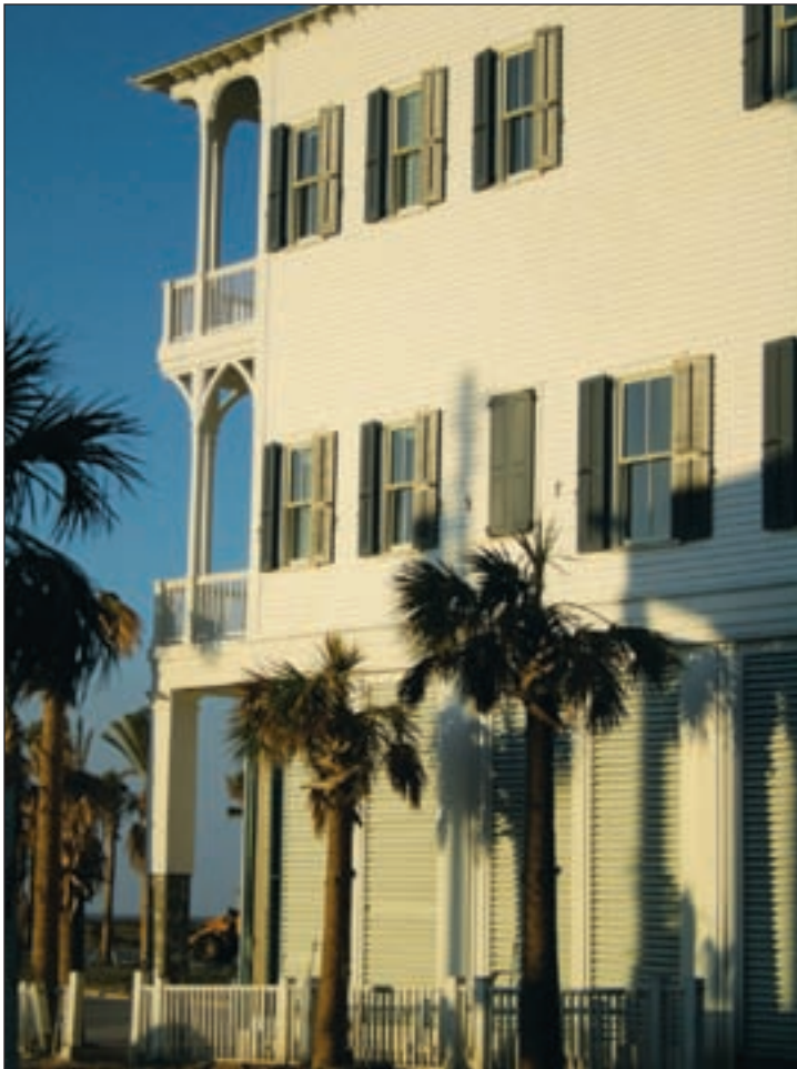
Figure 8-6. Beachtown, TX, under construction
