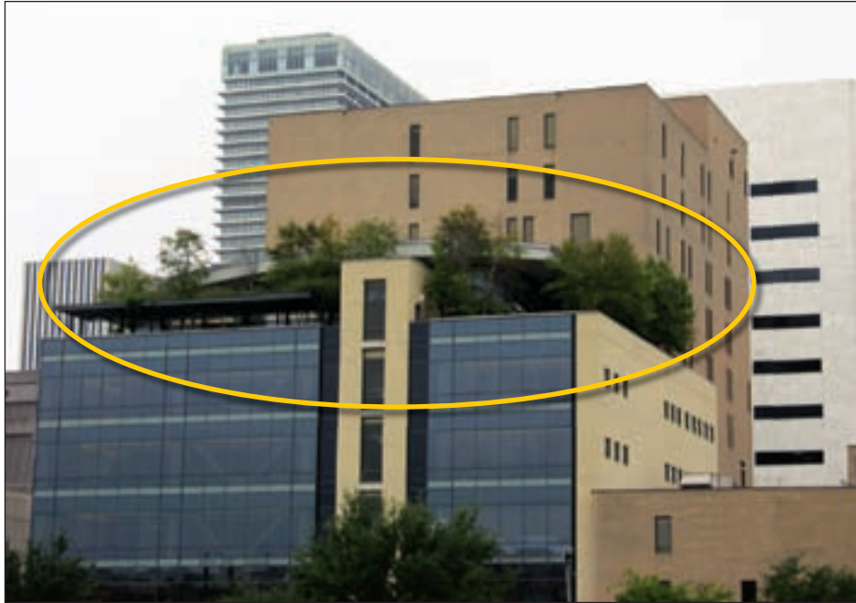
Figure 5-29. View of a vegetative roof in the downtown area
