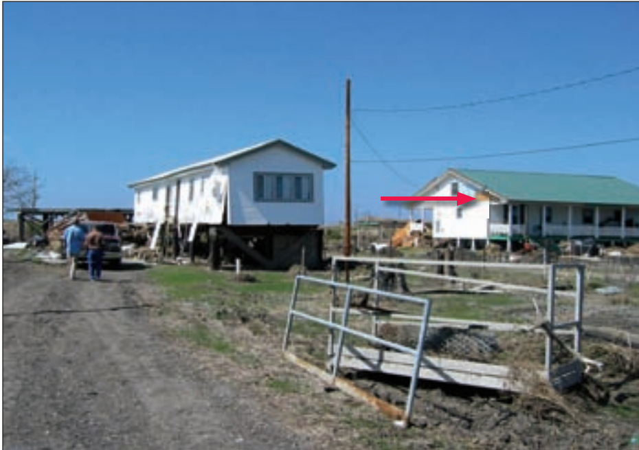
Figure 3-139. Zone A manufactured home in the Golden Meadows section of Lafourche Parish, LA, sustained 3 to 4 feet of flooding above the floor, but did not shift or float off of its foundation. The red arrow indicates the flood level reported by neighbors.
