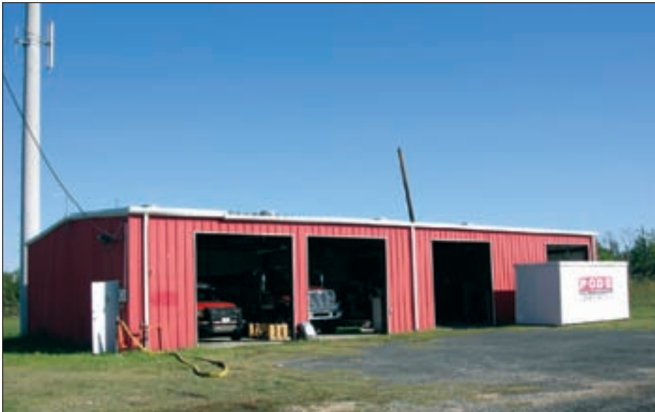
Figure 4-53. General view of High Island Fire Station
