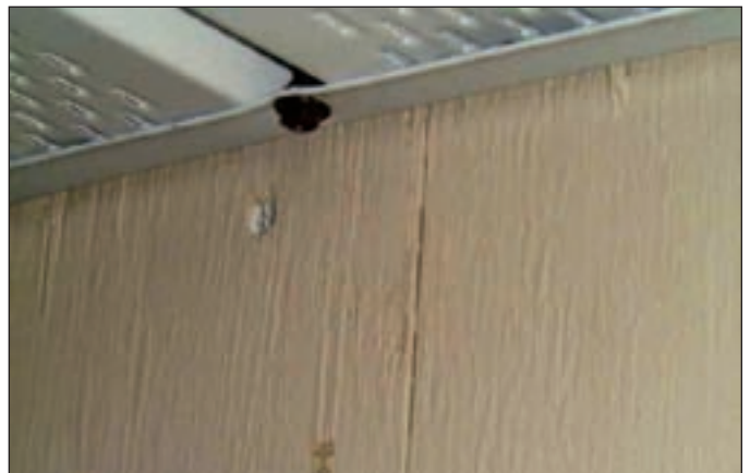
Figure 5. Screws through wall channel.
