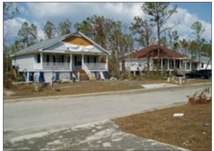
Figure 10. The site on the left is mapped Zone AE, and lies directly along the Gulf of Mexico shoreline. Limited obstructions to waves indicate the site could be classified as a Coastal A zone. The site on the right is over \frac{1}{2} mile from the Gulf shoreline, is mapped as Zone AE, and has a base flood stillwater level sufficient to support >1.5' wave heights – but obstructions to waves (e.g., trees and other buildings between the site and the shoreline) and distance from the source of flooding would indicate the area is not a Coastal A zone.
