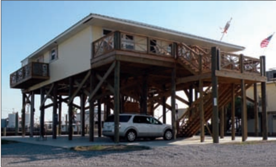
Figure 3-1. Louisiana house sufficiently elevated on a foundation that withstood Ike flood loads
