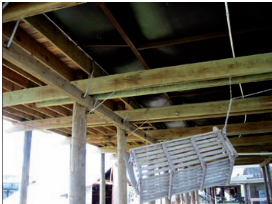
Figure 3-138. The framing and anchoring system of the house shown in Figure 3-137. Strapping secured the home's walls and frames to its foundation. While the strapping held the home to its foundation during Ike, it could not be determined if the strapping would resist a design wind event (Estimated wind speed during Ike: less than 60 mph, 3-second gust).
