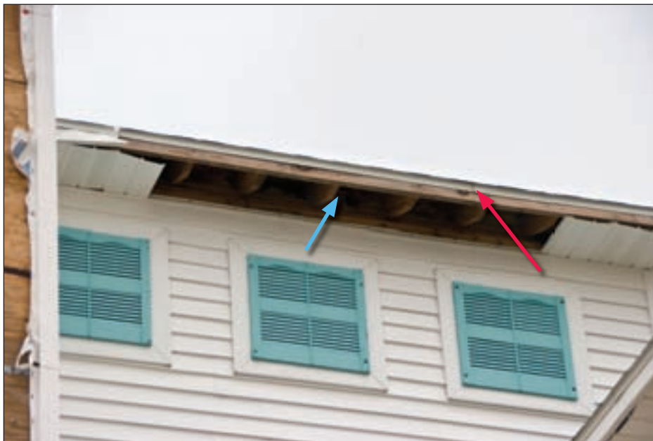
Figure 3-106. Loss of fascia cover (red arrow) led to loss of soffit (blue arrow), exposing the attic to wind-driven rain (San Luis, TX; Hurricane Ike estimated wind speed in this area: 93 mph, Exposure C)
