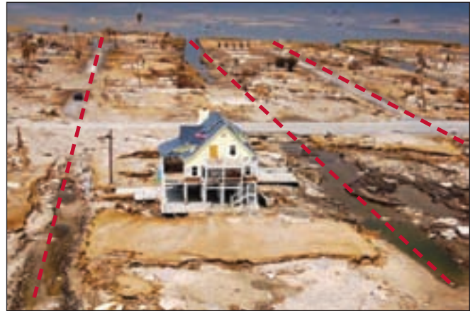
Figure 9. Linear scour and erosion patterns aligning with canals and roads (Bolivar Peninsula, TX, Hurricane Ike).
