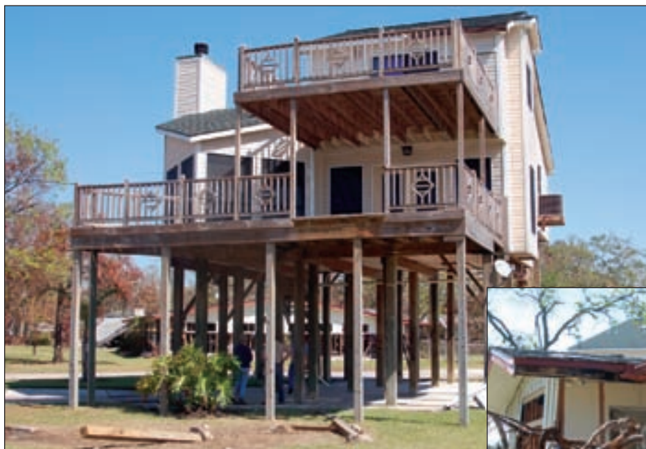
Figure 3-8. This elevated house (Zone V, BFE = 15 feet) suffered no significant damage due to flooding. The nearby at-grade house in the background, shown in the inset, was heavily damaged (Baytown, TX).
