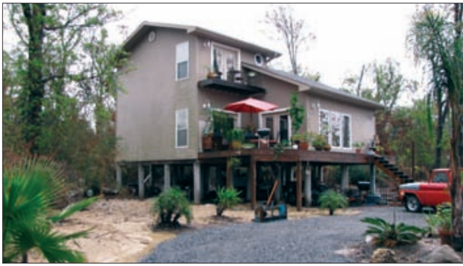
Figure 3-24. This Bridge City, TX, house sustained no structural damage, despite the fact that the owner reported that Ike flood levels rose above the lowest floor
