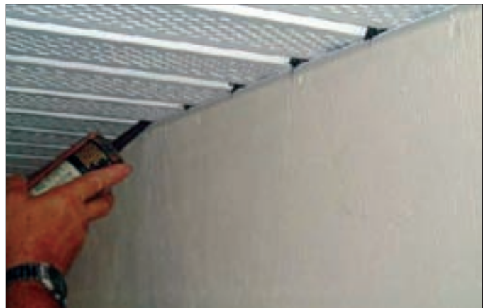
Figure 4. Applying dabs of sealant.
