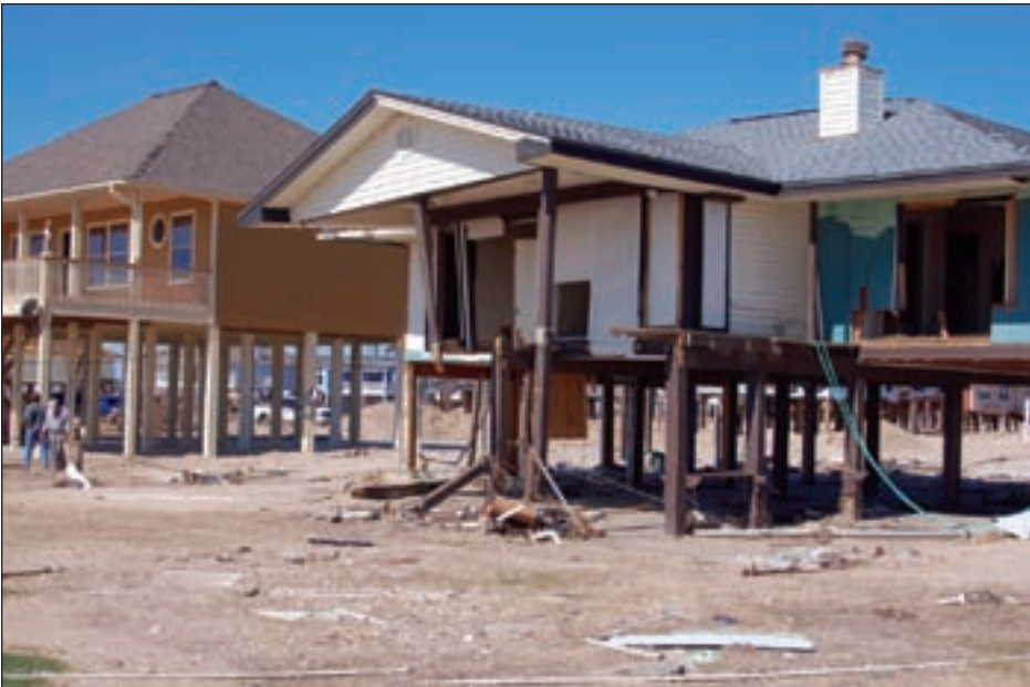
Figure 3-6. Unlike the older and lower house on the right, the Zone V house on the left was elevated approximately 5 feet above the 16-foot National Geodetic Vertical Datum (NGVD) BFE and sustained no structural damage due to flooding (Crystal Beach, TX)
