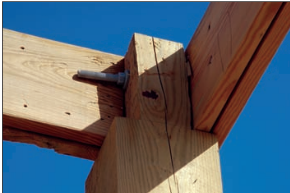
Figure 3-51. Poor beam connection to corner column
