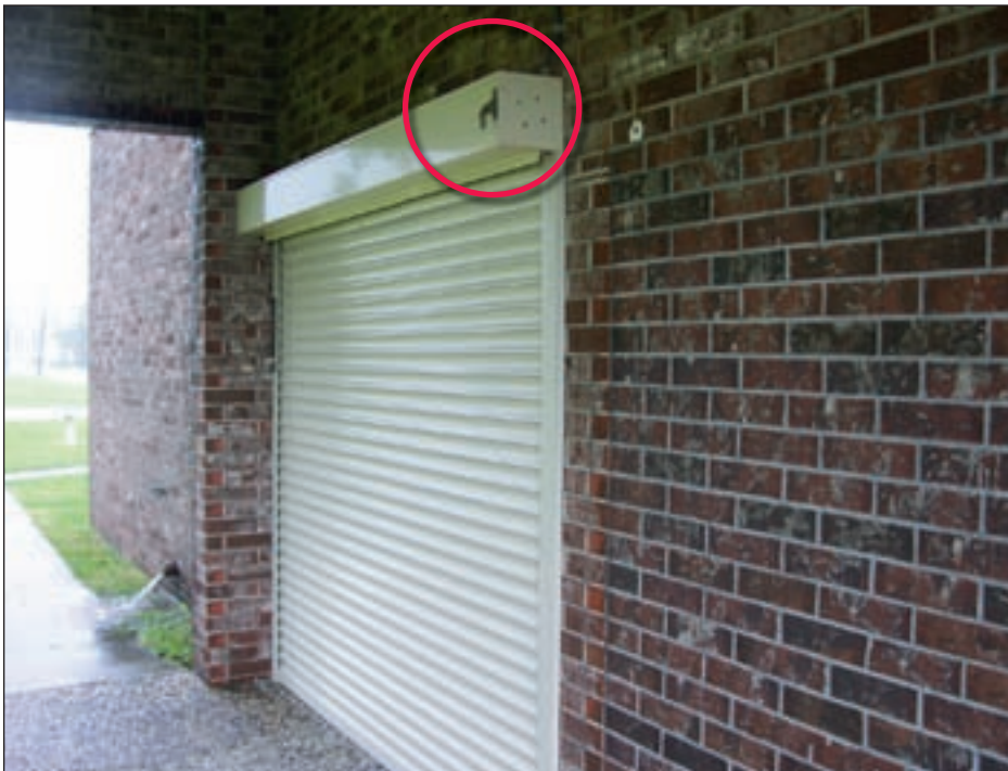
Figure 4-51. View of a new motorized shutter; the toggle in the red circle allows the shutter to be manually raised
