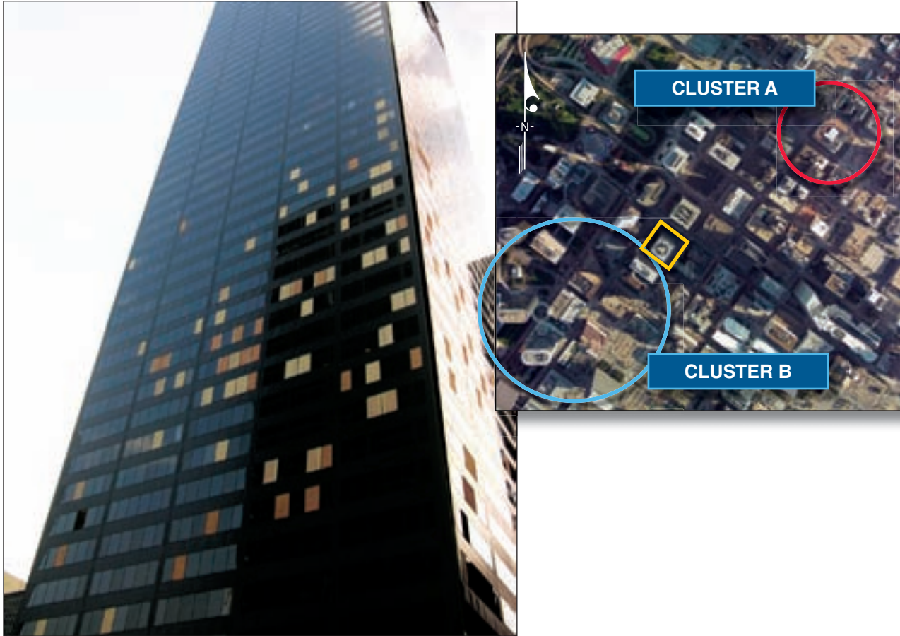
Figure 5-2. Building with glazing damage; location shown by yellow square in inset
