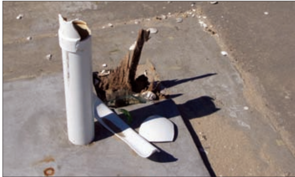
Figure 3-27. Deterioration in the wood piling likely contributed to the foundation failure (Bolivar Peninsula, TX)
