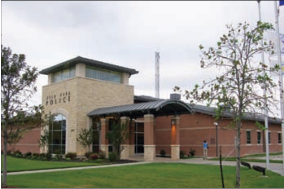
Figure 4-47. General view of Deer Park Police Station
