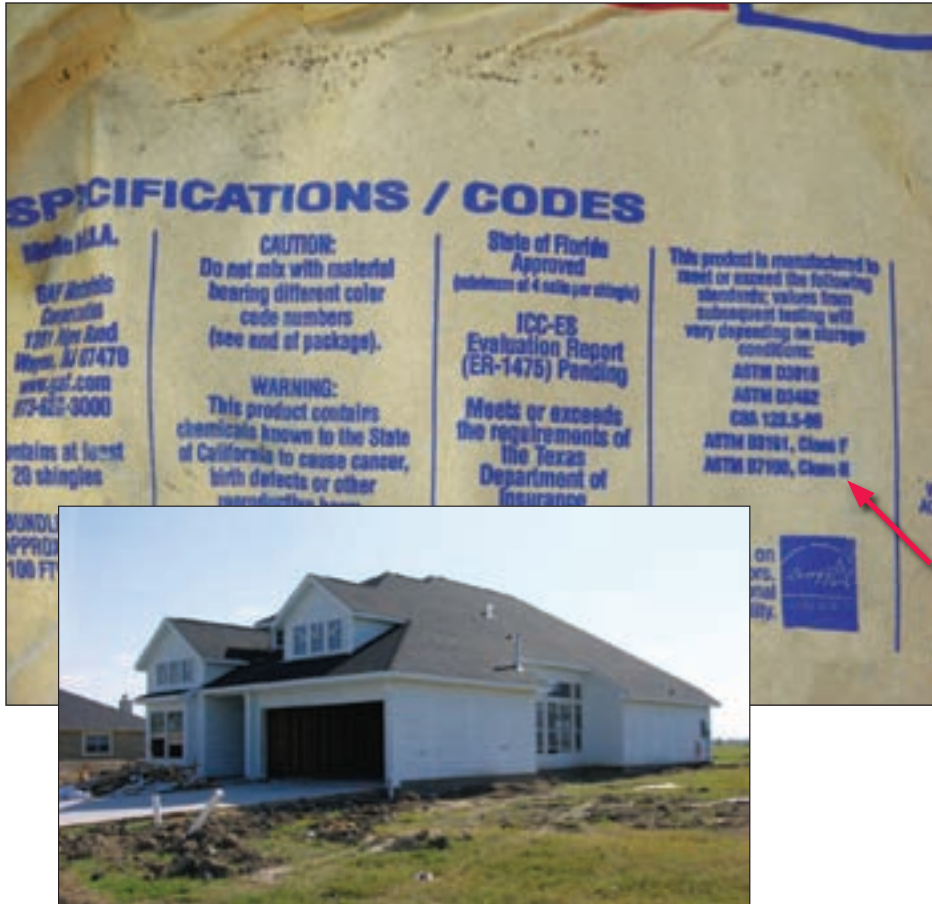
Figure 3-61. View of a shingle bundle wrapper at the Webster, TX, house shown in the inset. This shingle has a Class H rating (red arrow) (Hurricane Ike estimated wind speed in this area: 104 mph).
