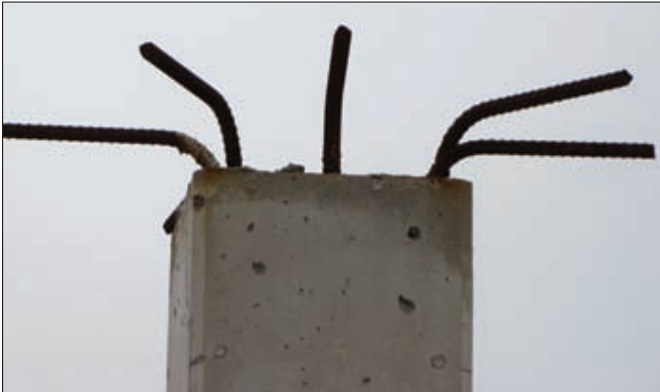
Figure 3-26. Reinforcing steel extending from the top of a concrete column (building under construction) (Galveston Island, TX)
