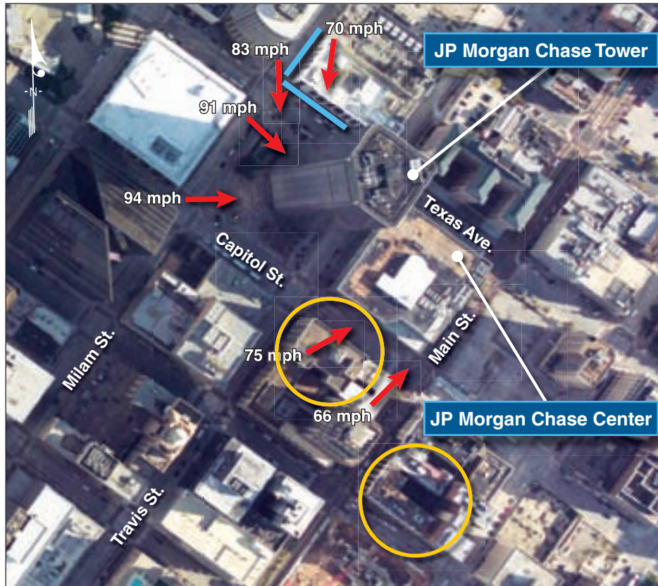
Figure 5-10. Locations of possible debris sources that impacted the JP Morgan Tower and Center. Aggregate-surfaced roofs within cluster A area shown by yellow circles. Blue lines show location of failed metal panel veneer.
