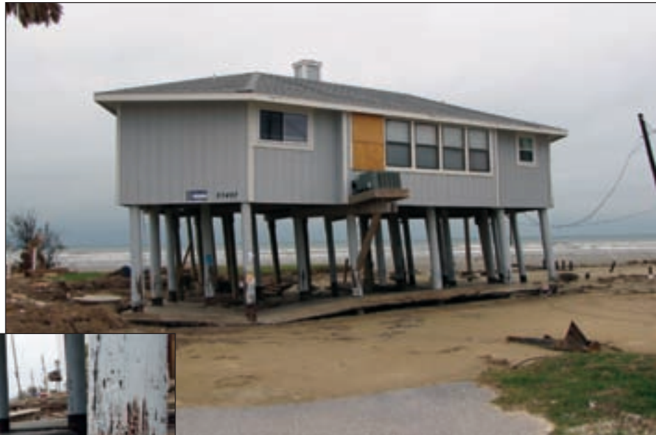
Figure 3-21. Failure of a timber pile foundation undermined by scour and erosion. Inset shows close-up of concrete slab failure and rotation of some of the foundation piles (Galveston Island, TX; Zone V).
