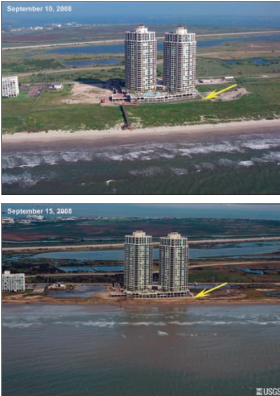
Figure 3-16. Pre- and post-Ike aerial photographs of the east end of Galveston Island, TX, illustrating some of the most significant loss of dunes and vegetation during Ike
