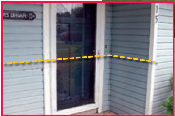
Figure 3-10. The Ike flood level reached approximately 3 feet above the floor slab (1 foot above the 6-foot BFE) of this Zone A house (see inset), which was reported to have been similarly inundated during Hurricane Rita. The MAT was told that the house will be elevated (Lake Charles, LA).
