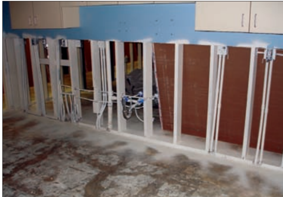
Figure 4-37. Hackberry Rural Medical Clinic interior repairs in progress
