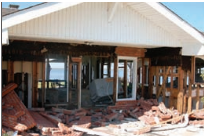
Figure 5. Hurricane Ike damage to buildings. The upper left and upper right photos are of buildings that were close to the Gulf of Mexico shoreline and subjected to storm surge and large waves above the lowest floor. The lower left photo is of a building close to Galveston Bay shoreline and subjected to storm surge and small waves. The lower right photo is of a Cameron Parish, Louisiana, school that was approximately 1.3 miles from the Gulf shoreline, but subjected to storm surge and small waves.
