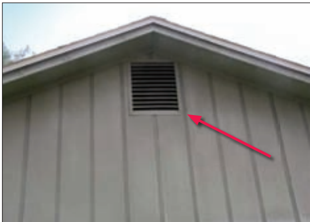
Figure 3-108. Gable end vent (red arrow)
