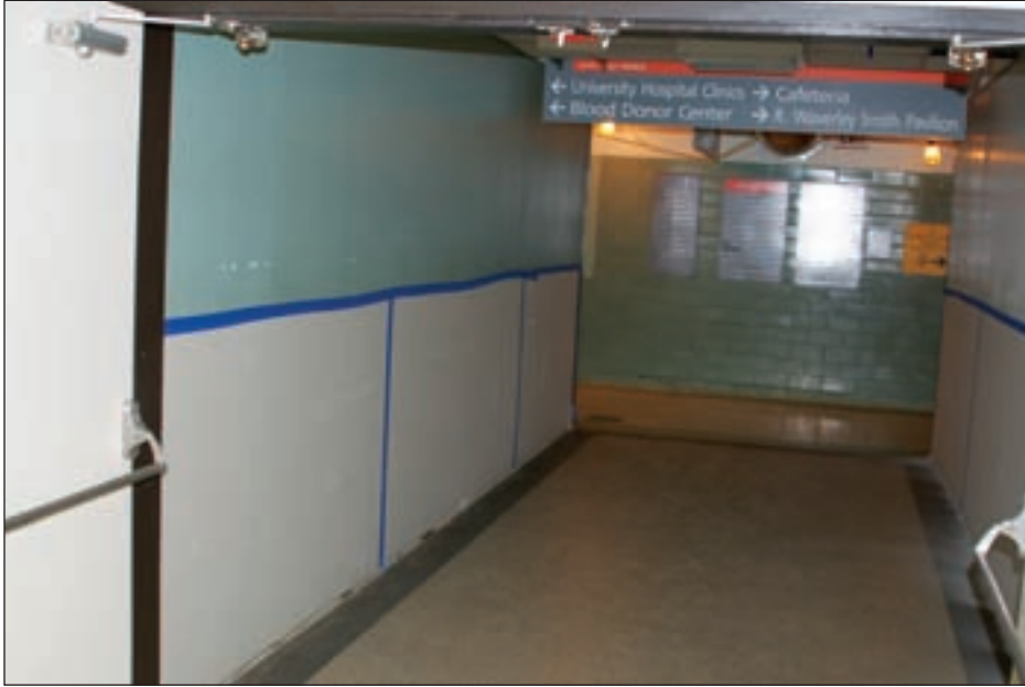
Figure 4-26. Replaced lower interior wall sections leading to UTMB Building 90
