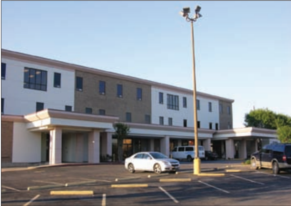
Figure 4-38. General view of Oceanview Transitional Care Center
