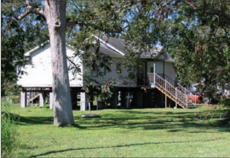
Figure 3-141. Zone A house elevated with Increased Cost of Compliance funds on masonry piers (Iberia Parish, LA). There was no evidence of pier reinforcement, mortar between masonry blocks, or ties between the piers and the elevated home.
