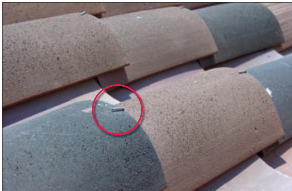
Figure 4-63. All of the tile tails were hooked
