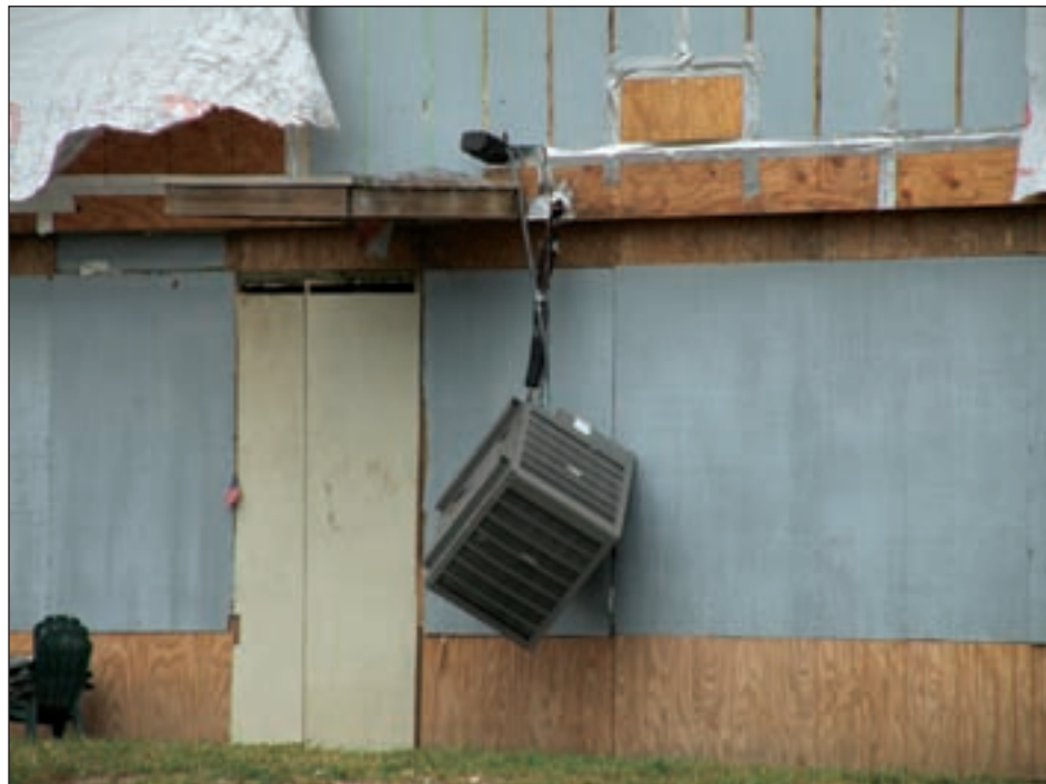
Figure 3-112. Improperly secured condensing unit was knocked from its platform (Kahala Beach, TX; Hurricane Ike estimated wind speed in this area: 80 mph, Exposure B)
