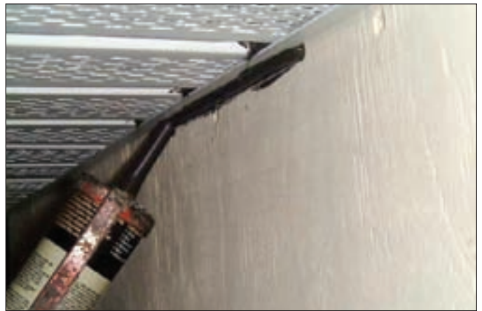
Figure 3. Applying a bead of sealant. (Note: Black sealant was used so that it would be visible in the photograph. Normally a matching sealant color would be used.)
