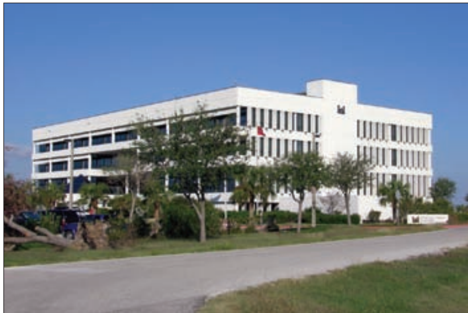
Figure 4-60. General view of the USACE Administration Building in Galveston, TX
