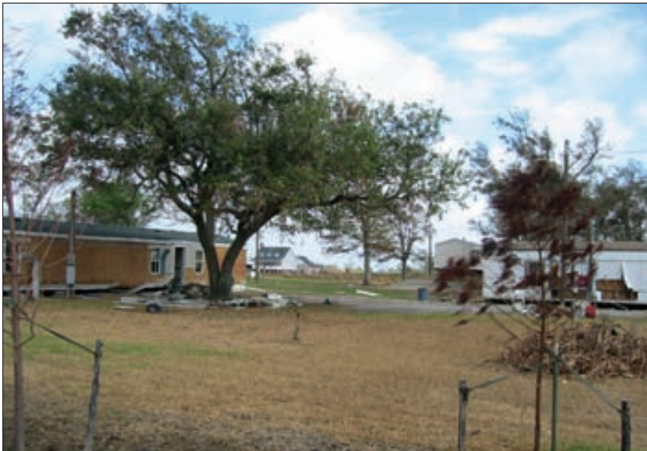
Figure 3-136. Two manufactured homes in Cameron, LA. Homes were displaced off foundations and siding peeled due to inundation and storm surge of approximately 4 feet above ground.
