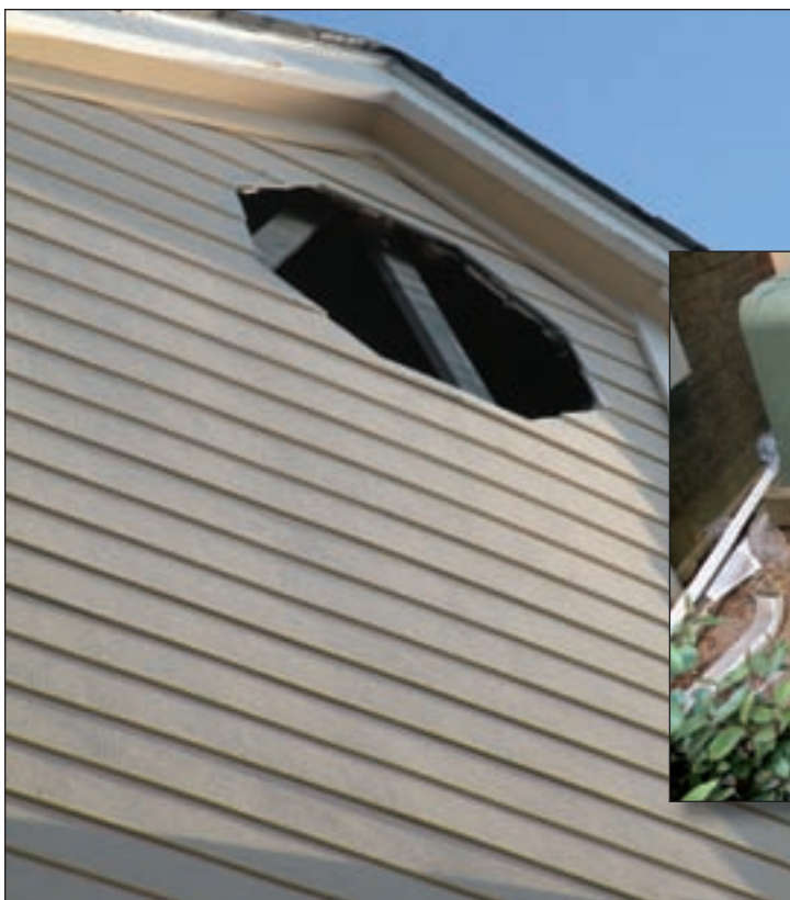
Figure 3-108. Gable end vent (red arrow)
