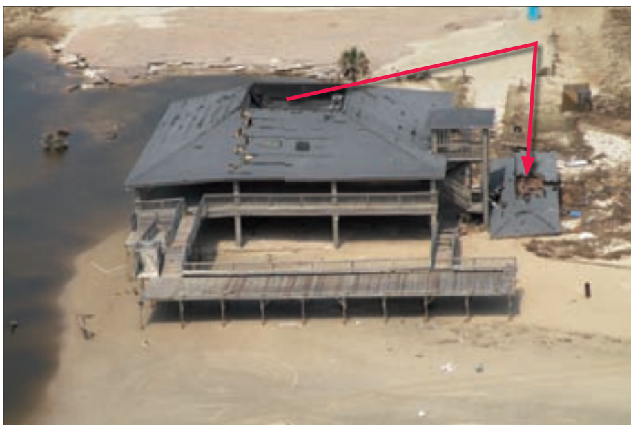
Figure 3-39. Galveston, TX, West End Beach house with roof structure removed by Hurricane Ike. The cause of the failure is unknown, but Ike wind speeds in this area were below design speeds (Hurricane Ike estimated wind speed in this area: 93 mph, Exposure C).
