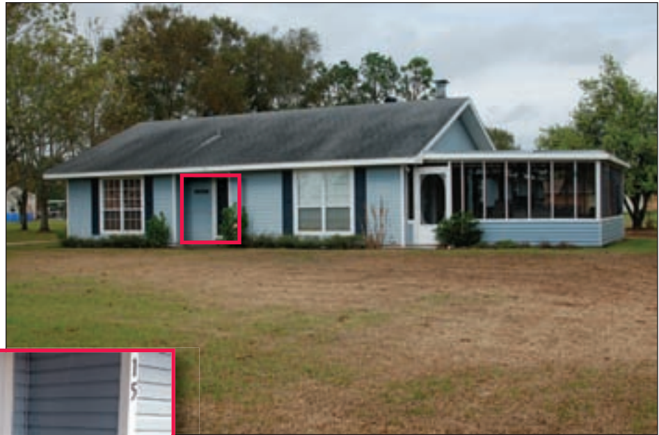
Figure 3-10. The Ike flood level reached approximately 3 feet above the floor slab (1 foot above the 6-foot BFE) of this Zone A house (see inset), which was reported to have been similarly inundated during Hurricane Rita. The MAT was told that the house will be elevated (Lake Charles, LA).
