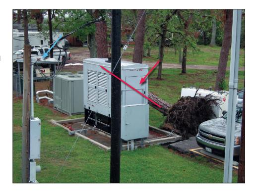
For critical facilities where a total loss of power for several days is tolerable (for instance, a community center that serves to house emergency workers brought in after a storm), it can be appropriate to save money and locate the generator outdoors. For facilities where loss of power is not tolerable (such as hospitals and EOCs), however, it is very unwise to place them outdoors or in enclosures that lack sufficient wind and windborne debris resistance.
