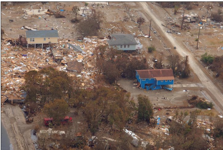
Figure 3-33. Roofs, walls, and other parts of destroyed houses washed landward to and inland of this location, approximately ½ mile from the Gulf shoreline of Bolivar Peninsula, TX
