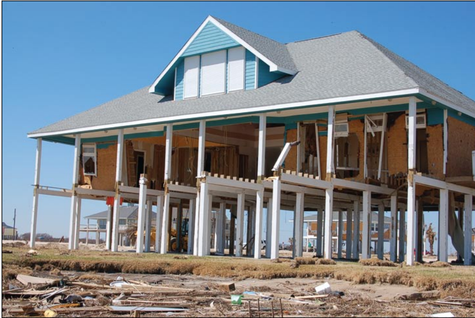
Figure 3-32. Seaward side of Zone V house struck by waves. The deck, the elevated floor system, and the seaward walls were destroyed or heavily damaged (Bolivar Peninsula, TX).
