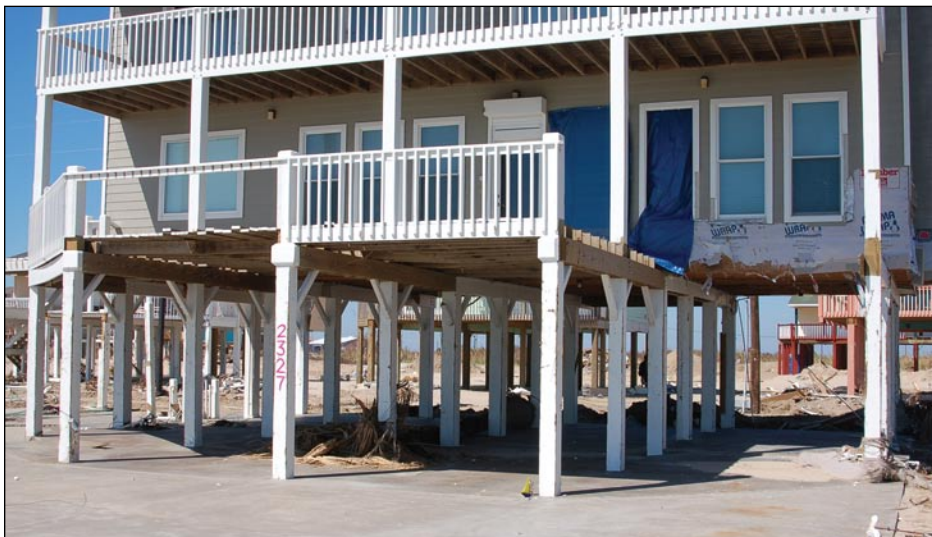
Figure 3-123. Typical concrete parking slab beneath a pile-supported house (Bolivar Peninsula, TX)
