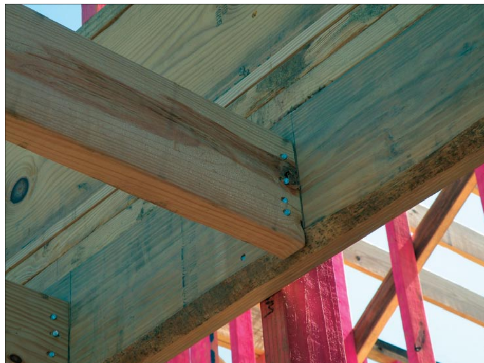
Figure 3-55. Toe-nailed connection of floor joists on band beam on house under construction. Floor joist should be installed using either galvanized metal joist hangers or ledger beams (LaPorte, TX).
