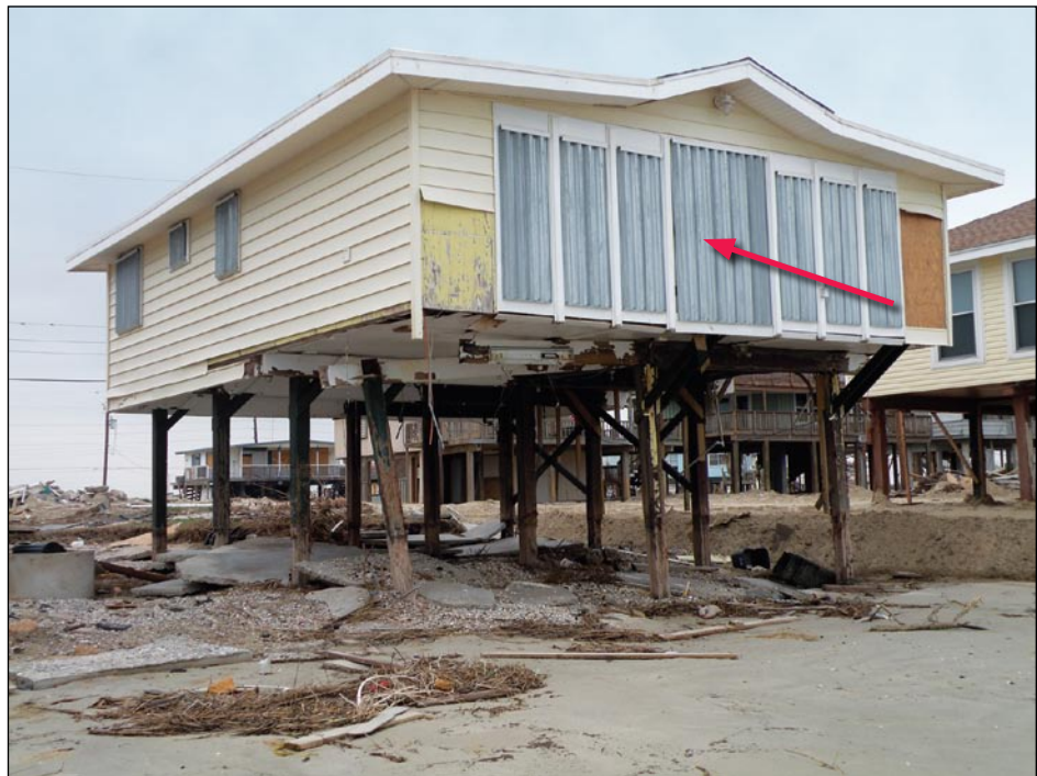
Figure 3-100. Corrugated metal shutters on house in West Galveston, TX (Hurricane Ike estimated wind speed in this area: 95 mph, Exposure C)
