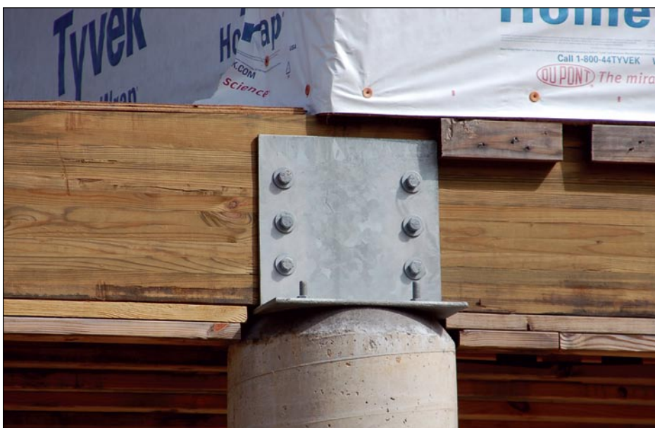
Figure 3-49. Strong concrete column-to-beam steel saddle connector
