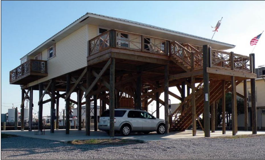
Figure 3-1. Louisiana house sufficiently elevated on a foundation that withstood Ike flood loads
