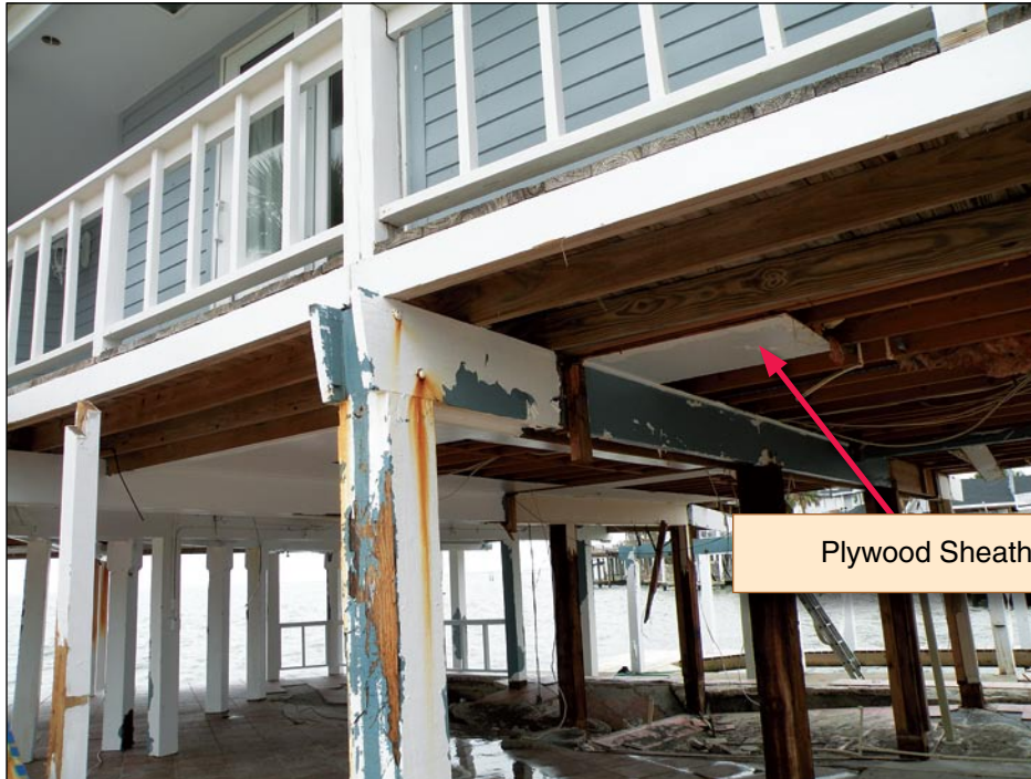
Figure 3-119. Plywood sheathing removed by storm surge (Jamaica Beach, TX, house on West Bay)
