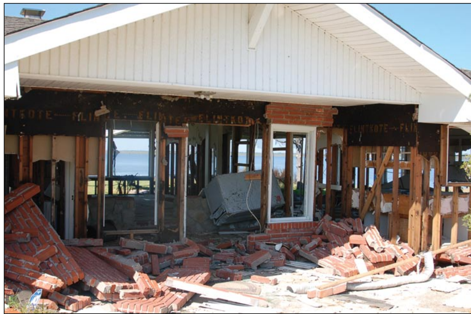
Figure 3-35. Damage to at-grade house in Zone V likely caused by wave and surge along the northern Galveston Bay shoreline in Baytown, TX
