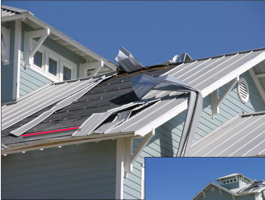
Figure 3-70. These architectural metal panels unlatched from the concealed clips. The red line shows location of the first row of clips (Galveston Island, TX; Hurricane Ike estimated wind speed in this area: 110 mph).
