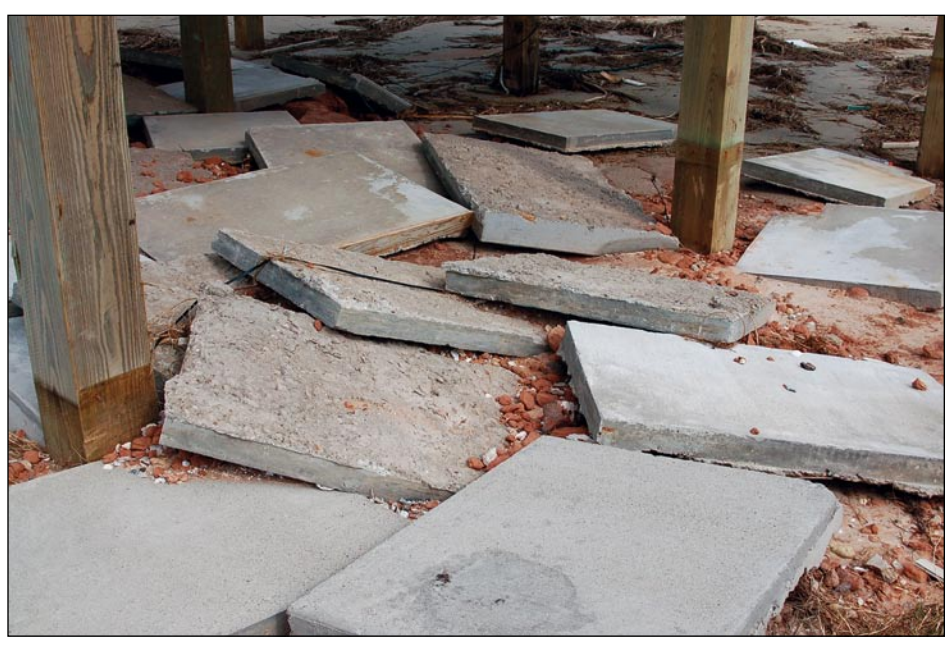
Figure 3-129. Thin, unreinforced parking slab sections separated when undermined and collapsed in place, with no apparent adverse impact to the foundation (Galveston Island, TX)
