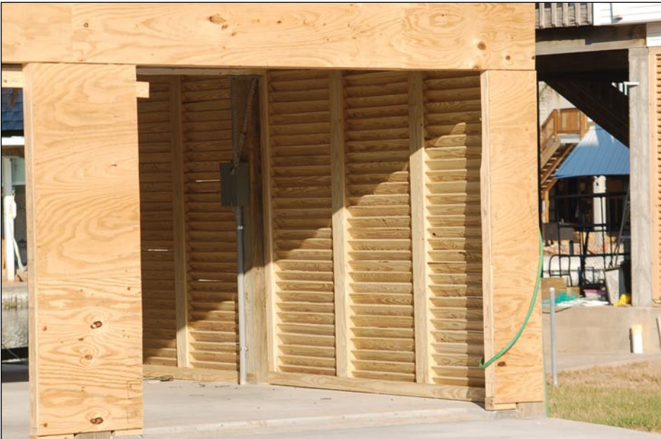
Figure 3-118. Solid breakaway walls lost during Ike are being replaced with louvered panels (Tiki Island, TX)
