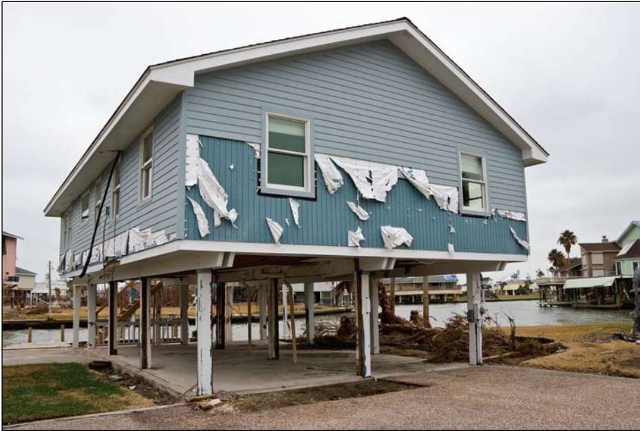
Figure 3-88. Fiber cement lap siding was blown off this West Bay, Galveston Island, TX, house (Hurricane Ike estimated wind speed in this area: 100 mph, Exposure B)
