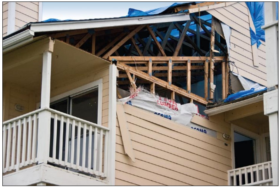
Figure 3-76. Loss of fiberboard sheathing and fiber cement siding from gable end wall of an apartment complex (West Bay, Galveston Island, TX; Hurricane Ike estimated wind speed in this area: 90 mph, Exposure B)
