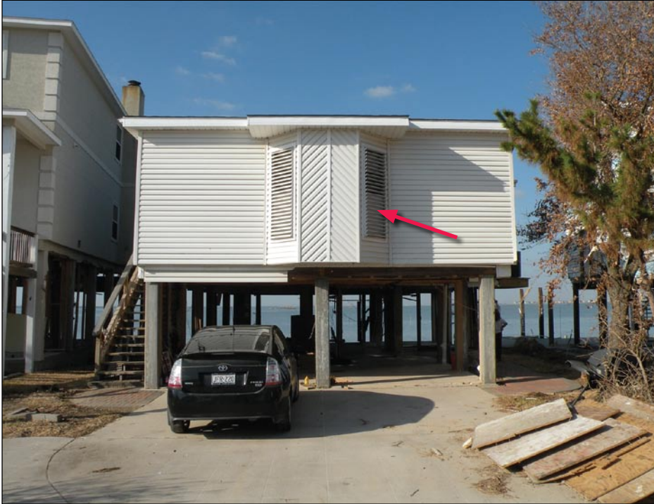
Figure 3-97. Tiki Island, TX, house with adjustable shutters (Hurricane Ike estimated wind speed in this area: 103 mph, Exposure C)
