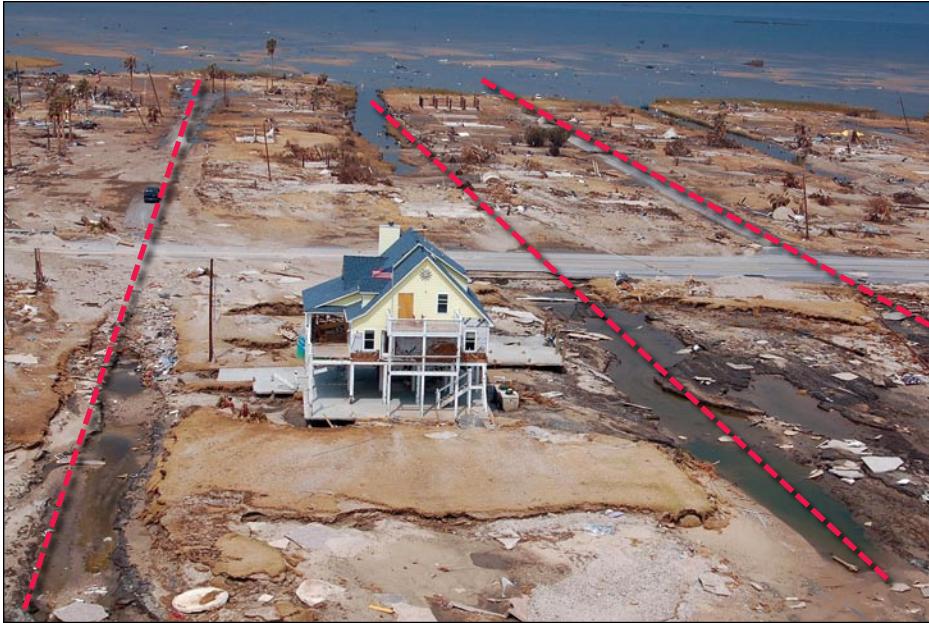
Figure 3-22. Linear scour features tend to align with canals and roads as storm surge returns to the Gulf. Houses such as this one were fortunate not to be undermined and lost during Ike, as many homes undoubtedly were (Bolivar Peninsula, TX).
