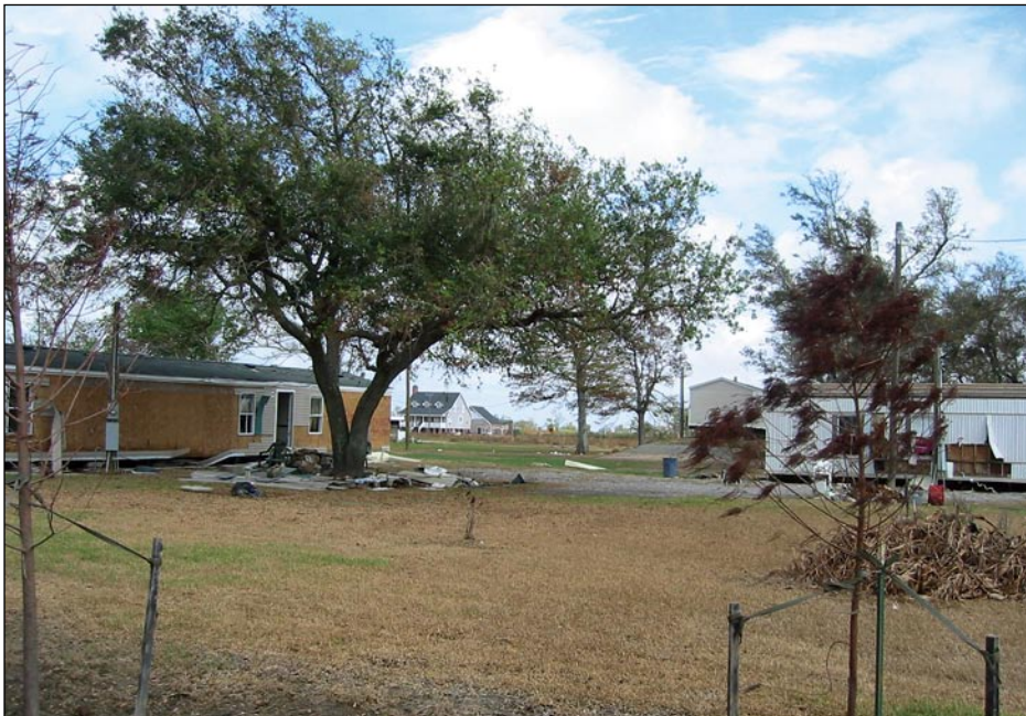
Figure 3-136. Two manufactured homes in Cameron, LA. Homes were displaced off foundations and siding peeled due to inundation and storm surge of approximately 4 feet above ground.
