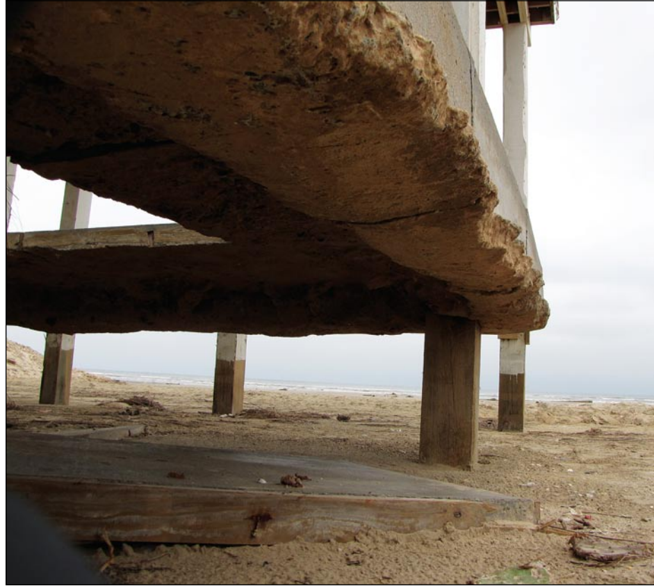
Figure 3-125. Pile-founded house with a slab thickened to create grade beams. The unthickened portion of the slab collapsed when undermined (Galveston Island, TX).
