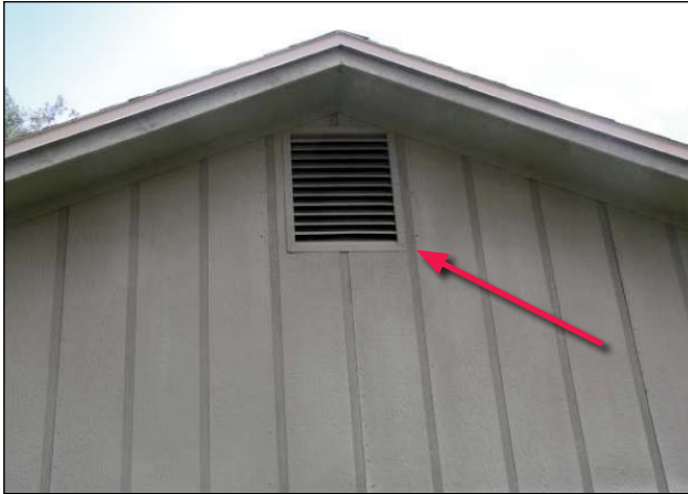
Figure 3-108. Gable end vent (red arrow)
