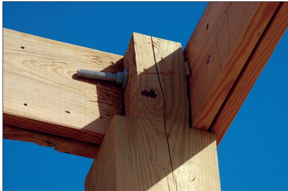
Figure 3-51. Poor beam connection to corner column
