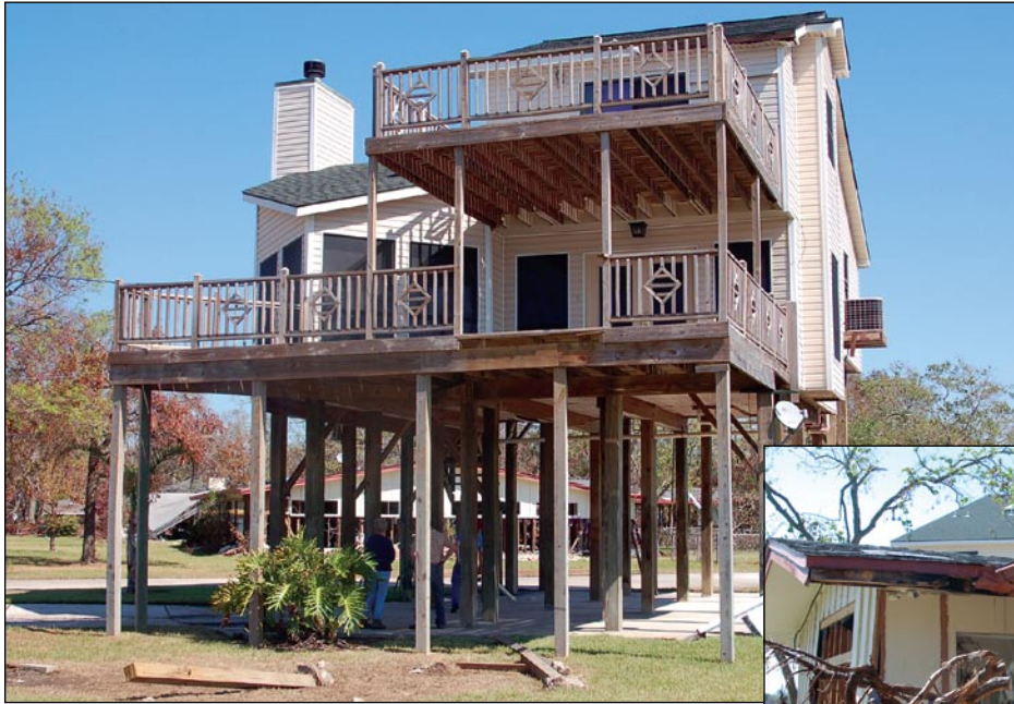
Figure 3-8. This elevated house (Zone V, BFE = 15 feet) suffered no significant damage due to flooding. The nearby at-grade house in the background, shown in the inset, was heavily damaged (Baytown, TX).
