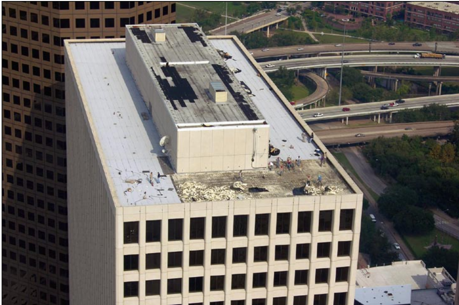
Figure 5-28. Roof covering damage on the main and penthouse roofs of building B-1
