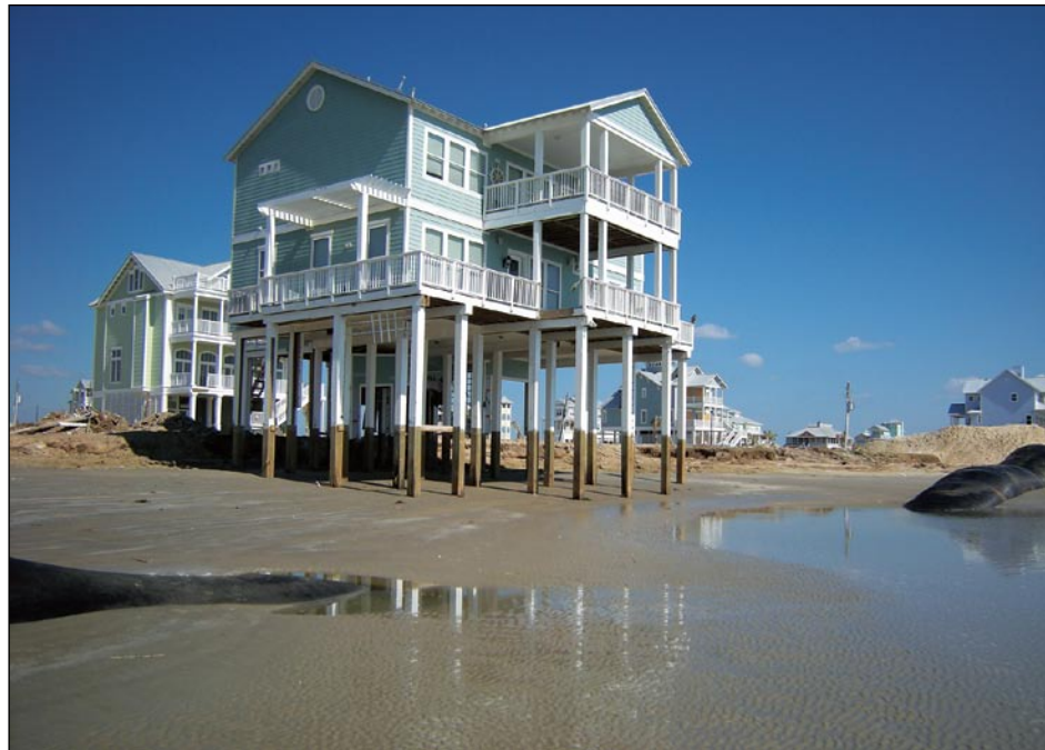
Figure 8-3. Broken geotextile tube at Beachside Drive, Galveston Island, TX
