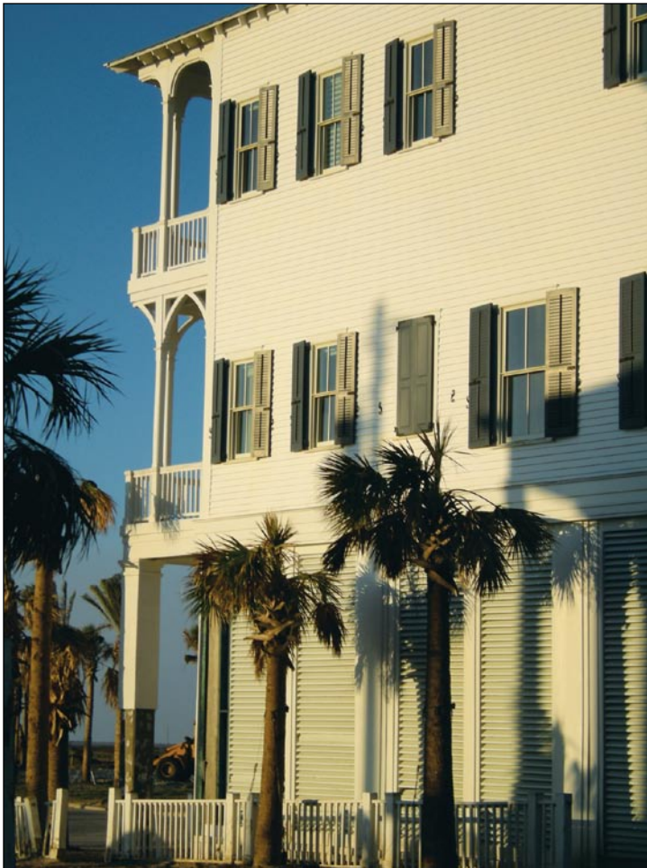
Figure 8-6. Beachtown, TX, under construction
