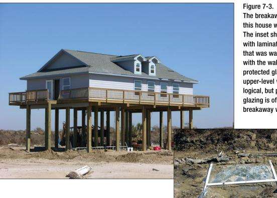
The breakaway walls at this house were destroyed. The inset shows a window with laminated glazing that was washed away with the walls. Using protected glazing on the upper-level windows is logical, but protected glazing is of little value in breakaway walls.
