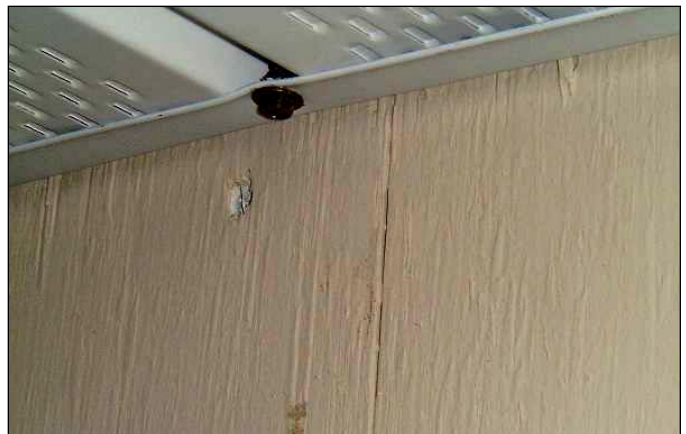
Figure 5. Screws through wall channel.
