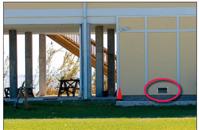
Figure 5. Flood opening in a below-BFE enclosure wall.
