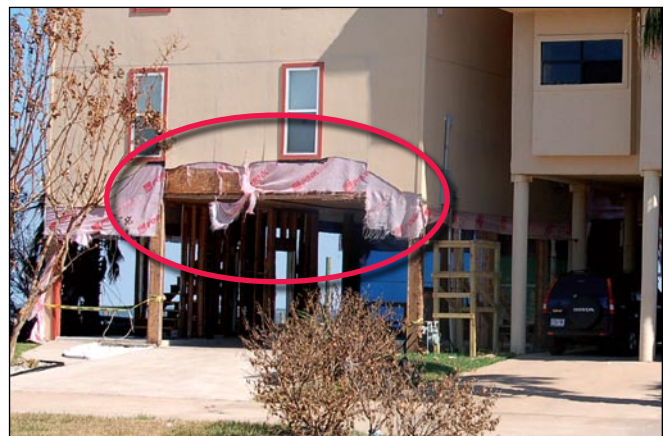
Figure 3. NFIP-compliant breakaway wall construction.
