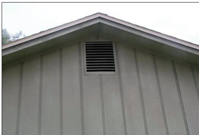
Figure 9. Gable end vent.
