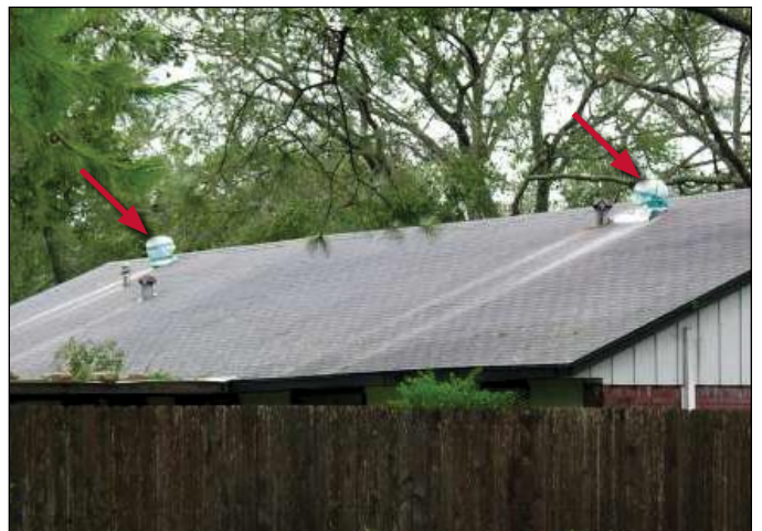
Figure 14. Plastic wrapped turbine.
