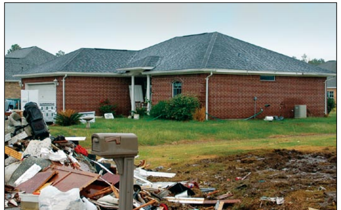
Figure 1. Bridge City, TX, homes were flooded during Ike, even though they were constructed outside the SFHA and in Zone B. The flood level was approximately 4' above the closest BFE.
