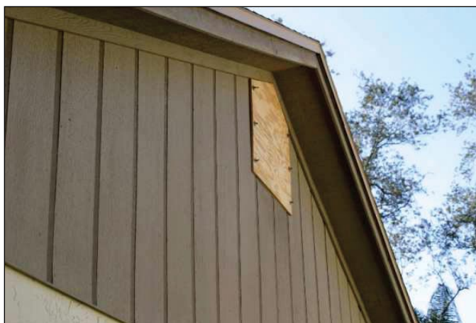
Figure 10. Shuttered gable end vent.
