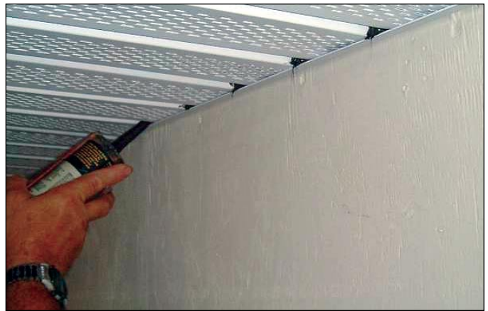
Figure 4. Applying dabs of sealant.
