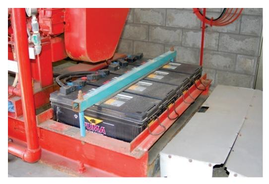
Figure 6.4.7.4-3 Batteries anchored with equipment skid (Photo courtesy of Eduardo Fierro, BFP Engineers).
