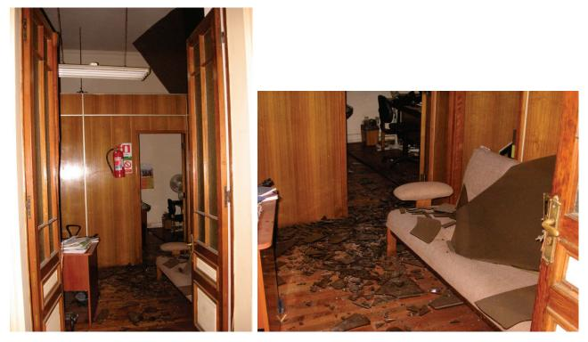
Figure 6.3.2.3-1 Glass shards fallen from the top of partial height office partitions in the reception area during the magnitude-8.8 2010 Chile Earthquake (Photo courtesy of Rodrigo Retamales, Rubén Boroschek & Associates).
