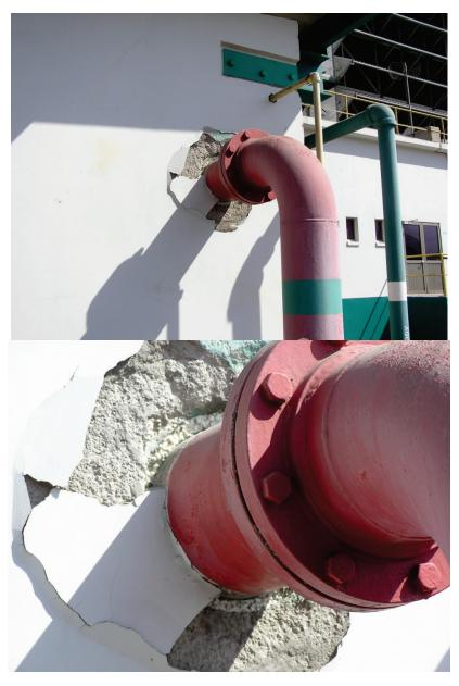
Figure 6.4.3.8-2 Exterior stucco damage at wall penetration for fire protection piping in the 2001 magnitude-8.4 Peru Earthquake (Photos courtesy of Eduardo Fierro, : BFP Engineers).
