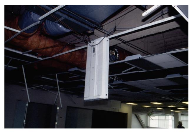
Figure 6.4.9.1-3 Light fixture without adequate independent support dangling along one edge from ceiling grid, damaged in the 1994 magnitude-6.7 Northridge Earthquake (Photo courtesy of Degenkolb Engineers).
