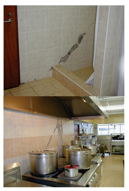
Figure 6.3.3.1-2 Damage to adhered tile veneer in locker room and kitchen at industrial facility in the 2001 Peru Earthquake (Photo courtesy of Eduardo Fierro, BFP Engineers). Tile was adhered to CMU partitions which were built integral with the concrete frame. While only a limited number of tiles were broken, equipment had to be disconnected and many tiles removed to repair cracks in the wall and facilitate the repair of the veneer.
