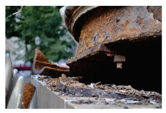
Figure 6.5.6.3-2 Leaning fountain after the 2010 Chile Earthquake; corrosion was a factor (Photos courtesy of Eduardo Fierro, BFP Engineers).
