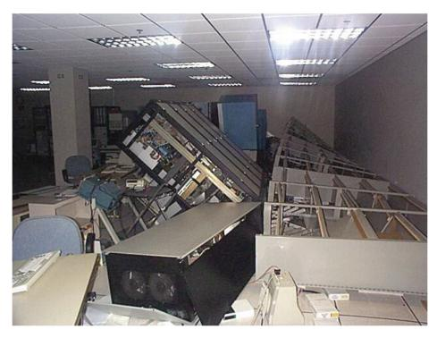
Figure 6.5.3.2-1 Damage to communication and computer racks (Photo courtesy of Degenkolb Engineers).
