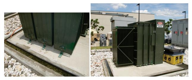
Figure 6.4.7.3-5 Outdoor liquid type electrical power transformer which converts incoming medium voltage to 480 volt utilization voltage for critical facility. Note use of manufacturer supplied diagonal elements on cooling fin assembly to minimize dynamic loading on liquid filled fin assembly which contains numerous welded connections. Post earthquake photo from the 2010 M 7.0 Haiti Earthquake (photos courtesy of Philip J. Caldwell).
