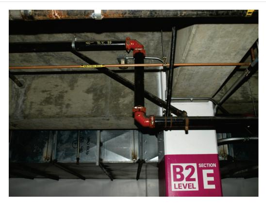
Figure 6.4.4.1-9 Transverse and longitudinal restraints on fire protection distribution line (Photo courtesy of Cynthia Perry, BFP Engineers).
