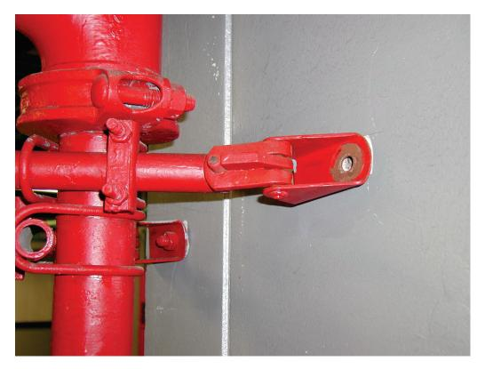
Figure 6.4.4.1-2 Wall-mounted pipe restraint failed due to inadequate connection to structural framing in the 2001 magnitude-8.4 Peru Earthquake (Photo courtesy of Eduardo Fierro, BFP Engineers).
