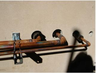
Figure 6.4.3.7-3 Wall-mounted pipe restraint examples using standard strut shapes and connectors (Photo courtesy of Cynthia Perry, BFP Engineers). Bottom view still under construction; pipes temporarily attached with plastic ties.
