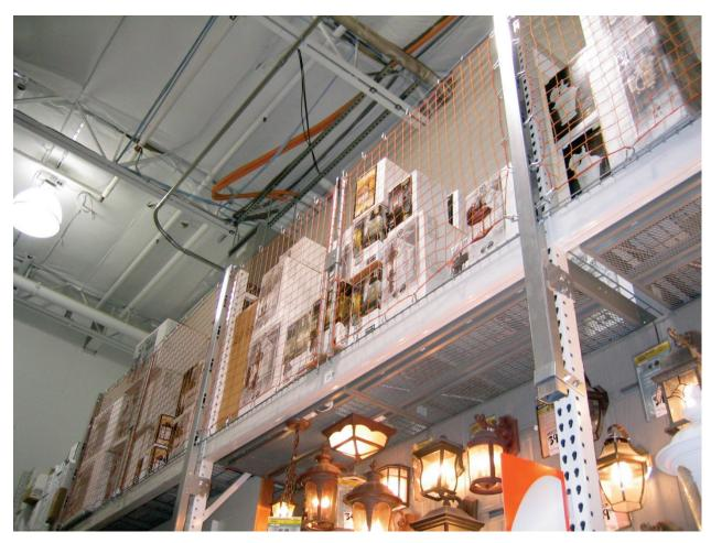
Figure 6.5.1.2-6 Photo showing netting used to keep storage on upper portions of steel storage racks in a big box hardware store (Photo courtesy of Mike Mahoney, FEMA).
