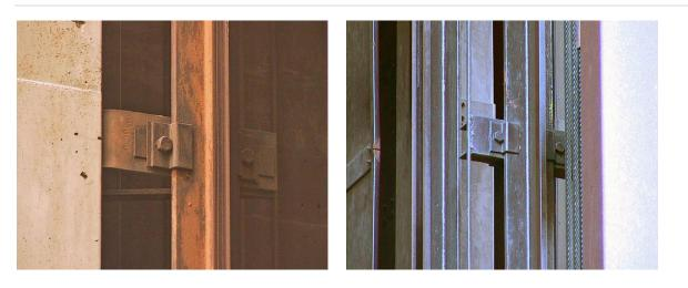
Figure 6.4.10.2-2 Examples of brackets and clips attaching the elevator guide rails to the structure (Photo courtesy of Eduardo Miranda, Stanford University).
