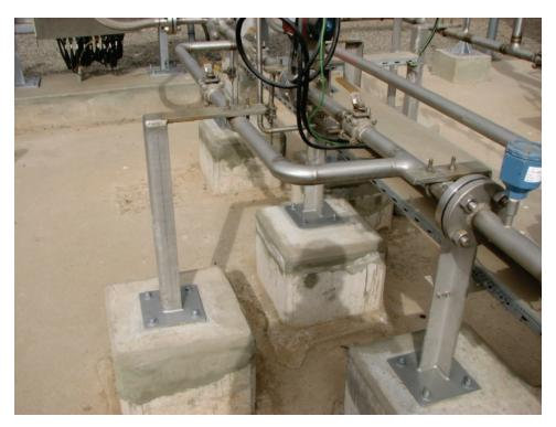
Figure 6.4.3.5-4 Floor/ground-mounted supports for industrial piping in Chile; piping undamaged in the 2010 magnitude-8.8 Chile Earthquake. Pipe supports include concrete pedestal, base plate, and built-up welded support stand. (Photos courtesy of Antonio Iruretagoyena, Rubén Boroschek & Associates).
