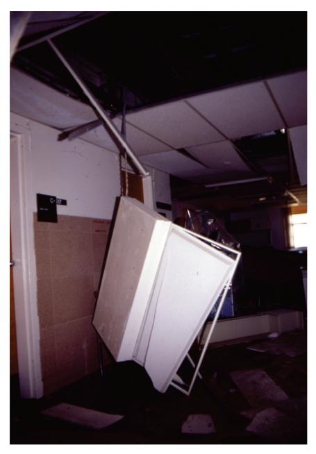
Figure 6.4.9.1-4 Light fixture without independent support dangling from conduit as a result of the 1994 Northridge Earthquake (Photo courtesy of Degenkolb Engineers).
