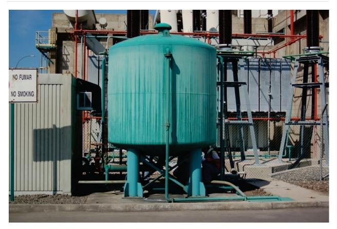
Figure 6.4.2.1-7 Gusset plates and cross bracing added at base of vertical tank on four legs following the 2001 magnitude-8.4 Peru Earthquake (Photo courtesy of Eduardo Fierro, BFP Engineers).
