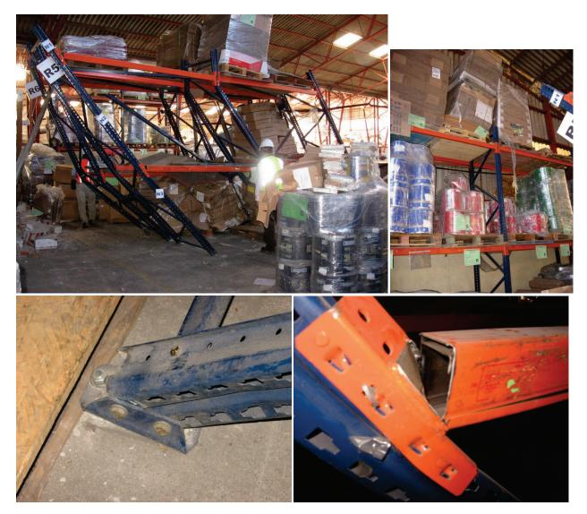
Figure 6.5.1.2-4 Failure of anchored racks in the 2010 magnitude-8.8 Chile Earthquake. The racks are leaning precariously due to inadequate bracing in the longitudinal direction and weak connections between the components. The welded fitting at the end of the beam failed at the weld in many places. Note that most items were shrink wrapped so merchandise did not scatter (Photos courtesy of Rodrigo Retamales, Rubén Boroschek & Associates).
