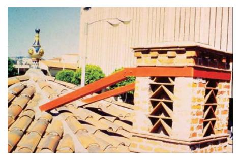
Figure 6.3.7.1-4 Braced chimney (FEMA, 2004).
