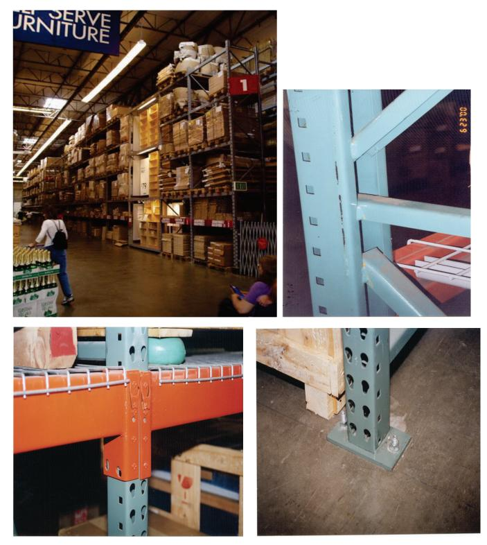
Figure 6.5.1.2-5 Typical pallet storage rack configuration and details (Photos courtesy of Maryann Phipps, Estructure).
