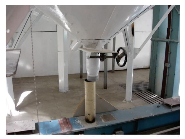
Figure 6.4.11.1-1 Misalignment between rice storage hopper and conveyor following the 2010 magnitude-8.8 Chile Earthquake (Photo courtesy of Rodrigo Retamales, Rubén Boroschek & Associates). Where various system components interface with a conveyor, the seismic restraints for the various parts should be coordinated to maintain alignment following an earthquake.
