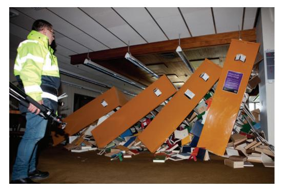
Figure 6.5.2.2-1Photo showing collapsed library shelving in the 2010 magnitude-7.1 Canterbury<br/>New Zealand Earthquake (Photo courtesy of University of Canterbury).
