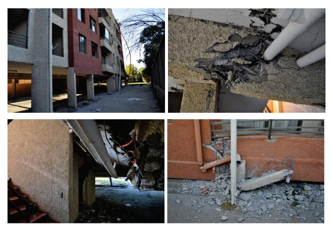
Figure 6.4.5.2-3 Photos displaying resilience of piping systems; this building suffered a partial structural collapse along one side in the 2010 Chile Earthquake. The only broken pipe (shown at lower right) was along the collapsed side; the other piping had broken pipe supports in some locations but the joints remained largely intact, even with these very large deformations (Photos courtesy of Eduardo Fierro, BFP Engineers).
