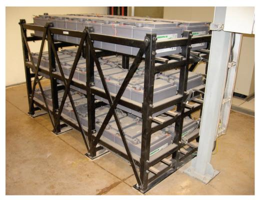
Figure 6.4.7.4-4 Battery rack that performed well in the 2010 magnitude-8.8 Chile Earthquake (Photo courtesy of Rodrigo Retamales, Rubén Boroschek & Associates).
