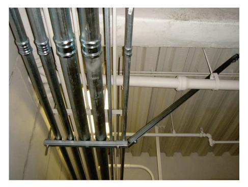
Figure 6.4.8.1-2 Rigid strut bracing provides restraint against earthquake forces perpendicular to the piping. Similar bracing is required in the direction parallel to the conduit (Photo courtesy of Maryann Phipps, Estructure).
