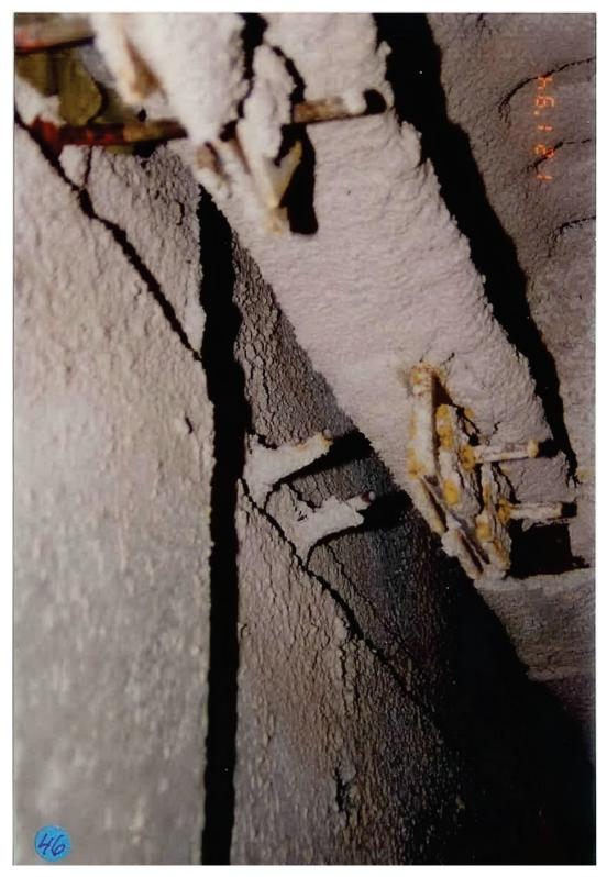
Figure 6.3.1.3-5 Close-up photo of two fractured connection bolts in a prefabricated panel in the 1994 Northridge Earthquake; corrosion of the rods may have contributed to the failure. (Photo courtesy of OSHPD).
