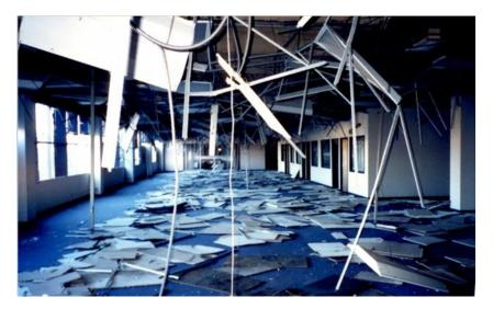
Figure 2.4.2-1 Complete loss of suspended ceilings and light fixtures in the 1994 Northridge Earthquake (FEMA 74, 1994).
