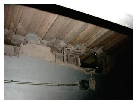
Figure 6.3.2.1-1 Damage along the top of a reinforced concrete masonry unit partition built flush with soffit of metal deck at an industrial facility in the 2001 magnitude-8.4 Peru Earthquake (Photo courtesy of Eduardo Fierro, BFP Engineers).
