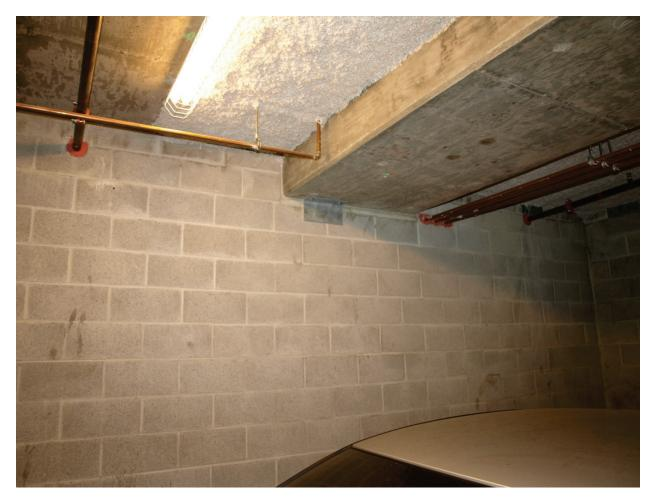
Figure 6.4.3.8-6 Series of pipe penetrations through a full-height CMU partition wall. Note pipe suspended from floor above; partition anchored to floor below and detailed with steel clip angles intended to provide lateral restraint for the wall but allow relative slip between the wall and slab above. The hangers will move with the floor above and the pipe at penetration will move with the wall. Lateral restraints are located immediately above floor (Photo courtesy Cynthia Perry, BFP Engineers).
