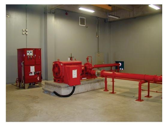
Figure 6.4.4.1-8 There was no damage to the *fire suppression equipment in this control room in the 2001 Peru Earthquake because the pump and the control panel were well anchored and the piping had flexible connections with adequate sized wall penetration and no overhead falling hazards (Photo courtesy of Eduardo Fierro, BFP Engineers).*
