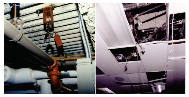
Figure 6.4.4.1-3 Damage to suspended fire protection piping from the 1994 Northridge Earthquake. Failed vibration isolators at left; failed C-clamps without beam clamp restraining straps shown at right (Photos courtesy of Mason Industries).
