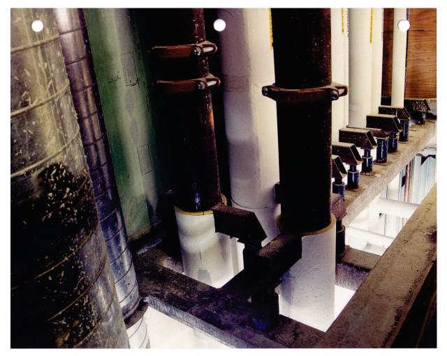
Figure 6.4.3.4-2 Riser supports provide lateral restraint with vertical sliding guides that allow thermal movement; restraint hardware consisting of tube sections is welded to either side of pipe (Photo courtesy of Mason Industries).
