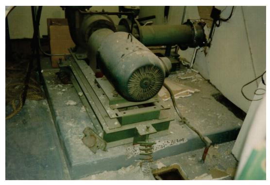
Figure 6.4.1.3-2 Failure of pump mounted on three vibration isolators and damage at wall penetration (Photo courtesy of Mason Industries).
