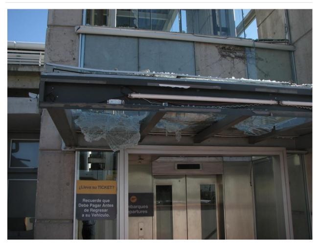
Figure 6.4.10.2-10 Glazing failures caused additional hazards at Santiago airport elevator in the 2010 Chile Earthquake (Photo courtesy of Antonio Iruretagoyena, Rubén Borsochek & Associates).
