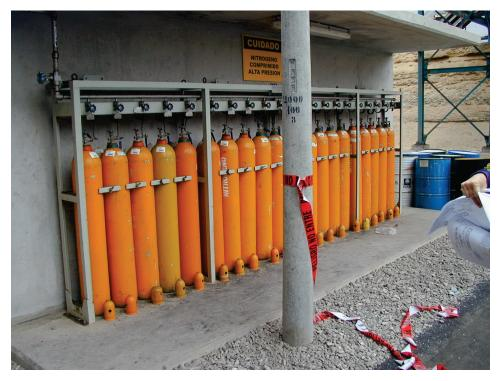
Figure 6.4.2.3-2 Gas cylinder anchorage with attached gas lines undamaged in the 2001 magnitude-8.4 Peru Earthquake (Photo courtesy of Eduardo Fierro, BFP Engineers).
