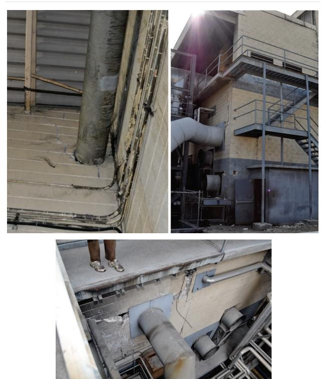
Figure 6.4.3.8-3 Wall penetrations for piping and ducts contributed to damage to unreinforced masonry walls at an industrial facility in the 2010 magnitude-7 Haiti Earthquake (Photos courtesy of Eduardo Fierro, BFP Engineers). The piping and ducts were not damaged but the walls cracked and will need to be repaired.
