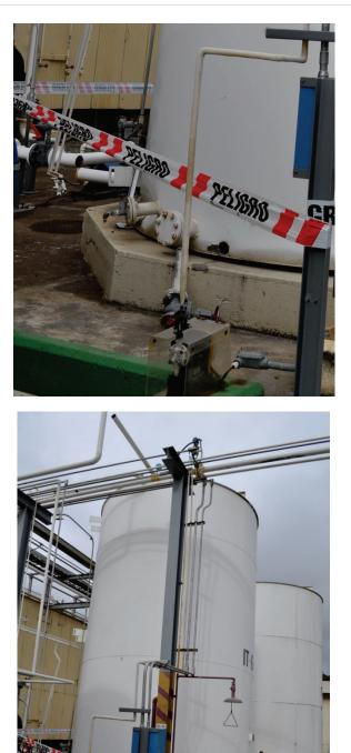
Figure 6.4.5.1-3 Elephant foot damage to inadequately anchored fuel tank in the 2010 Chile Earthquake also resulted in damage to fuel lines. Close-up photo shows failed pipe at welded joint (left) and pipe segment with attached valve (foreground) tore out of the tank wall (Photos courtesy of Eduardo Fierro, BFP Engineers).
