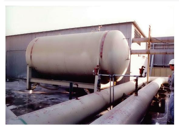
Figure 6.4.2.1-3 Horizontal tank strapped to structural support frame on hospital roof; one strap failed and tank slid six inches in the 1994 Northridge Earthquake (Photo courtesy of OSHPD).
