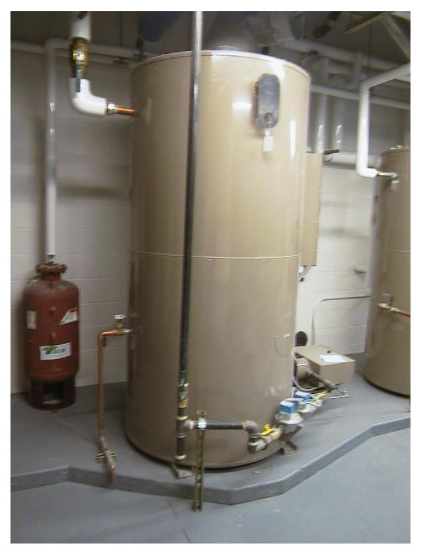
Figure 6.4.2.4-5 Base-mounted water heater located in a school; equipment supplied with metal base for mounting (Photo courtesy of EQE for the Salt Lake City School District).
