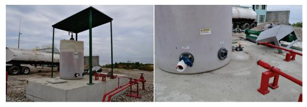
Figure 6.4.4.1-5 Unanchored holding tank slid on concrete pad, breaking fire protection piping and disabling the fire protection system in the 2010 Haiti Earthquake. In this case, the piping was well anchored but the tank was unrestrained (Photo courtesy of Eduardo Fierro, BFP Engineers).
