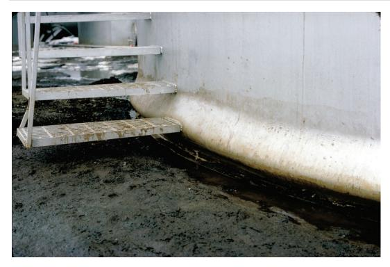
Figure 6.4.2.2-2 Tank with "elephant's foot" buckle at the base in the 1964 magnitude-9.2 Anchorage, Alaska earthquake (Photo courtesy of PEER, Steinbrugge Collection, No. S2508)
