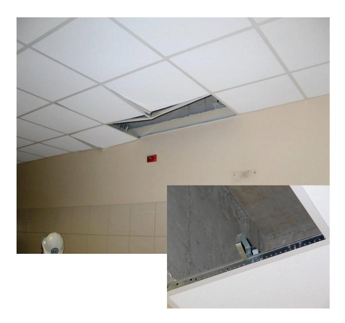
Figure 6.3.4.1-4 Fallen ceiling tiles at Talca Hospital in the 2010 Chile Earthquake, in spite of the use of clips as shown in detail at right. Most ceilings observed in Chile did not have seismic detailing (Photos courtesy of Bill Holmes, Rutherford & Chekene).
