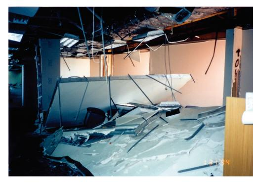
Figure 6.3.2.2-1 Out-of-plane failure of inadequately braced partial height metal stud partitions in the 1994 Northridge Earthquake (Photo courtesy of Wiss, Janney, Elstner Associates).
