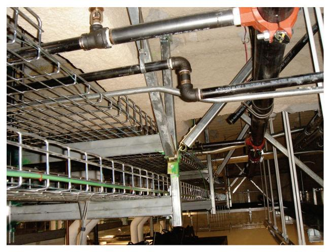
Figure 6.4.8.1-4 Lateral and longitudinal rigid strut bracing for trapeze supporting electrical raceways (Photo courtesy of Maryann Phipps, Estructure).
