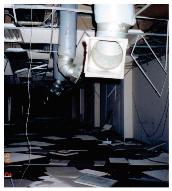
Figure 6.4.6.2-1 Air diffusers fell to the floor; ducts hanging through ceiling grid as a result of the 1994 Northridge Earthquake (FEMA 74, 1994).
