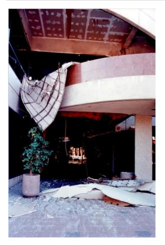
Figure 2.4.1-4 Failure of heavy stucco soffit at building entrance in the 1994 Northridge Earthquake (FEMA 74, 1994).
