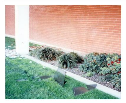
Figure 2.4.1-2Shards of broken untempered glass that fell several stories from a multistory<br/>building in the 1994 Northridge Earthquake. Failures of this type can be very<br/>hazardous, especially if glazing is located above exit ways (FEMA 74, 1994).
