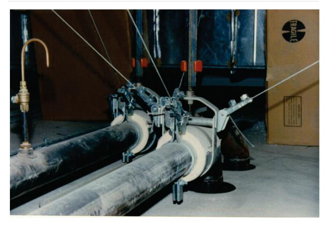
Figure 6.4.3.8-5 Floor penetration with oversized opening and vertical and lateral restraints immediately above floor (Photo courtesy of Mason Industries).
