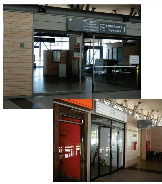
Figure 6.3.2.3-2 Damage to glazed doors at the Concepción airport in the 2010 Chile Earthquake. In the top photo the glazing in the sliding glass door shattered; in the lower photo the glass is intact but the door frames are misaligned (Photos courtesy of Rodrigo Retamales, Rubén Boroschek & Associates). Available at: http://www.fema.gov/earthquake-publications/fema-e-74-reducing-risks-nonstructural-earthquake-damage Last Modified: December 2012
