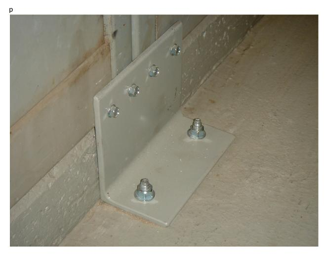
Figure 6.4.7.1-10 Detail of cabinet base anchorage (Photo courtesy of Maryann Phipps, Estructure).
