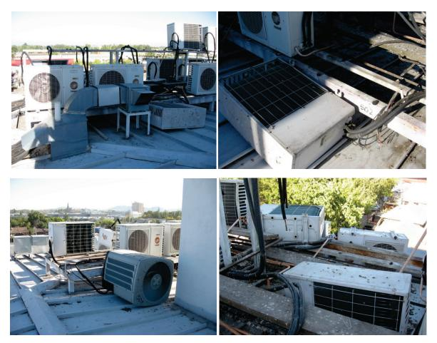
Figure 6.4.1.4-3 Numerous poorly anchored rooftop units toppled in the 2010 Chile Earthquake (Photos courtesy of Rodrigo Retamales, Rubén Boroschek & Associates).
