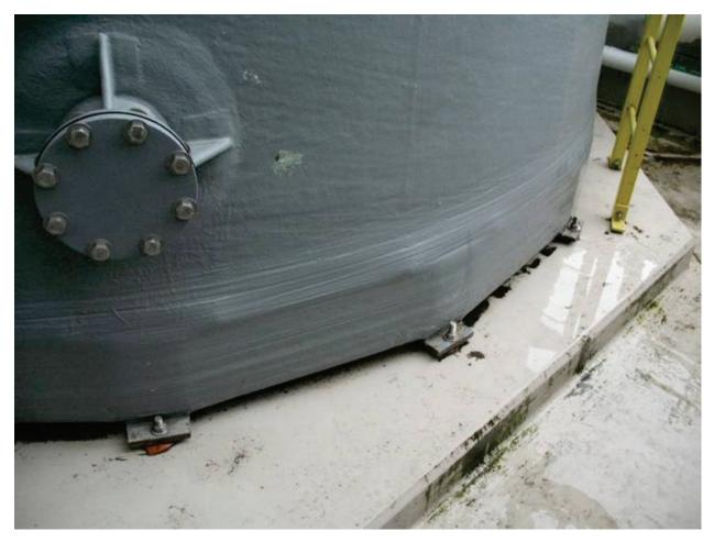
Figure 6.4.2.2-6 Anchors at base of fiberglass reinforced plastic tank (Photo courtesy of Jeffrey Soulages, Intel).
