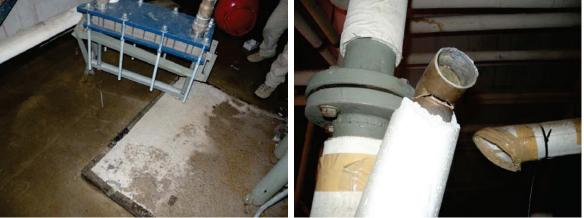
Figure 6.4.5.2-1 Broken copper hot water piping for at the San Carlos Hospital in the 2010 Chile Earthquake. Piping failure caused by movement of inadequately braced boiler shown at left (Photos courtesy of Gilberto Mosqueda, SUNY Buffalo).
