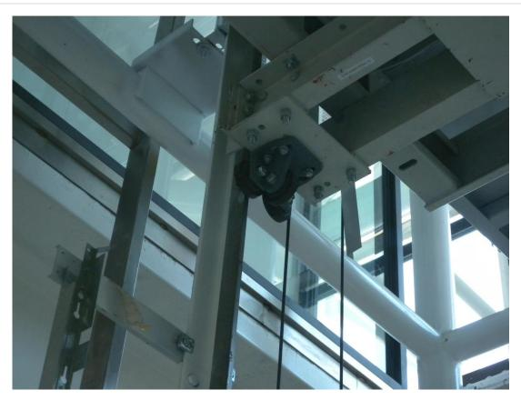
Figure 6.4.10.2-9 Derailed car roller assembly of the guide rail at the Santiago airport in the 2010 Chile Earthquake (Photo courtesy of Gilberto Mosqueda, SUNY Buffalo). The three rollers are supposed to travel along three sides of the stem of the T-shaped steel guide rail.
