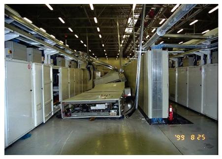
Figure 6.4.7.1-2Unanchored electrical cabinets overturned in a paper products plant during the<br/>1999 magnitude-7.4 lzmit, Turkey earthquake (Photo courtesy of NISEE lzmit<br/>Collection, No. IZT-682, photograph by Halil Sezen).
