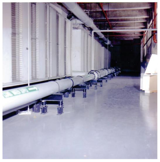
Figure 6.4.3.5-3 Floor-mounted supports for insulated pipe with vibration isolation (Photo courtesy of Mason Industries).
