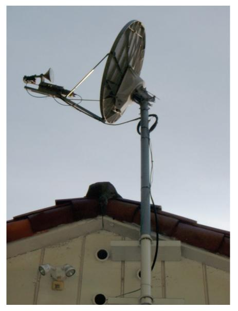
Figure 6.4.7.6-6 Antenna mast mounted to wood stud wall using blocking to clear eves (Photo courtesy of Cynthia Perry, BFP Engineers).
