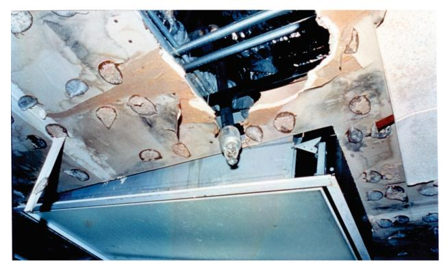
Figure 6.4.4.1-1 Sprinkler pipe ruptured at the elbow joint due to differential motion within the ceiling plenum. Water leakage from broken fire sprinklers and water lines contributed to the decision to close this hospital for several days following the 1994 magnitude-6.7 Northridge Earthquake (Photo courtesy of Robert Reitherman).
