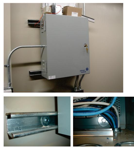
Figure 6.4.8.2-2 Wall anchorage for electrical panel; standard strut anchored to wall studs and panel anchored to strut (Photo courtesy of Maryann Phipps, Estructure).
