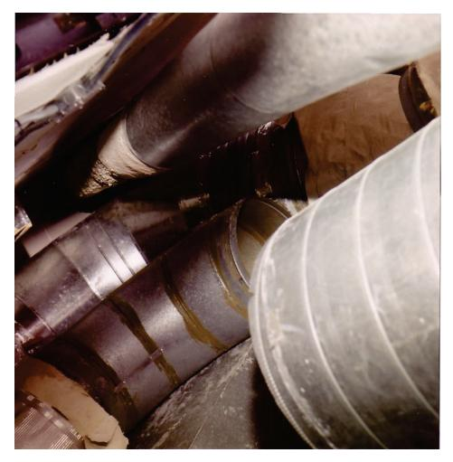
Figure 6.4.6.1-1 Unbraced ducts separated at bend in the 1994 magnitude-6.7 Northridge Earthquake (Photo courtesy of Mason Industries).
