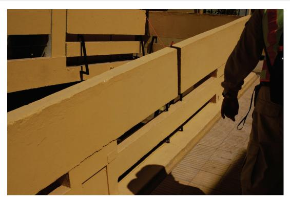
Figure 6.3.1.3-6 Residential building with precast concrete corridor and balcony railing panels. Some panels were damaged and subsequently many were removed to prevent falling. Location in Rancaqua, Chile 154 miles northeast of the epicenter; estimated PGA of 0.3g during the 2010 magnitude-8.8 Chile Earthquake (Photo courtesy of Antonio Iruretagoyena, Rubén Boroschek & Associates).
