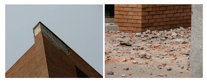
Figure 6.3.1.1-4 Failed adhered veneer fallen from parapet in Santiago following the 2010 magnitude-8.8 Chile Earthquake. (Photos courtesy of Antonio Iruretagoyena, Rubén Boroscheck & Associates)
