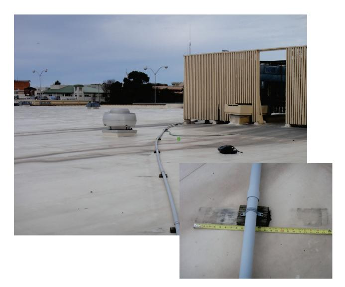
Figure 6.4.3.6-2 Unrestrained wood sleepers on roof-mounted piping slid a foot in either direction in 2010 magnitude-6.5 Eureka Earthquake (Photos courtesy of Maryann Phipps, Estructure).
