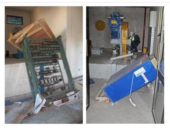
Figure 6.4.10.2-6 Overturned control panels in the 2010 Chile earthquake (Photos courtesy of Eduardo Miranda, Stanford University).
