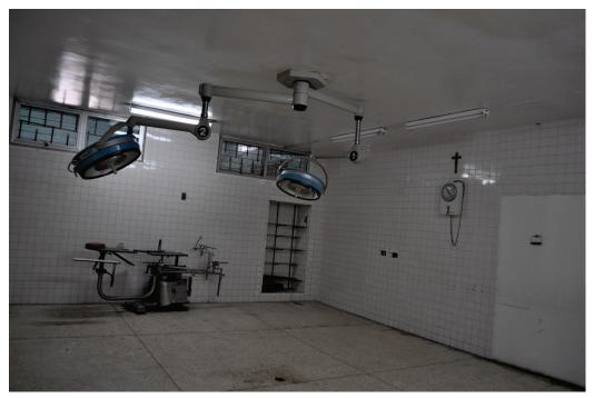
Figure 6.4.9.4-1 Operating room lights undamaged although hospital evacuated due to collapse of adjacent wing in the 2010 magnitude-7 Haiti Earthquake. Fixture anchored to underside of concrete slab (Photo courtesy of Ayhan Irfanoglu, Purdue University).
