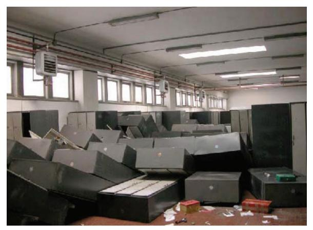
Figure 6.5.5.1-3 Unanchored cabinets toppled in the 1994 Northridge Earhtquake (Photo courtesy of Wiss, Janney, Elstner)
