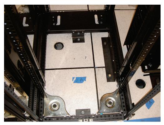
Figure 6.5.3.1-6 Base of data cabinet with supplemental angles bolted to strut bracing below floor (Photo courtesy of Maryann Phipps, Estructure).
