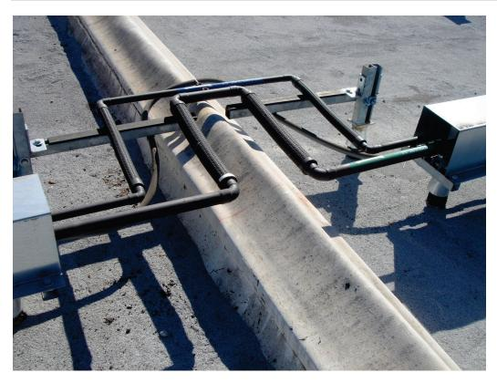
Figure 6.4.3.3-4 Flexible pipe connections at rooftop expansion joint (Photo courtesy of Maryann Phipps, Estructure).
