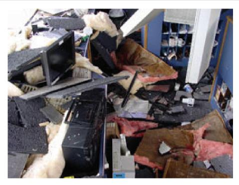
Figure 6.5.3.3-2 Damage to control tower at the SeaTac Airport in the 2001 Nisqually Earthquake (Photo courtesy of JCP Geologists).
