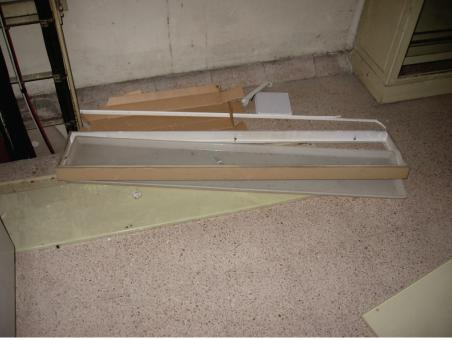
Figure 6.4.9.2-2 Overhead surface-mounted fixture anchored to underside of concrete slab damaged in the 2010 Chile Earthquake. Back of fixture housing remained anchored to the concrete slab above and the bulbs remained in place but the lens and sides of housing fell indicating that internal connections in the fixture were inadequate (Photos courtesy of Rodrigo Retamales, Rubén Boroschek & Associates).
