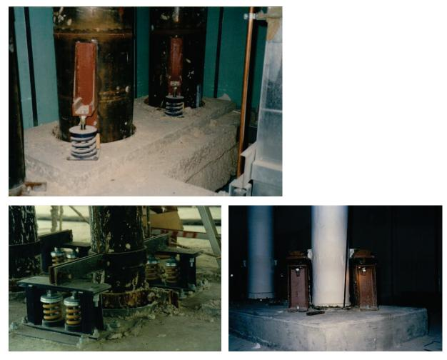
Figure 6.4.3.4-3 Different schemes for riser supports at floor penetrations with vibration isolation: first one with restraint hardware welded to pipe, second with two sets of riser clamps, and third with riser clamp inside the insulation (Photos courtesy of Mason Industries).
