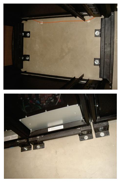
Figure 6.5.3.2-3 Base anchorage details for data cabinets; top photos shows internal anchorage, bottom photo shows external anchorage (Photos courtesy of Maryann Phipps, Estructure).
