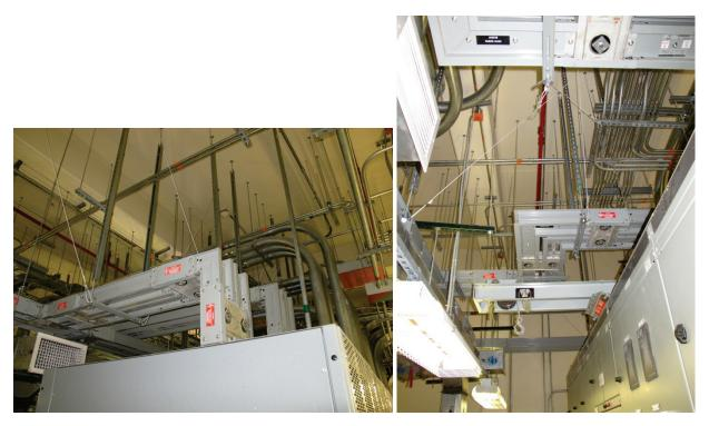
Figure 6.4.7.3-3 High ampacity power busway routing power from generator paralleling switchgear to facility. Note use of lateral restraints in addition to gravity hanger. Supplied uninterrupted power to critical facility during the 2010 M 7.0 Haiti earthquake. (photos courtesy of Philip J. Caldwell)
