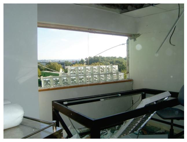
Figure 6.3.1.5-3 Damaged glass block panel from the Los Angeles Hospital in the 2010 Chile Earthquake; relatively new hospital building that had to be evacuated for repairs (Photo courtesy of Bill Holmes, Rutherford & Chekene). Blocks were installed with steel reinforcing bars in the top and bottom horizontal joints.
