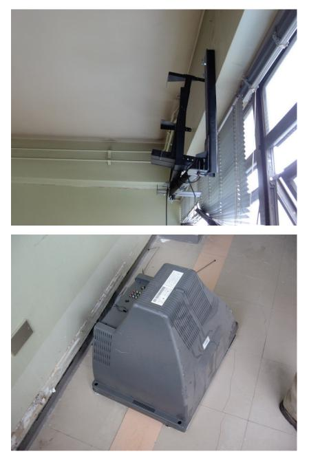
Figure 6.5.3.4-1 Wall-mounted monitor fell from the bracket in a hospital in the 2010 magnitude-8.8 Chile Earthquake; bracket still anchored to the wall (Photos courtesy of Rodrigo Retamales, Rubén Boroschek & Associates)
