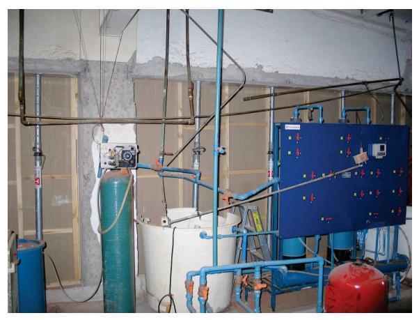
Figure 6.3.2.1-6 An infill masonry wall collapsed onto the distilled water equipment spilling two 150 gallon containers; water leaked past the perimeter edge of the floor slab into the operating room suite below resulting in the closure of 3 of 6 the operating rooms. Replacement gypsum board partition seen in photo. Hospital built in 2005 in Los Angeles, Chile. Damage from the 2010 Chile Earthquake (Photo courtesy of Bill Holmes, Rutherford & Chekene).
