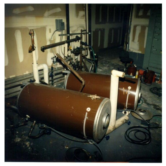
Figure 6.4.2.4-1 Unanchored water heaters overturned (Photo courtesy of Mason Industries).
