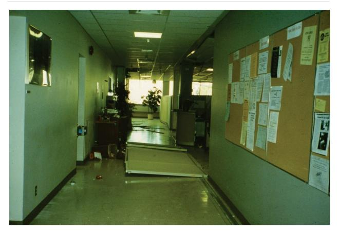
Figure 6.5.5.2-2 Damage to unbraced demountable partition in Silicon Valley office building in the 1989 magnitude-6.9 Loma Prieta Earthquake (Photo courtesy of Maryann Phipps, Estructure).
