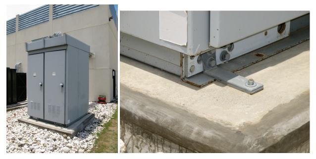
Figure 6.4.7.3-4 Outdoor low voltage switchgear supplying incoming utility power to critical facility. Note equipment frame seismic anchorage load path is bolted at both equipment frame and pad with a continuous rigid load path. Post earthquake photo from the 2010 M 7.0 Haiti earthquake. (photos courtesy of Philip J. Caldwell)
