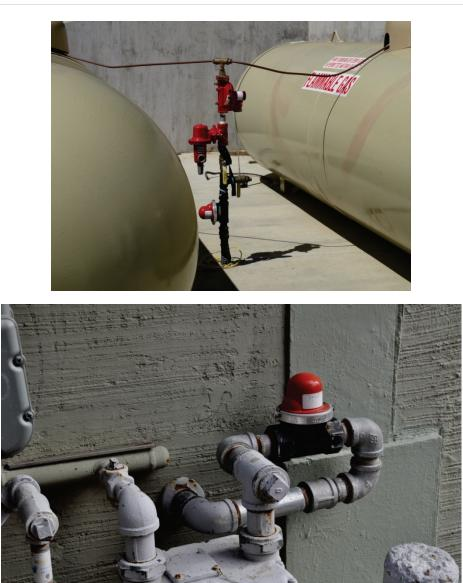
Figure 6.4.5.1-8 Two examples of seismic shut-off valves in San Francisco Bay Area. Top photo at Marine Mammal Center; lower photo at six unit apartment building in Oakland (Photos courtesy of Cynthia Perry, BFP Engineers).
