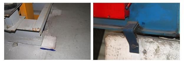
Figure 6.4.10.2-5 Details of bent bracket (left) and large displacement at the base of elevator machines (Photos courtesy of Eduardo Miranda, Stanford University).
