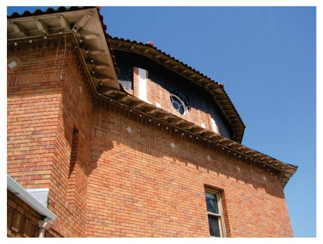
Figure 6.3.1.1-1 Failure of adhered masonry veneer at the Atascadero City Hall in the 2003 magnitude-6.5 San Simeon Earthquake (Photo courtesy of Mike Mahoney, FEMA).
