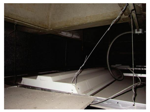
Figure 6.4.9.1-5 Example of light fixture with only one safety wire attached; the Salt Lake City schools require four wires for a fixture of this size and weight and also require tighter turns on the wire (Photo courtesy of Salt Lake City School District). Investigations in ceiling plenums often reveal missing wires.
