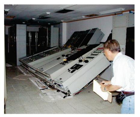
Figure 6.4.7.1-1 Overturned equipment in the 1985 magnitude-8 Mexico Earthquake, note absence of anchorage of equipment base to floor (Photo courtesy of Degenkolb Engineers).
