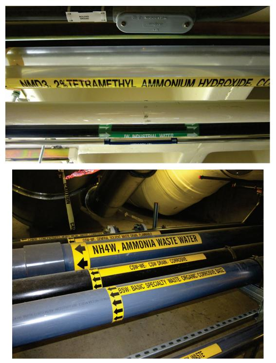
Figure 6.4.5.1-5 Two examples of double walled piping used for secondary containment of hazardous fluids. Preassembled double walled pipe with centering devices or spacers separating the inner and outer pipe is available commercially, but as shown here, the outer pipe was installed and leak tested prior to pulling the inner pipe through. Note the yellow color coded labels indicate reactive materials; flow direction also marked prominently (Photos courtesy of Jeffrey Soulages, Intel Corporation).
