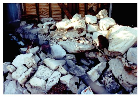
Figure 6.3.1.2-3 Rubble from failed anchored veneer as a result of the 1994 Northridge Earthquake (Photo courtesy of Robert Reitherman).
