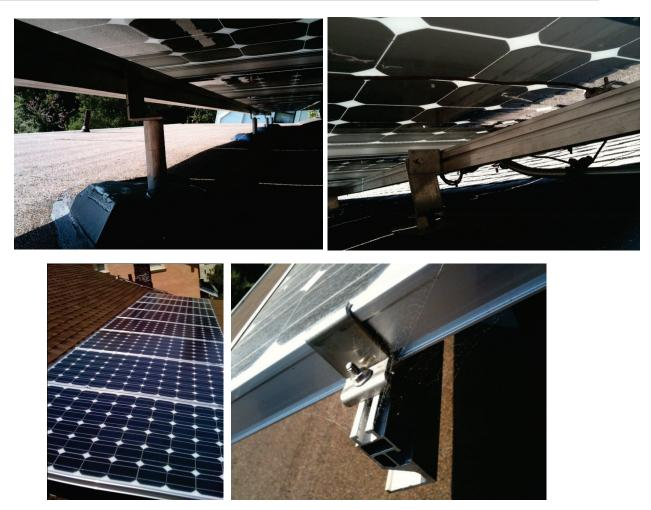
Figure 6.4.7.5-3 Residential photovoltaic system in Berkeley, California mounted over the transition between two different roof slopes (Photos courtesy of Heber Santos). Short standoff used on tar and gravel flat portion (upper left); aluminum flashing and mounting bracket used on sloped portion with composition tile roofing (upper right). The profile of one type of proprietary mounting track is seen at lower left.
