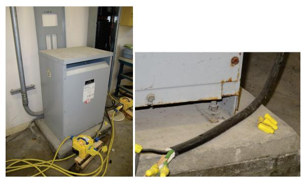
Figure 6.4.7.3-2 Typical electrical distribution dry type transformer. Note the use of manufacturer supplied anchor locations on base channels. Post earthquake photo from the 2010 Haiti M 7.0 Earthquake (photos courtesy of Philip J. Caldwell).
