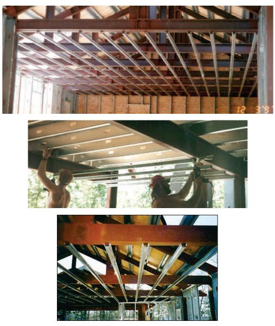
Figure 6.3.4.2-6 Mitigation examples with 1-1/2" hat channels at 16" on centers screwed in place with #12 self drilling screws and furring strips ready to receive gypsum board (Photo courtesy of Excalibur Steel). No special seismic details are required for this type of ceiling where the gypsum board is well secured directly to furring strips.
