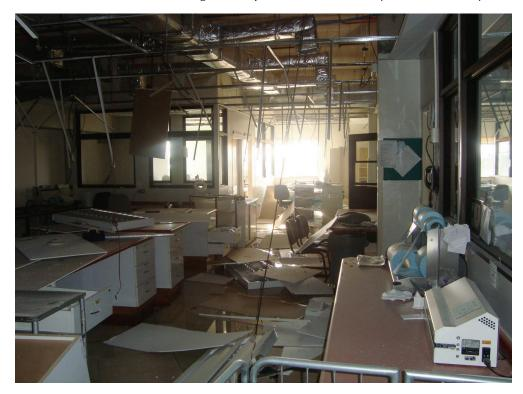
Figure 6.3.4.1-3 Generalized failure of ceiling grid, tiles, lights, and diffusers at the Los Angeles Hospital in the 2010 magnitude-8.8 Chile Earthquake (Photo courtesy of Bill Holmes, Rutherford & Chekene).
