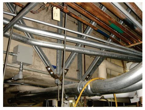
Figure 6.4.8.1-3 Rigid strut bracing for trapeze supporting electrical conduit; conduit attached to trapeze with conduit clamp that provides lateral and longitudinal restraint (Photo courtesy of Maryann Phipps, Estructure).
