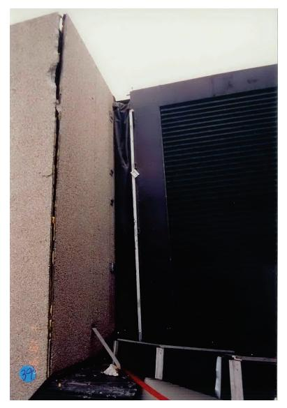
Figure 6.3.1.3-3 Precast panel damage at a building corner in the 1994 Northridge Earthquake (Photo courtesy of OSHPD).
