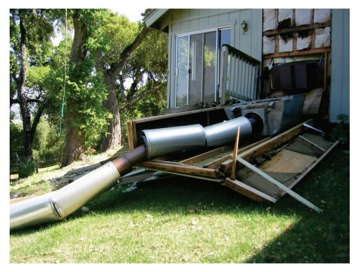
Figure 6.3.7.1-2 Residential metal flue in wood frame chimney that failed in the 2003 magnitude-6.5 San Simeon earthquake. The house fell off its cripple wall, pushing over the chimney (Photo courtesy of Michael Mahoney).
