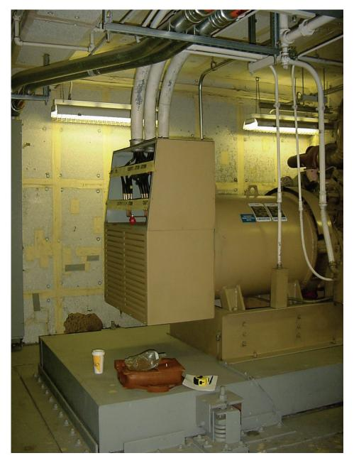
Figure 6.4.7.2-1 Emergency generator is anchored to a concrete inertia base. The inertia base is mounted on spring isolators and restrained by steel angle snubbers on all sides (Photo courtesy of Maryann Phipps, Estructure).
