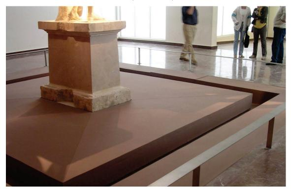
Figure 6.5.6.3-3c Completed installation of statue on platform with base isolation (Photo courtesy of University at Buffalo, SUNY).
