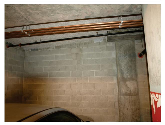
Figure 6.3.2.1-8 Full-height concrete masonry unit walls detailed with steel clip angles (3 angles visible in photo). Configuration shown includes perpendicular walls, sloping ramp above, and column with column capital. Although wall detailed with sealant joints along edges of column and column capital, it is not clear that the concrete frame can move independently of these CMU walls (Photo courtesy of Cynthia Perry, BFP Engineers).
