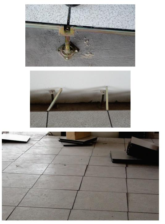
Figure 6.5.3.1-2 Damage to access floor with short anchored pedestals in the 2010 magnitude-6.7 Chile Earthquake; floor did not have lateral bracing. Note many tiles misaligned (Photos courtesy of Antonio Iruretagoyena, Rubén Boroschek & Associates).
