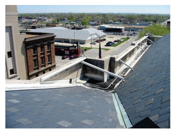
Figure 6.3.5.1-5 Bracing of unreinforced masonry parapet (Photo courtesy of Degenkolb Engineers).
