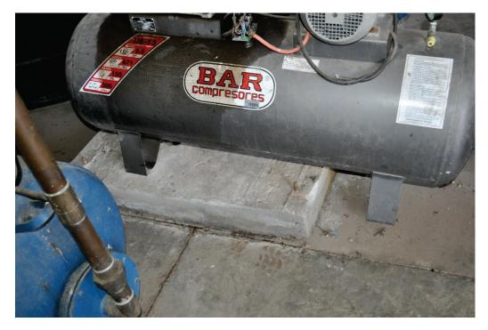
Figure 6.4.1.4-1 Poorly anchored compressor jumped off the undersized anchor bolts in the 2010 magnitude-8.8 Chile Earthquake (Photo courtesy of Eduardo Fierro, BFP Engineers).
