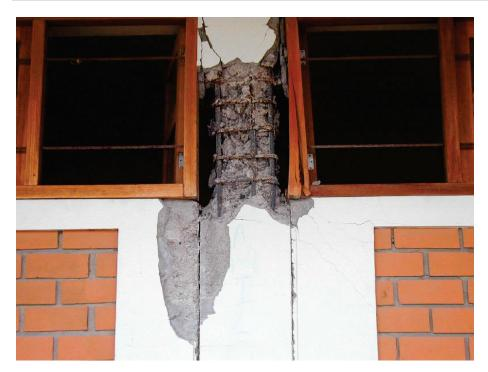
Figure 6.3.2.1-3 Damage to structural column ("captive column") due to restraint caused by partial height masonry wall in the 2001 Peru Earthquake (Photo courtesy of Eduardo Fierro, BFP Engineers).
