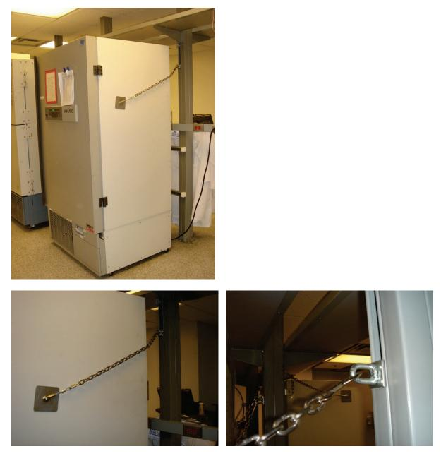
Figure 6.5.5.3-5 Typical tethering details for kitchen equipment and vending machines. Tether provided on both sides of equipment and does not penetrate the equipment housing (Photos courtesy of Maryann Phipps, Estructure).
