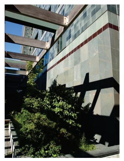
Figure 6.3.1.1-5 Landscaping strip restricts pedestrian access adjacent to adhered veneer façade. Larger units used within lower 6 feet; smaller units used above (Photo courtesy of Cynthia Perry, BFP Engineers).
