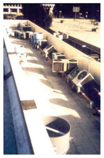
Figure 6.4.1.4-2 Unanchored rooftop units thrown off their supports during an earthquake (Photo courtesy of Maryann Phipps, Estructure).
