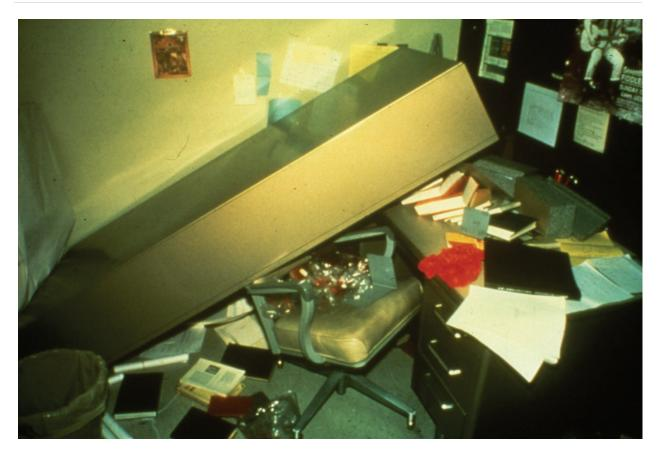
Figure 6.5.2.1-3 Bookcase overturned onto desk in the 1971 magnitude-6.6 San Fernando Earthquake (Photo courtesy of Degenkolb Engineers).
