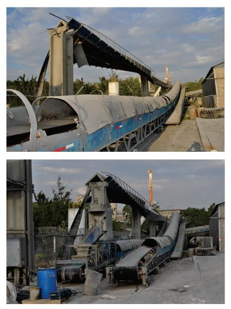
Figure 6.4.1.2-1 Damage to conveyors and equipment at a cement plant in the 2010 magnitude-7 Haiti Earthquake (Photos courtesy of Eduardo Fierro, BFP Engineers).
