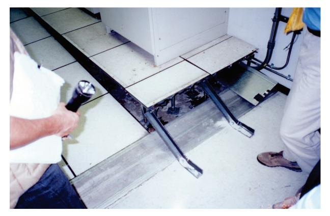
Figure 6.5.3.1-1 Temporary bracing for access floor collapsed in the1994 magnitude-6.7 Northridge Earthquake (Photo courtesy of Wiss, Janney, Elstner Associates).
