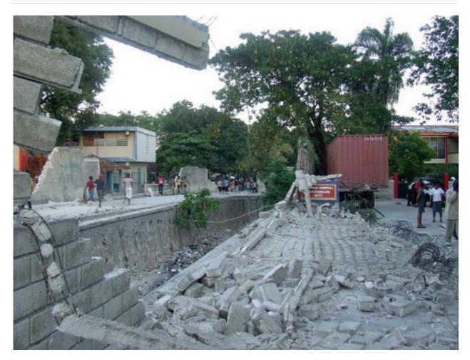
Figure 6.3.9.1-2 Freestanding masonry fences with inadequate reinforcement collapsed covering both sides of this street in Port-au-Prince in the 2010 magnitude-7 Haiti Earthquake (Photo courtesy of Yves Montoban). Many miles of such fencing collapsed in the 2010 Haiti Earthquake.
