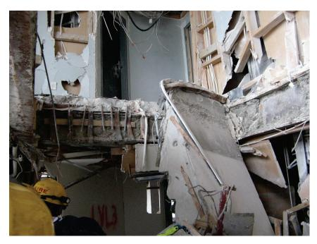
Figure 6.3.8.1-4 Stair support condition at Forsyth-Barr Building in Christchurch, New Zealand. Precast stair runs have completely pulled off supports and collapsed into stairwell (Photo courtesy of Des Bull, Holmes Consulting Group).
