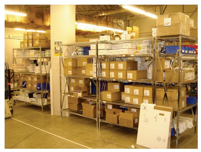
Figure 6.5.1.1-7 Fixed base shelving units anchored directly to concrete slab through base plate (Photo courtesy of Maryann Phipps, Estructure).
