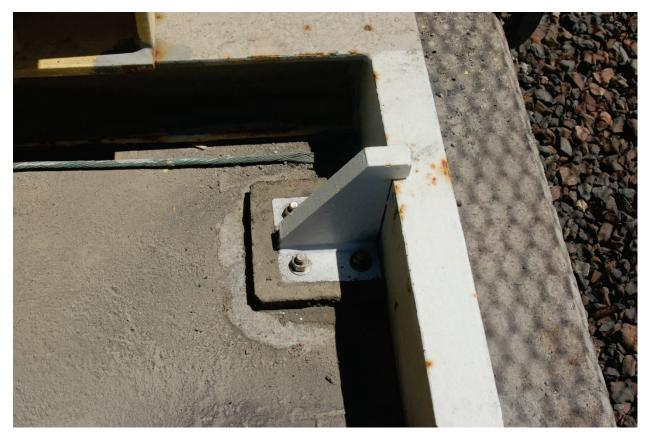
Figure 6.4.1.1-5 Alternate detail for skid mounted equipment (Photo courtesy of Eduardo Fierro, BFP Engineers).
