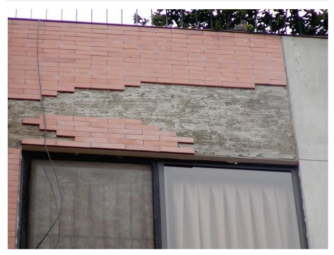
Figure 6.3.1.1-2 Close-up of failed adhered veneer. (Photo courtesy of Eduardo Fierro, BFP Engineers).
