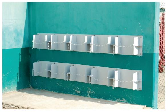
Figure 6.4.2.3-4Wall-mounted cylinder restraints upgraded with stiffener plates following the<br/>2001 Peru Earthquake(Photo courtesy of Eduardo Fierro, BFP Engineers).
