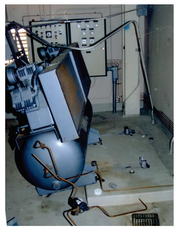
Figure 6.4.1.3-1Failure of compressor mounted on vibration isolators in the 1994 Northridge<br/>Earthquake (Photo courtesy of Wiss, Jenney, Elstner Associates).
