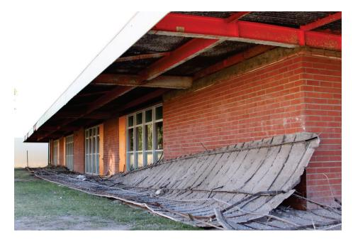
Figure 6.3.4.3-3 Collapse of exterior soffit at Jefferson Elementary School in Calexico in the 2010 Baja California Earthquake; approximately 1200 sq ft of soffit collapsed at this school built in the 1960's (Photo courtesy of Baja Earthquake Reconnaissance Team, Earthquake Engineering Research Institute (EERI), published in the EERI July 2010 Newsletter).
