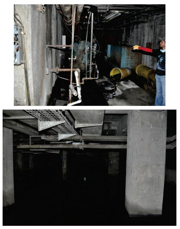
Figure 6.4.5.1-2 Basement level at power plant in Port-au-Prince flooded with oil and water in the 2010 magnitude-7 Haiti Earthquake creating hazardous conditions for inspection and clean-up (Photos courtesy of Eduardo Fierro, BFP Engineers).
