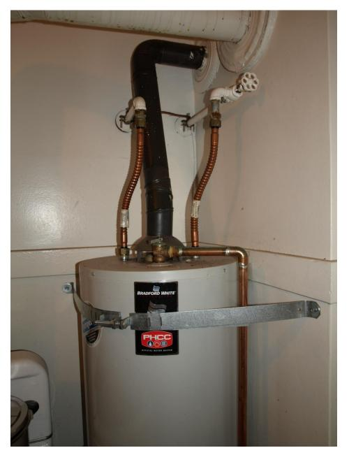
Figure 6.4.2.4-4 Corner installation using a commercially available strap; note flex copper tubing for water hook up (Photo courtesy of Cynthia Perry, BFP Engineers).
