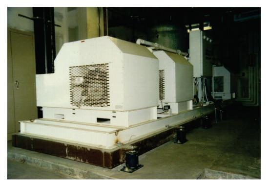
Figure 6.4.1.3-5 Restrained springs used to support heavy equipment (Photo courtesy of Mason Industries).
