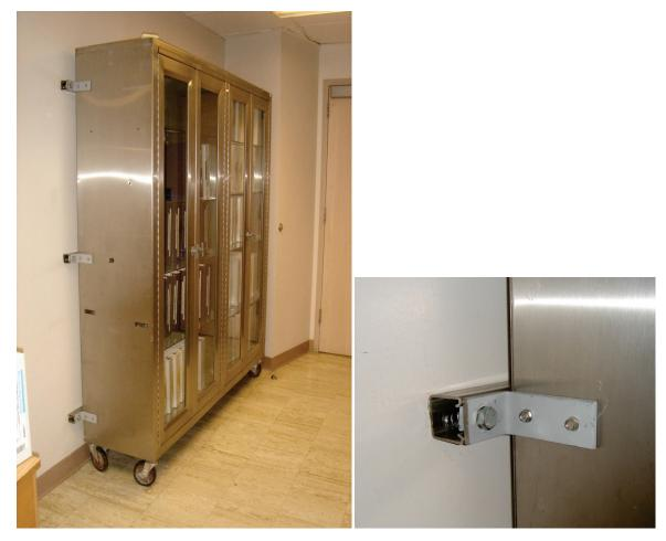
Figure 6.5.1.1-8 Mobile shelving unit restrained by connection to strut fastened to full height metal studs (Photo courtesy of Maryann Phipps, Estructure).
