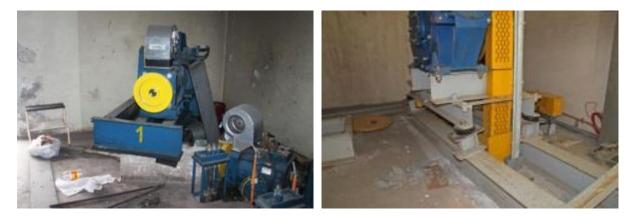
Figure 6.4.10.2-4 Examples of damage to elevator machines produced by inadequate anchorage to the structure (Photos courtesy of Eduardo Miranda, Stanford University).
