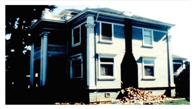
Figure 6.3.7.1-3 Chimney collapse (Photo courtesy of Earthquake Engineering Research Institute).
