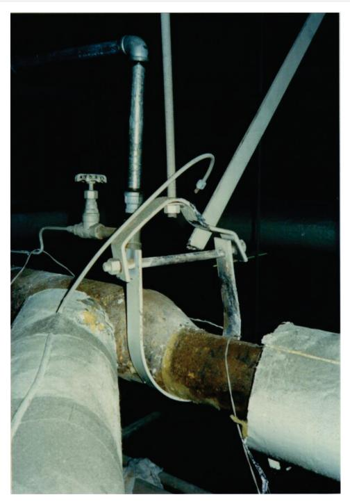
Figure 6.4.3.1-3 Pipe brace failed at connection in 1994 Northridge Earthquake; insulation removed prior to photo (Photo courtesy of Mason Industries).
