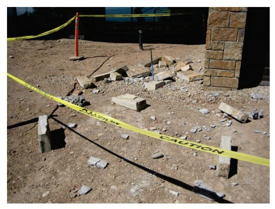
Figure 6.3.1.2-2 Fallen sandstone veneer as a result of a magnitude-4.4 earthquake (Photo courtesy of Simpson Gumpertz and Heger).
