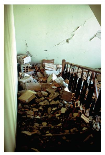
Figure 6.3.2.1-4 View of stairway in the Banco Central Building, Managua, Nicaragua after the 1972 magnitude 6.2 Managua Earthquake. Most of the stairs were covered with debris that resulted from the failure of the hollow tile partitions surrounding the stairs (Photo courtesy of PEER Godden Collection, No. J94).
