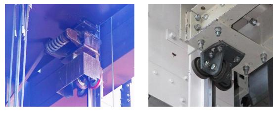
Figure 6.4.10.2-3 Examples of rolling guides at the bottom of a car (Photos courtesy of Eduardo Miranda, Stanford University).
