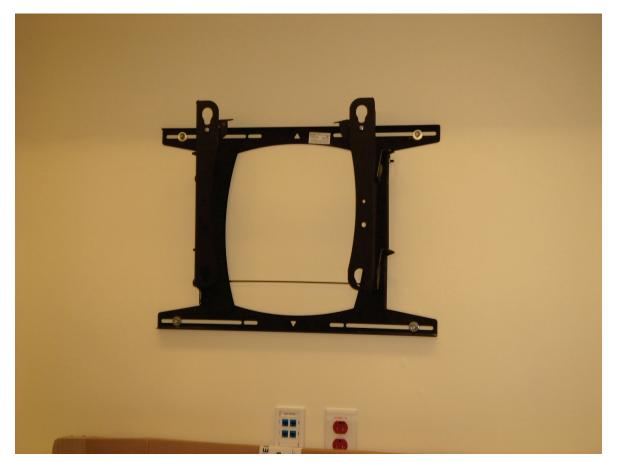
Figure 6.5.3.4-2 Wall-mounted television bracket anchored with sheet metal screws to wall studs at four locations. Bracket must be rated for the weight of television or monitor and that the unit must be securely attached to the bracket (Photo courtesy of Maryann Phipps, Estructure).
