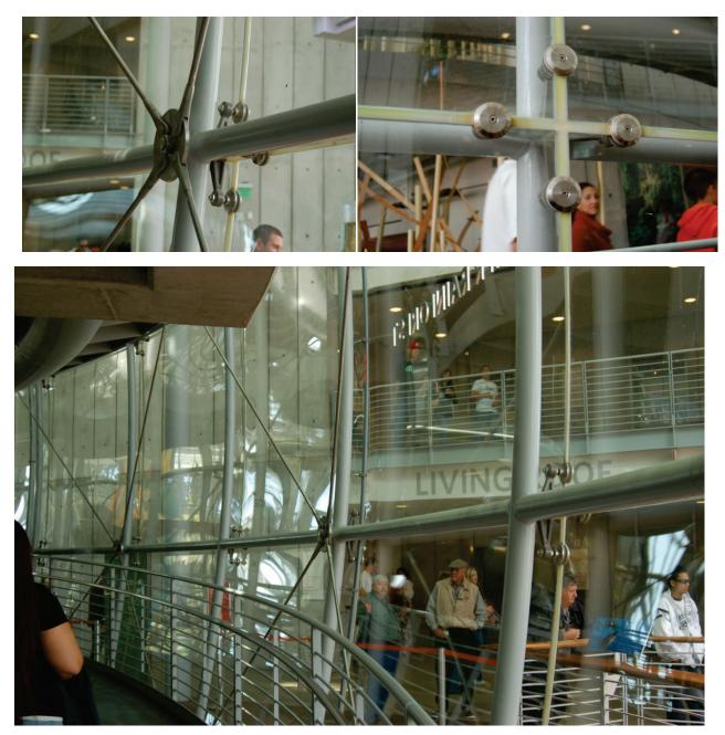
Figure 6.3.2.3-5 Specialized glazing details for glass dome using specialty hardware, such as large sealant joints required to accommodate thermal movement and seismic deformations at the California Academy of Sciences, San Francisco, California (Photos courtesy of Cynthia Perry, BFP Engineers).
