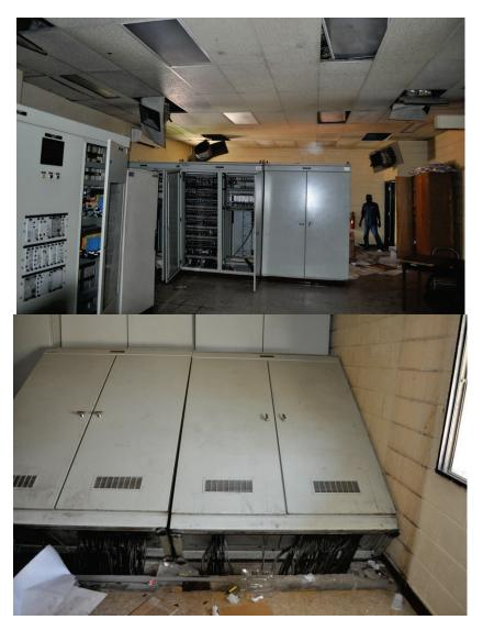
Figure 6.4.7.1-3 Damage to unanchored electrical cabinets at power plant in Port-au-Prince in the 2010 magnitude-7 Haiti Earthquake (Photos courtesy of Eduardo Fierro, BFP Engineers).
