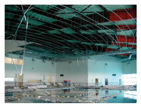
Figure 6.3.4.3-2a Complete collapse of a large suspended gypsum board ceiling over a swimming facility in Japan (Photo courtesy of Shojiro Motoyui, Tokyo Institute of Technology). This type of failure has been replicated on the E-defense shake table and occurs when the U-shaped clip holding the cross furring (M-bar) to the main runners (channel) opens into a V-shape and drops the furring grid. This type of failure is not common in the U.S.
