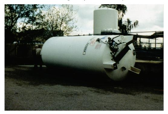
Figure 6.4.2.1-2 A vertical tank at hospital overturned due to inadequate anchorage in the 1994 Northridge Earthquake (Photo courtesy of OSHPD).
