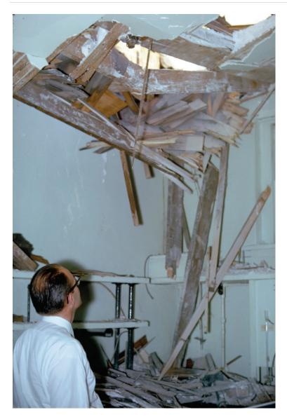
Figure 6.3.5.1-3Damage to roof framing caused by failure of overhanging brick masonry during<br/>the 1962 magnitude-5.8 Cache Valley, Utah earthquake (Photo courtesy of<br/>PEER Steinbrugge Collection, No. S828).
