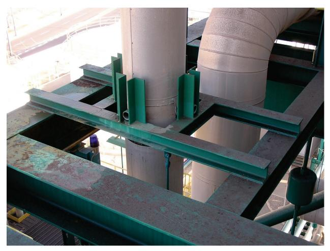
Figure 6.4.3.4-4 Insulated boiler pipe risers with welded lugs (small pipe sections) which travel vertically in guides providing lateral seismic restraint (Photo courtesy of Eduardo Fierro, BFP Engineers).
