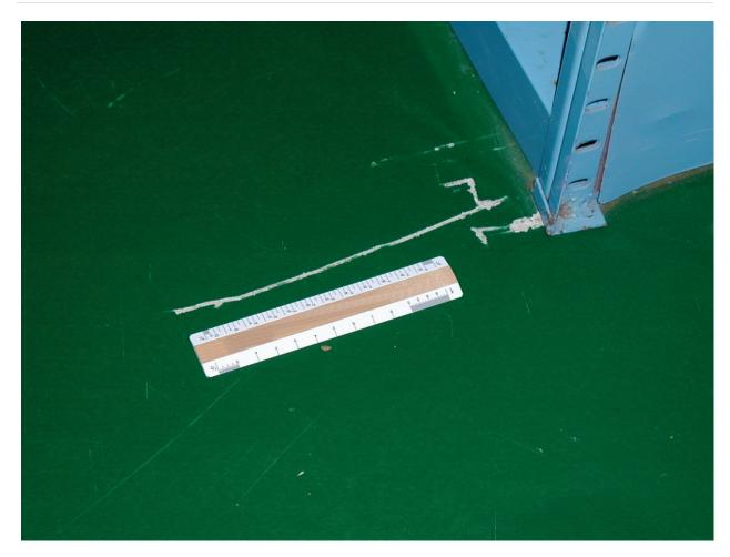
Figure 6.5.1.1-2 Unanchored storage shelving slid nine inches without falling but contents scattered in the 2001 magnitude-8.4 Peru earthquake; unit lifted to original position prior to photo (Photo courtesy of Eduardo Fierro, BFP Engineers).
