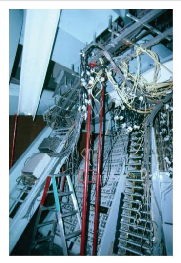
Figure 6.5.3.2-2 Damage to communication and computer racks (Photo courtesy of Degenkolb Engineers).
