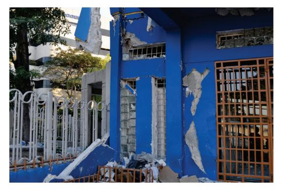
Figure 6.3.1.5-1 Damage to glass block in building with reinforced concrete frame and concrete masonry infill in the magnitude-7 2010 Haiti Earthquake (Photo courtesy of Eduardo Fierro, BFP Engineers). Note some blocks failed at rigid mortar joints and stayed in the frame, others fell out of the frame, and others broke in place. This building also suffered structural damage.
