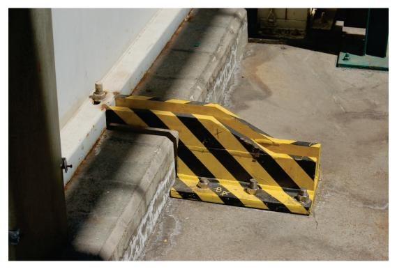
Figure 6.4.1.1-3 Added lateral capacity provided for skid-mounted equipment added following the 2001 Peru Earthquake (Photo courtesy of Eduardo Fierro, BFP Engineers).
