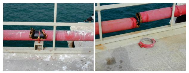
Figure 6.4.4.1-6 Damage to industrial fire protection piping located on jetty in 2001 Peru Earthquake. Longitudinal slip at U-bolt shown at left; this U-bolt still intact but other U-bolts broke and fell off the jetty. Failure of joint coupling and crushing of pipe shown at right (Photo courtesy Eduardo Fierro, BFP Engineers).
