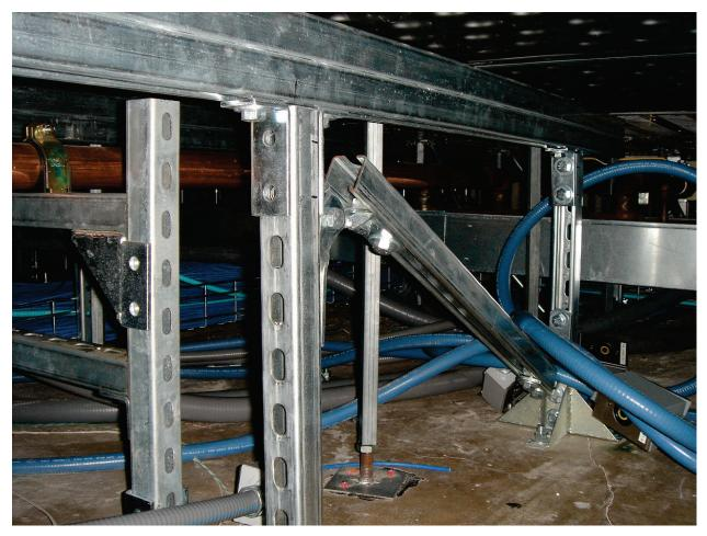
Figure 6.5.3.1-8 Strut framing added to brace data cabinet located on access floor. Bolts from angles above are connected to strut framing below (Photo courtesy of Maryann Phipps, Estructure).
