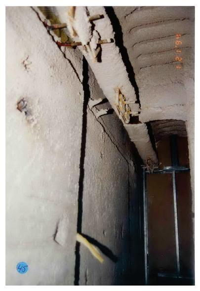
Figure 6.3.1.3-4 Interior view of precast panel showing response of three sets of push-pull connections in the 1994 Northridge Earthquake (Photo courtesy of OSHPD).
