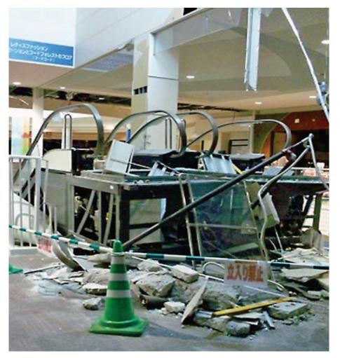
Figure 6.4.10.3-1 Photo of escalator, located in the Sendai area of Japan, which fell from the floor above onto the escalator on the floor below during the magnitude-9.0 Great Tohoku Earthquake of March 11, 2011. The probable cause of this collapse was that the relative displacements between floors exceeded the connection bearing width capacity of the escalator. This type of failure creates a serious life safety hazard (Photo source: Nekkei Architecture).
