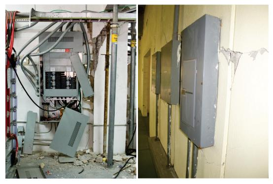
Figure 6.4.7.3-8 Example of rugged equipment. Post earthquake photos of two different essential facilities which sustained significant structural damage during the 2010 M 7.0 Haiti Earthquake. Wall mounted electrical power distribution panels were undamaged and remained functional even though the walls they were mounted to were severely damaged during the earthquake (photos courtesy of Philip J. Caldwell).
