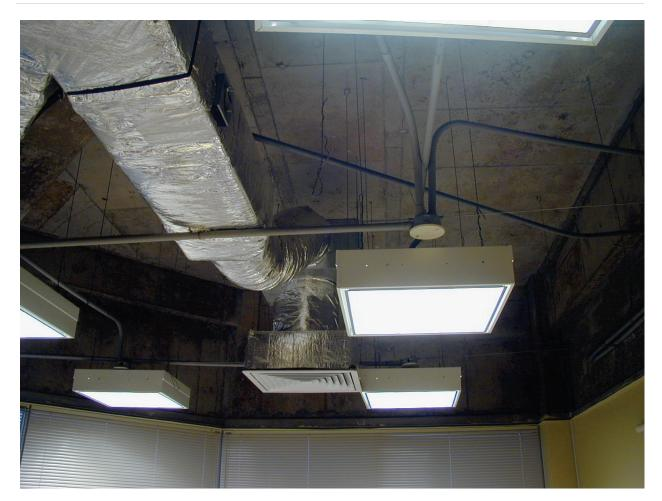
Figure 6.4.9.1-2 Overhead lights with four vertical hangers to the structure. Unbraced acoustic ceiling system was damaged beyond repair in the 2001 magnitude-8.4 Peru Earthquake but none of the diffusers or lights fell because they had independent supports. Ceiling was demolished prior to photo (Photo courtesy of Eduardo Fierro, BFP Engineers).
