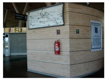
Figure 6.4.9.2-1 Numerous failures of ceilings and lights were observed at the Concepción airport in the 2010 magnitude-8.8 Chile Earthquake. Photo shows surface-mounted fixture on wall that remained in place but the lens fell and the bulbs were dislodged (Photo courtesy of Rodrigo Retamales, Rubén Boroschek & Associates).
