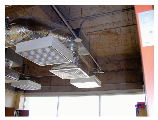
Figure 6.4.6.2-2 HVAC diffuser attached to the structure with four vertical hangers; ceiling system was damaged beyond repair in the 2001 Peru Earthquake but none of the diffusers or lights fell. Ceiling was demolished prior to photo (Photo courtesy of Eduardo Fierro, BFP Engineers).
