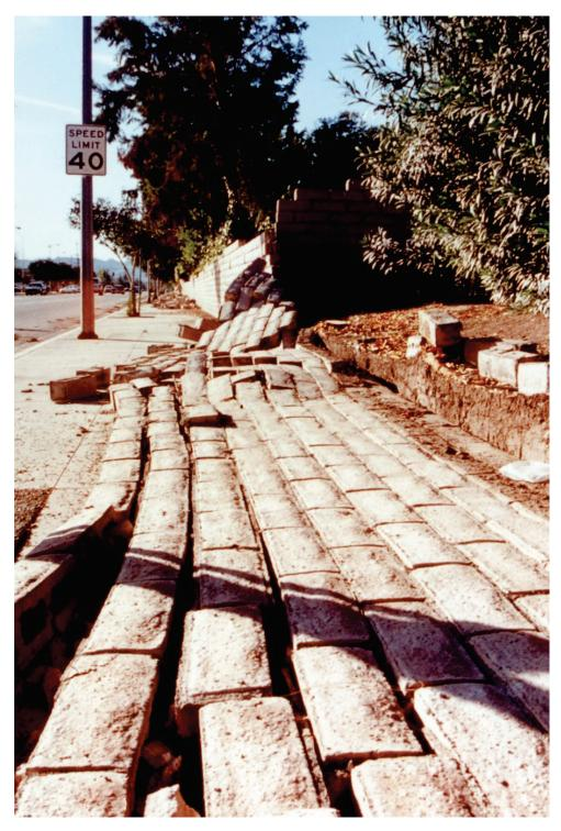
Figure 6.3.9.1-1 Collapse of freestanding CMU walls covering much of the sidewalk in the 1994 magnitude-6.7 Northridge Earthquake (Photo courtesy of Robert Reitherman). The rubble reveals that the wall was unreinforced.
