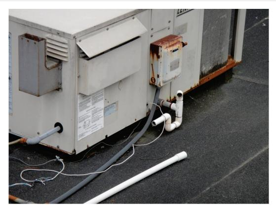
Figure 6.4.3.6-3 Unrestrained roof-mounted piping broke at the connection to the equipment in the 2010 Eureka Earthquake. Piping mounted on wood sleepers should typically be restrained to the roof, not free to slide (Photo courtesy of Maryann Phipps, Estructure).
