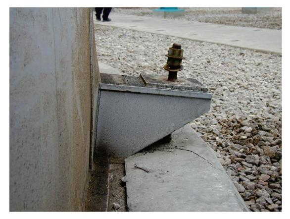
Figure 6.4.2.2-1 Damage to ductile connection at base of a 5000 cubic meter diesel fuel tank in the 2001 magnitude-8.4 Peru Earthquake. All eight connections were damaged; damage included bolt elongation, deformation of tank wall, and cracked concrete pad (Photo courtesy of Eduardo Fierro, BFP Engineers).
