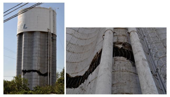
Figure 6.4.3.7-2 Pipe supports attached to wall of damaged silo (Photo courtesy of Eduardo Fierro, BFP Engineers). In spite of structural damage to silo, cast-in-place pipe supports were still intact and the piping did not fall.
