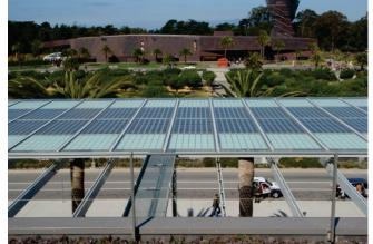
Figure 6.4.7.5-1 60,000 photovoltaic cells are incorporated into the glass canopy surrounding the Academy of Science, San Francisco, California (Photos courtesy of Cynthia Perry, BFP Engineers). The photovoltaic system provides 10% of the electricity needed for the facility. Panels must be securely attached to resist wind loads but also because these cantilevered members may be subject to vertical as well as horizontal seismic forces.
