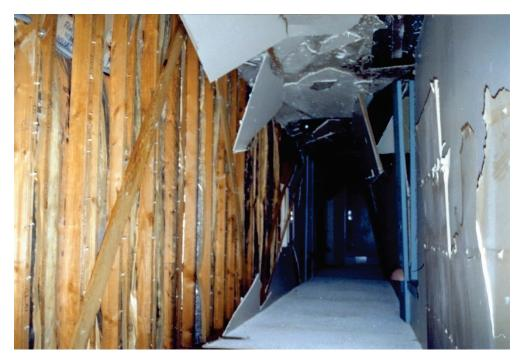
Figure 6.3.2.2-2 In-plane damage to wood stud wall spanning floor-to-floor caused by differential movement between the two floors in the 1994 Northridge Earthquake (Photo courtesy of Wiss, Janney, Elstner Associates).
