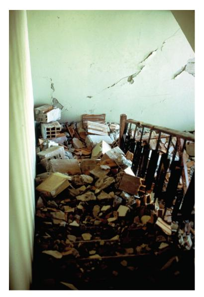
Figure 6.3.8.1-2 View of stairway in the Banco Central Building, Managua, Nicaragua after the 1972 magnitude-6.2 Managua Earthquake. Most of the stairs were covered with debris that resulted from the failure of the hollow tile partitions surrounding the stairs. This photograph highlights the need to not only prevent direct damage to stairway framing and connections, but also to protect against damage to surrounding walls (Photo courtesy of PEER Godden Collection, No. J94).
