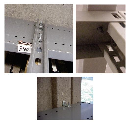
Figure 6.5.2.2-6 Examples of struts and hardware used to retrofit library shelving at the University of California, Berkeley (Photos courtesy of Mary Comerio, Dept. of Environmental Design, University of California Berkeley).
