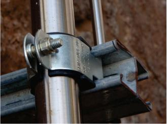
Figure 6.4.5.1-7 Process nitrogen piping outside engineering building on the UC Berkeley campus; strut clamp has rubber fittings to protect the stainless steel piping (Photos courtesy of Cynthia Perry, BFP Engineers).
