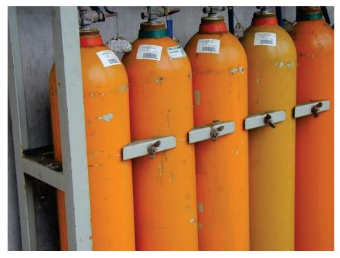
Figure 6.4.2.3-3 Detail of undamaged gas cylinder installation (Photo courtesy of Eduardo Fierro, BFP Engineers).
