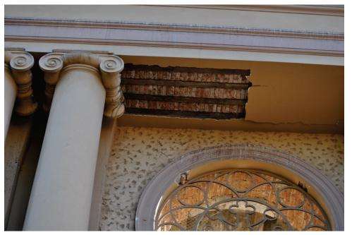
Figure 6.3.4.2-2 Damage to stucco soffit of historic church in the 2010 Chile Earthquake (Photo courtesy of Eduardo Fierro, BFP Engineers). Stucco applied directly to the underside of the slab above without furring; portion at left has fallen, portion at right delaminated.
