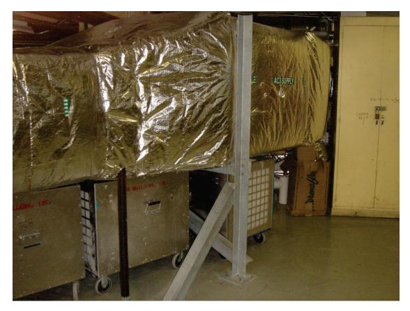
Figure 6.4.6.1-5Floor-mounted rectangular duct supported on braced support stand built up<br/>from steel angles (Photo courtesy of Maryann Phipps, Estructure).
