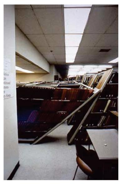
Figure 6.5.2.2-3 Longitudinal failure of library shelving units (Photo courtesy of NISEE-PEER, U.C. Berkeley). Transverse ties used to tie units together but this was not enough to prevent longitudinal failure.
