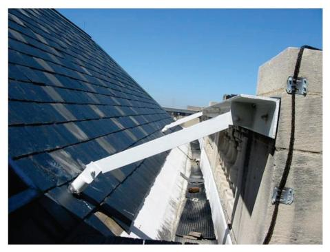
Figure 6.3.5.1-6 Close-up of parapet bracing (Photo courtesy of Degenkolb Engineers).
