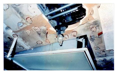
Figure 2.4.3-1 Broken sprinkler pipe at Olive View Hospital in Sylmar, California as a result of the 1994 Northridge, Earthquake. Pipe ruptured at the elbow joint due to differential motion of the pipe and ceiling (FEMA 74, 1994).
