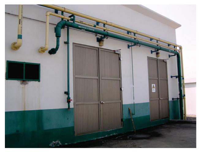
Figure 6.4.3.7-1 Wall-mounted supports for horizontal and vertical pipe runs with exterior exposure. Photo shows minor damage at wall penetration of green pipe and minor movement at some U-bolts, but restraints generally performed well (Photo courtesy of Eduardo Fierro, BFP Engineers). Note that lateral restraint near an elbow can be used to provide longitudinal restraint for a perpendicular pipe run.
