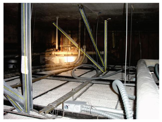
Figure 6.3.4.3-4 Details of suspended and braced plaster ceiling, Rigid bracing and compression posts (highlighted) are provided at 6 ft by 8 ft on center. Note cross furring saddle tied to black channel (main runner) from below; supplementary framing for lights runs parallel to cross furring and saddle tied to main runner from above (Photo courtesy of Maryann Phipps, Estructure).
