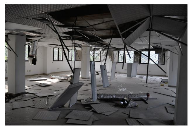
Figure 6.4.9.1-1 Numerous fluorescent fixtures dangling from electrical conduit; installed without safety wires in unbraced suspended acoustical ceiling and damaged in the 2010 magnitude-7 Haiti Earthquake. Loose bulbs, lenses, ceiling panels, diffusers and ducts also on the floor (Photo courtesy of Ayhan Irfanoglu, Purdue University).
