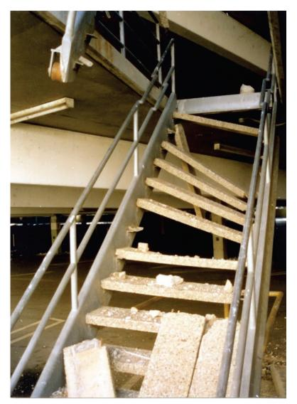
Figure 6.3.8.1-1 Stairway damaged by drift in the 1994 magnitude-6.7 Northridge, California earthquake (Photo courtesy of Wiss, Jenney, Elstner Associates).
