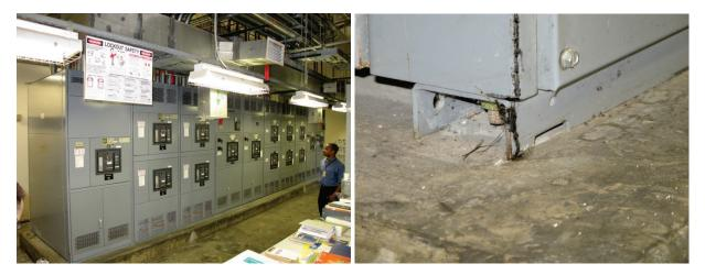
Figure 6.4.7.3-9 Incoming power switchgear for critical facility anchored through base undamaged by the 2010 Haiti M 7.0 Earthquake. Visual inspection of equipment base channels did not reveal any structural damage or equipment displacement on concrete equipment pad. Similar equipment located nearby which did not have a rigid seismic restraint with a continuous load path shifted on its pad (photos courtesy of Philip J. Caldwell).
