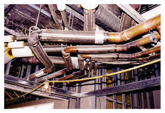
Figure 6.4.3.3-5 Flexible pipe connections at building separation (Photo courtesy of Mason Industries).
