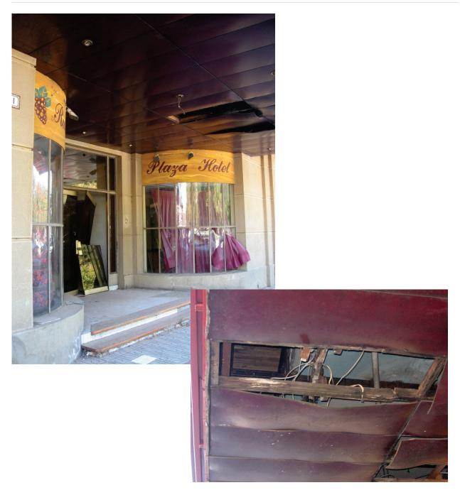
Figure 6.3.4.2-3 Damage to soffit paneling and wood framing at hotel in the 2010 Chile Earthquake; panels and wood framing show signs of prior water damage and deterioration. Note also damage to storefront glazing and glass doors (Photos courtesy of Rodrigo Retamales, Rubén Boroschek & Associates). Available at: http://www.fema.gov/earthquake-publications/fema-e-74-reducing-risks-nonstructural-earthquake-damage Last Modified: December 2012
