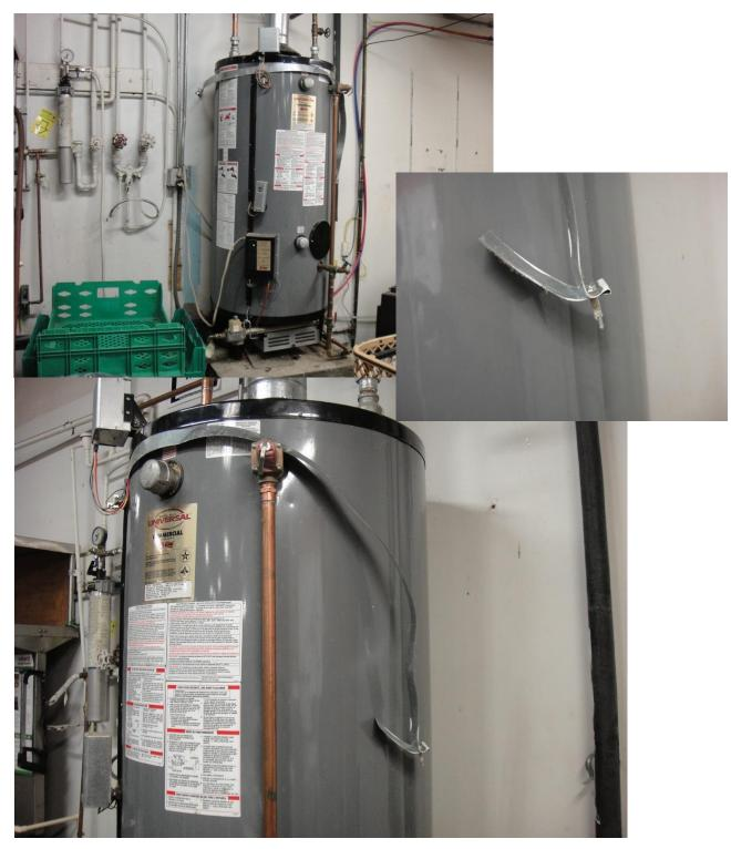
Figure 6.4.2.4-3 Damaged water heater in the 2010 magnitude-6.5 Eureka Earthquake. The water heater strap pulled out from the supporting concrete wall as a result of inadequate anchorage. The tank moved sufficiently to break interconnected water lines which were rigidly connected to the tank.
