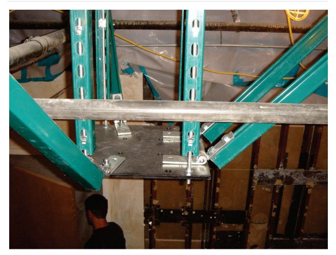
Figure 6.4.9.4-3 Engineered support and bracing for operating room lights located in California hospital. Steel plate has predrilled holes to receive fixture attachments (Photo courtesy of Maryann Phipps, Estructure).
