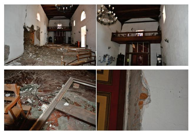
Figure 6.3.2.3-3 Failed wood framed glazing assembly in the 2010 Chile earthquake (Photo courtesy of Eduardo Fierro, BFP Engineers). The wood framing was held in place by metal or rebar brackets embedded in the masonry wall. The adobe wall on the left of the door collapsed and the brackets on the right side pulled out of the brick masonry wall (lower right). The glazing assembly at the rear entrance of the chapel was anchored overhead to the wood balcony framing and was undamaged.
