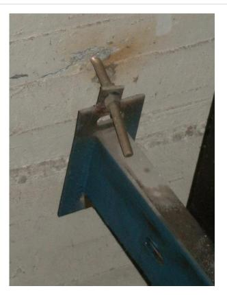
Figure 6.4.10.2-8 Damage to guide rail support brackets in the 2010 Chile Earthquake (Photo courtesy of Gilberto Mosqueda, SUNY Buffalo).
