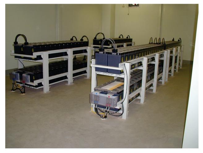
Figure 6.4.7.4-2 Anchored battery racks (Photo courtesy of Eduardo Fierro, BFP Engineers).
