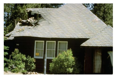
Figure 6.3.7.1-1 Chimney collapsed and fell through the roof; approximately 2,600 chimneys were destroyed in the 1992 Big Bear City, California earthquake (NGDC, 2009).
