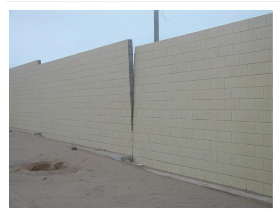
Figure 6.3.9.1-3 Damage to reinforced masonry boundary fence at industrial facility in Southern Peru; out-of-plane movement at construction joint in wall without sufficient reinforcing for the level of shaking experienced at this location in the 2001magnitude-8.4 Peru Earthquake (Photo courtesy of Eduardo Fierro, BFP Engineers). Additional boundary steel or reinforced concrete boundary columns located either side of construction joints would improve the performance of this type of fence.
