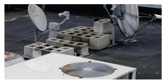
Figure 6.4.7.6-3 Damage or movement of ballasted antennae was not observed on this rooftop in the 2010 magnitude-6.5 Eureka Earthquake (Photo courtesy of Maryann Phipps, Estructure).
