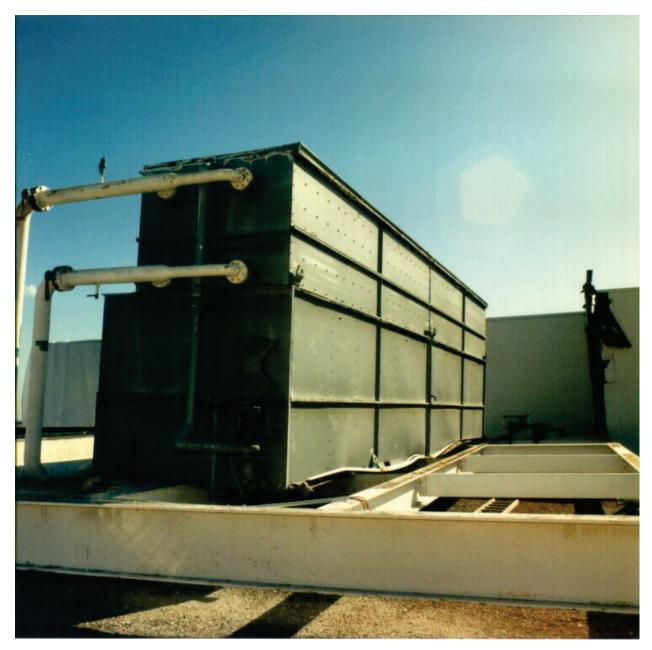
Figure 6.4.1.3-4 Rooftop equipment on isolators collapsed onto skid (Photo courtesy of Mason Industries).
