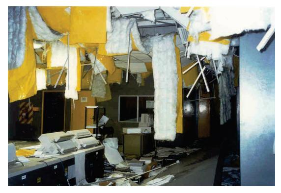
Figure 6.3.4.1-1 Failure of suspended ceiling system including lights, air diffusers, and insulation in control room of an industrial plant in the 2001 magnitude-8.4 Peru Earthquake (Photo courtesy of BFP Engineers).
