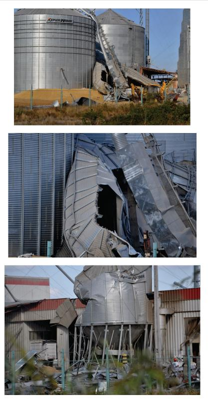
Figure 6.4.1.2-2 Damage to silos, conveyors and equipment at a grain operation in the 2010 magnitude-8.8 Chile Earthquake (Photos courtesy of Eduardo Fierro, BFP Engineers).
