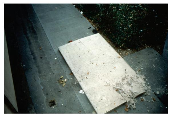
Figure 6.3.1.3-1 Failure of precast panel at parking garage that resulted in fatality in the 1987 magnitude-5.9 Whittier, California earthquake (Photo courtesy of Degenkolb Engineers).
