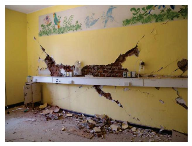
Figure 6.3.2.1-5 Damage to unreinforced brick partitions in patient rooms, and other mostly nonstructural damage, resulted in the evacuation of the Felix Bulnes Hospital in Santiago in the 2010 magnitude-8.8 Chile Earthquake (Photo courtesy of Gilberto Mosqueda, University of Buffalo, SUNY).
