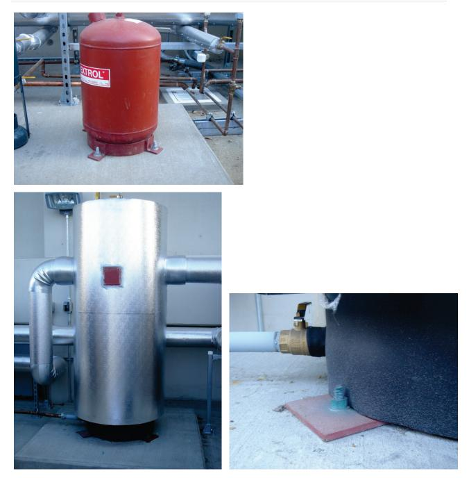
Figure 6.4.2.2-7 Examples of rigid base anchorage for small circular tanks (Photos courtesy of Maryann Phipps, Estructure).
