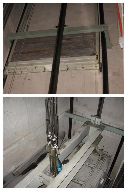
Figure 6.4.10.2-11 Unrestrained movement of the counterweights damaged the counterweight assembly and bent the counterweight guide rails; over half the subweights dropped onto the top of the cab and damaged the cab framing in the 2010
