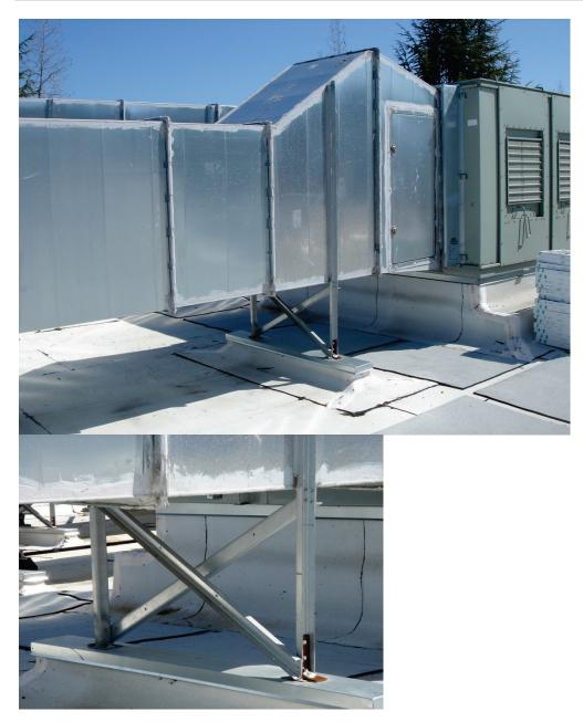
Figure 6.4.6.1-6Roof-mounted rectangular duct supported on braced support stand built up<br/>from steel channels (Photo courtesy of Maryann Phipps, Estructure).
