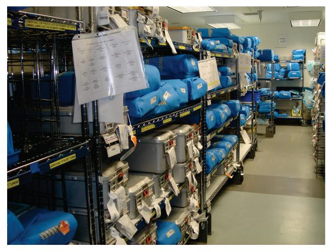
Figure 6.5.1.1-3 Mobile carts restrained at base with clip angles anchored to the floor and removable eyebolts attached from each cart to the angles (Photo courtesy of Maryann Phipps, Estructure).
