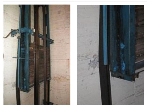
Figure 6.4.10.2-7 Damage to guide rails caused by derailment of the counterweight in a hospital in Chillan during the 2010 Chile earthquake (Photos courtesy of Eduardo Miranda, Stanford University).
