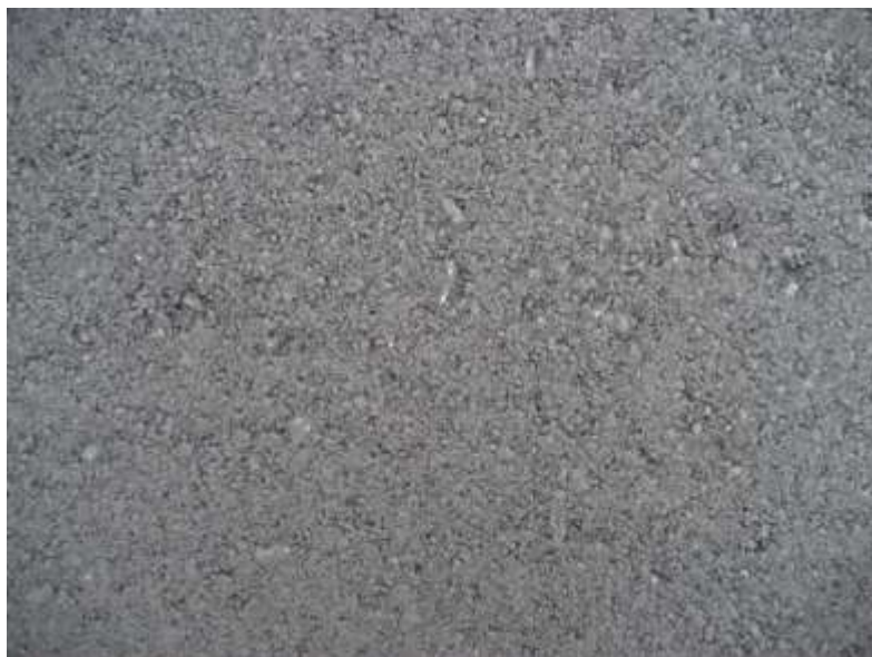
Figure 24. Surface texture of the 12.5 mm HMA overlay after final rolling.
