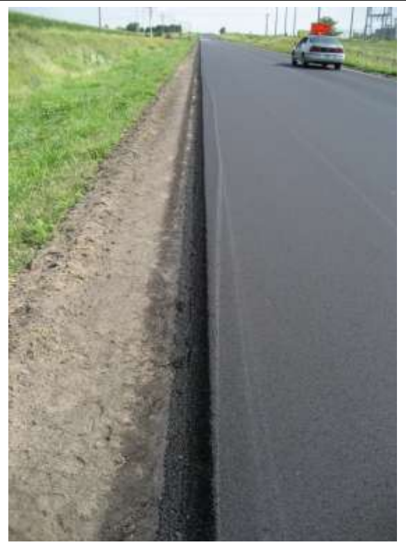
Figure 4. Graded shoulder ready for placing shoulder material.
