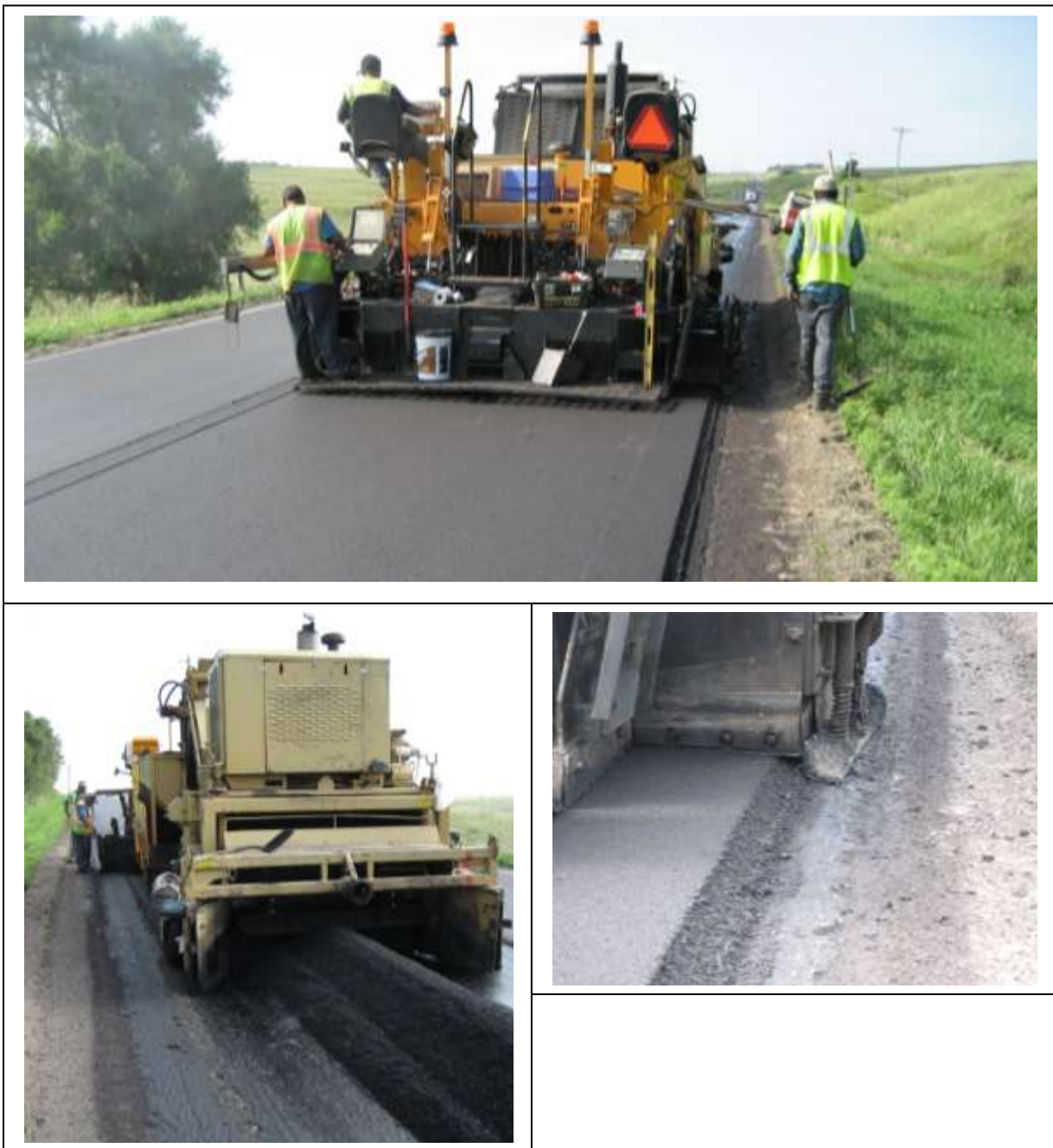
Figure 14. Equipment used to place the HMA overlay.
