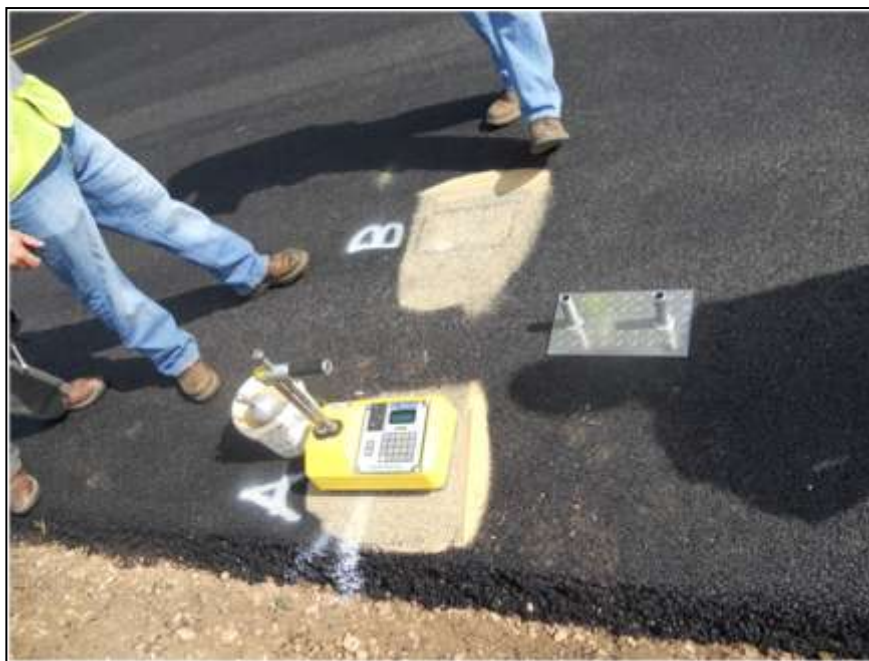
Figure 7. Nuclear gauge used to measure HMA density.
