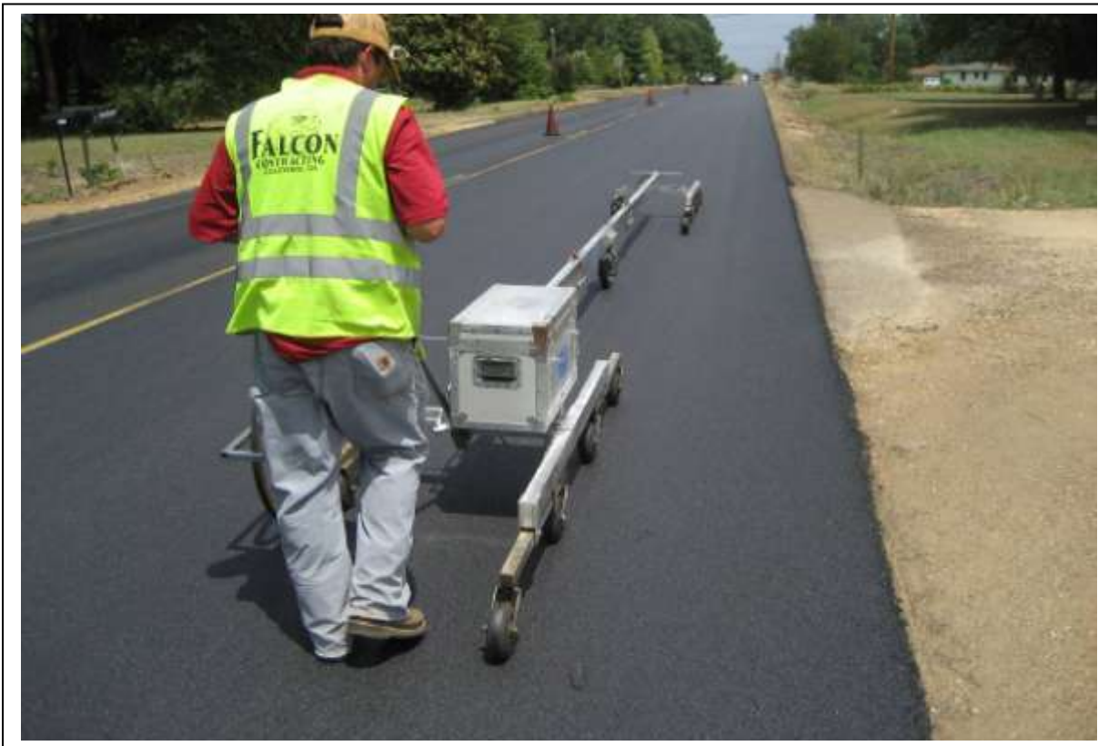
Figure 24. Longitudinal Profile Testing of Final Surface of Overlay
