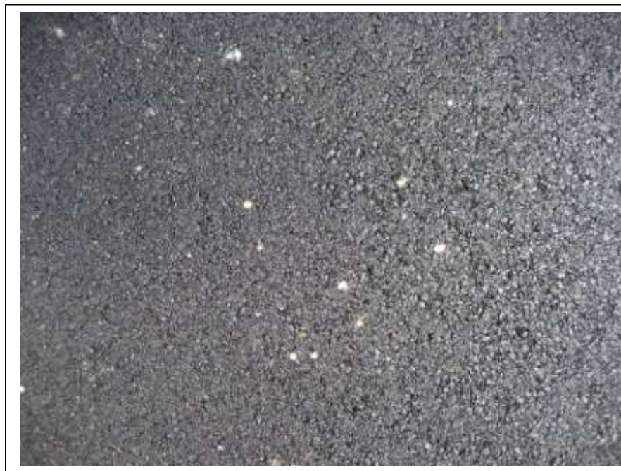
Figure 21. Surface texture of the 9.5 mm HMA overlay after final rolling.
