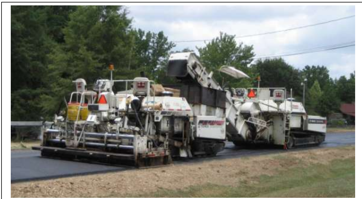
Figure 15. Equipment used to place the HMA overlay.
