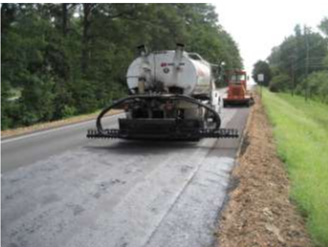
Figure 14. Surface preparation activities performed by the contractor prior to placing the HMA overlay.
