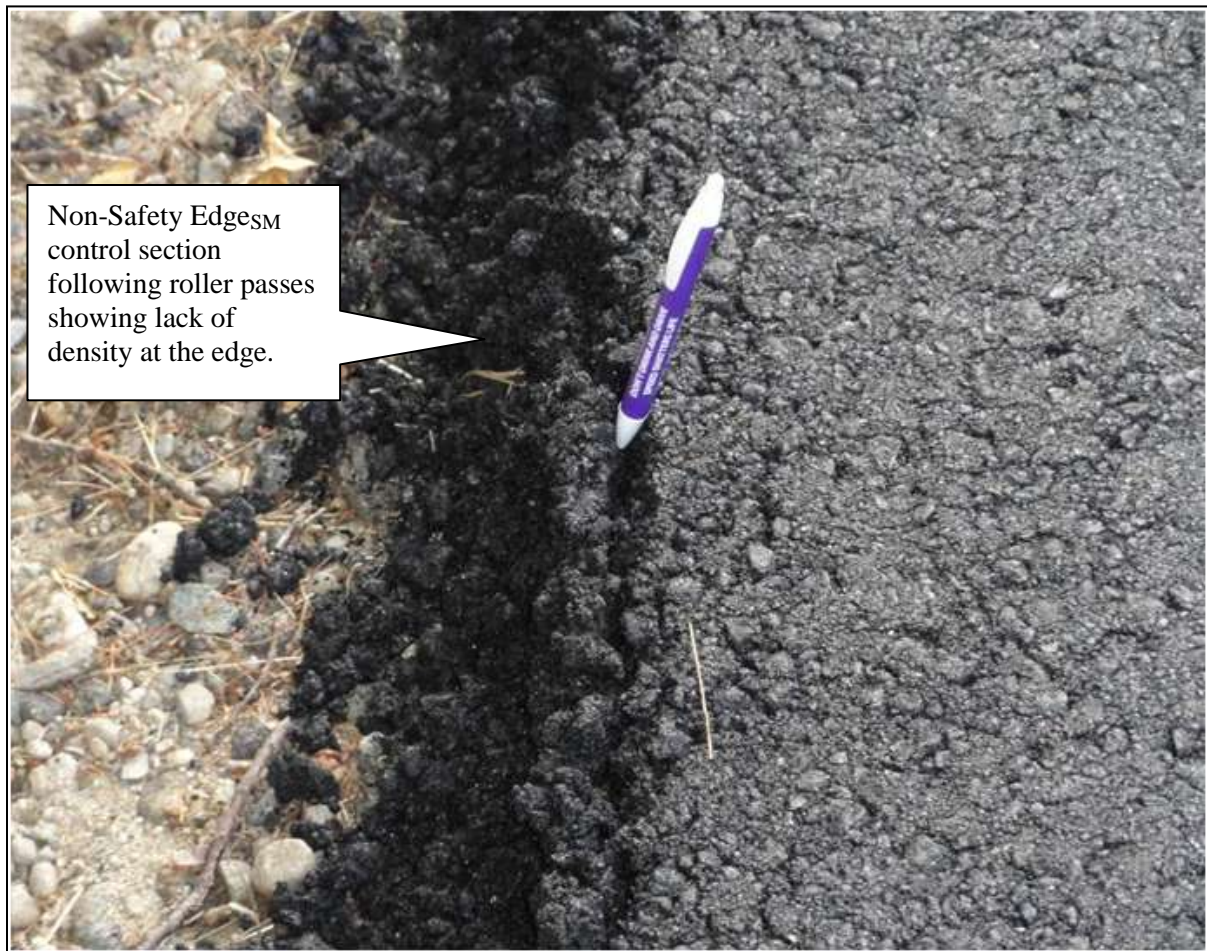
Figure 16. Non-Safety Edge SM control section showing the lack of density at edges even after roller passes.
