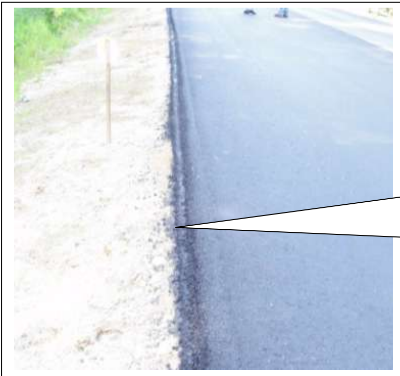
Figure 14. Both HMA lifts were paved using a Safety Edges SM device.
