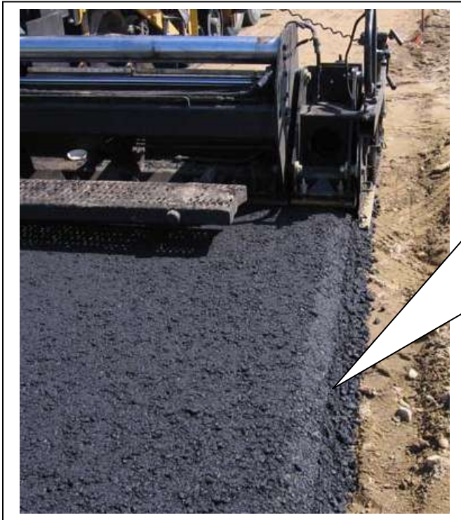
Figure 13. Paving the lower 3 inch HMA 19 mm base course with the Advant-Edger on the compacted Type D aggregate subbase.
