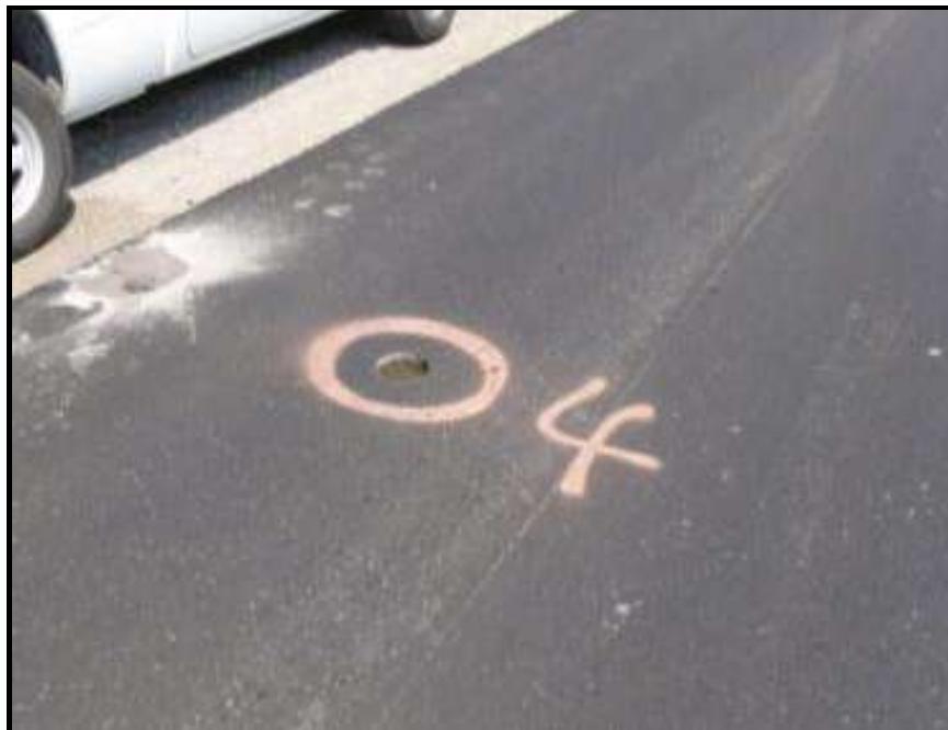
Figure 4. Safety Edge SM section with cores cut adjacent to the edge and at 3 ft. from the edge.
