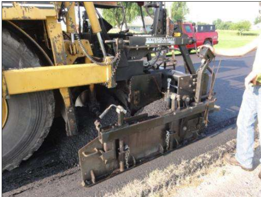
Figure 11. Blaw-Knox paver with the Caterpillar screed.
