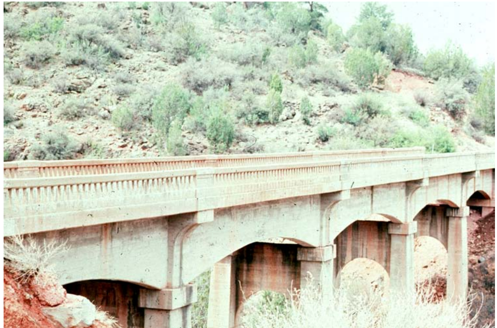
Figure 9.3.1 Concrete Deck Two-Girder Bridge
