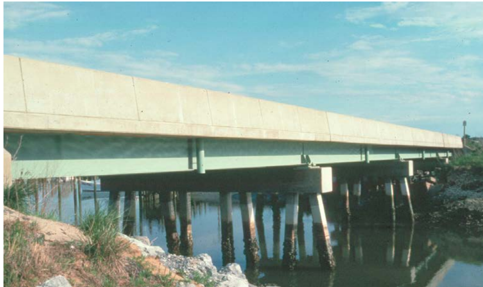
Figure 13.3.16 Concrete Pile Bent
