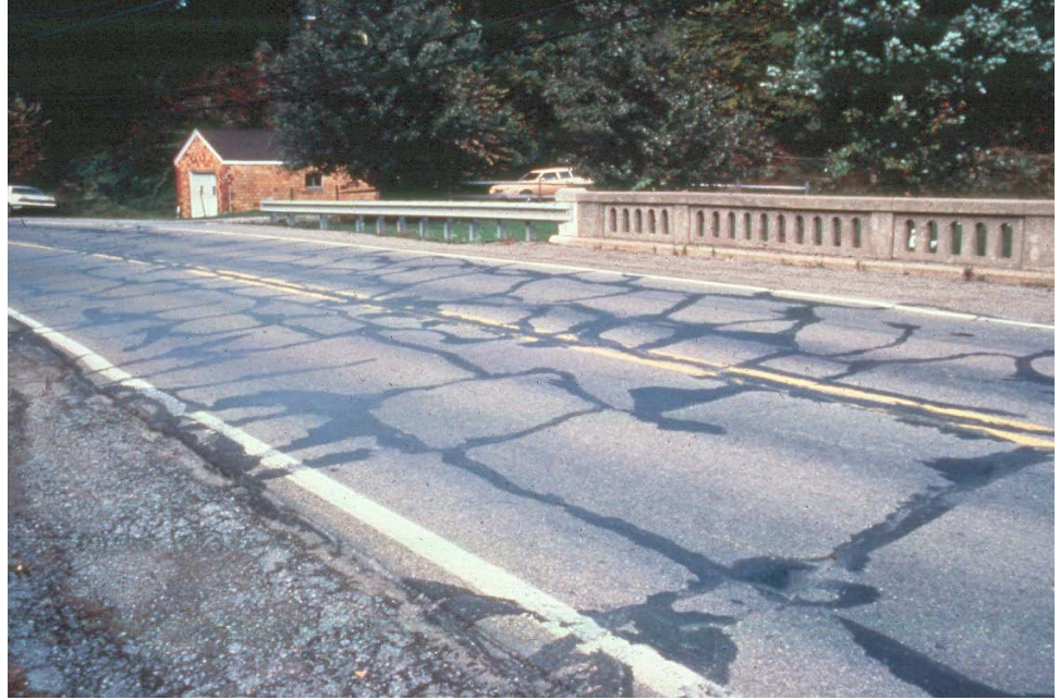
Figure 9.2.17 Asphalt Covered Tee Beam Deck
