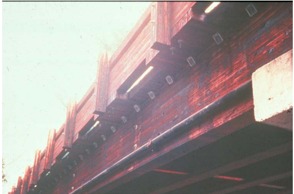
Figure 8.2.11 Elevation View of Beam of Glulam Multi-beam Bridge
