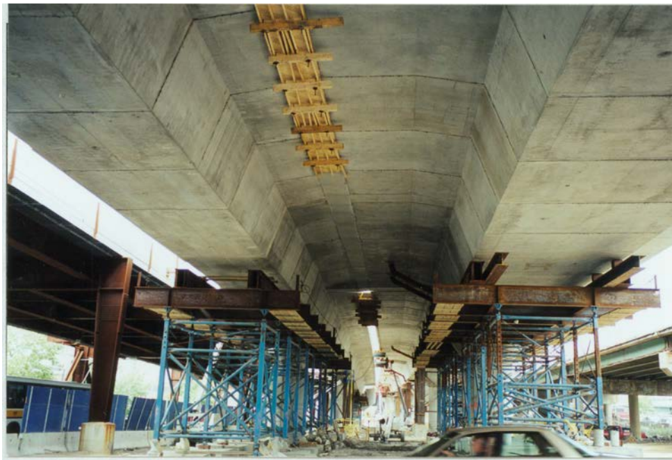
Figure 9.11.13 Adjacent Single Cell Boxes with Closure Pour
