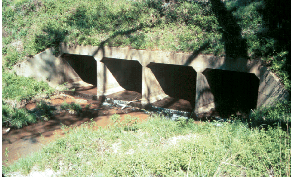
Figure 14.1.11 Multiple Cell Concrete Culvert
