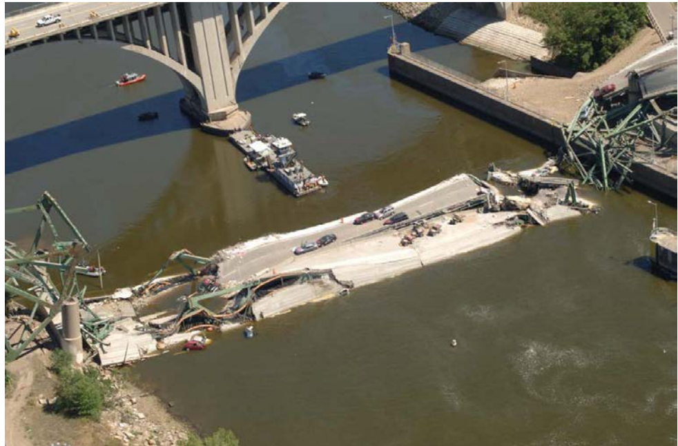
Figure 10.8.34 Collapsed I-35W Mississippi River Bridge
