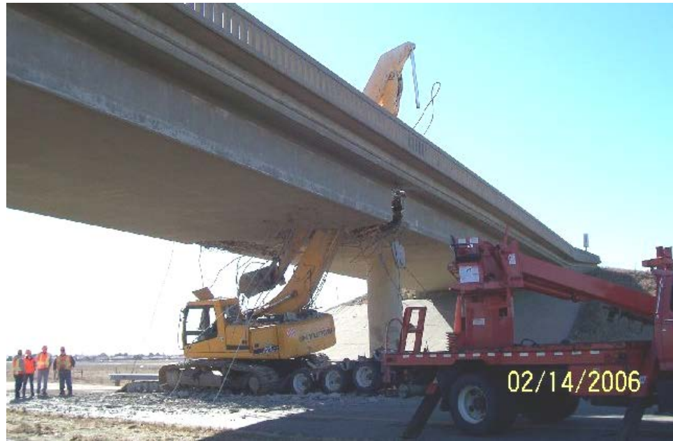
Figure 4.4.2 Accident Involving Construction Equipment and a Bridge
