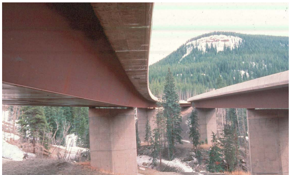
Figure 10.3.2 Curved Box Girder Bridge
