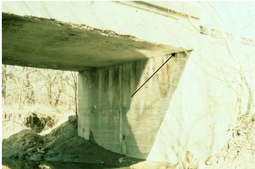
Figure 9.3.6 Bearing Area of a Through Two-Girder Bridge
