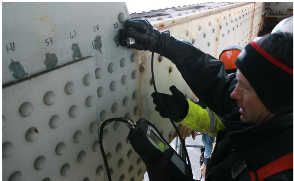
Figure 15.3.10 Ultrasonic Testing of a Gusset Plate Using a Portable UT
