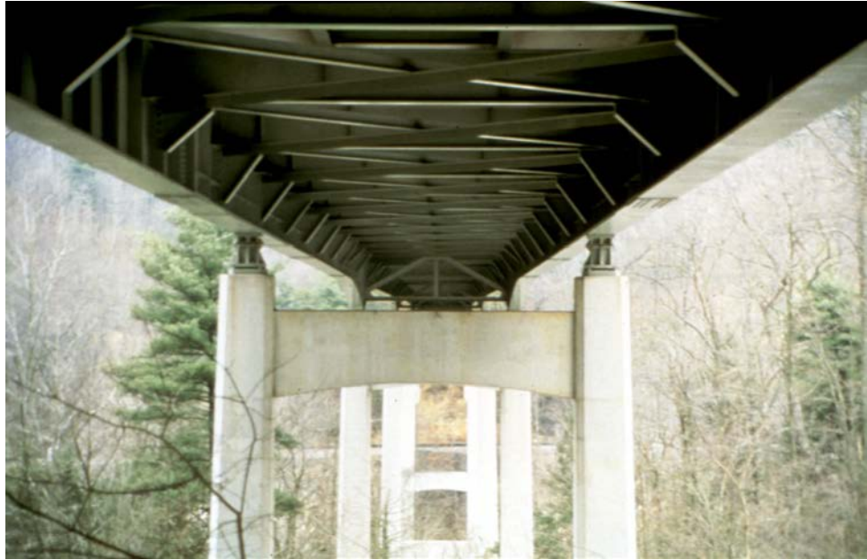
Figure 6.4.9 Non-redundant Two-Girder Bridge
