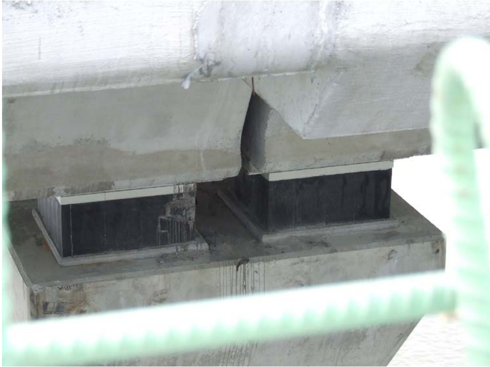
Figure 9.11.44 Segmental Box Girder Bearings at Intermediate Pier
