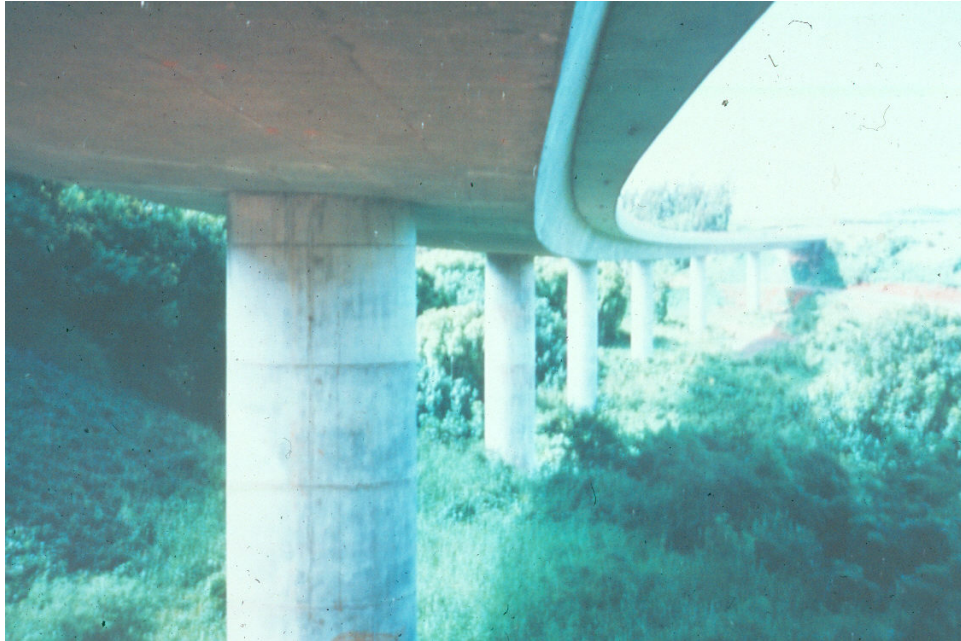
Figure 9.11.2 Cast-in-place Concrete Box Girder Bridge
