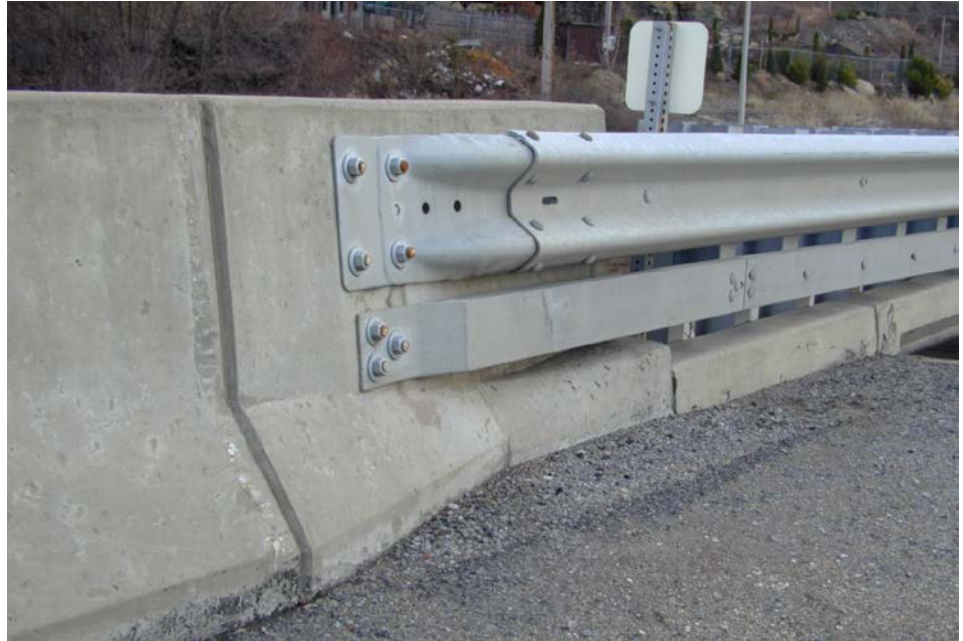
Figure 7.6.15 Proper Nesting of Guardrail at Transition
