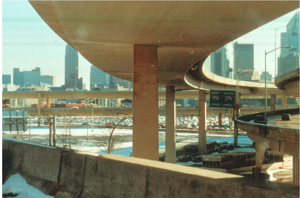
Figure 10.3.3 Box Girders With Multiple Interior Webs
