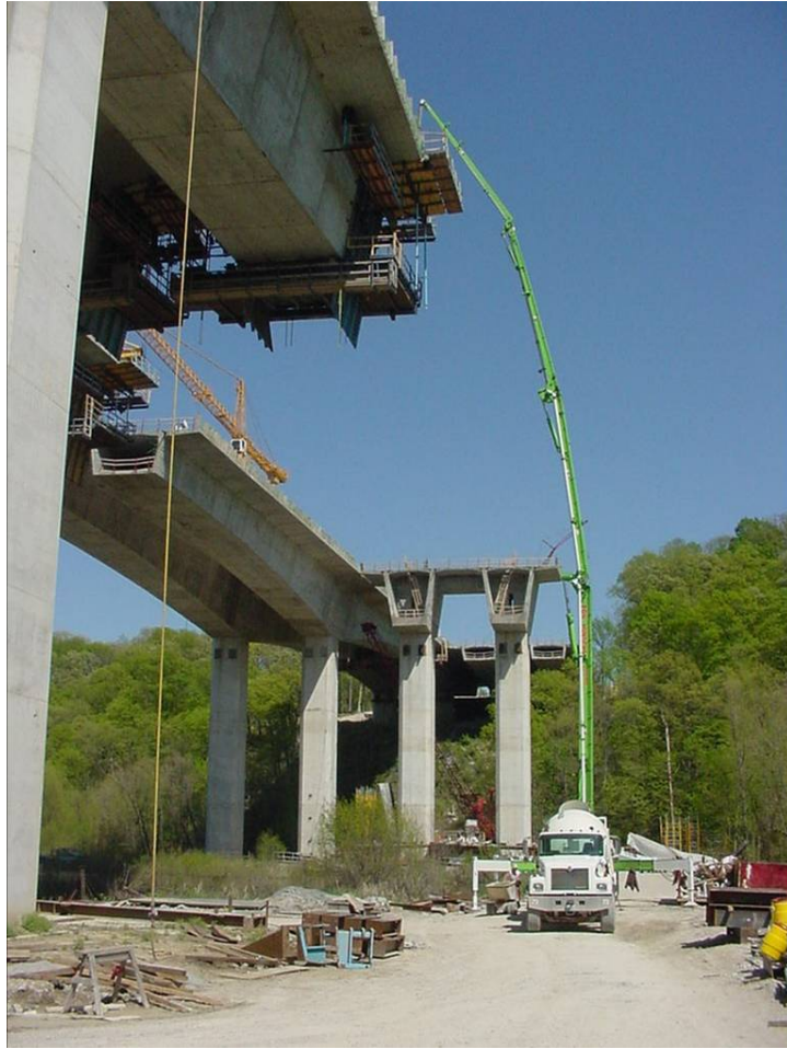
Figure 9.11.25 Progressive Placement Construction
