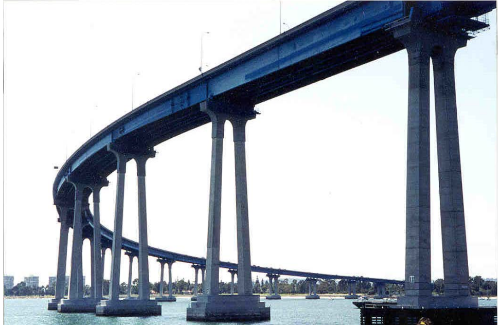
Figure 3.1.48 Curved Girder Bridge
