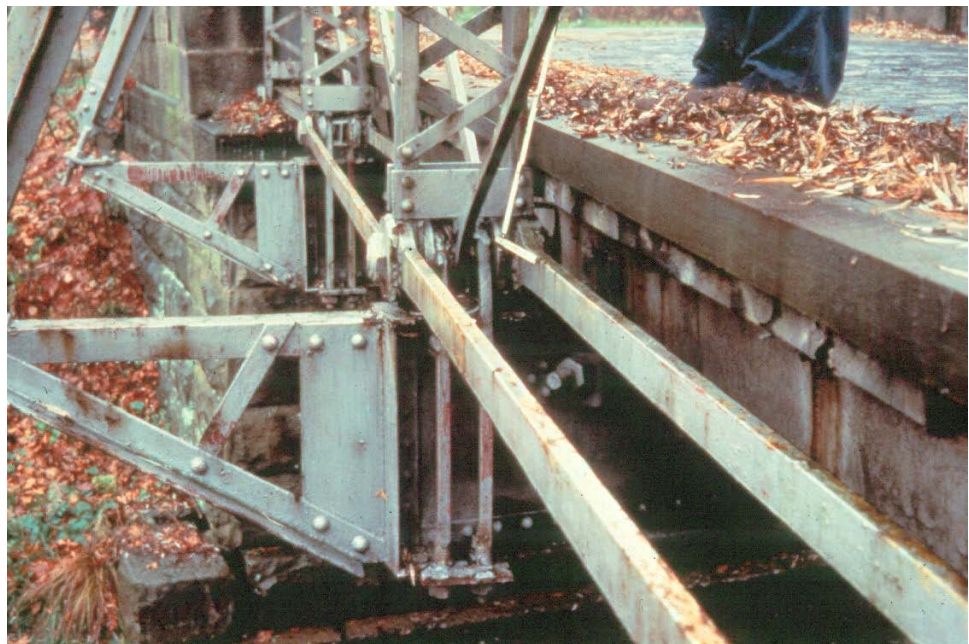
Figure 10.4.45 Bottom Chord with Eyebars
