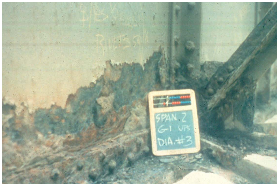
Figure 10.2.16 Lateral Bracing Connection on a Deck Girder Bridge
