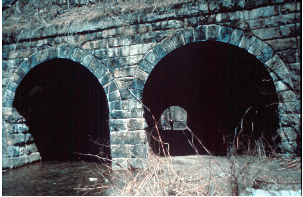
Figure 14.1.15 Stone Masonry Arch Culvert
