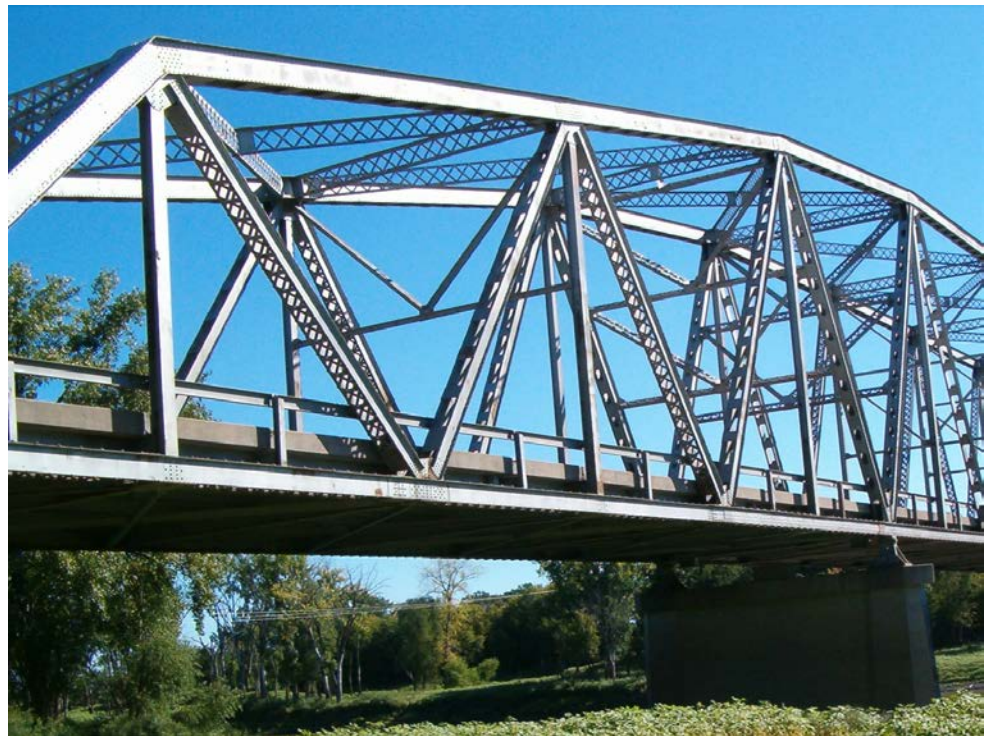
Figure 10.8.1 Steel Truss Superstructure with Gusset Plates
