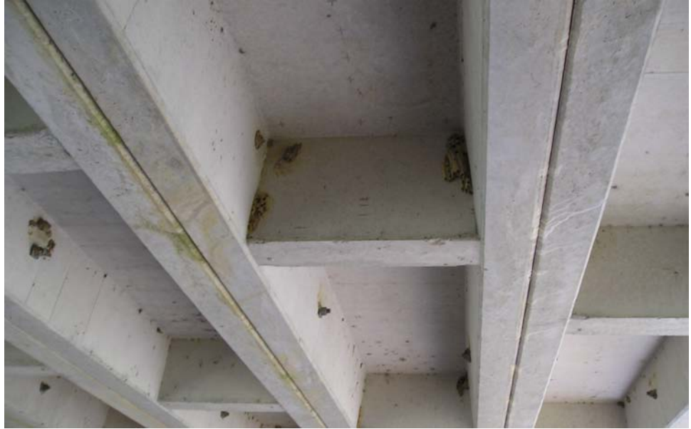
Figure 9.4.1 Underside View of Precast Channel Beam Bridge
