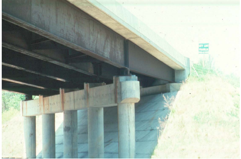
Figure 12.2.8 Column Bent or Open Bent
