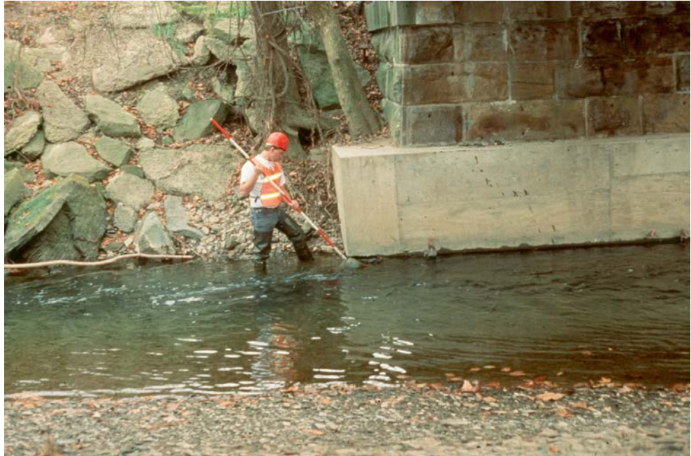
Figure 2.1.5 Inspection for Scour and Undermining
