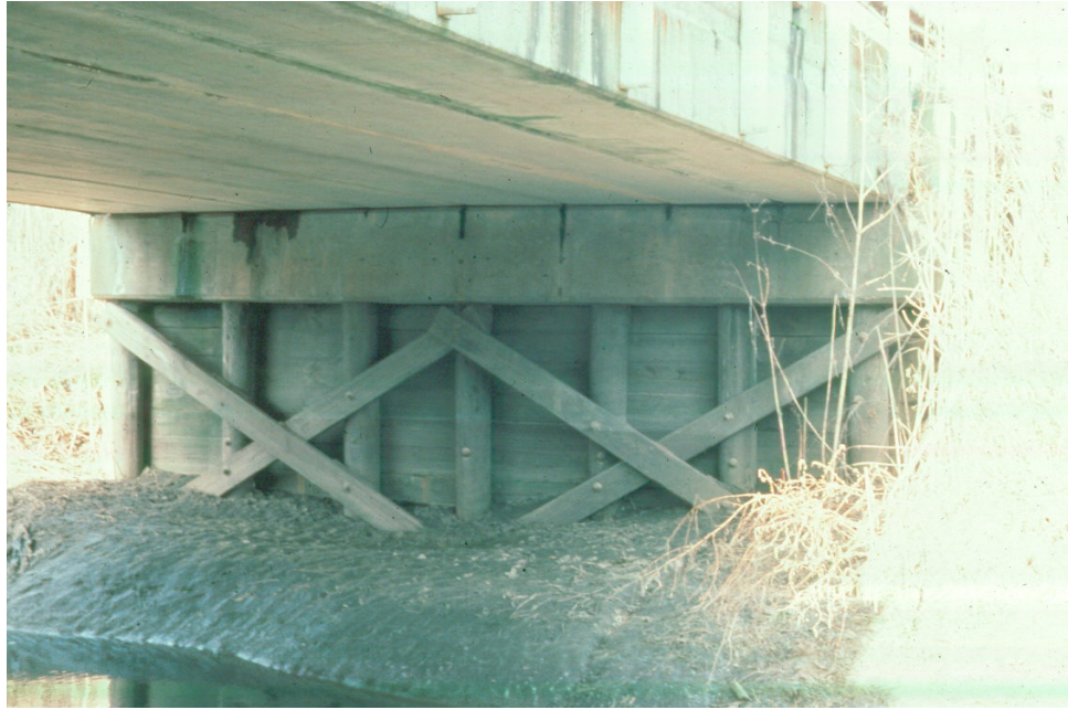
Figure 12.1.16 Combination: Timber Pile Bent Abutment with Reinforced Concrete Cap
