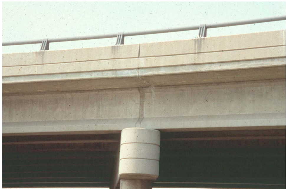
Figure 9.9.9 Continuous Prestressed I-Beam Bridge
