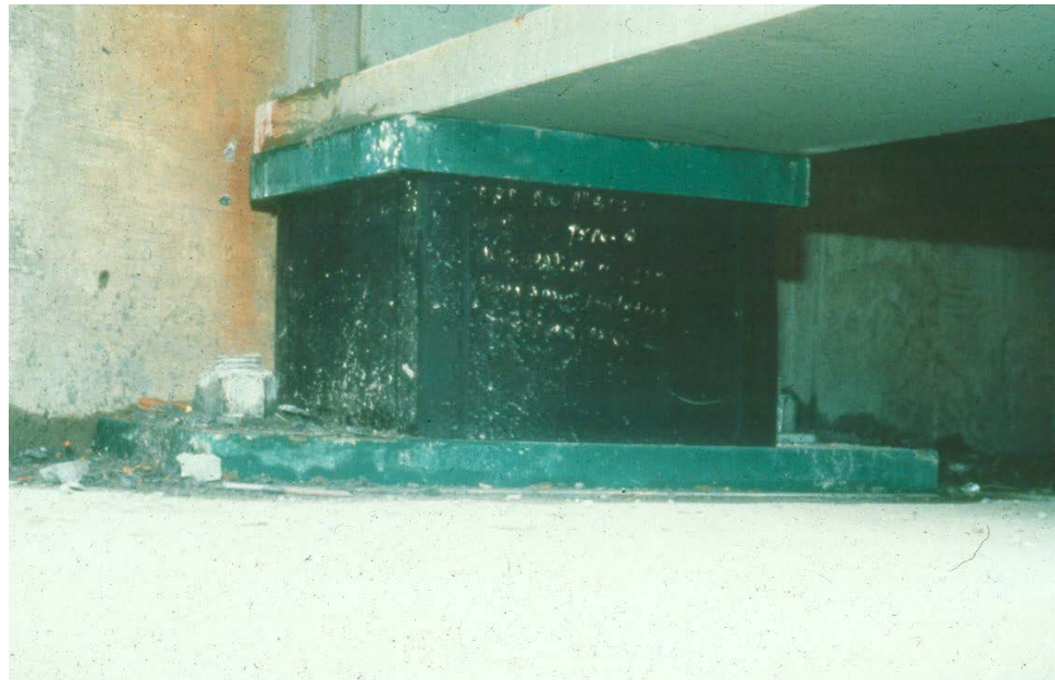
Figure 11.1.22 Lead Core Isolation Bearing
