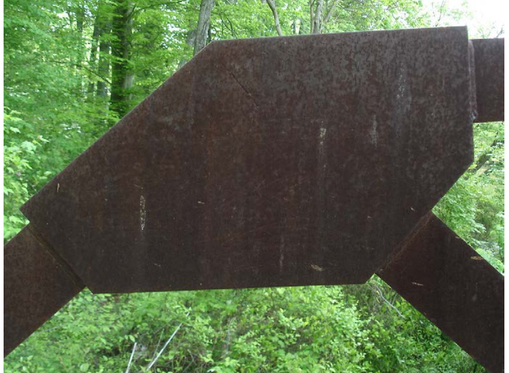
Figure 10.8.4 Steel Gusset Plate with Welded Connections
