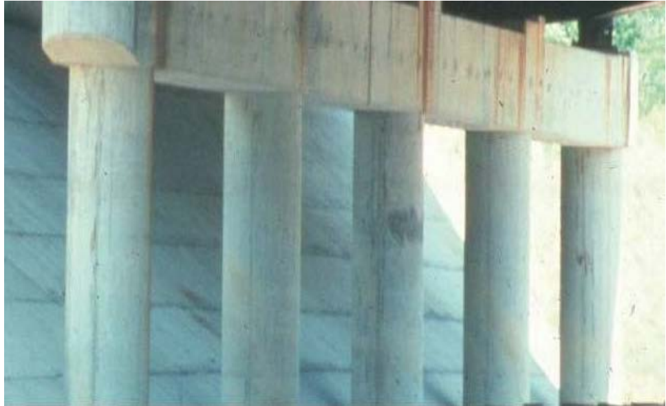
Figure 6.2.1 Round Concrete Members
