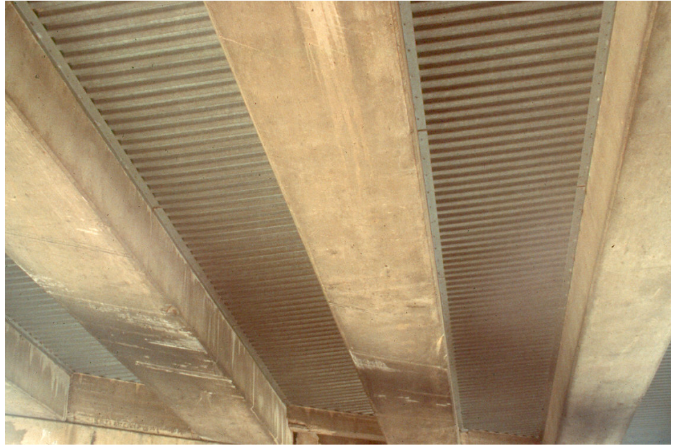
Figure 9.10.7 Underside of a Typical Spread Box Beam
