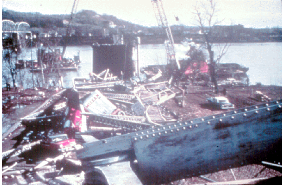
Figure 10.9.5 Collapsed Silver Bridge
