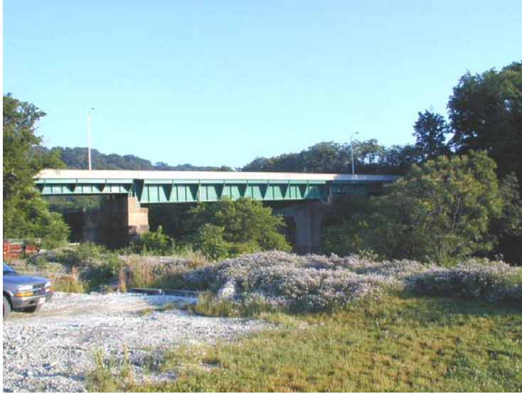
Photo No. 1 General Elevation (Upstream)
