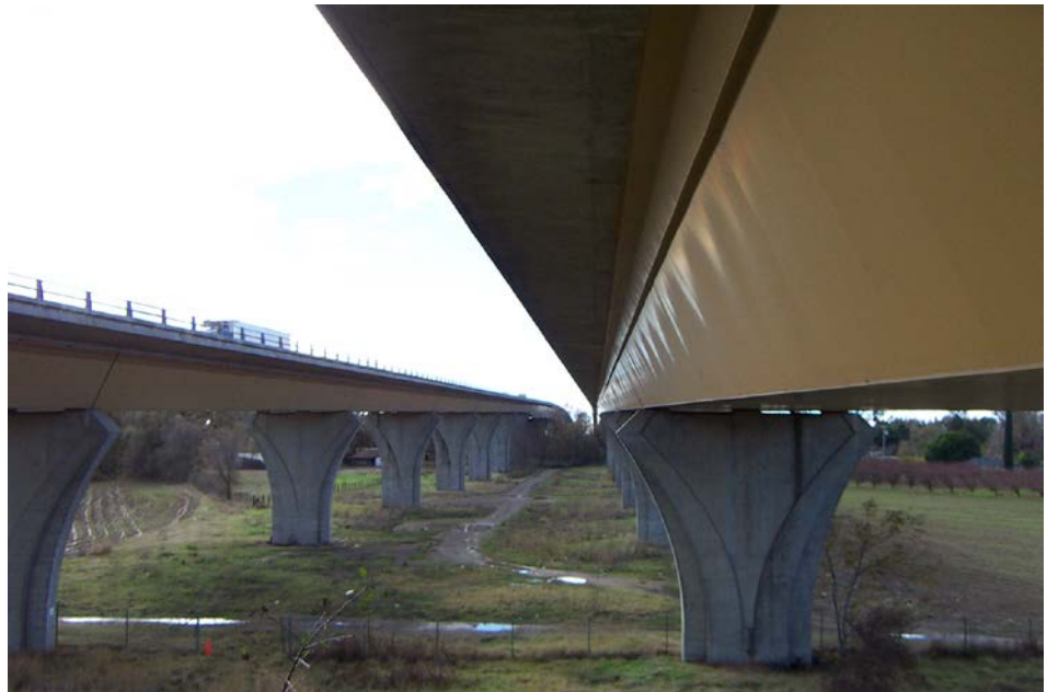
Figure 3.1.51 Box Girder Bridge
