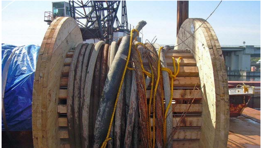
Figure 16.3.18 Frayed Cables Removed from a Floating Bridge
