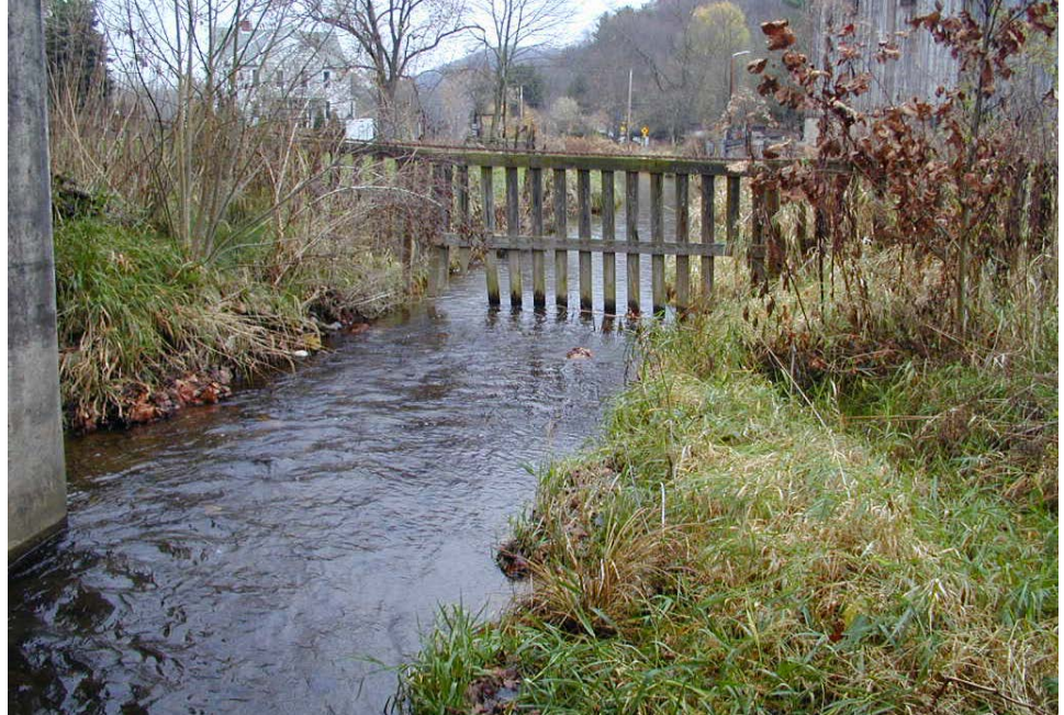
Figure 13.2.45 Fence in Stream at Bridge
