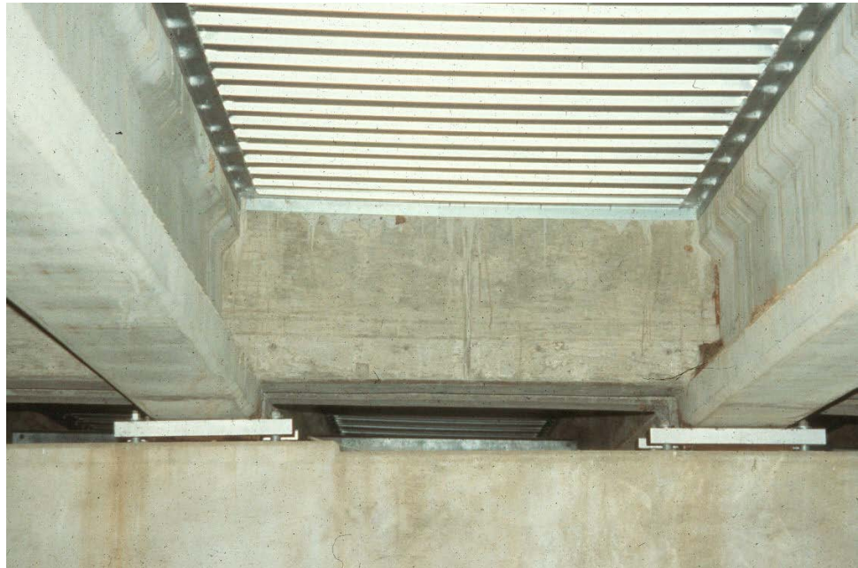
Figure 9.9.18 Concrete End Diaphragm
