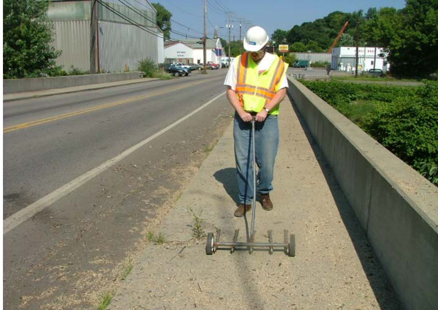
Figure 6.2.33: Inspector Using a Chain Drag
