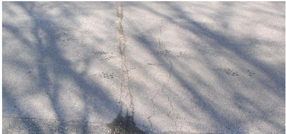
Figure 7.5.28 Asphalt Wearing Surface over an Expansion Joint
