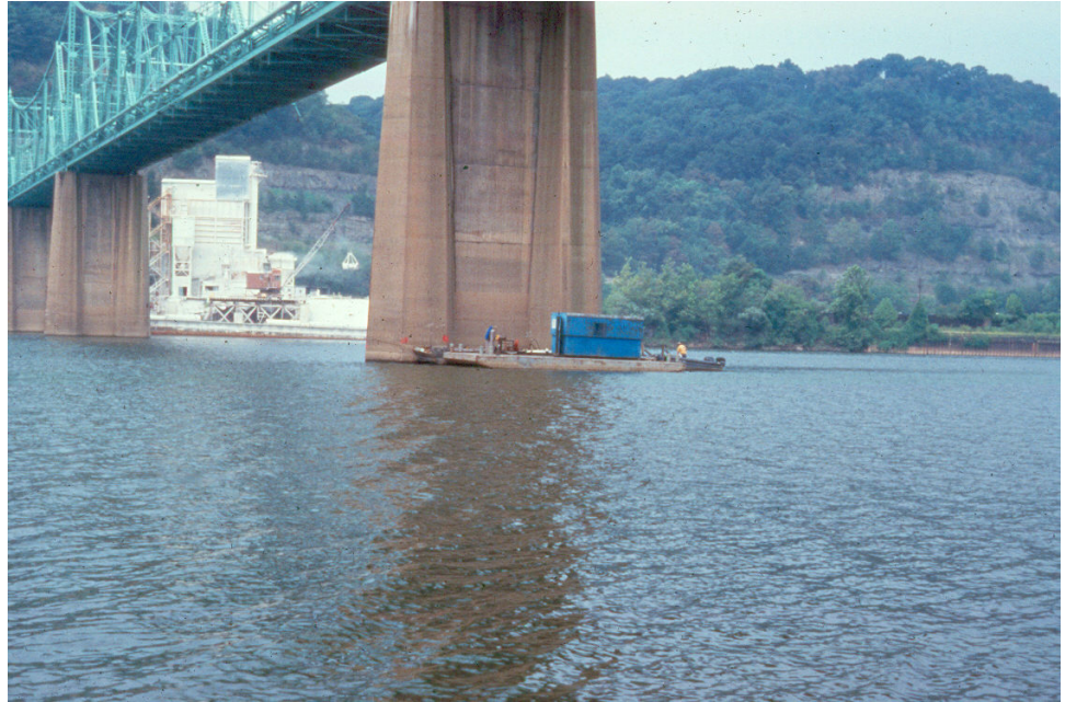
Figure 2.5.6 Inspection Operations from a Barge
