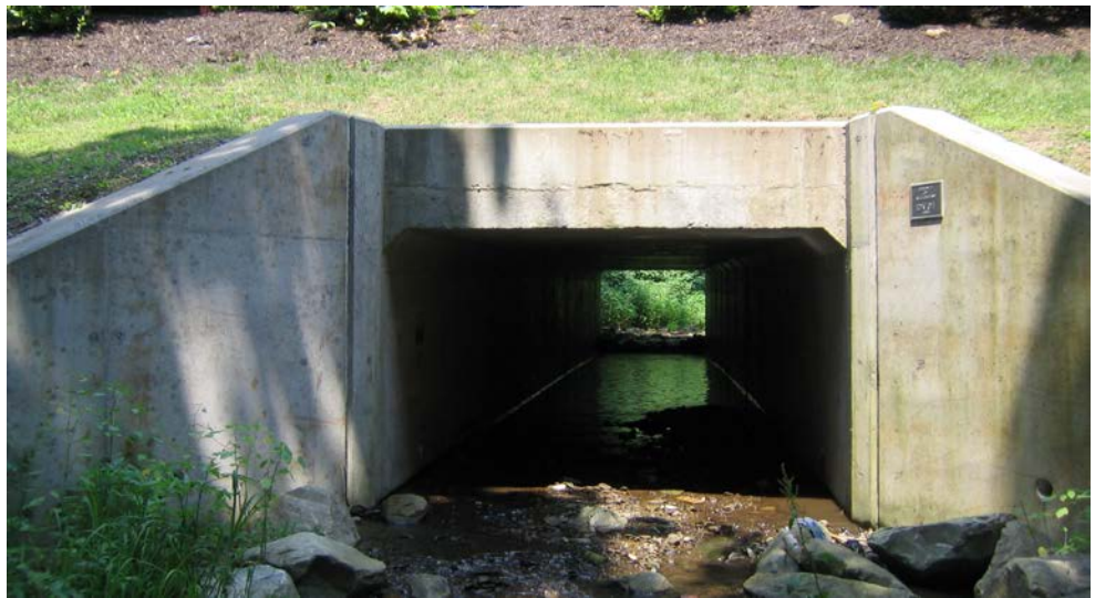
Figure 14.2.2 Concrete Box Culvert
