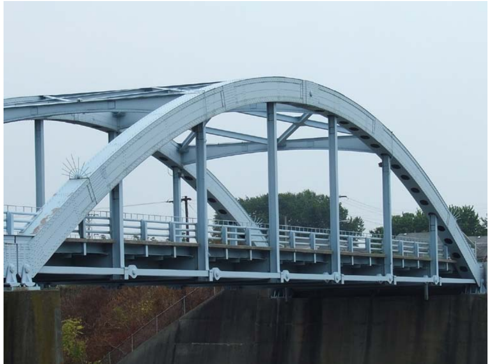
Figure 10.5.17 Tied Arch Bridge with Fracture Critical Eyebar Tie Members
