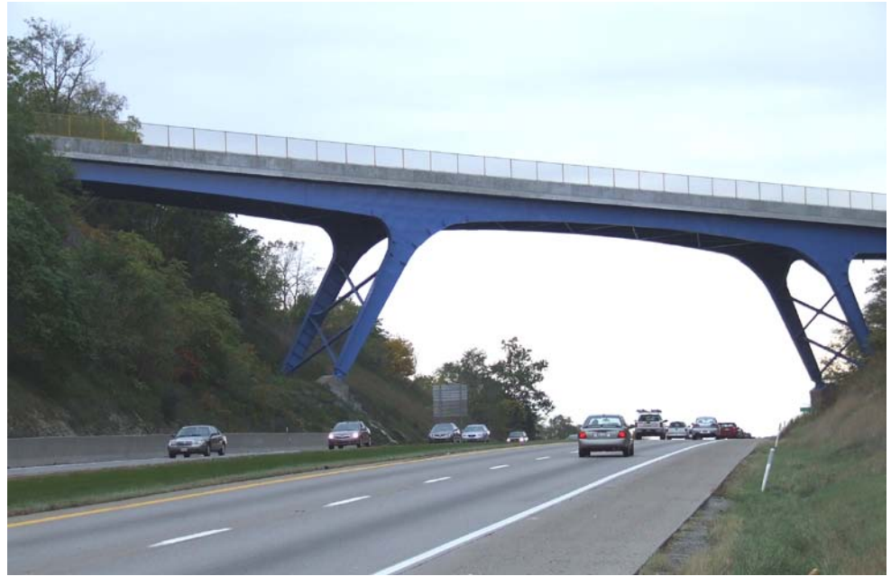
Figure 10.6.11 Fracture Critical Structure - No Load Path Redundancy
