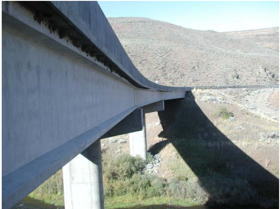
Figure 9.9.1 Prestressed I-beam Superstructure
