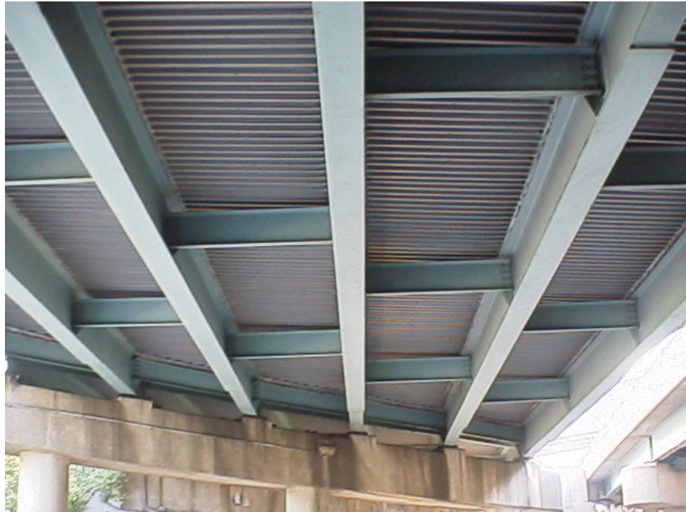
Figure 7.2.1 CIP Concrete Deck with Stay-in-Place Forms
