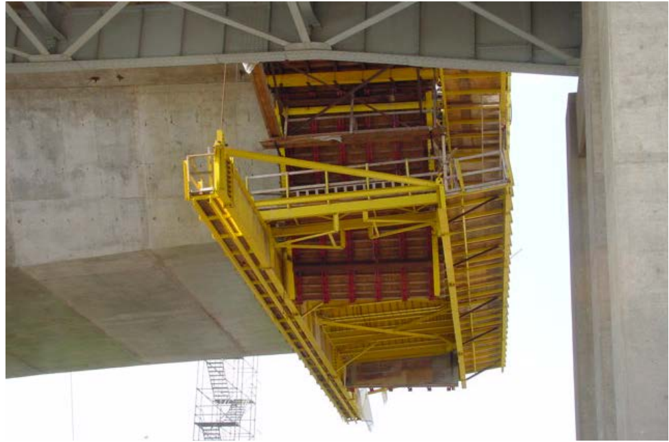
Figure 9.11.17 Cast-in-place Box Girder Segment
