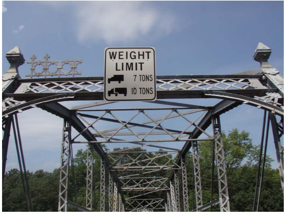
Figure 10.4.38 Portal Bracing with Attached Load Posting Sign
