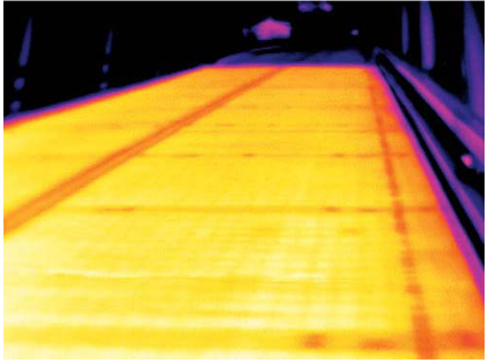
Figure 6.6.21 Thermographic Image of Bridge Deck
