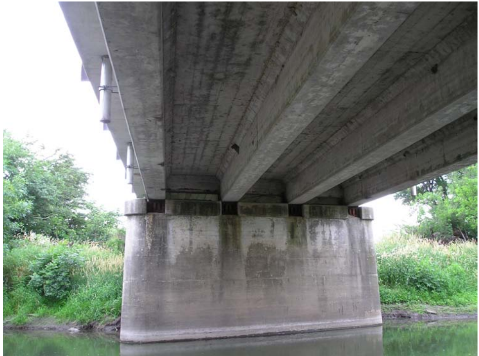
Figure 9.2.1 Simple Span Tee Beam Bridge
