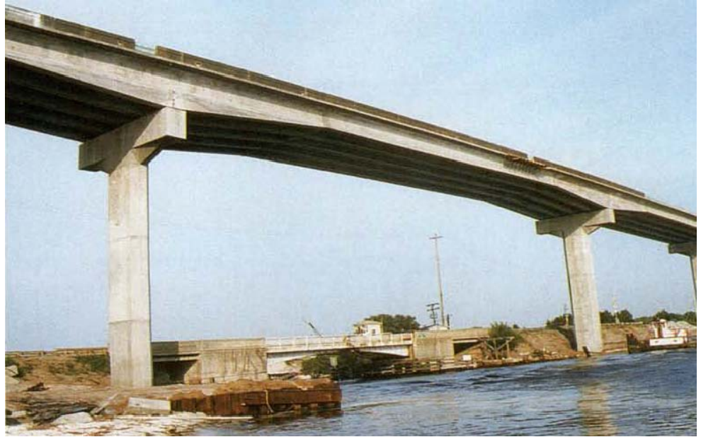
Figure 9.9.10 Spliced Bulb-Tees with Haunched Girder Sections Over Piers
