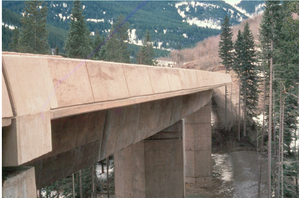
Figure 9.11.4 Cast-in-place Concrete Box Girder Bridge
