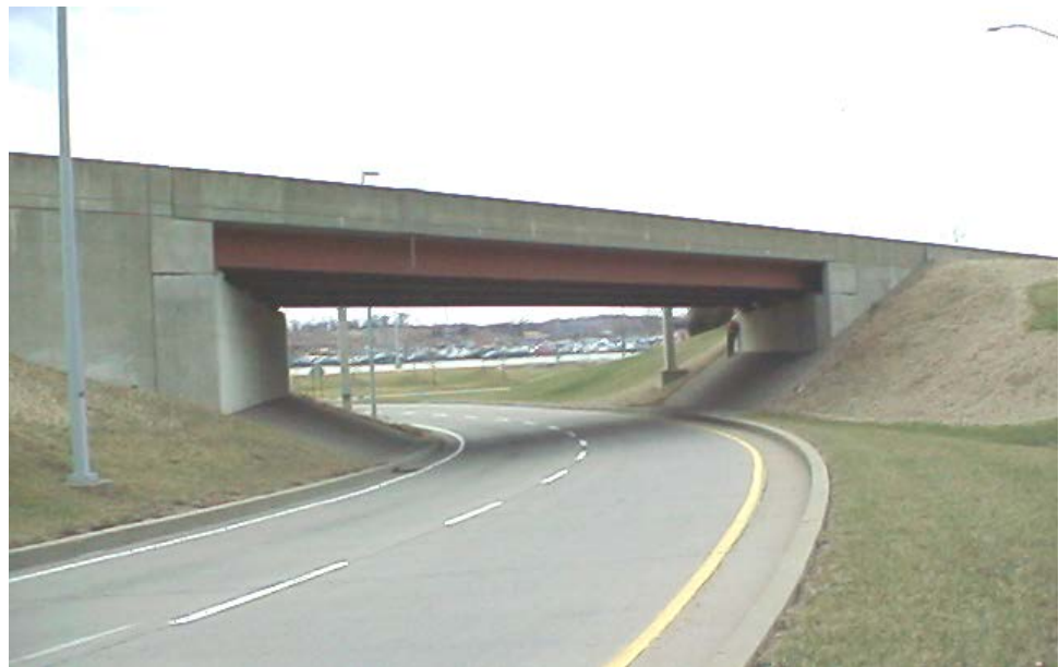
Figure 10.1.6 Single Span Fabricated Multi-girder Bridge
