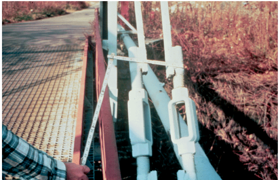
Figure 10.9.29 Welded Repair to Turnbuckles
