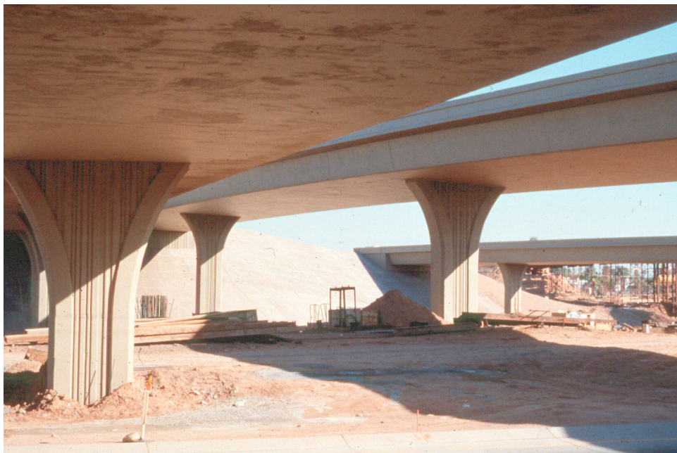
Figure 9.11.7 At-grade Casting – After Supporting Earth Removed
