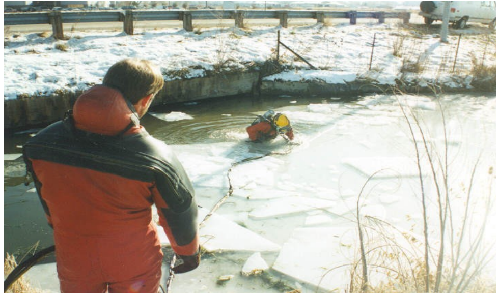
Figure 13.3.22 Inspection of Culvert With Limited Freeboard and Ice Cover
