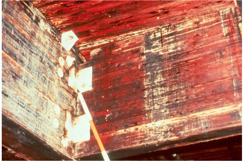
Figure 8.2.13 Typical Diaphragm for a Glulam Multi-beam Bridge
