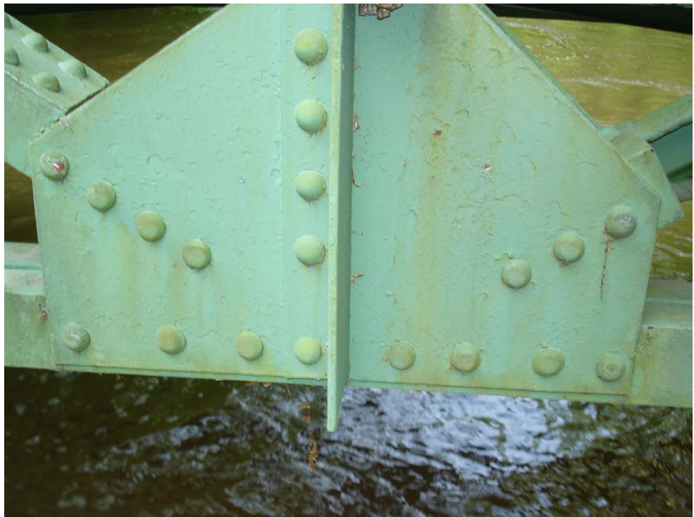
Figure 10.8.3 Steel Gusset Plate with Riveted Connections
