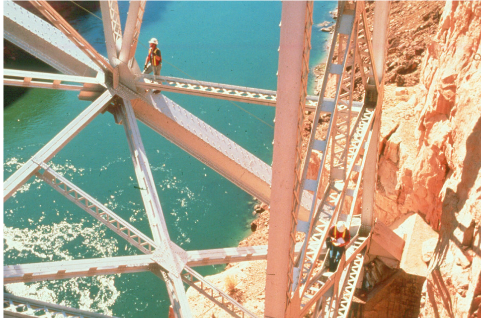
Figure 2.2.7 Inspection Involving Extensive Climbing
