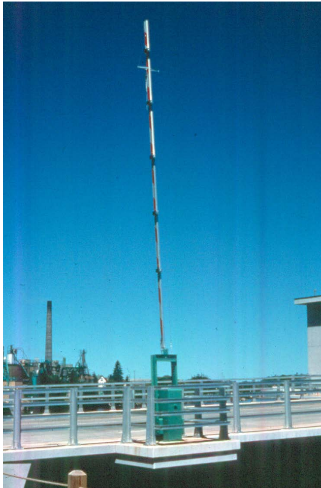
Figure 16.2.54 Traffic Control Gate
