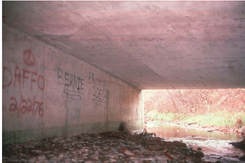
Figure 9.1.4 Bearing Area: Cast-in-Place Slab
