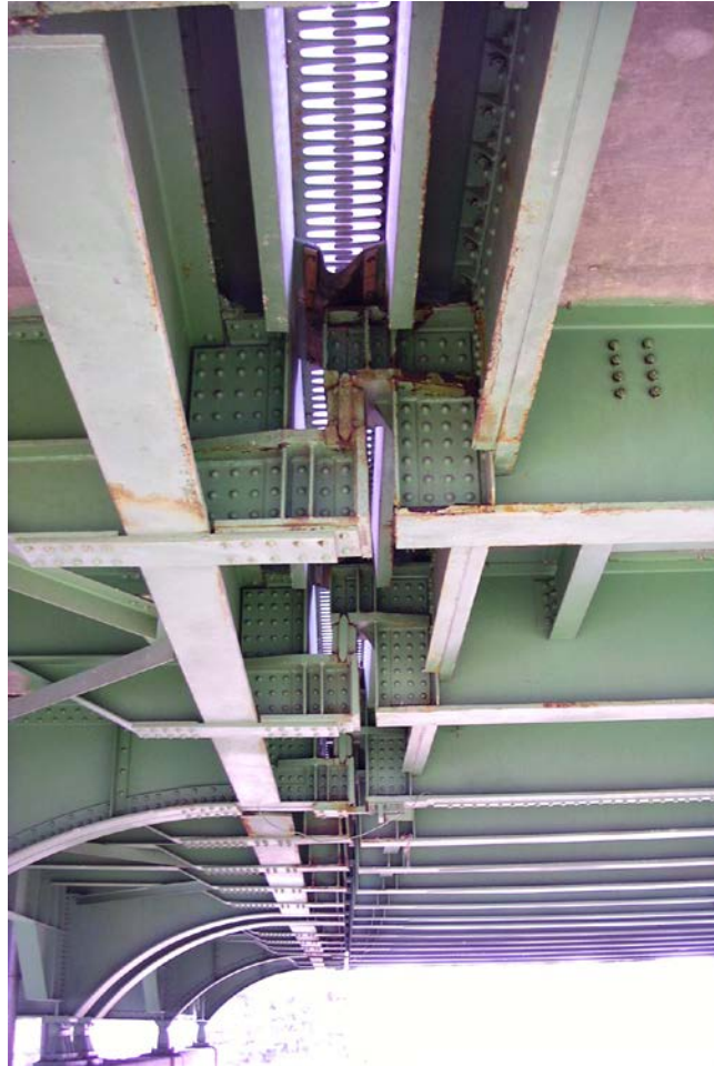
Figure 7.5.29 Support System under a Finger Plate Joint
