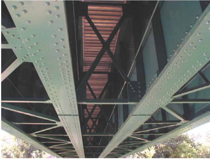
Photo No.9 General Underside View – Span 2
