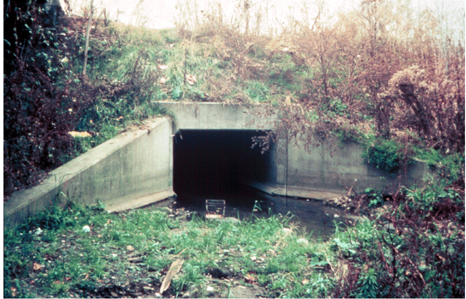
Figure 14.1.10 Concrete Box Culvert
