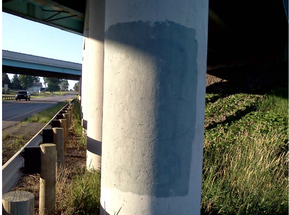
Figure 12.2.50 Repaired Concrete Column Bent
