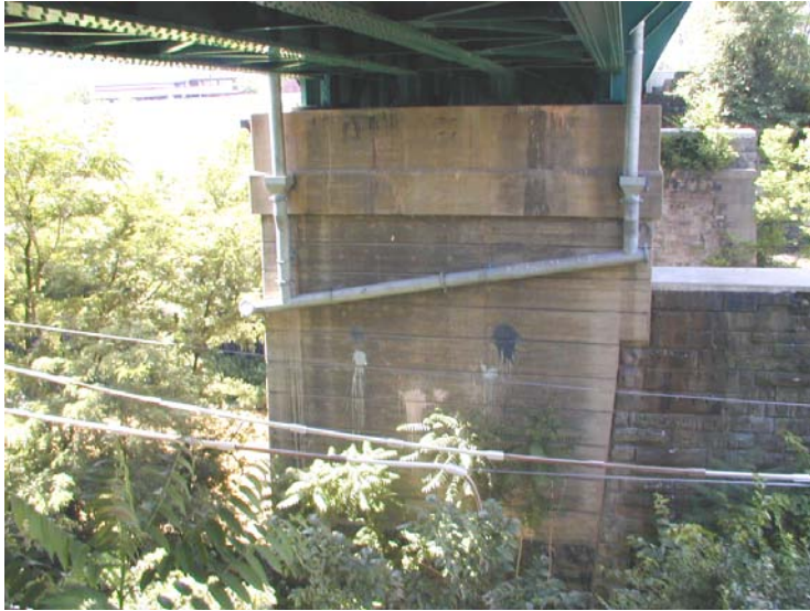
Photo No.7 Pier 2 - North Face (Looking South), note electrical lines
