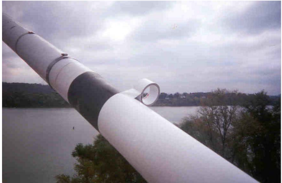
Figure 16.1.42 Cable Wrapping Placement
