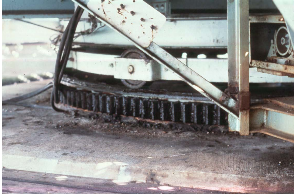
Figure 16.2.37 Balance Wheel in-place over Circular Rack
