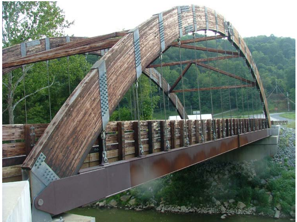
Figure 8.2.7 Glulam Arch Bridge (West Virginia)
