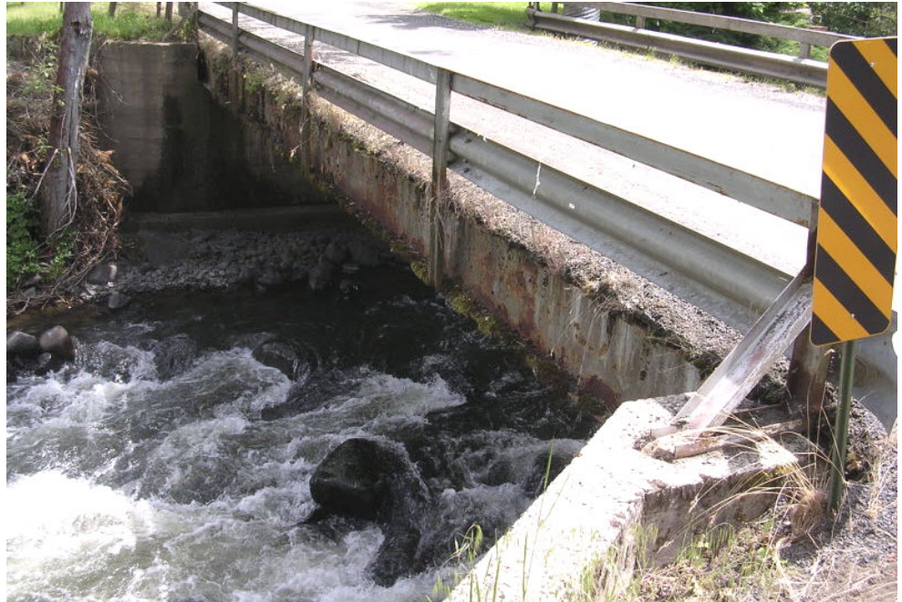
Figure 13.2.51 Fast Flowing Stream
