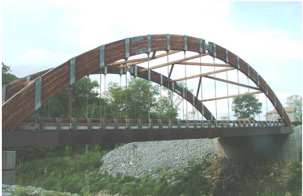
Figure 3.1.55 Through Arch Bridge
