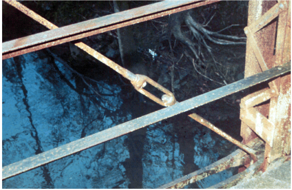
Figure 10.9.28 Turnbuckle on a Truss Diagonal
