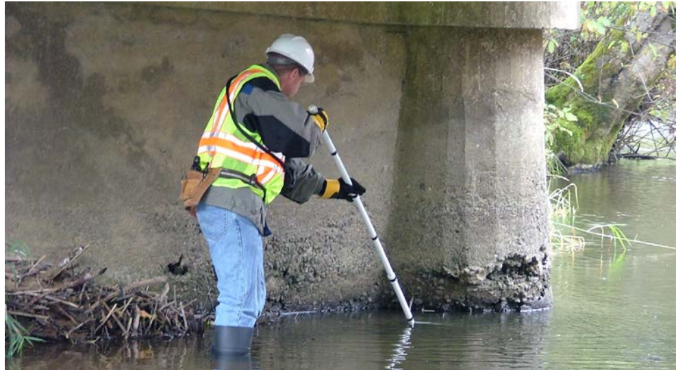
Figure 13.3.33 Inspector Performing a Wading Inspection
