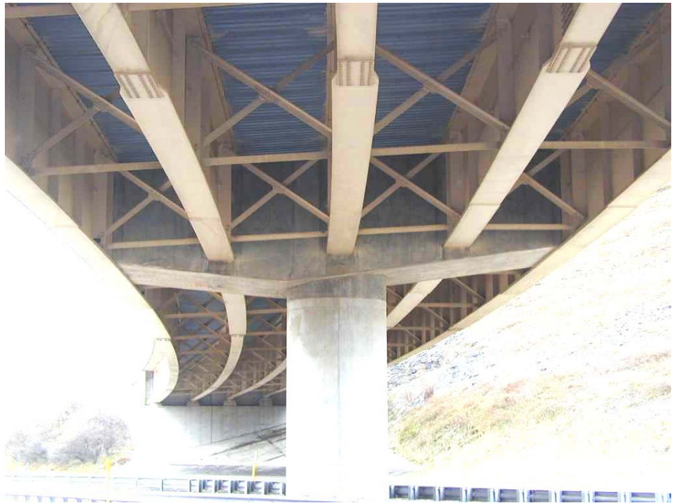
Figure 12.2.12 Integral Concrete Pier and Pier Cap
