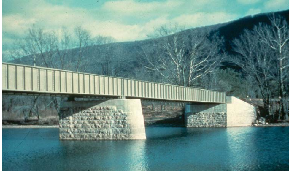
Figure 13.3.19 Solid Shaft Pier
