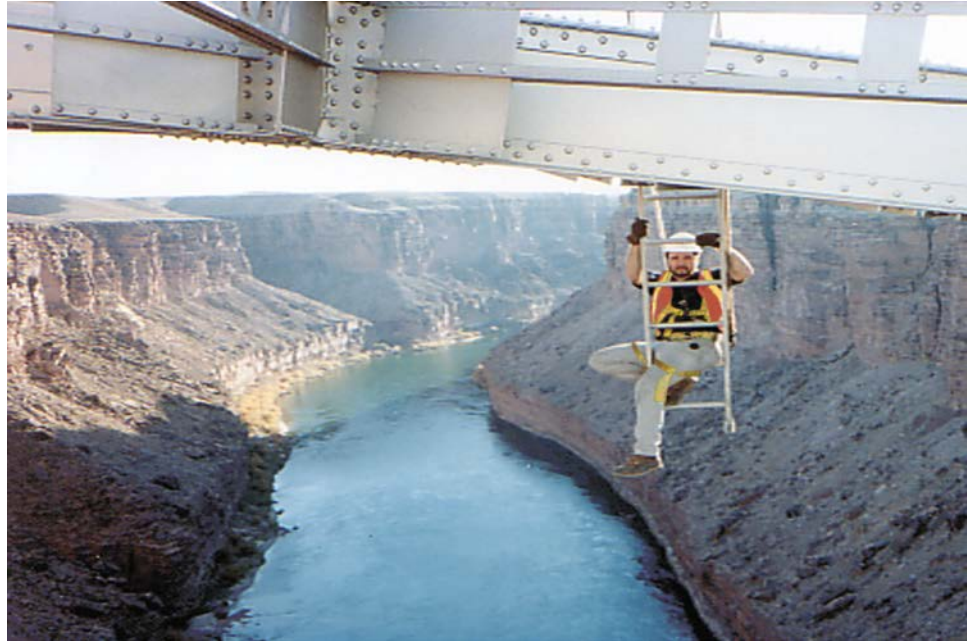
Figure 2.5.2 Inspector using a Hook-ladder
