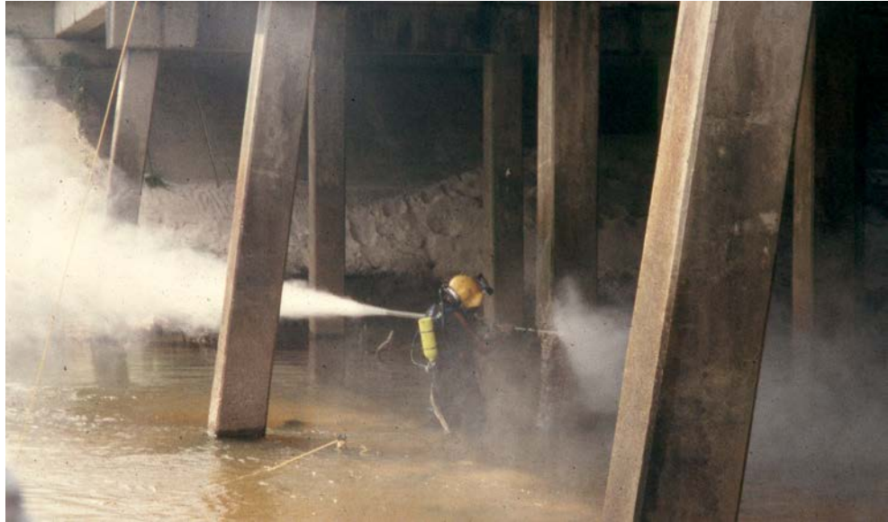
Figure 13.3.47 Cleaning with a Water Blaster
