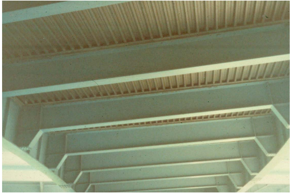
Figure 10.2.5 Two-Girder Bridge with Girder-Floorbeam System
