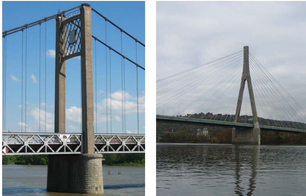
Figure 16.1.14 Tower Types: Concrete “Portal Tower” and “A-Frame Tower”
