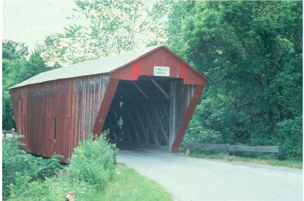
Figure 8.1.5 Town Truss Covered Bridge
