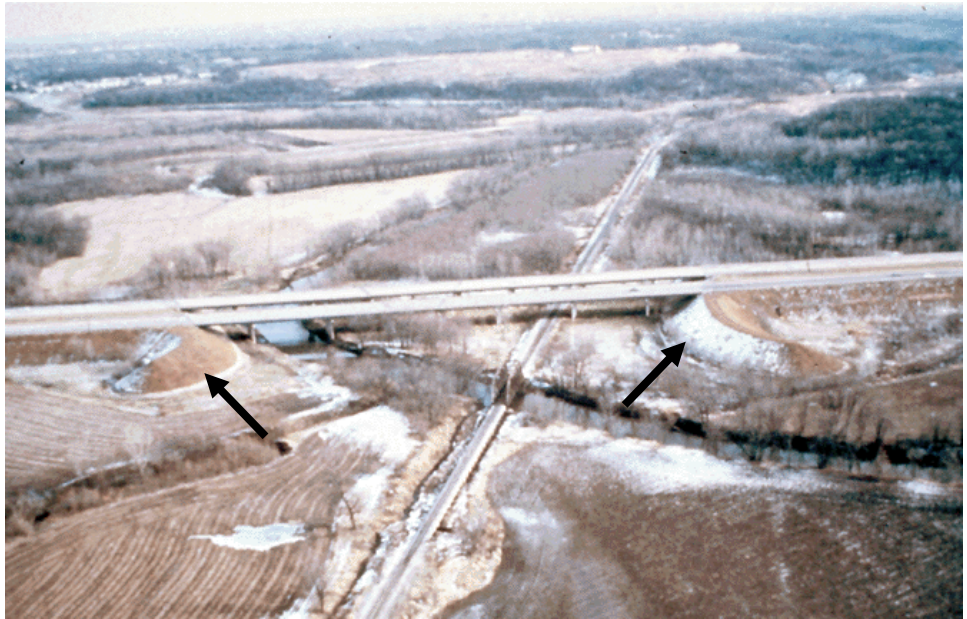
Figure 13.1.11 Guide banks Constructed on Kickapoo Creek Near Peoria, Illinois
