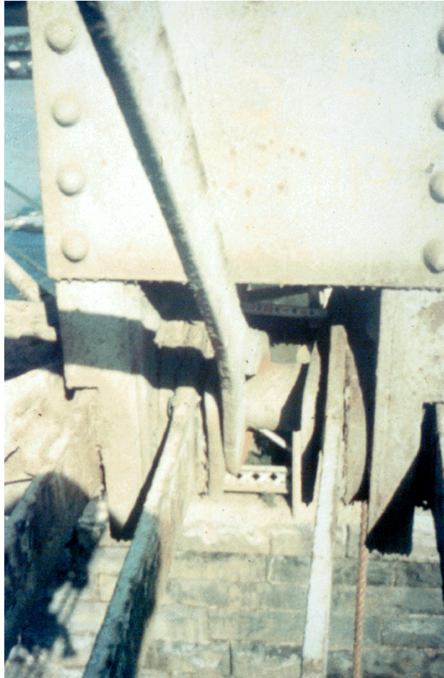
Figure 10.9.18 Non-redundant Eyebar Member
