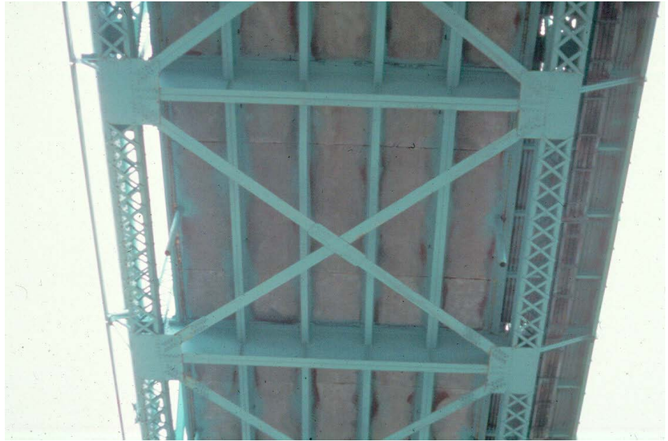
Figure 10.4.34 Lower Lateral Bracing
