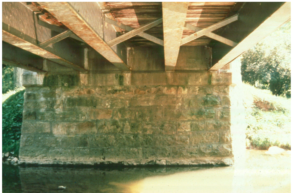
Figure 12.1.15 Stone Masonry Gravity Abutment
