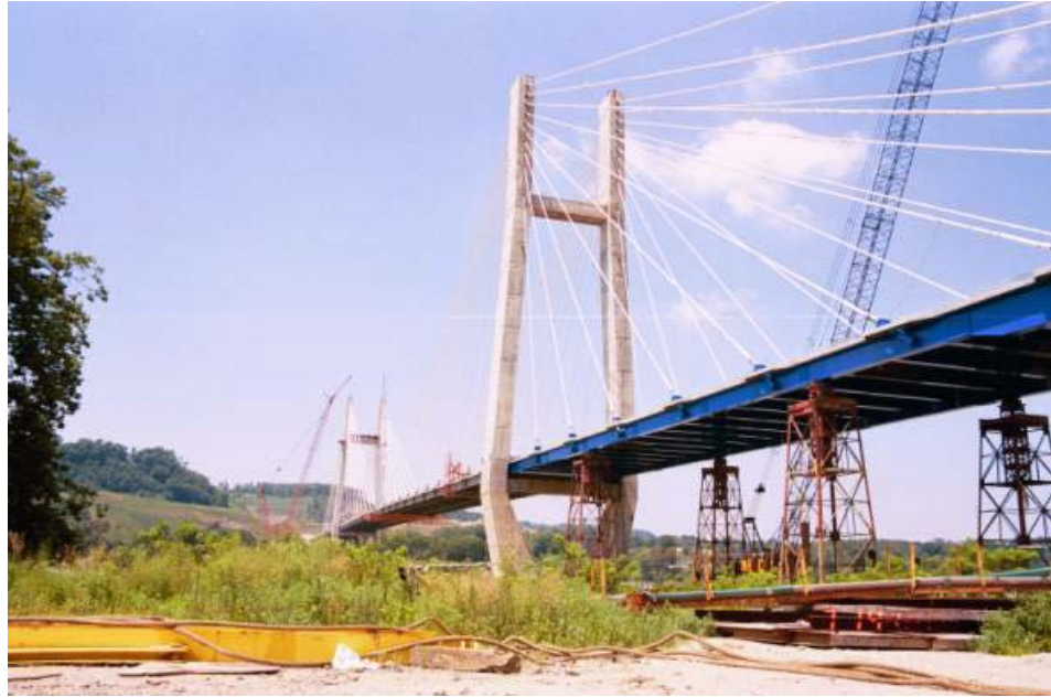
Figure 16.1.2 Maysville Cable-Stay Bridge
