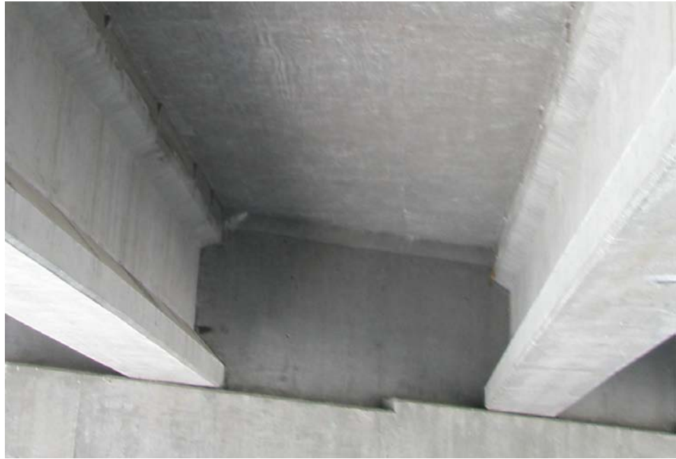
Figure 9.9.15 Bearing Area of a Typical Prestressed I-beam
