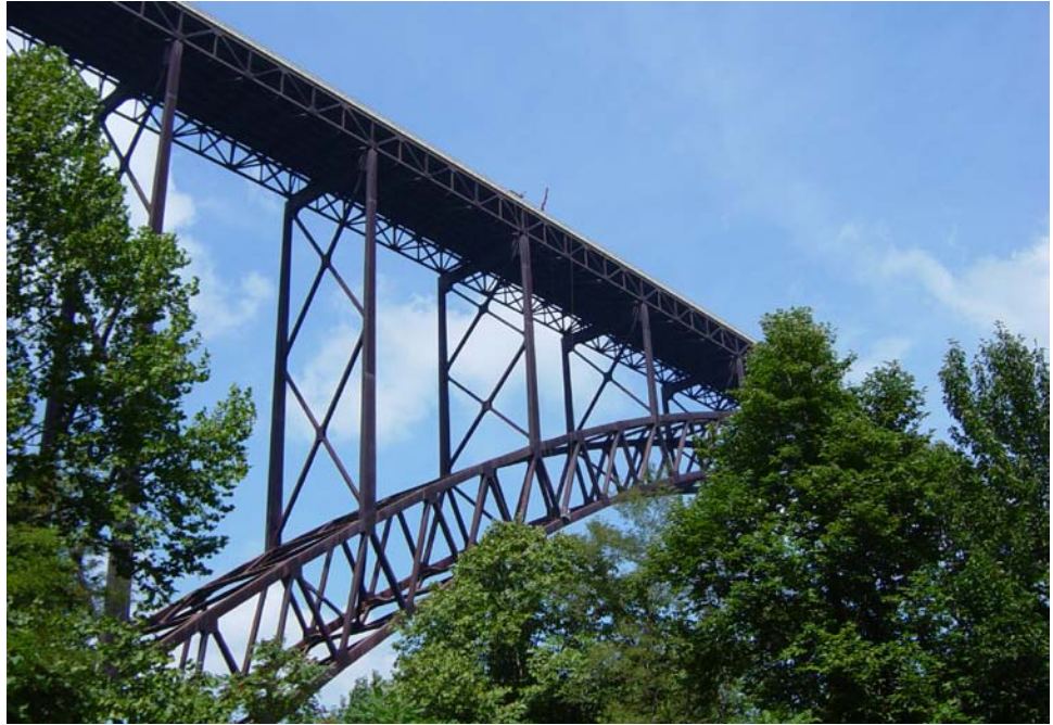
Figure 10.5.20 Braced Rib Deck Arch Showing Spandrel Columns
