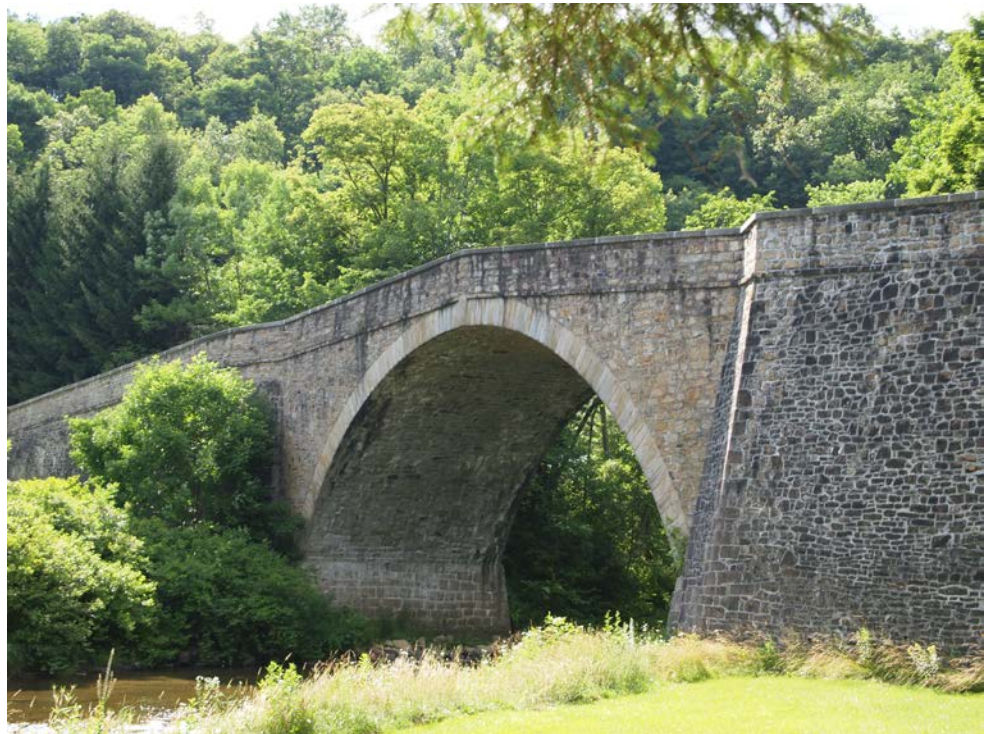
Figure 6.5.1 Stone Masonry Arch
