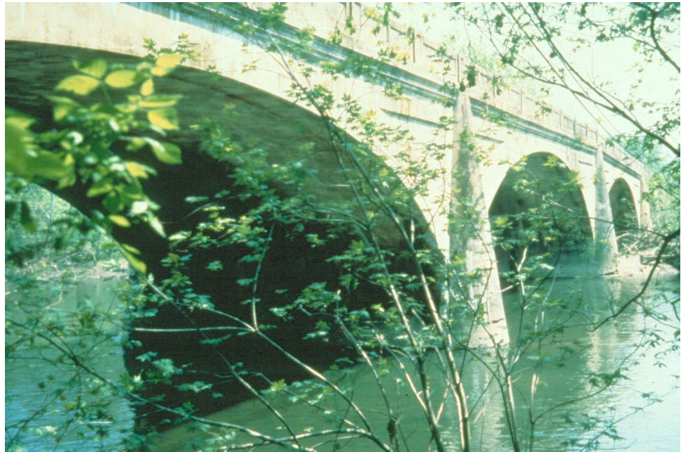
Figure 9.5.2 Multi-span Closed Spandrel Arch Bridge
