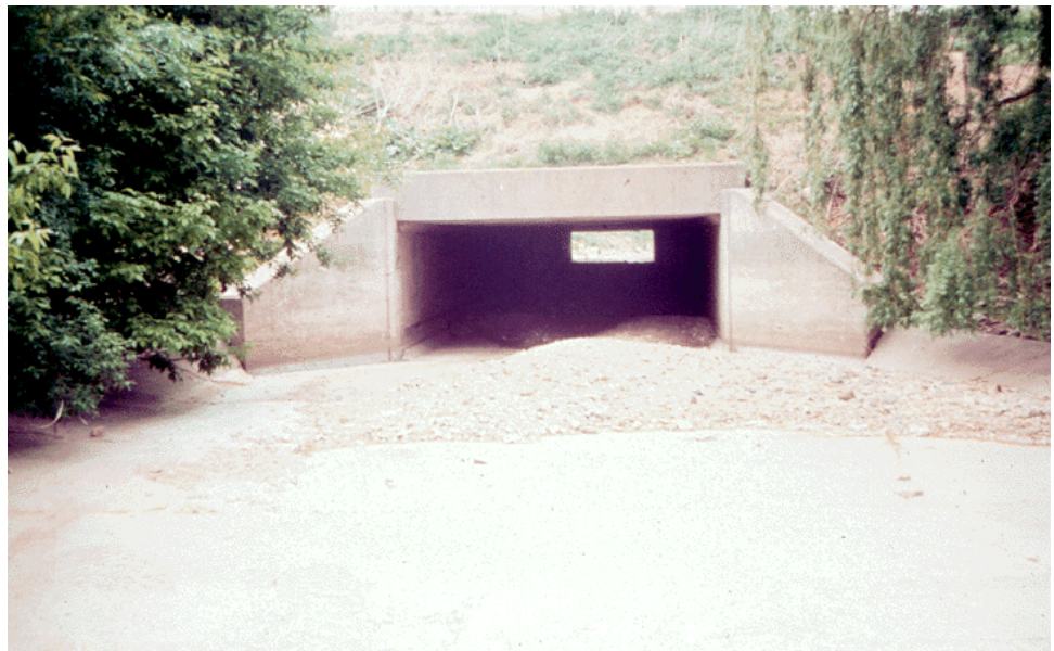
Figure 14.1.32 Headwall and Wingwall End Treatment on Box Culvert
