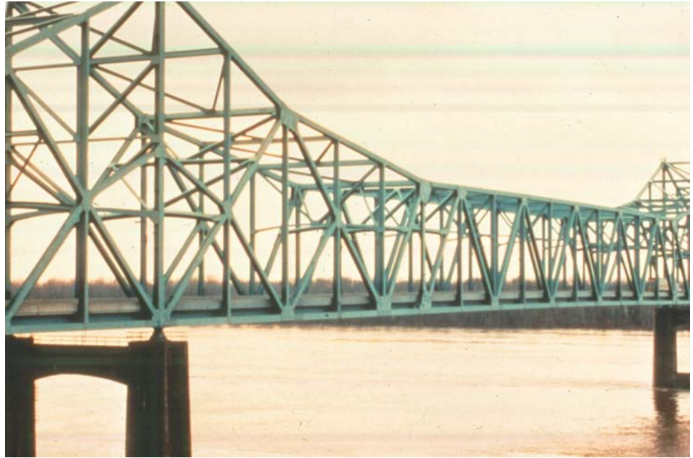
Figure 10.4.16 Cantilever Through Truss
