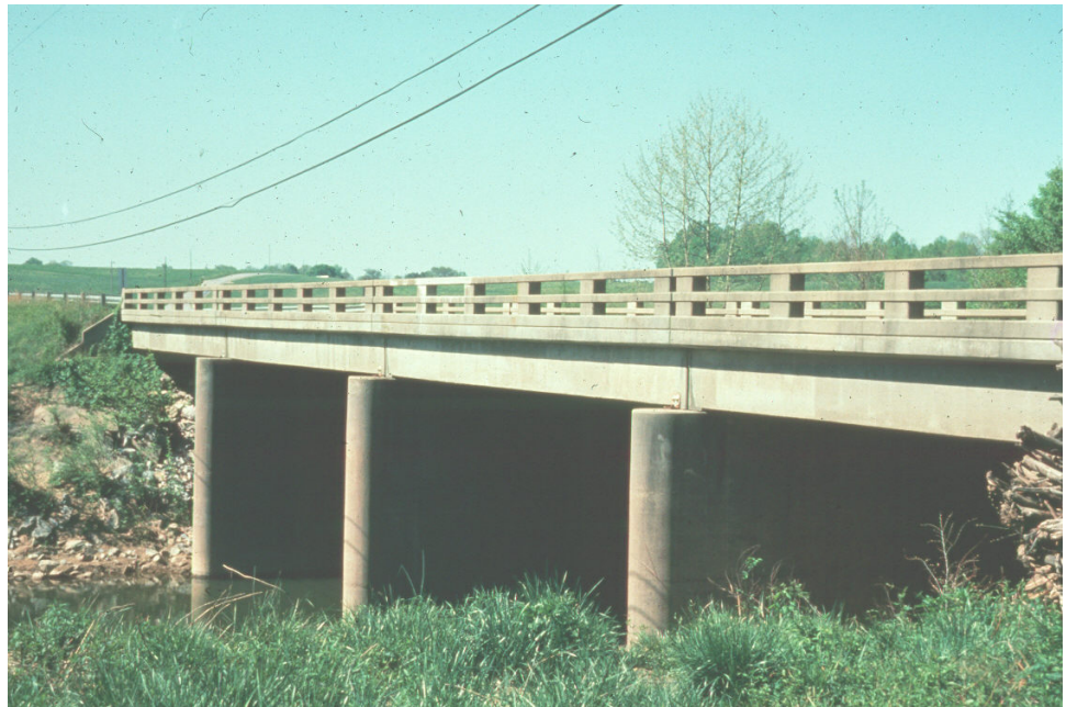
Figure 9.10.1 Typical Box Beam Bridge
