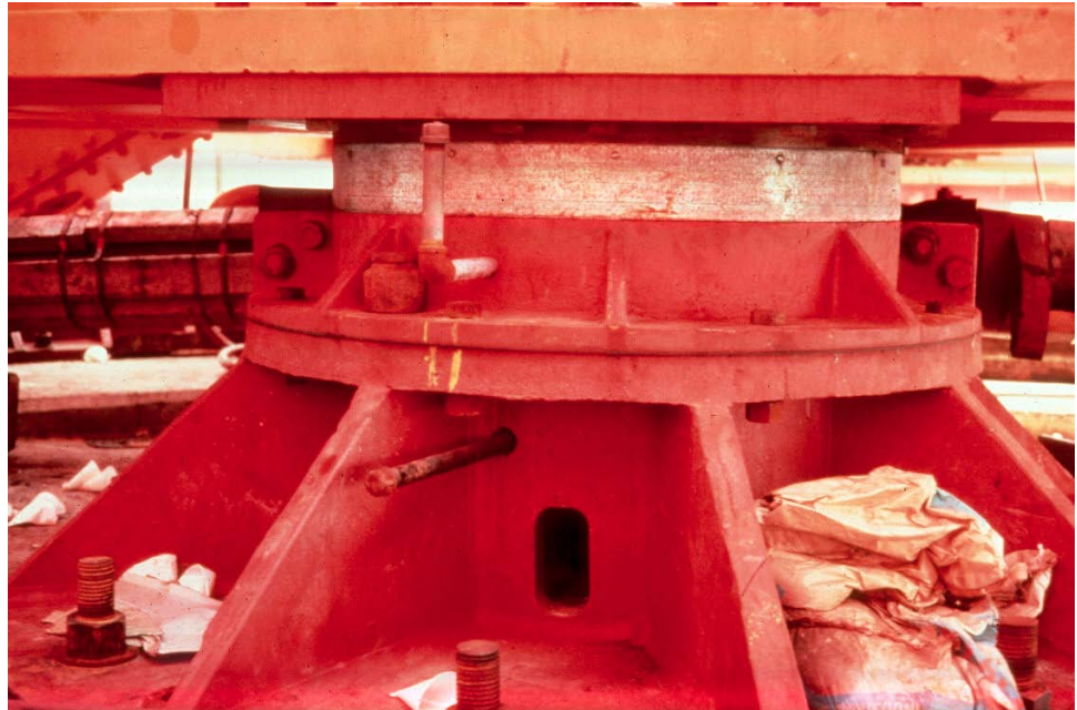
Figure 16.2.36 Center Pivot Bearing
