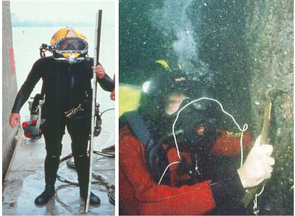
Figure 13.3.46 Diver with a Pry Bar and Diver with Hand Scraper
