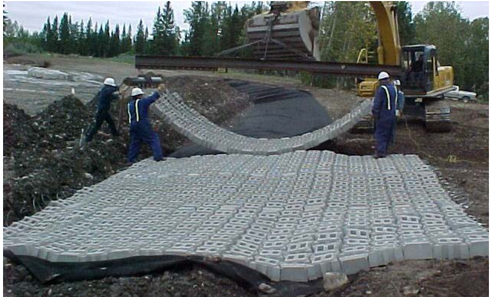
Figure 13.1.14 Concrete Revetment Mat
