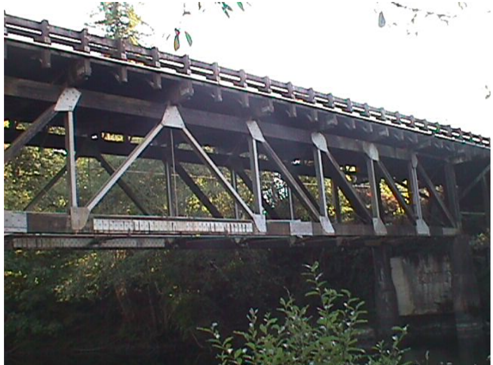
Figure 10.8.6 Steel Gusset Plates Connecting Timber Primary Truss Members
