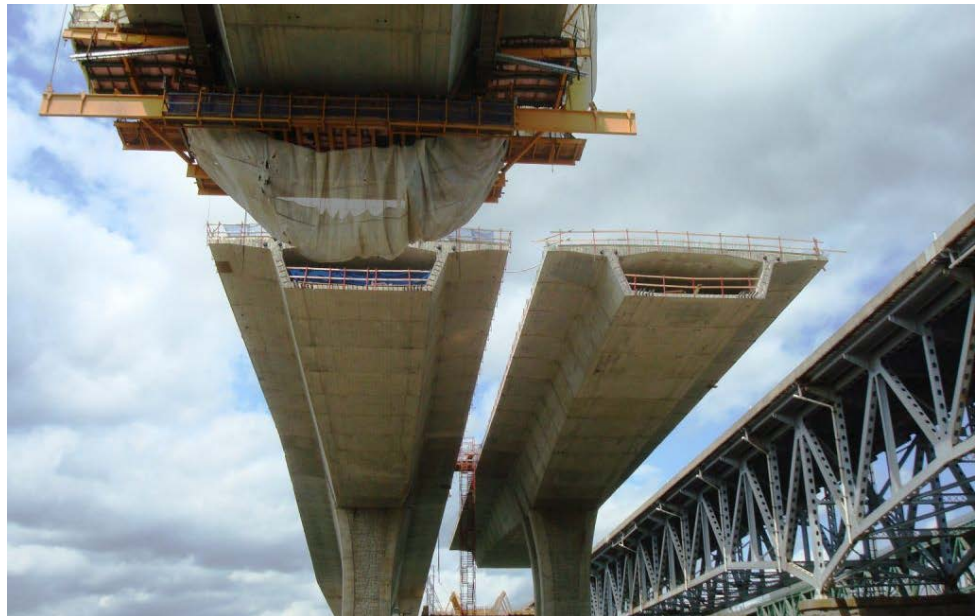
Figure 6.2.10 Post-tensioned Concrete Box Girders
