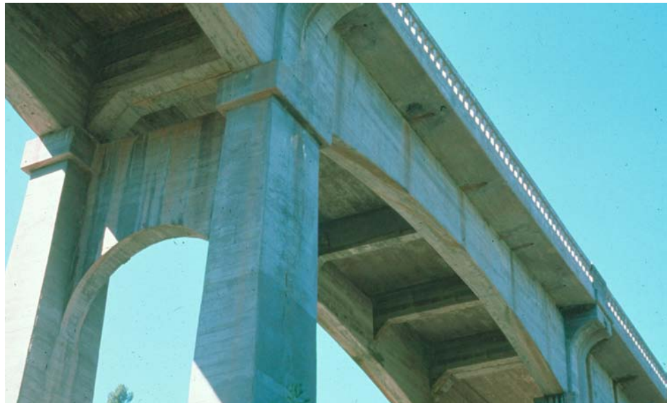
Figure 9.3.3 Concrete Deck Two-Girder, Underside View
