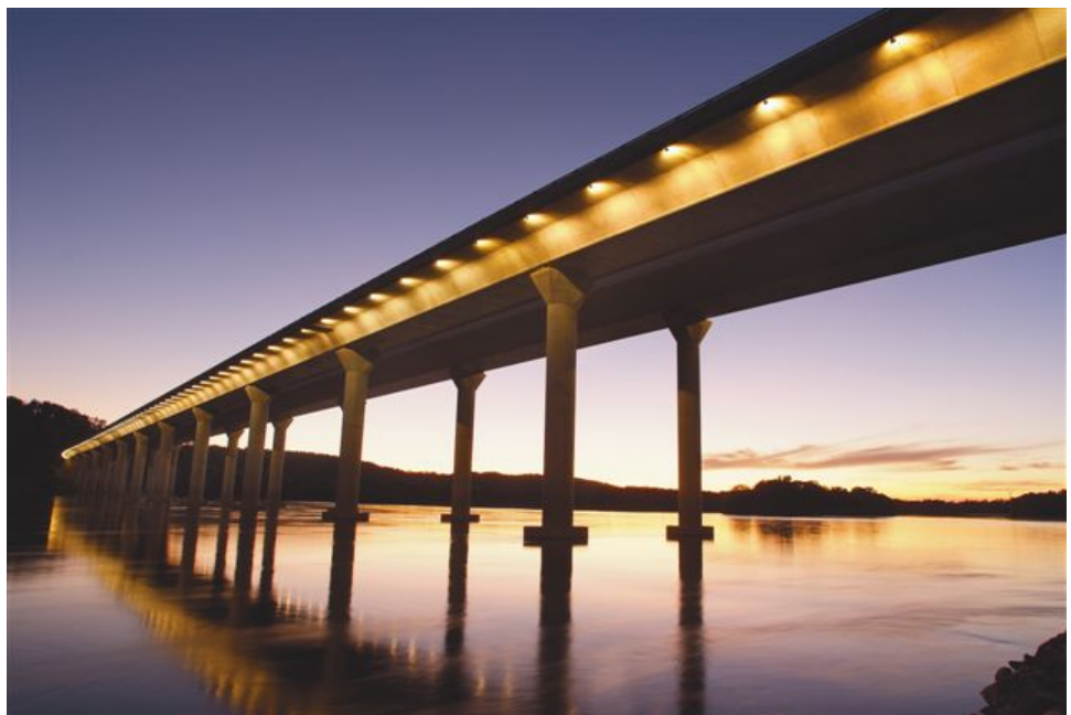
Figure 9.11.1 Segmental Precast Concrete Box Girder Bridge
