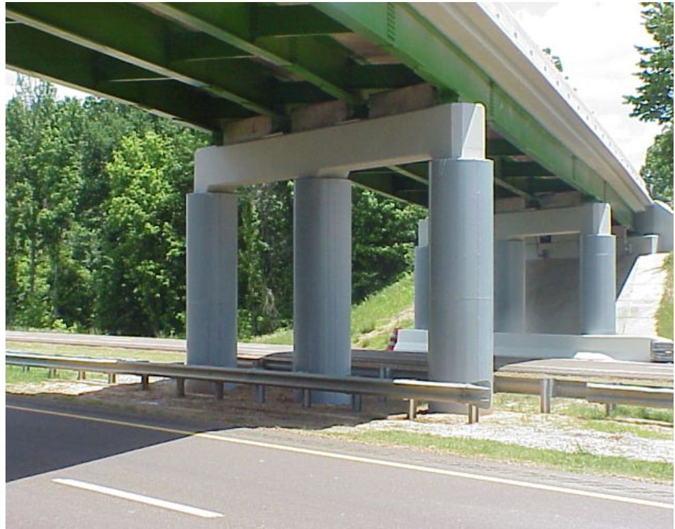
Figure 6.6.2 Seismic Retrofit of Concrete Columns Using FRP Composites
