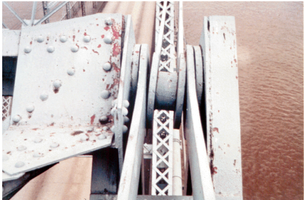
Figure 10.9.24 Asymmetry at an Eyebars Connection
