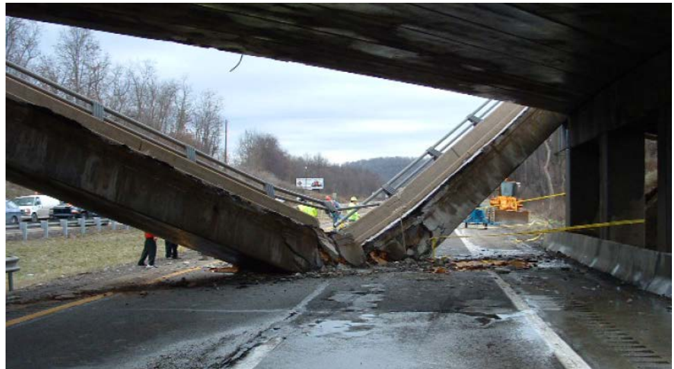
Figure 9.10.20 View Northeast of I-70 EB from Beneath Span 3
