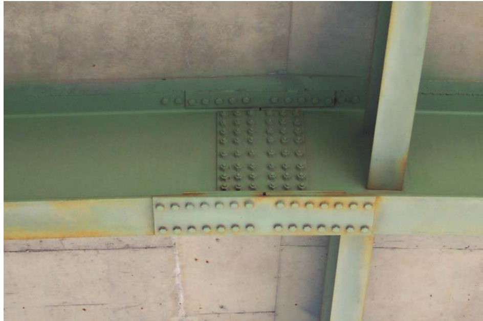
Figure 3.1.27 Bolted Field Splice
