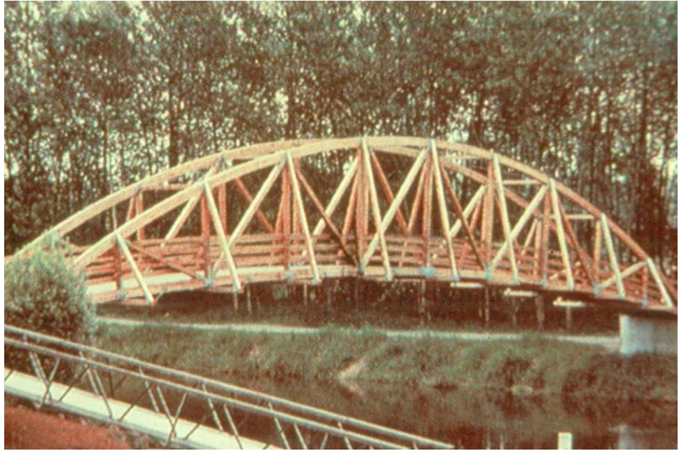
Figure 8.2.4 Bowstring Truss Pedestrian Bridge
