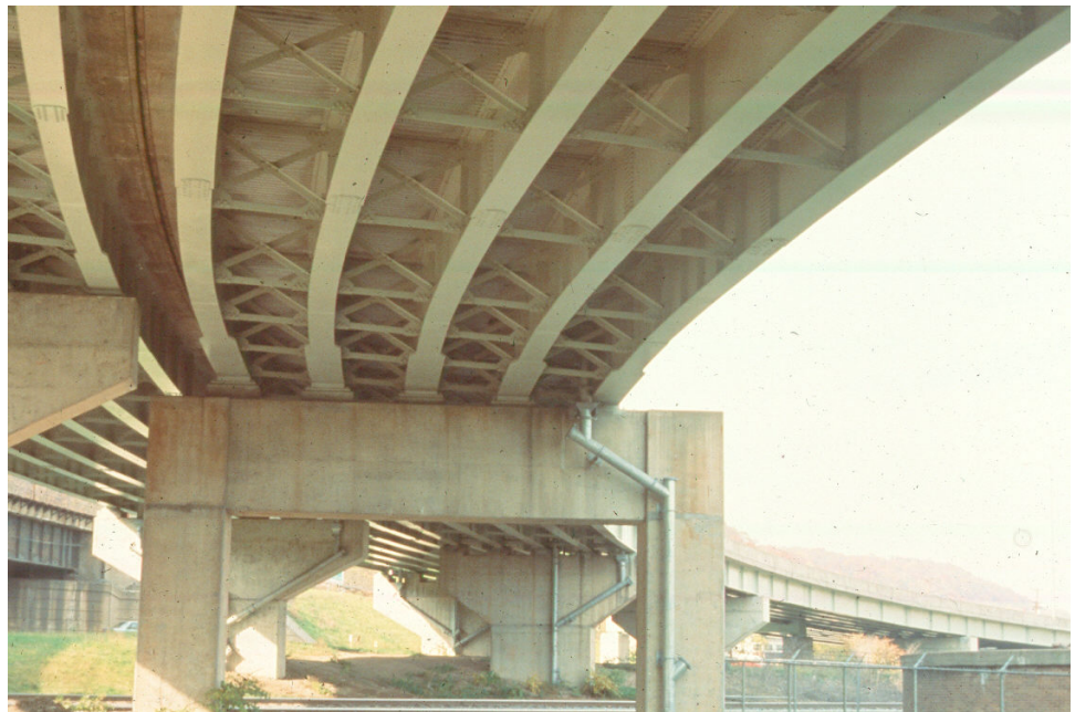
Figure 10.1.8 Curved Fabricated Multi-girder Bridge
