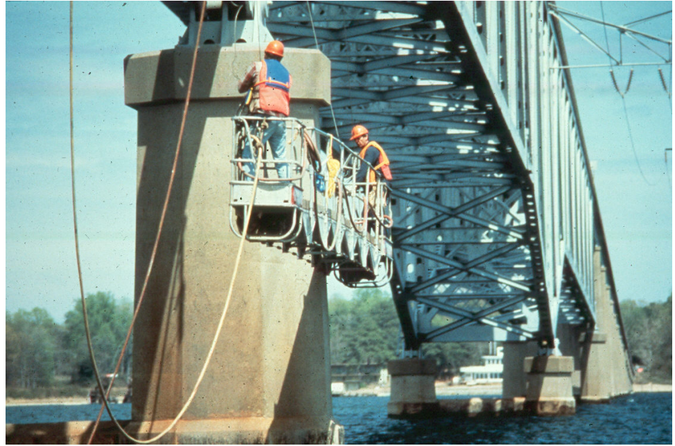
Figure 2.5.3 Rigging for Substructure Inspection
