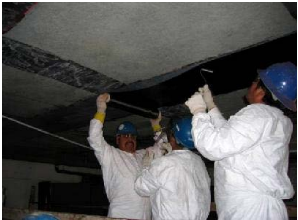
Figure 6.6.1 Concrete Beam Repaired Using FRP
