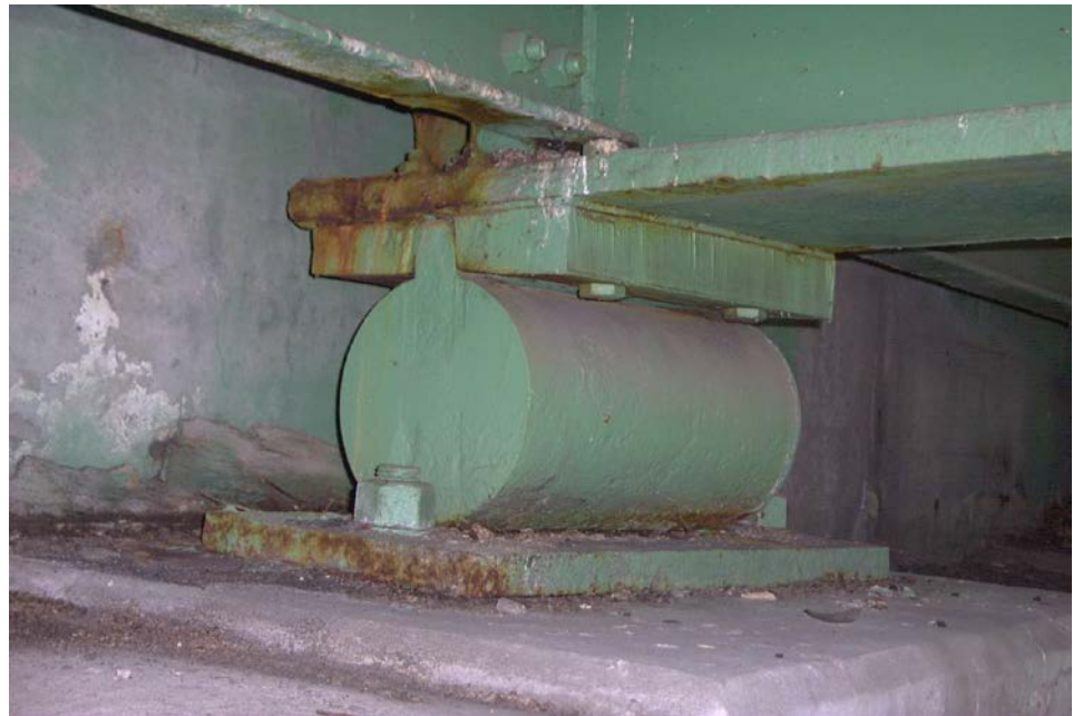
Figure 11.1.7 Single Roller Bearing
