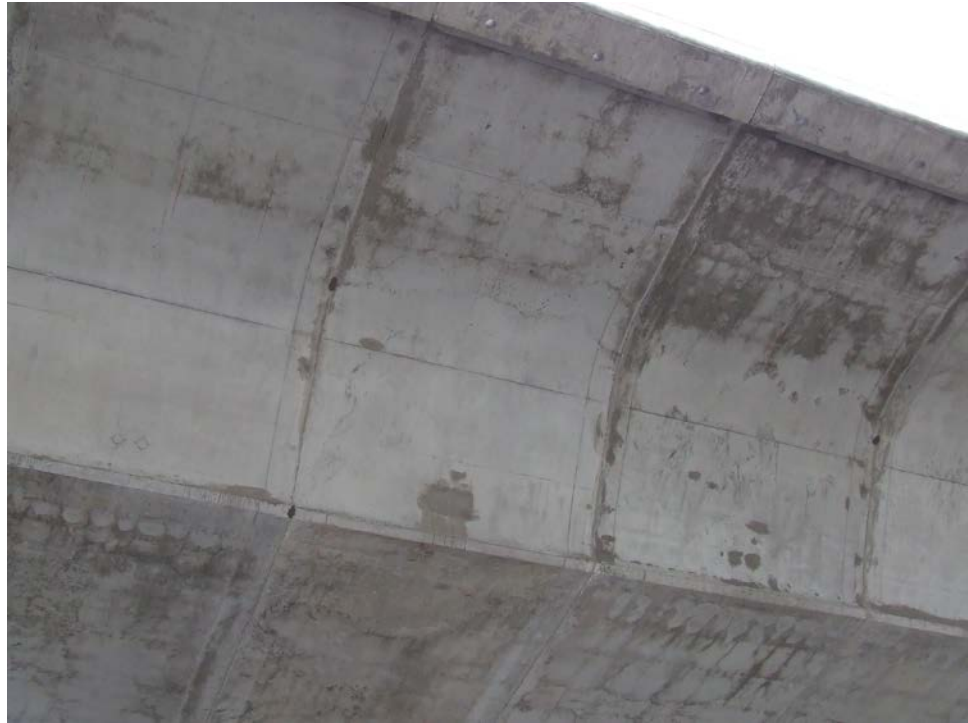
Figure 9.11.15 Close-up of Box Girder Segments
