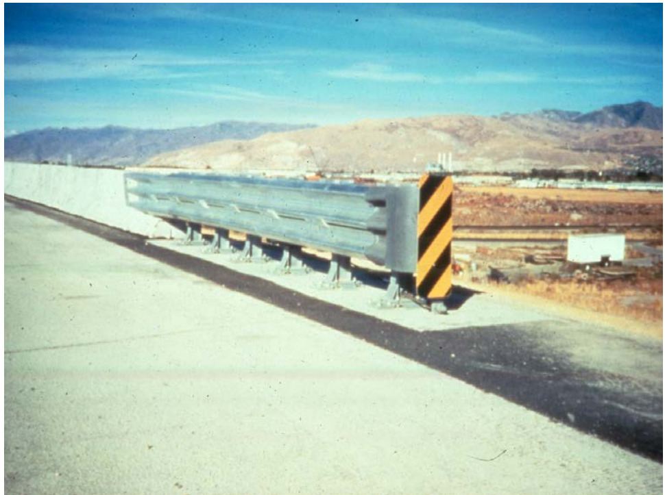
Figure 7.6.1 Bridge Safety Feature
