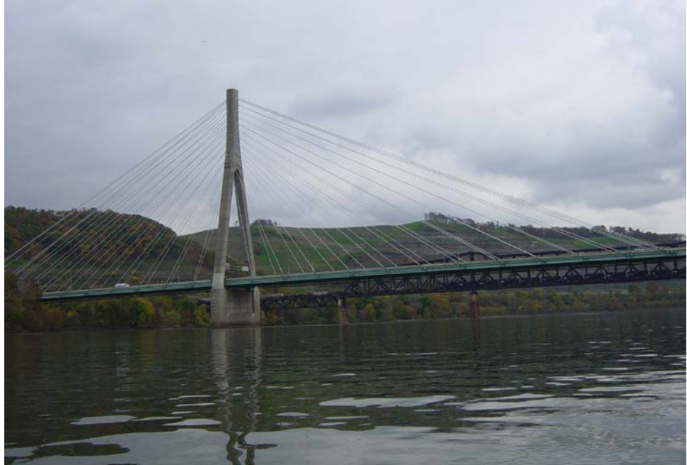
Figure 16.1.41 Cable-Stayed Bridge Cables
