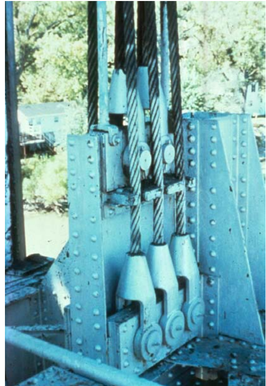
Figure 16.2.51 Wire Rope Sockets and Fittings
