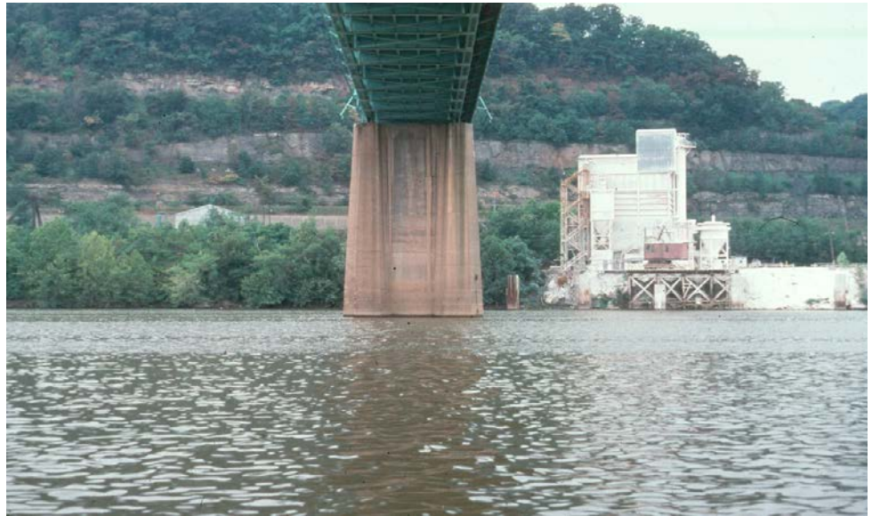
Figure 13.3.17 Column Pier with Solid Web Wall
