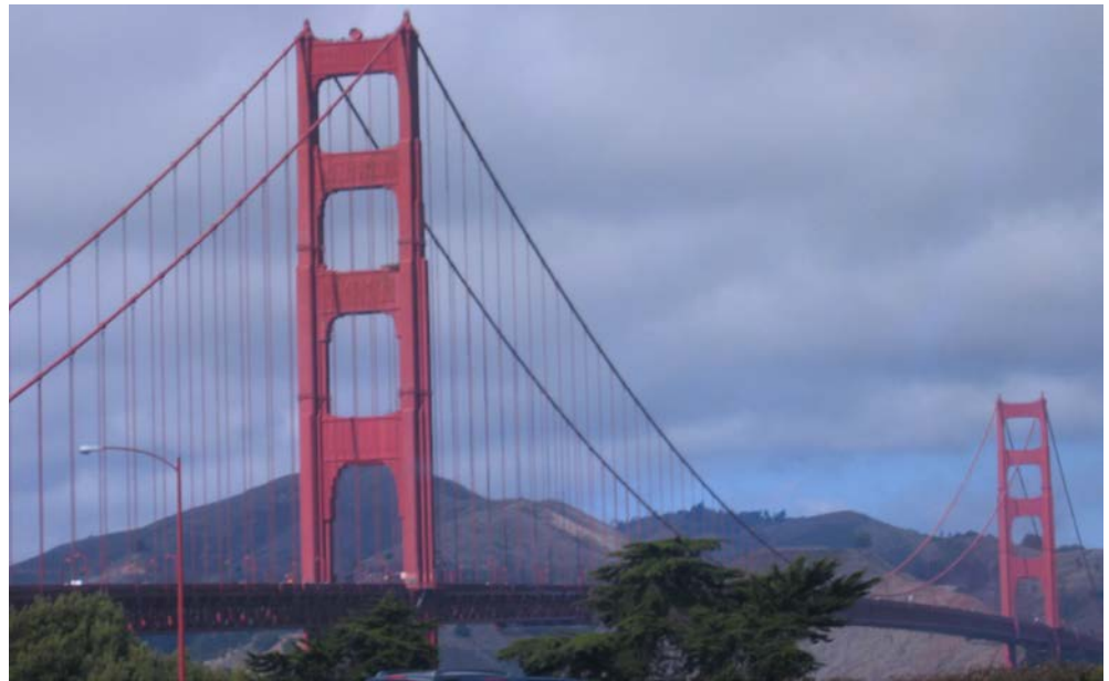
Figure 3.1.19 Cable-Supported Bridge: Suspension Cables and Hangers
