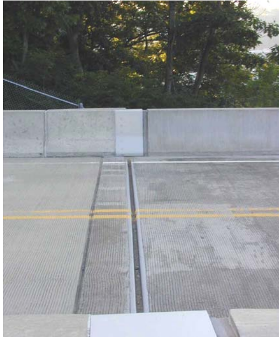
Photo No. 17 Strip Seal at North Abutment (typ.) – note minor debris accumulation
