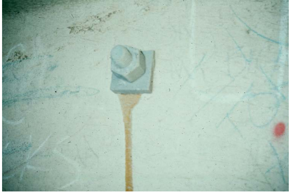
Figure 9.4.8 Close-up of Stem Tie-Bolt (Epoxy Resin)
