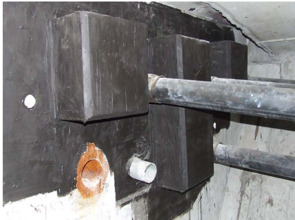
Figure 9.11.48 Box Girder Interior Diaphragm and Post-Tensioning Ducts
