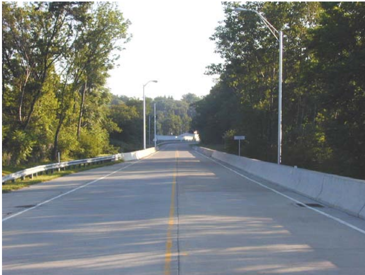
Photo No.2 South Approach (near)
