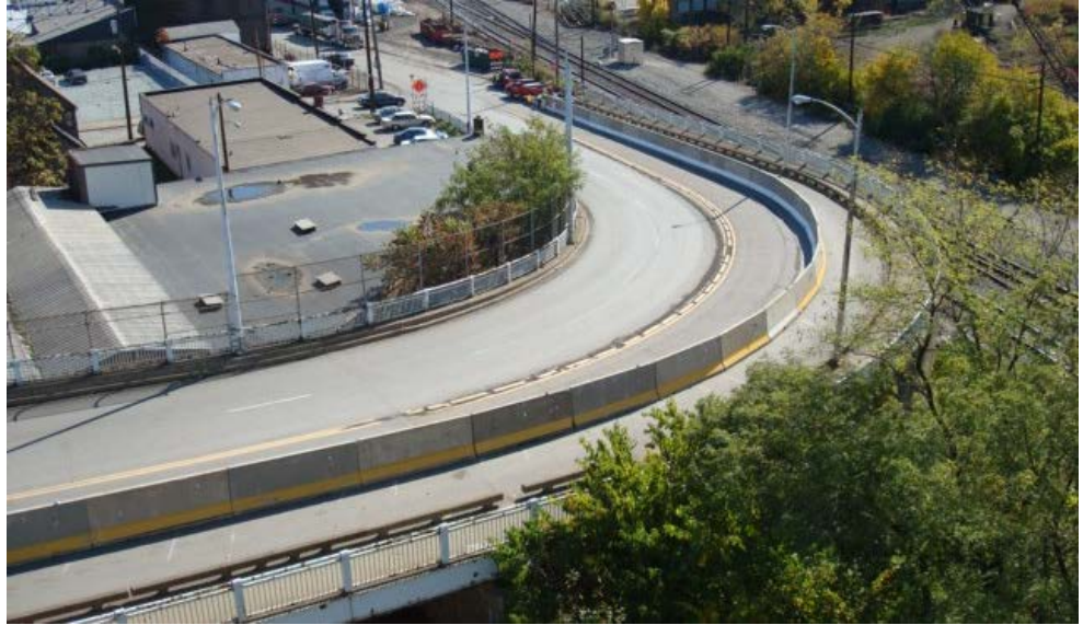
Figure 2.3.13 Temporary Traffic Barriers
