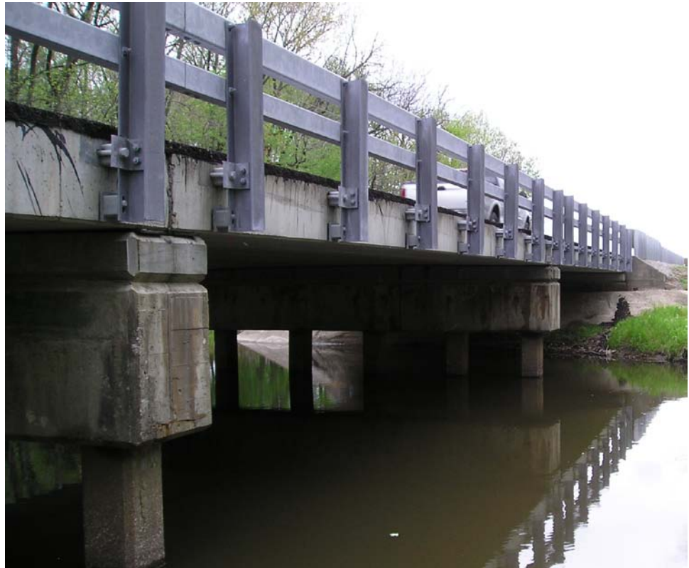
Figure 9.7.1 Typical Prestressed Slab Beam Bridge
