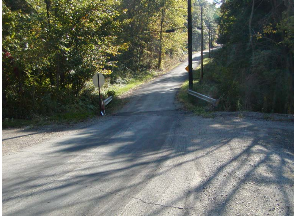
Figure 4.6.1 Near Approach - Toward Bridge
