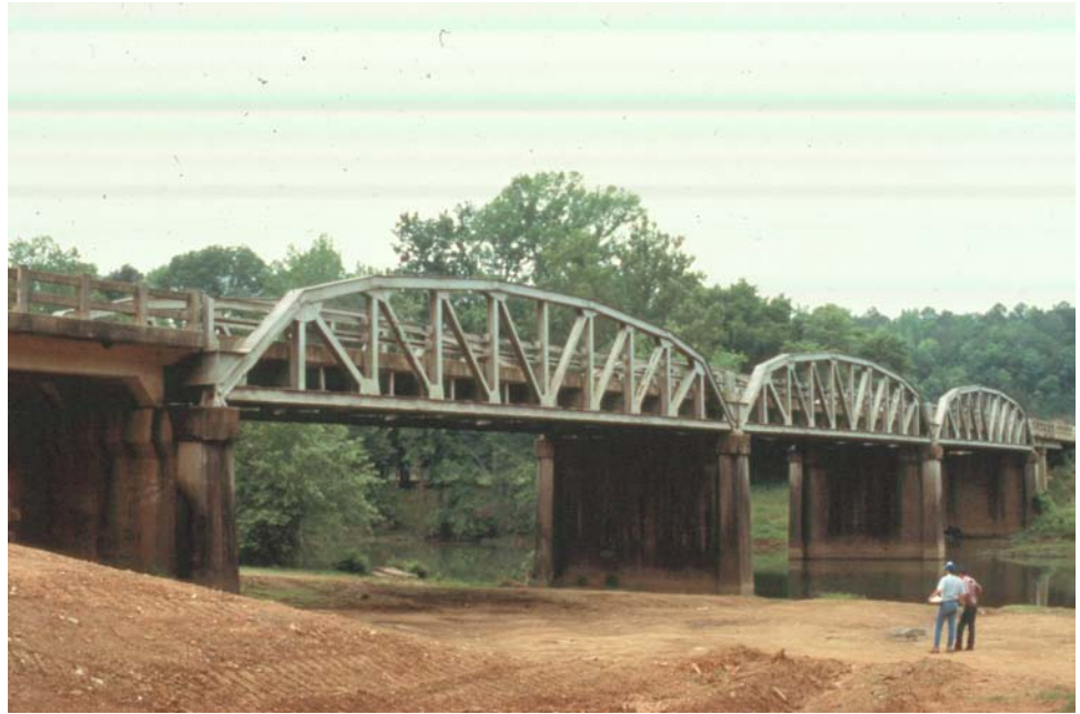
Figure 10.4.12 Multiple Span Pony Truss
