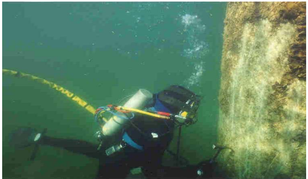
Figure 13.3.4 Diver Cleaning Pier Face For Inspection
