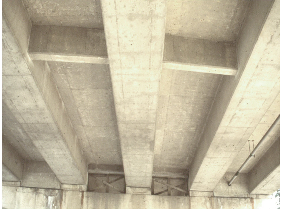
Figure 9.10.8 End and Intermediate Diaphragms on a Spread Box Beam Bridge
