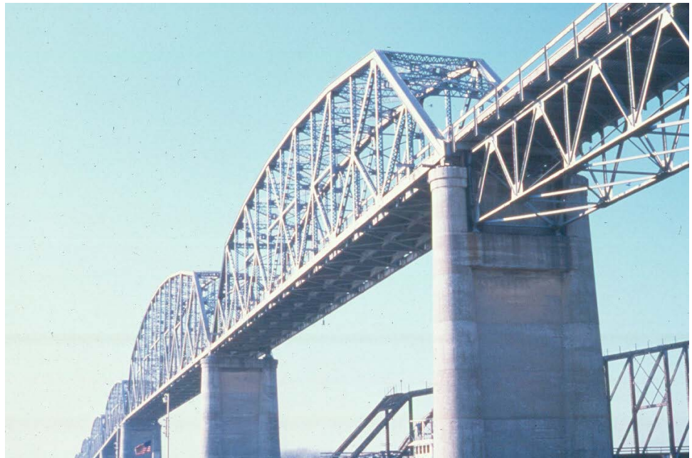
Figure 12.2.5 Column Pier with Web Wall
