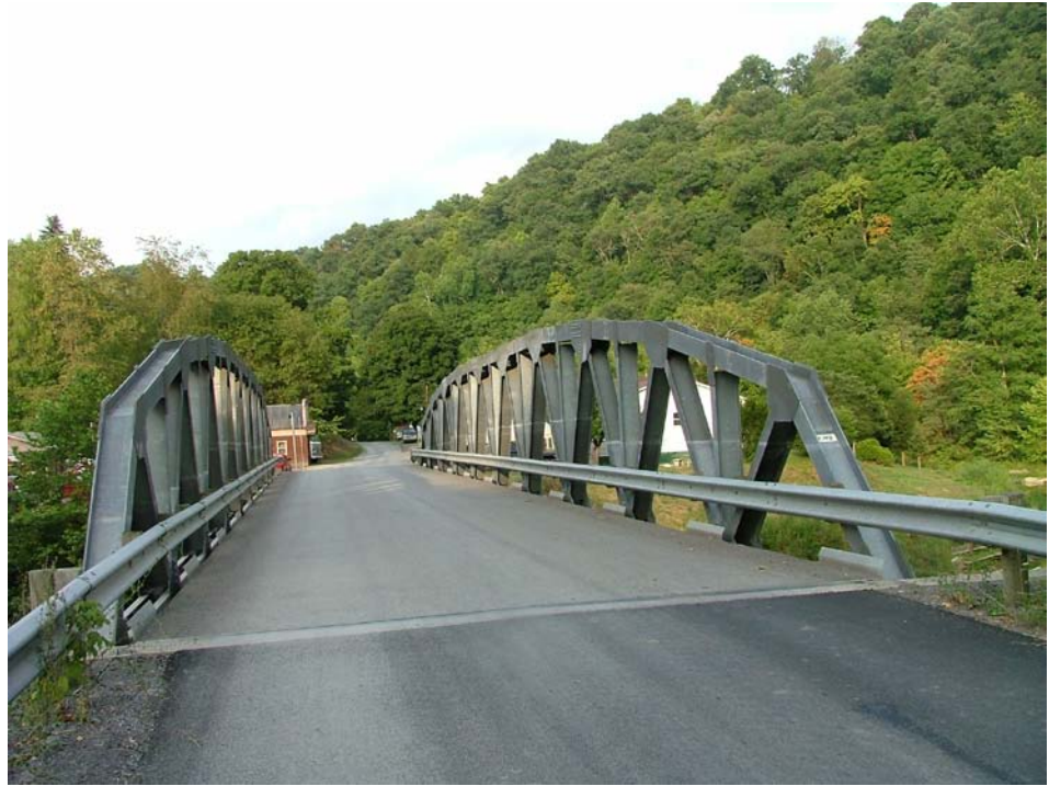
Figure 10.4.10 Single (Simple) Span Camel Back Pratt Truss
