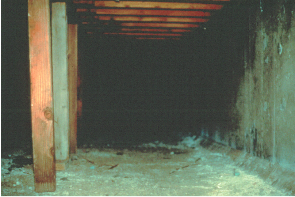
Figure 9.11.42 Interior Formwork Left in Place
