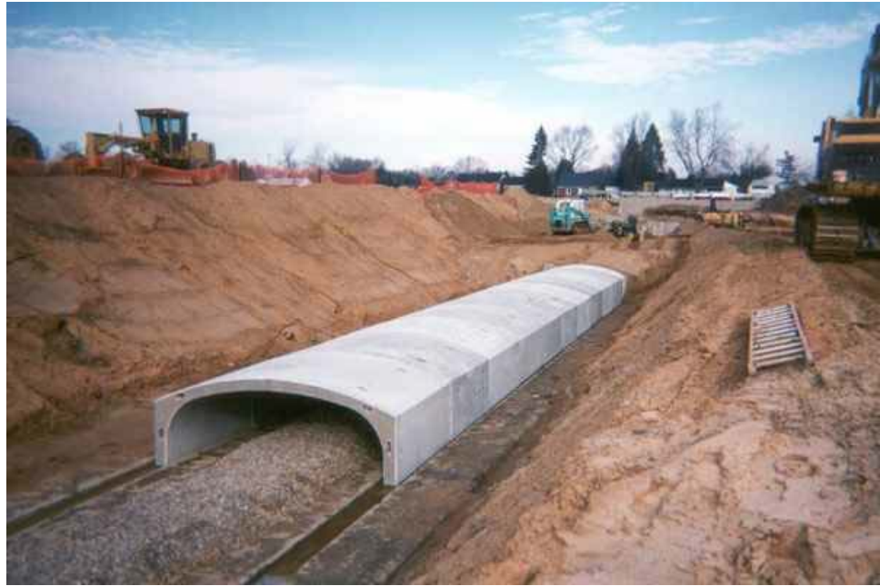
Figure 9.5.4 Precast Concrete Arch with Integral Vertical Legs
