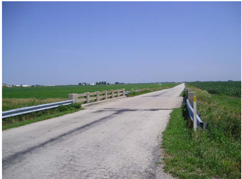
Figure 14.1.29 Approach Roadway at a Culvert Site
