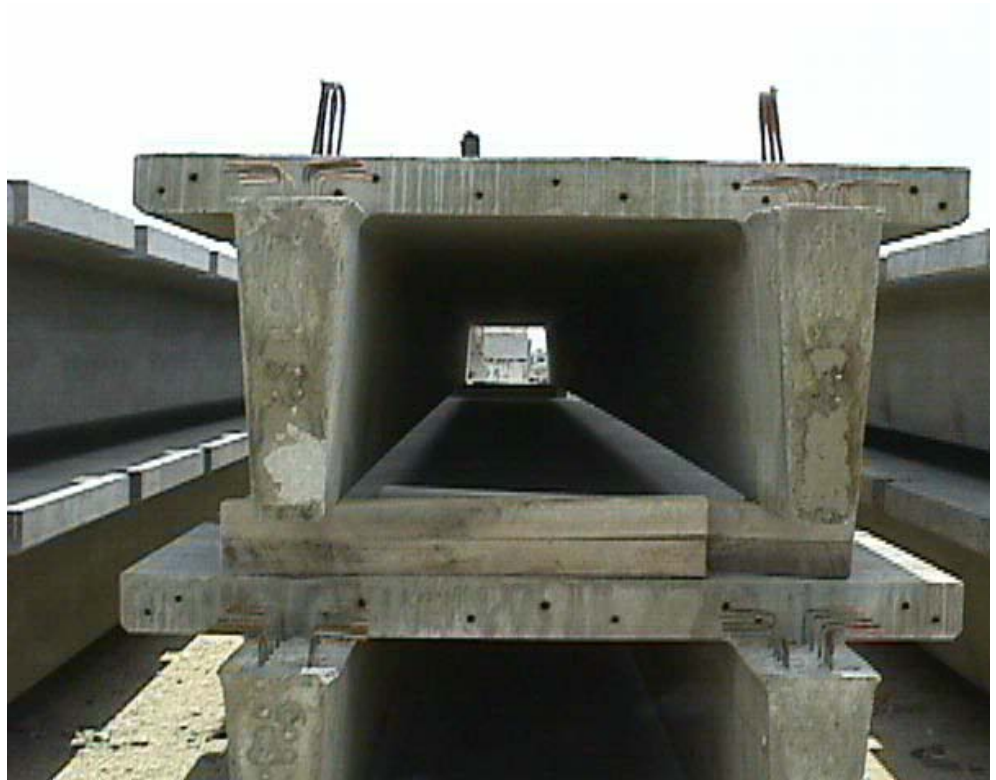
Figure 9.8.1 Typical Prestressed Double Tee Beam
