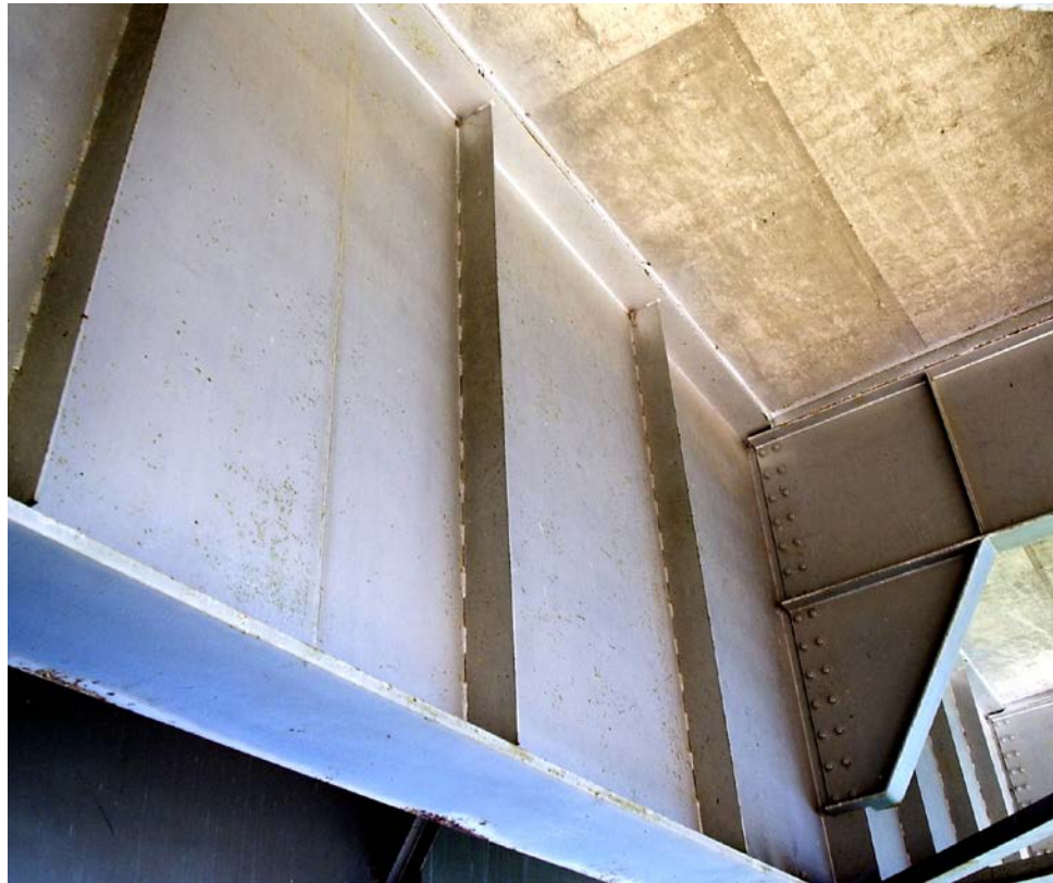
Figure 6.4.54 Intermittent or Stitch Welded Transverse Stiffeners
