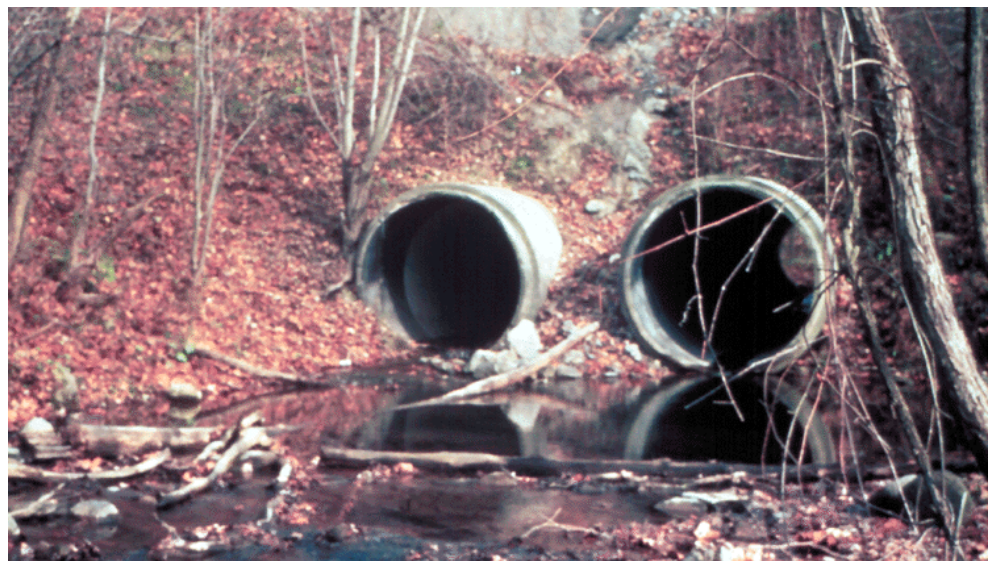
Figure 14.2.6 Twin Concrete Pipe Culvert
