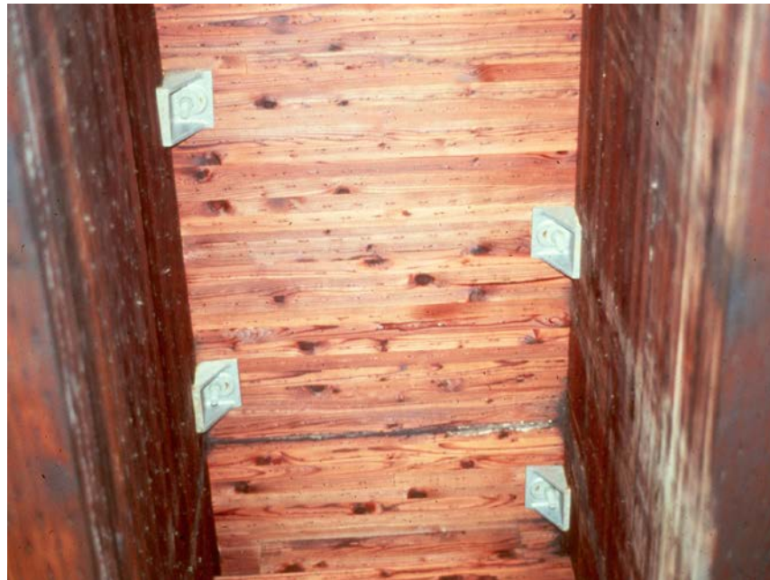
Figure 7.1.3 Glued-laminated Deck Panels Attached to Superstructure
