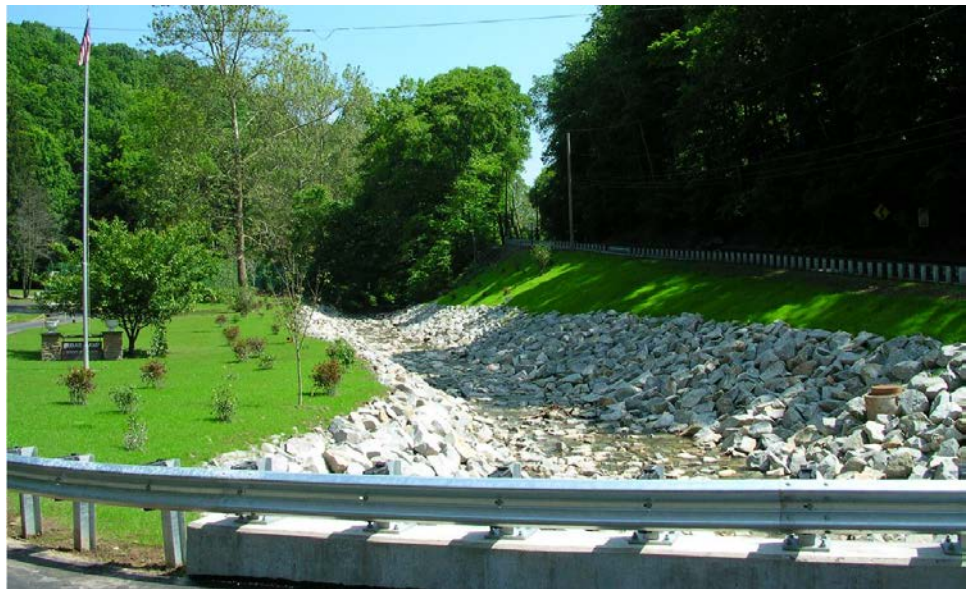
Figure 13.1.9 Crushed Stone Riprap
