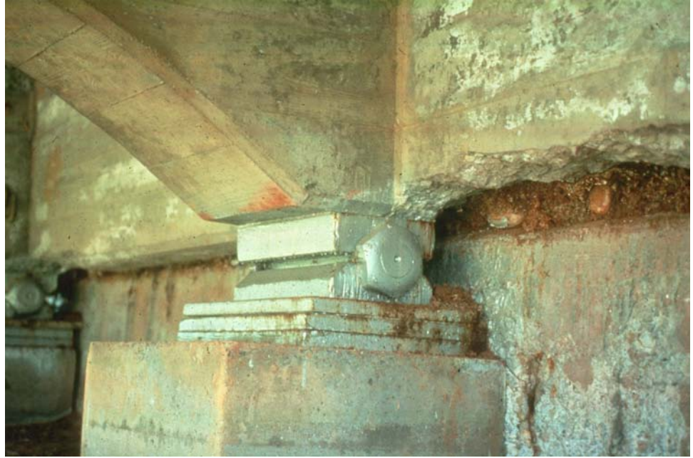
Figure 9.2.11 Steel Bearing Supporting a Cast-in-Place Concrete Tee Beam
