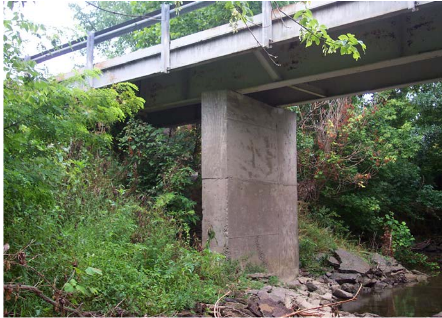
Figure 3.1.75 Solid Shaft Pier
