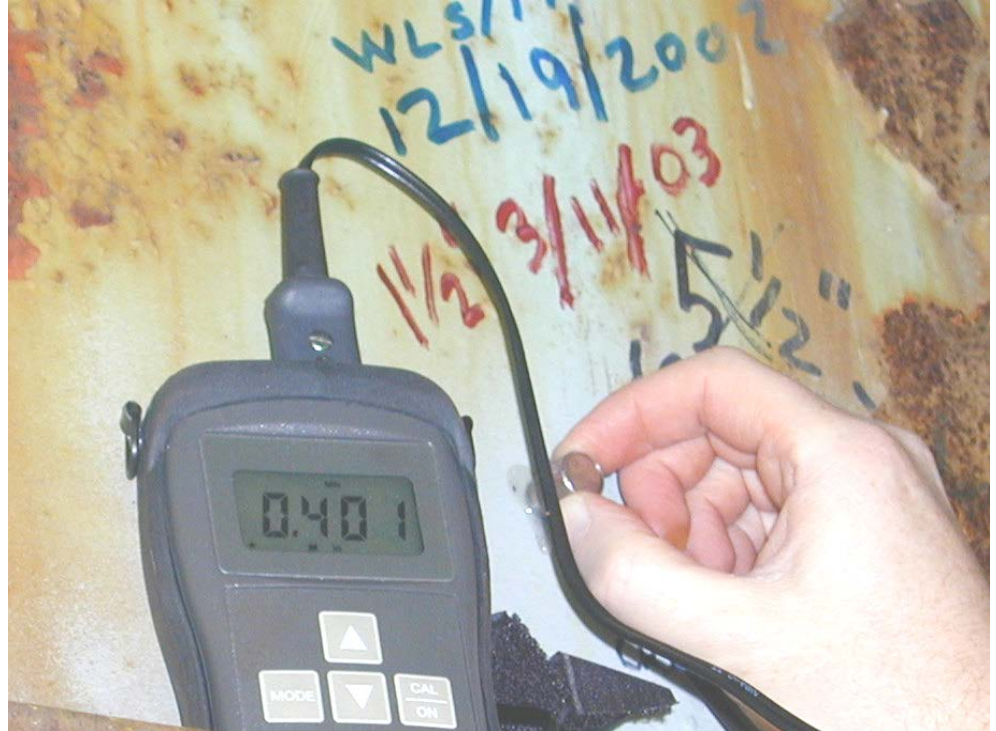
Figure 10.8.19 Inspector Using a D-meter to Measure the Thickness of the Gusset Plate
