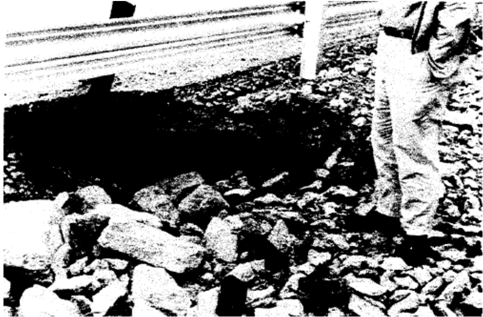
Figure 14.3.10 (Exhibit 68) Surface Hole Above Open Joint
