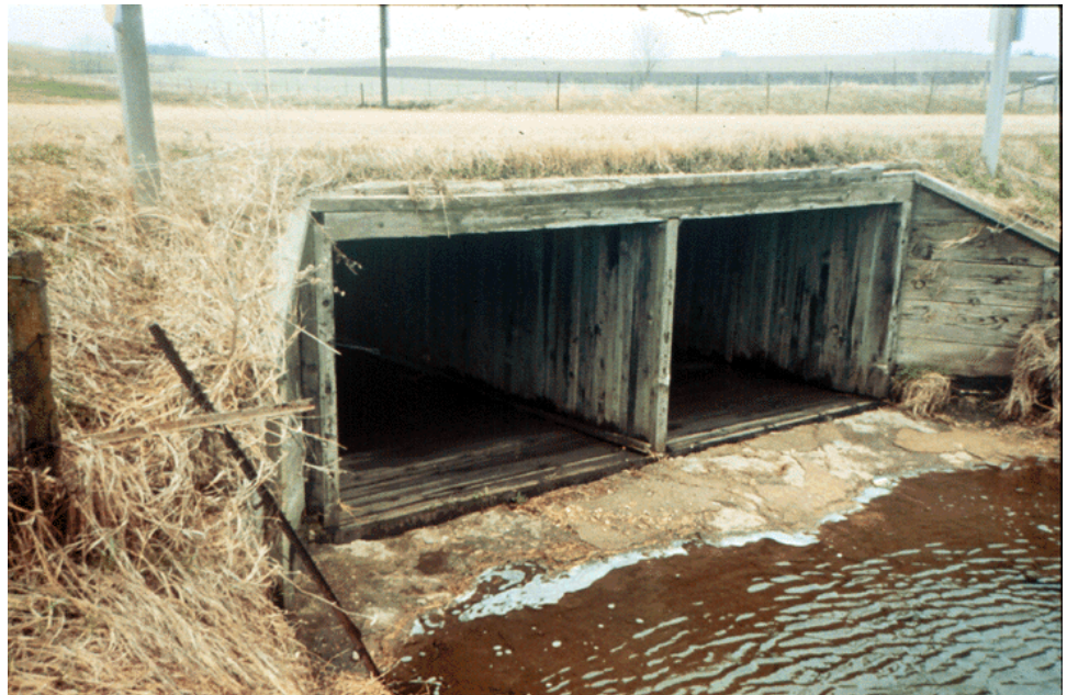
Figure 14.1.16 Timber Box Culvert
