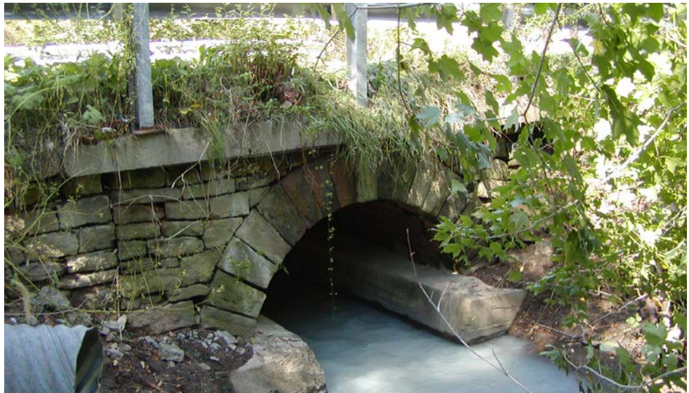
Figure 14.2.9 Stone Masonry Arch Culvert
