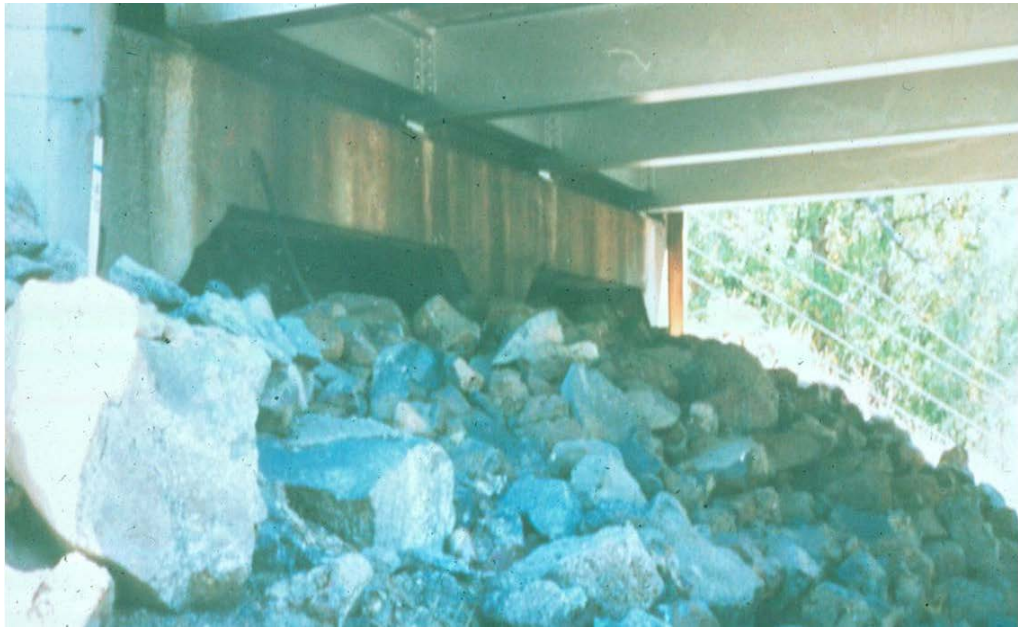
Figure 3.1.73 Spill-Through or Open Abutment
