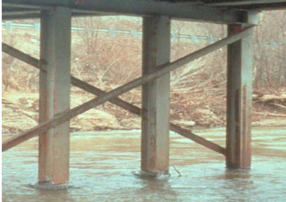
Figure 13.3.15 Steel Pile Bent
