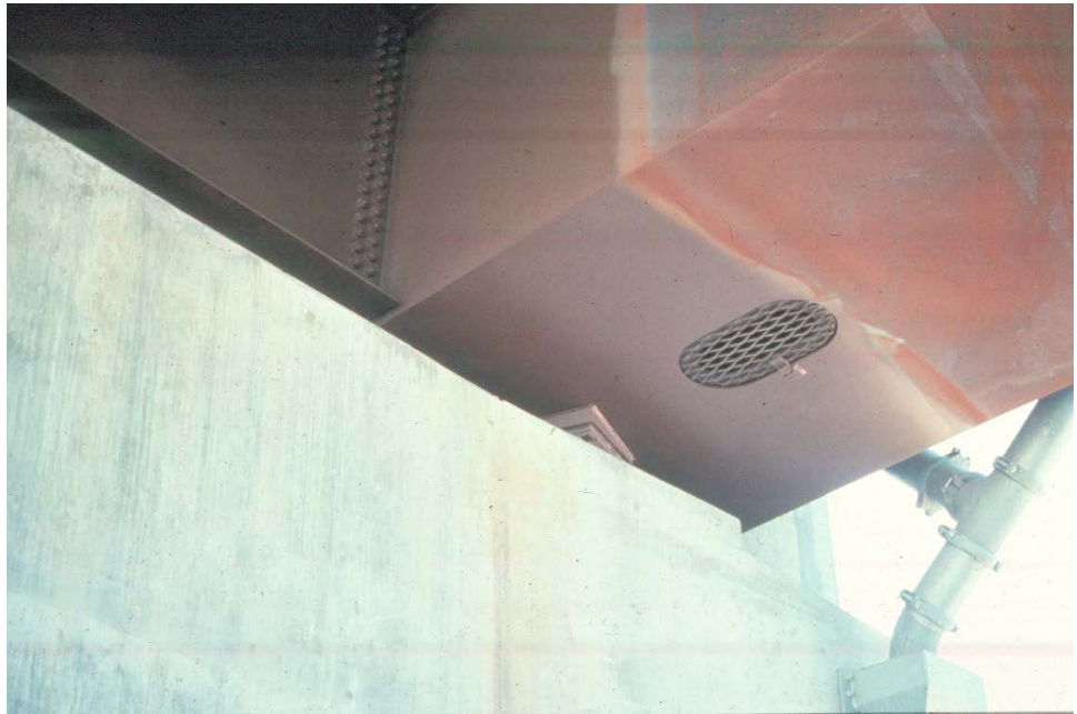
Figure 10.3.10 Box Girder Shear Zone
