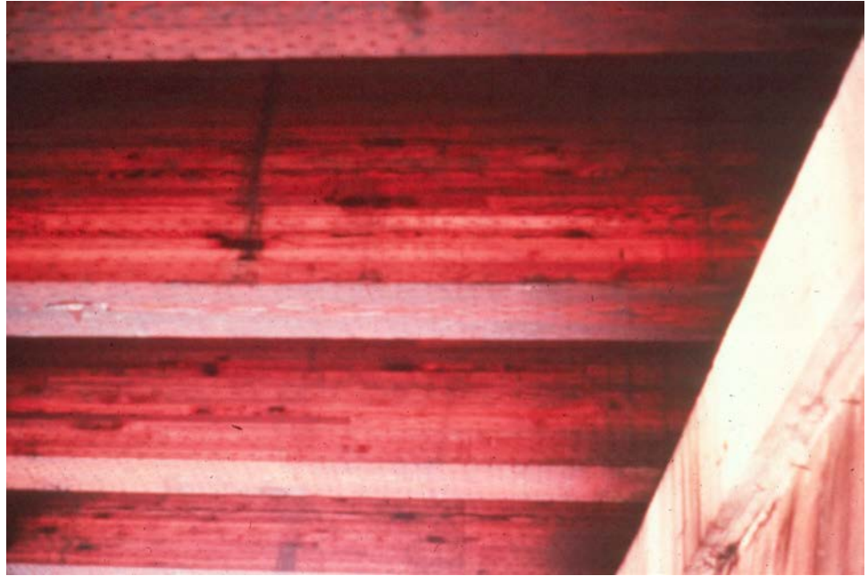
Figure 8.2.10 Close-up View of Glulam Bridge Showing Laminations
