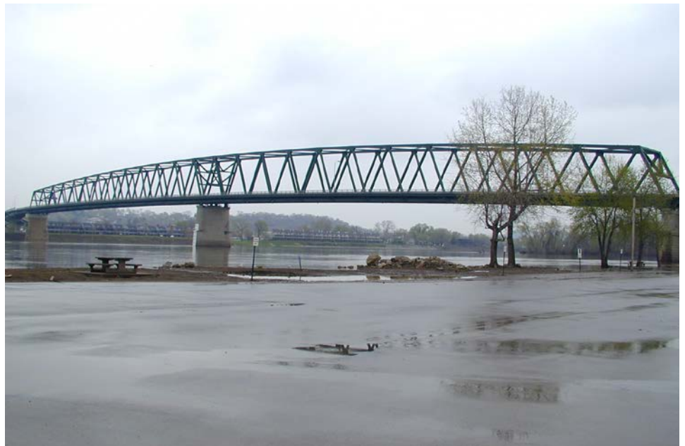
Figure 3.1.53 Through Truss Bridge
