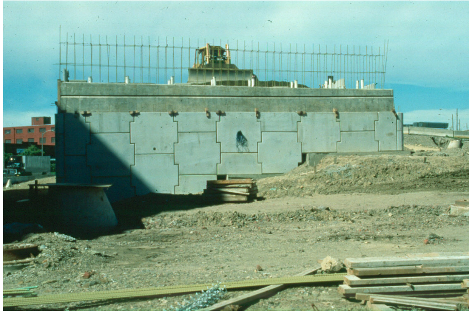
Figure 12.1.9 Mechanically Stabilized Earth Abutment (Note Precast Concrete Panels)
