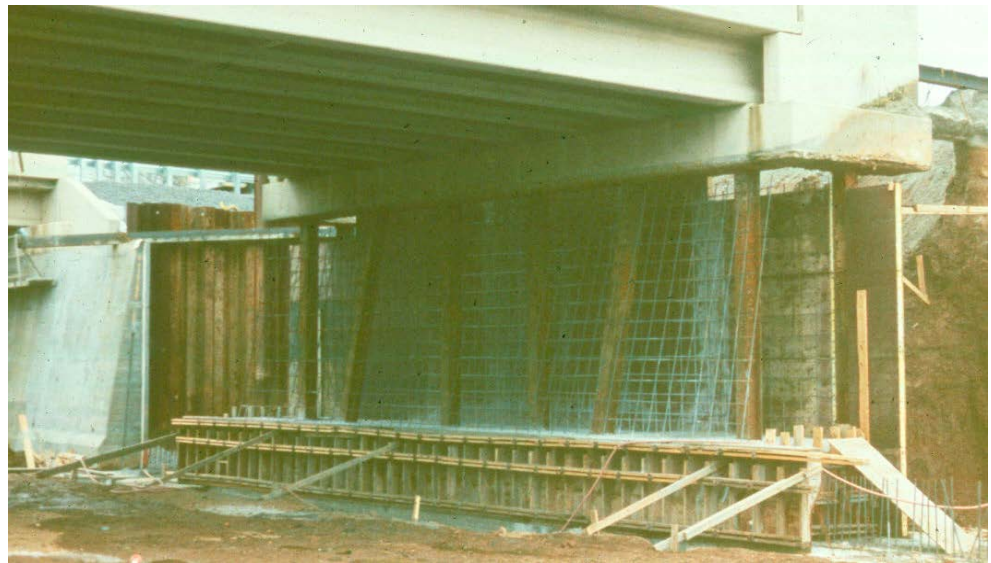
Figure 12.1.22 Stub Abutment on Piles with Piles Exposed
