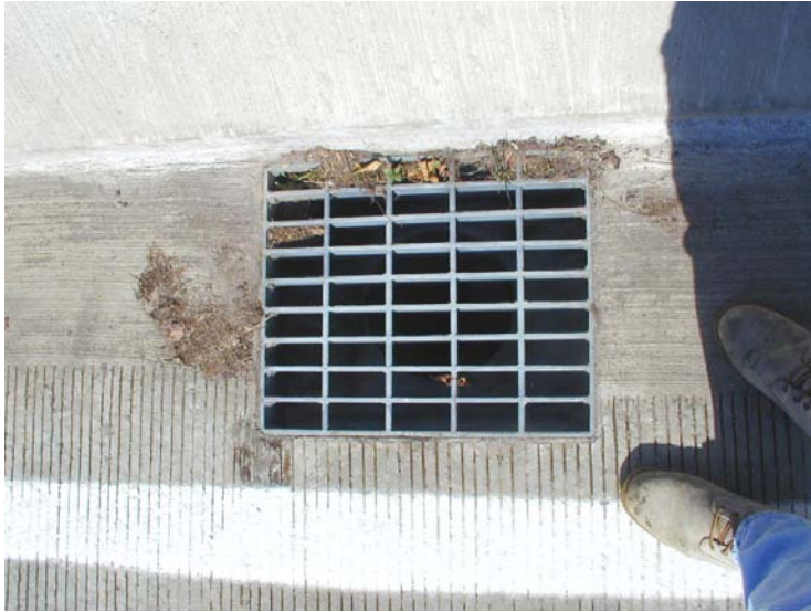
Photo No. 15 Typical PennDOT Type 1 Scupper
