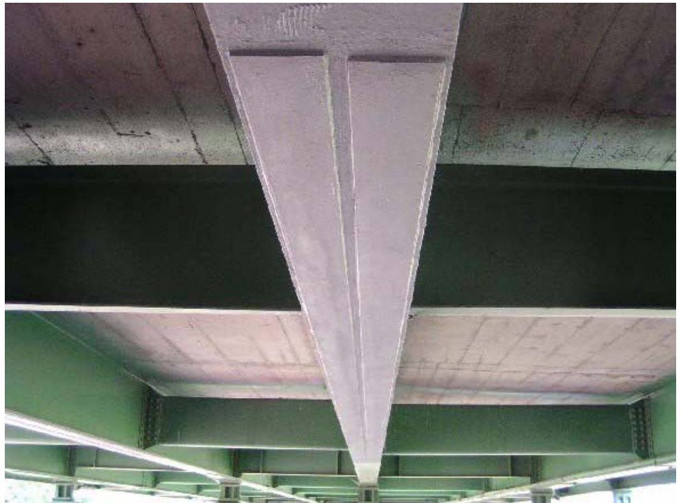
Figure 6.6.4 Externally Bonded CFRP Plates to Steel Girder Bottom Flange
