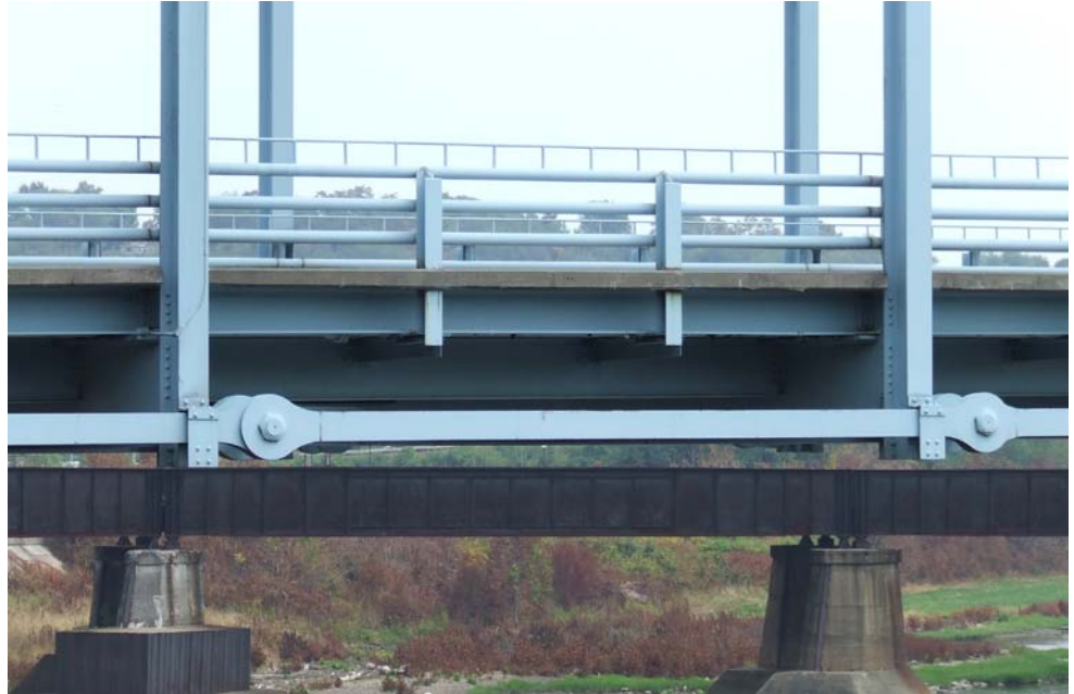
Figure 10.9.1 Typical Eyebare Tension Member on an Arch
