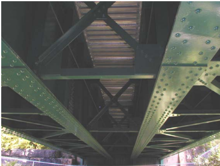
Photo No. 10 General Underside View – Span 3
