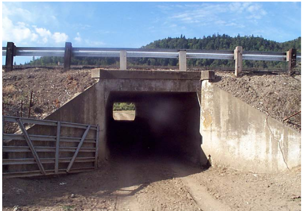
Figure 14.1.2 Box Culvert with Shallow Cover
