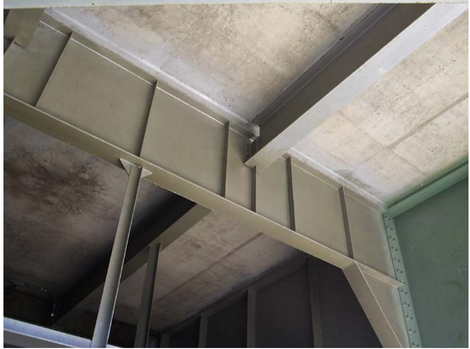
Figure 3.1.29 Underside View of a Bridge Deck
