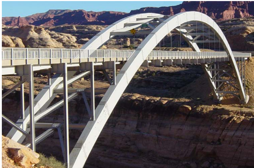
Figure 10.5.2 Through Arch Bridge
