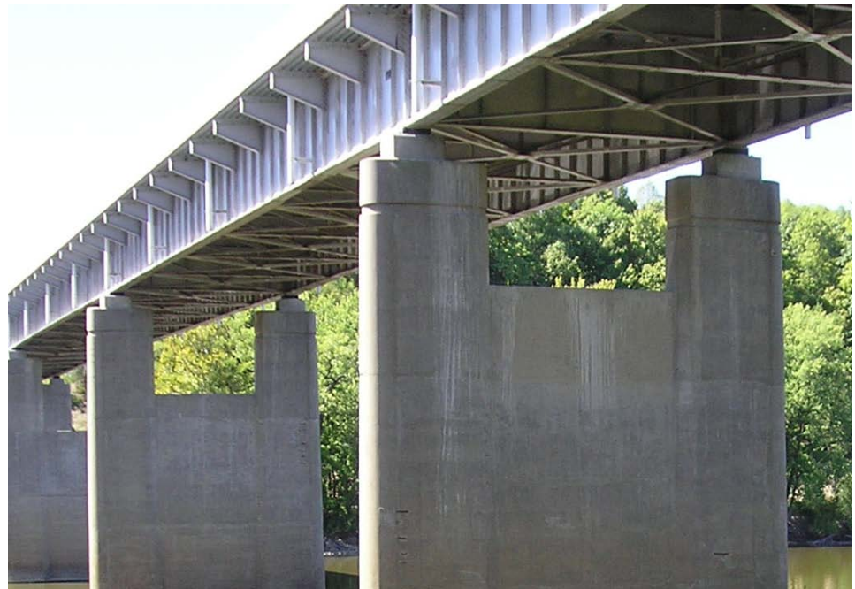
Figure 10.2.1 General View of a Deck Girder Bridge
