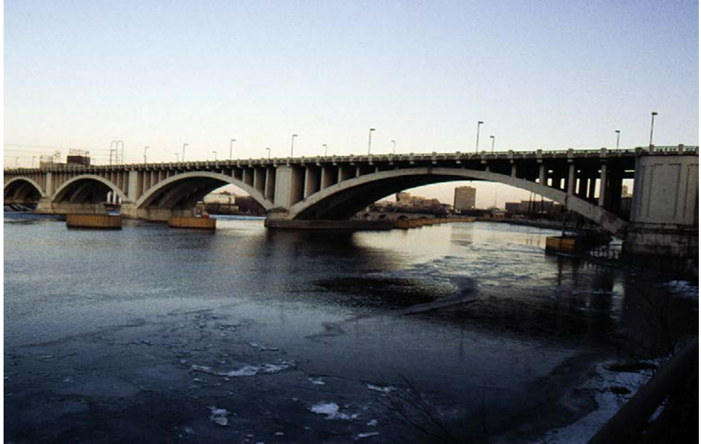
Figure 3.1.54 Deck Arch Bridge
