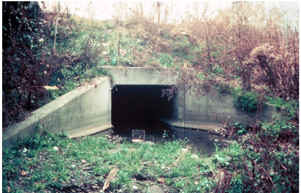
Figure 14.1.35 Culvert Headwall and Wingwall End Treatment
