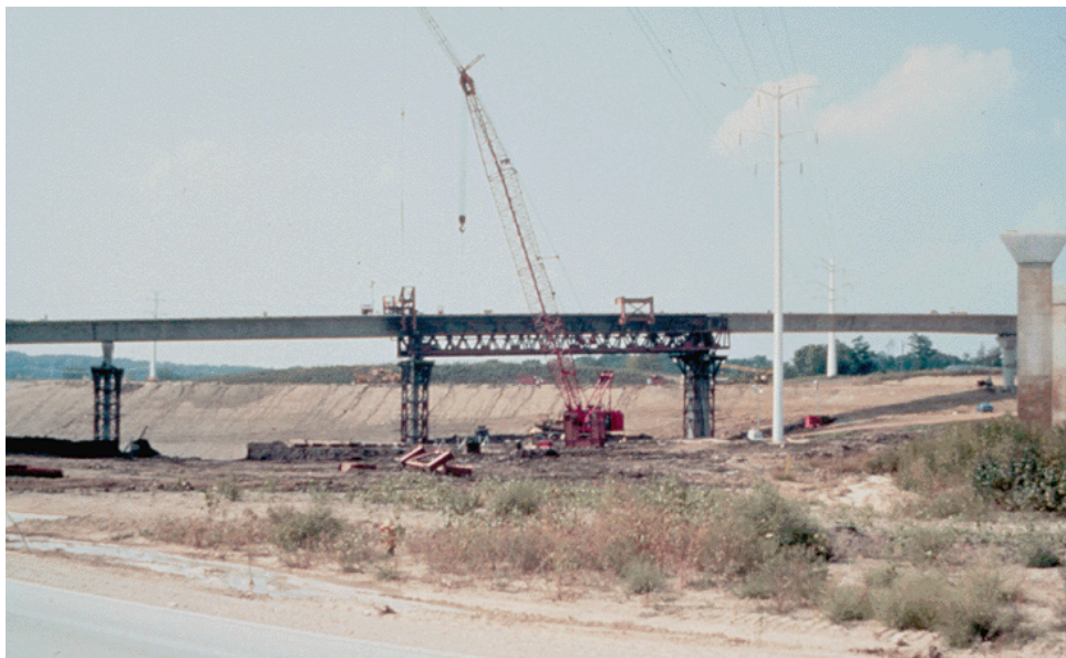
Figure 9.11.23 Span-by-span Construction (with Erection Truss)
