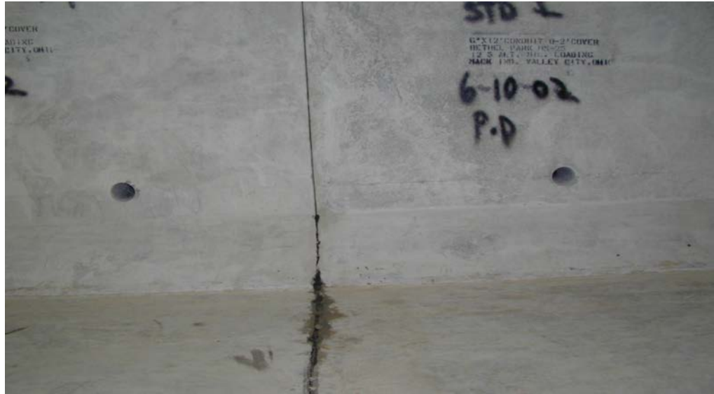
Figure 14.2.19 Precast Concrete Box Culvert Joint
