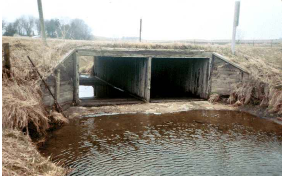
Figure 14.2.10 Timber Box Culvert
