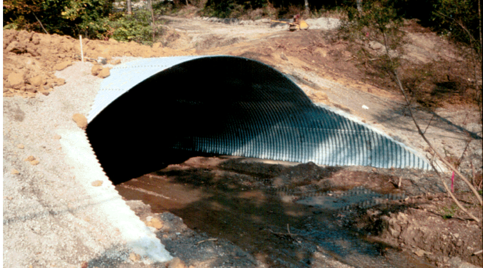
Figure 14.1.8 Pipe Arch Culvert
