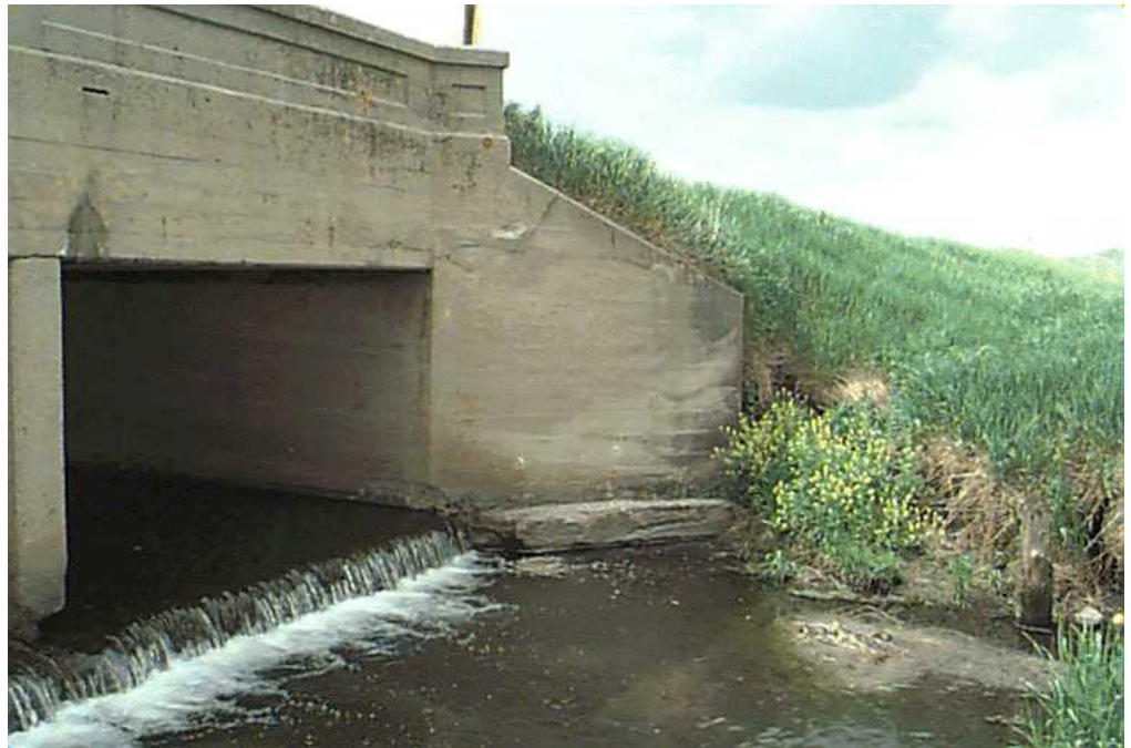
Figure 14.2.23 Cast-in-Place Concrete Headwall and Wingwall
