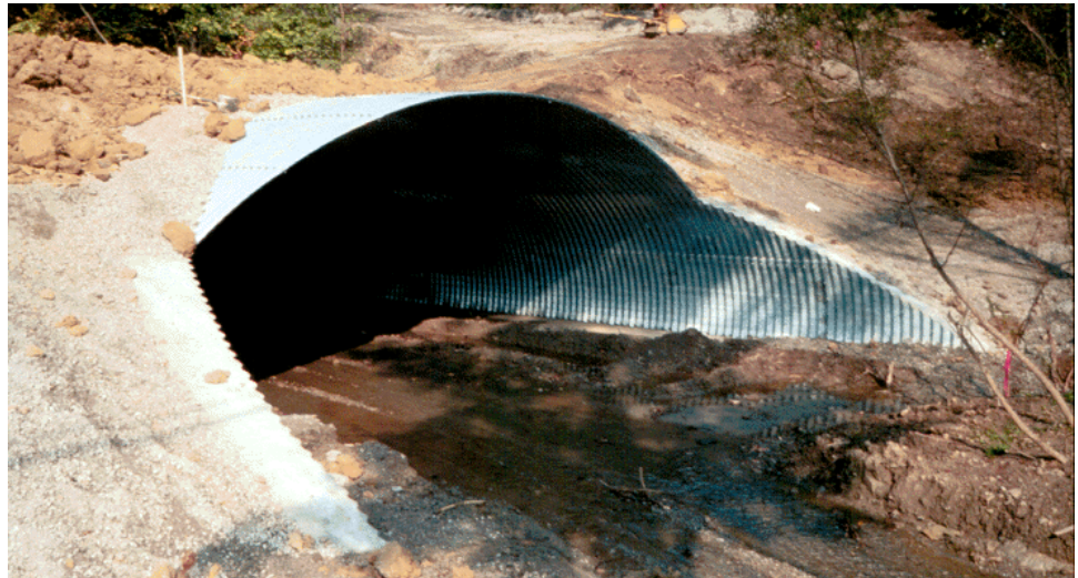
Figure 14.3.1 Pipe Arch Flexible Culvert
