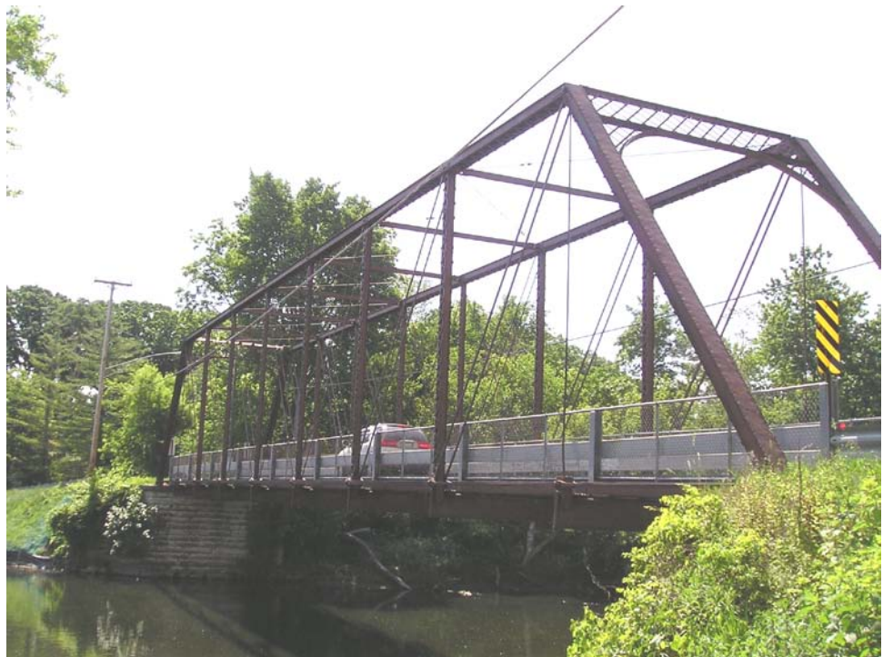
Figure 10.4.11 Single (Simple) Span Through Truss
