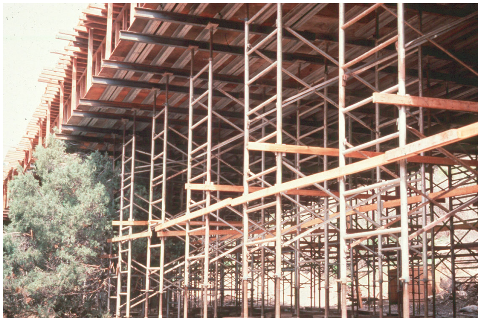
Figure 9.11.5 High Level Casting Formwork on Falsework
