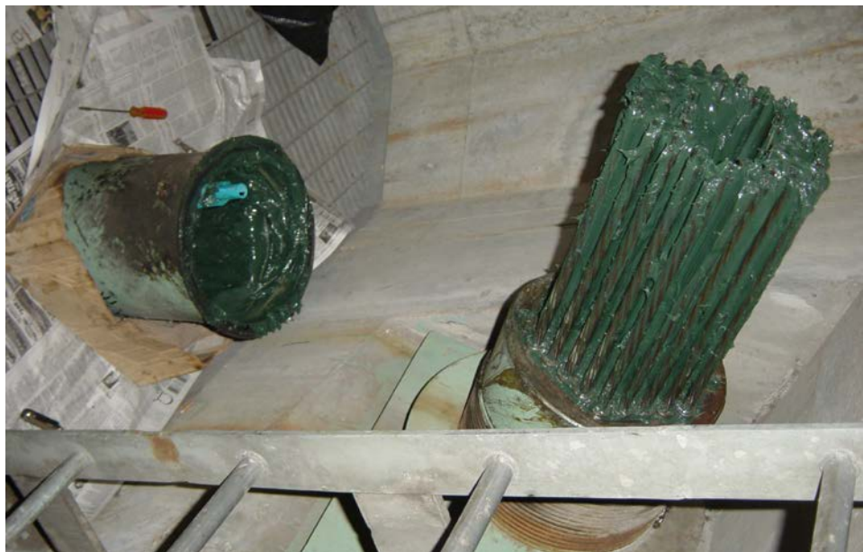
Figure 16.1.34 Anchor Inspection on Veterans Bridge
