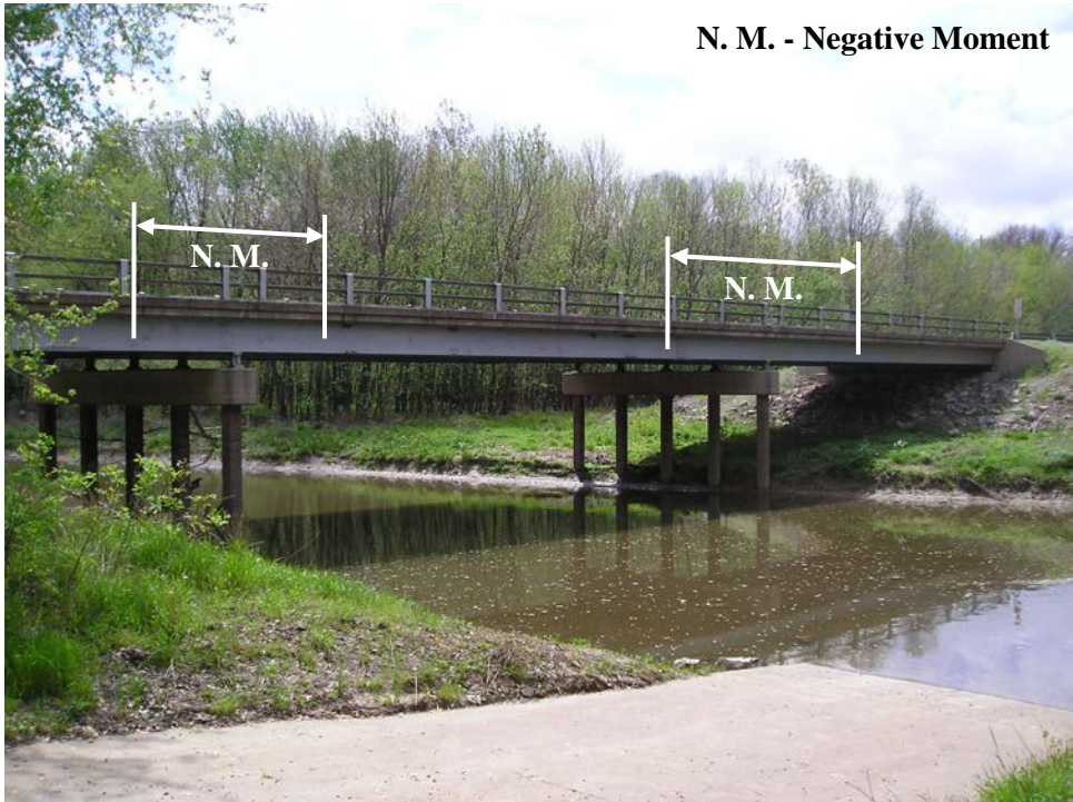
Figure 10.1.19 Negative Moment Region on a Continuous Span Rolled Multi-Beam Bridge
