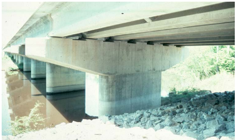
Figure 13.3.18 Cantilever or Hammerhead Pier
