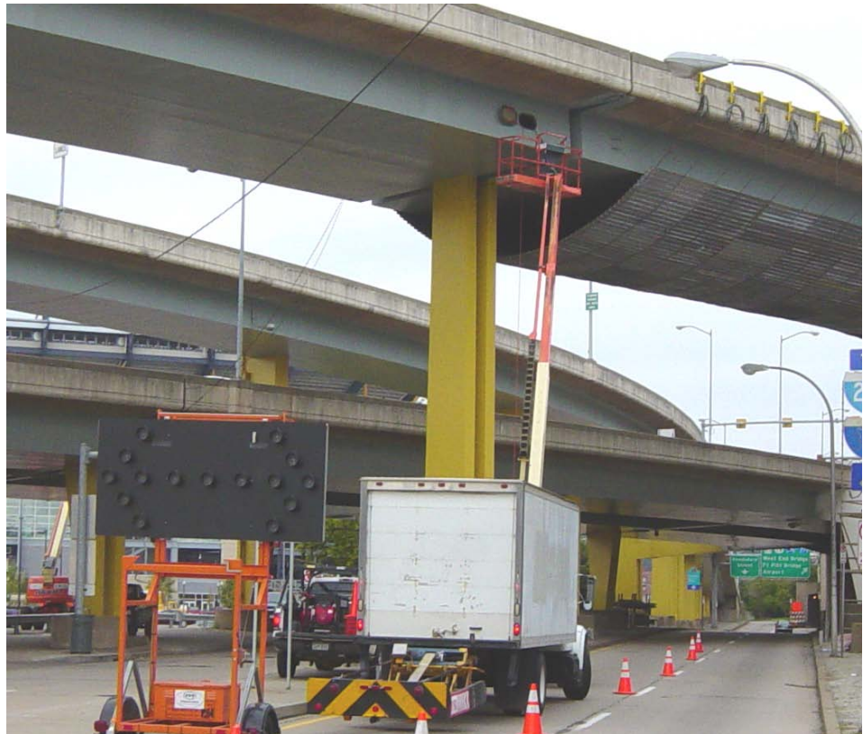
Figure 10.3.7 Box Girder Access Door
