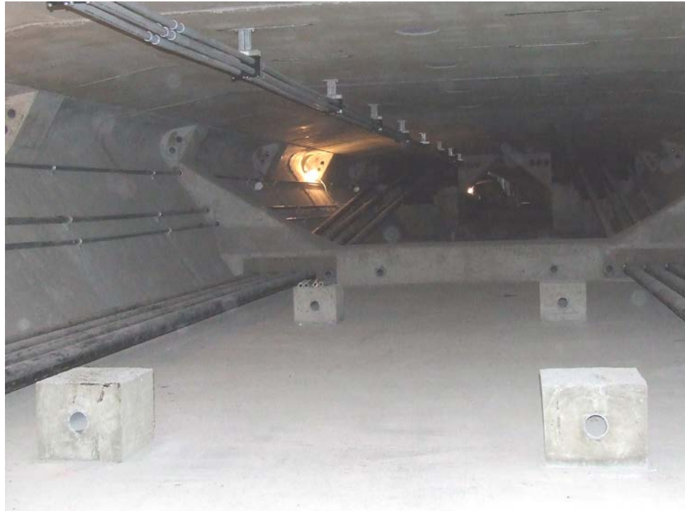
Figure 9.11.36 Temporary Deviation Blocks Used to Maintain Tendon Alignment During Construction
