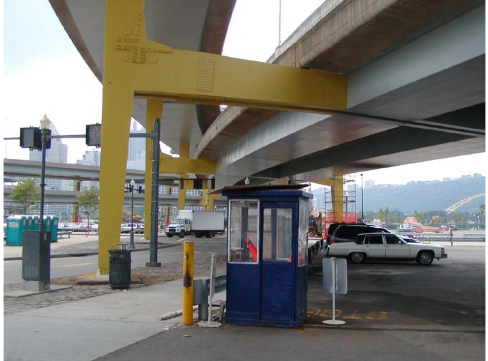
Figure 12.2.51 Fracture Critical Steel Bent
