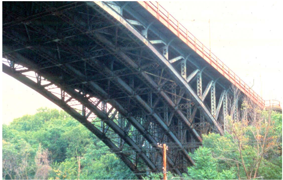
Figure 10.5.7 Spandrel Braced Deck Arch with Six Arch Ribs
