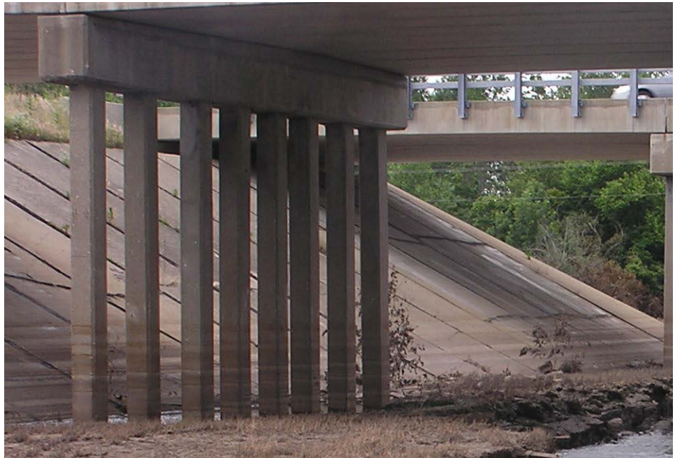
Figure 3.1.10 Concrete Pile Bent
