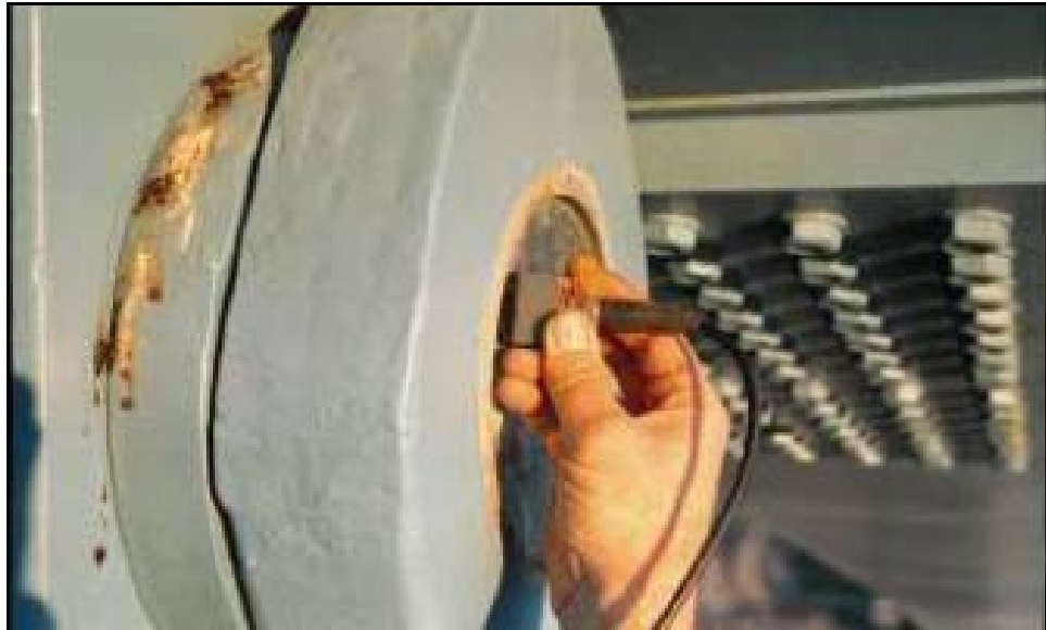
Figure 10.9.30 Ultrasonic Inspection of Eyebars Pin
