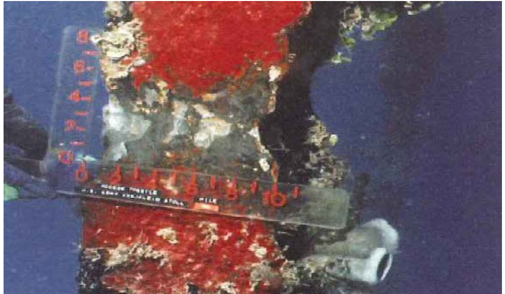
Figure 13.3.3 Level II Cleaning of a Steel Pile
