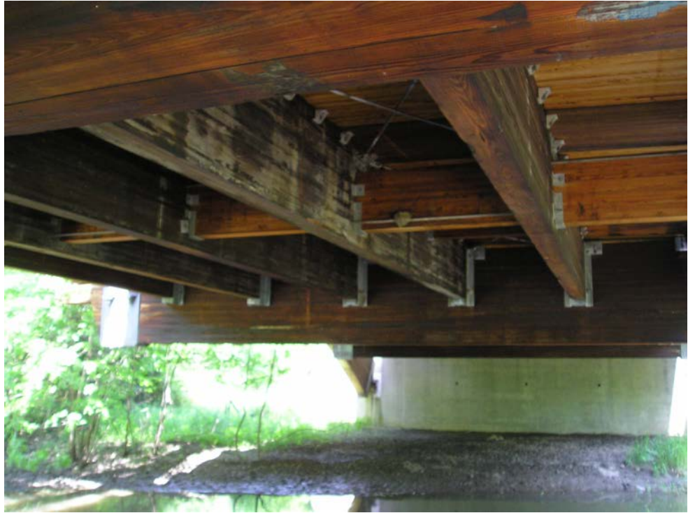
Figure 8.2.2 Underside View of a Glulam Multi-beam Bridge
