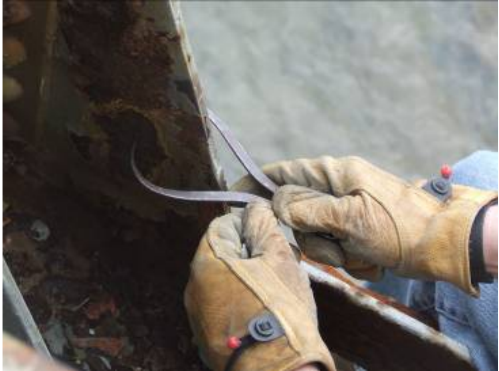
Figure 10.8.20 Inspector Using Calipers Measure the Thickness of the Gusset Plate
