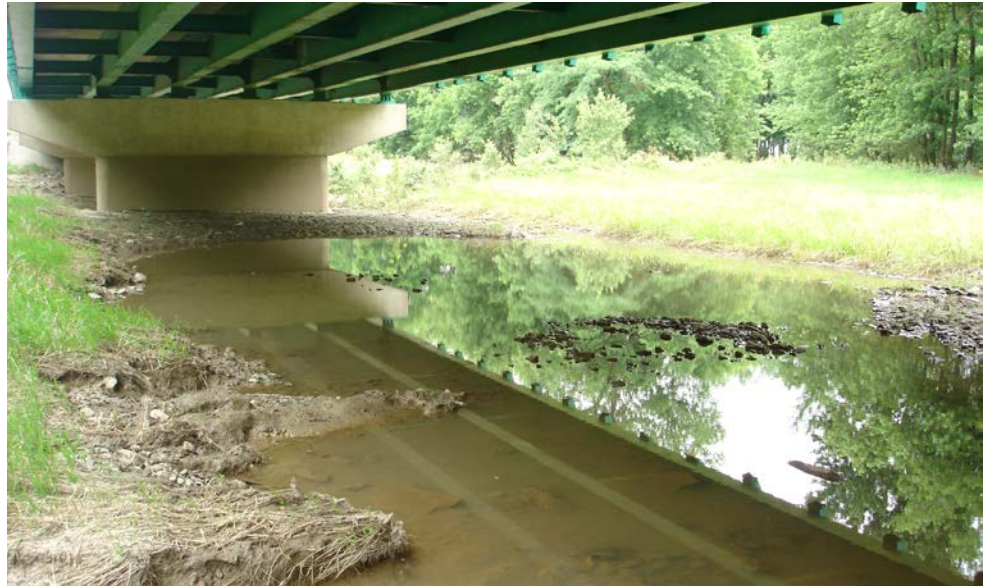
Figure 13.2.7 Contraction Scour Photograph
