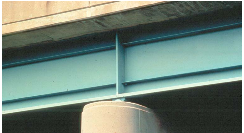
Figure 10.2.14 Longitudinal Stiffener in Tension Zone on a Two-Girder Bridge
