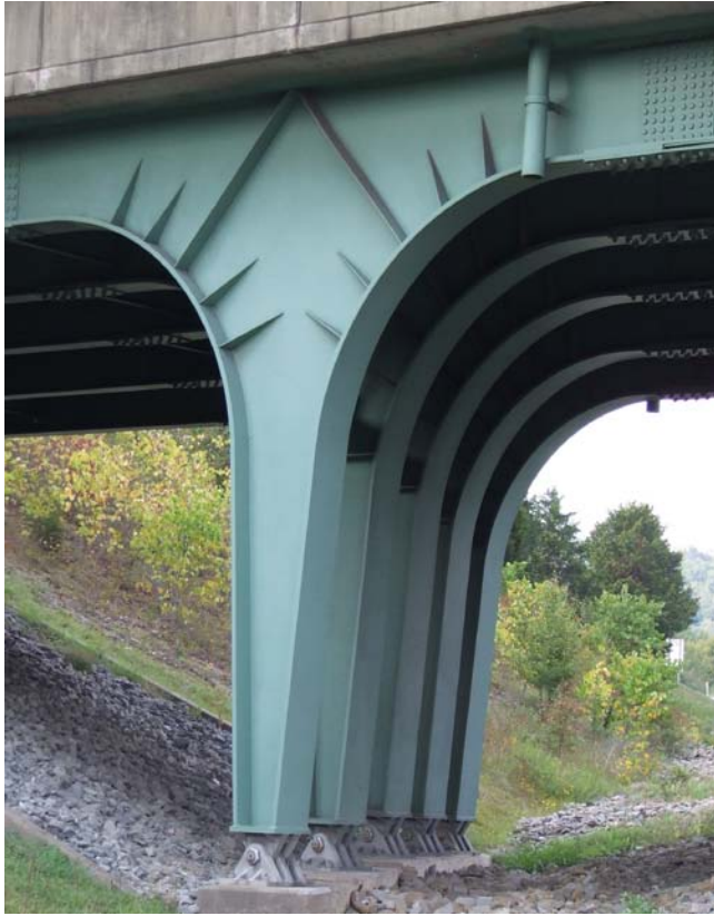
Figure 10.6.2 Typical Rigid Frame Constructed of Multiple Frames
