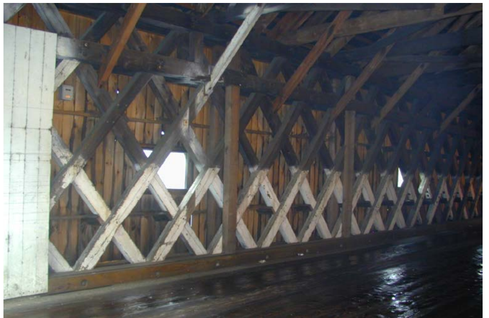
Figure 8.1.10 Town Truss Design
