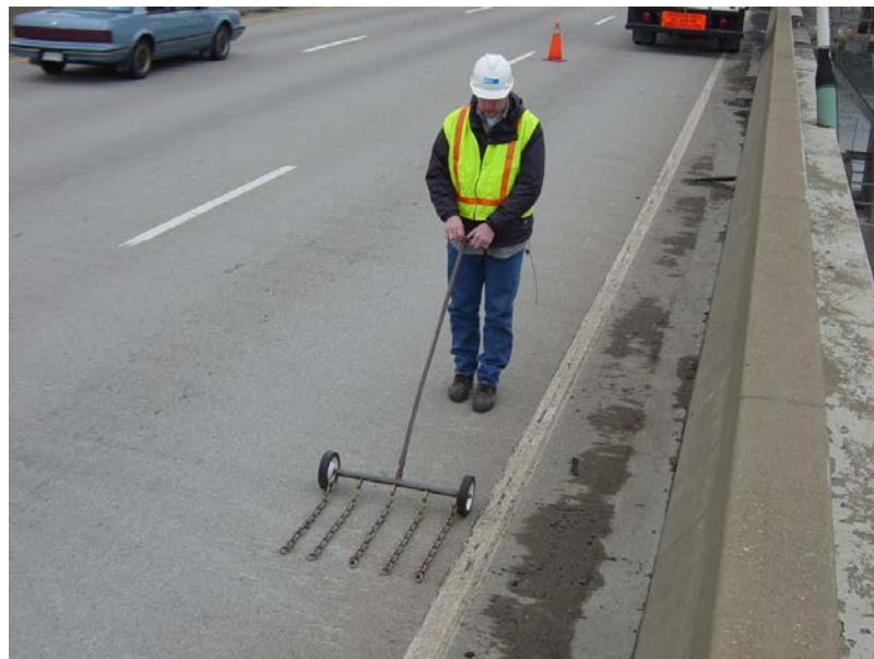
Figure 7.2.7 Sounding for Delaminated Areas of Concrete
