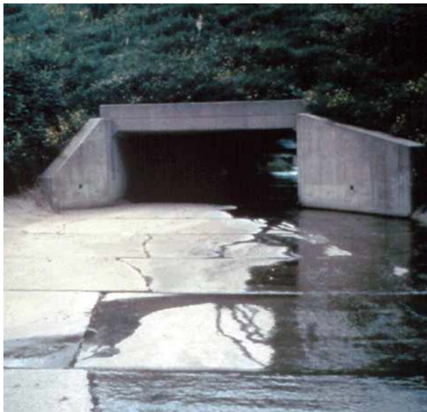
Figure 13.1.15 Formed Concrete Channel Lining
