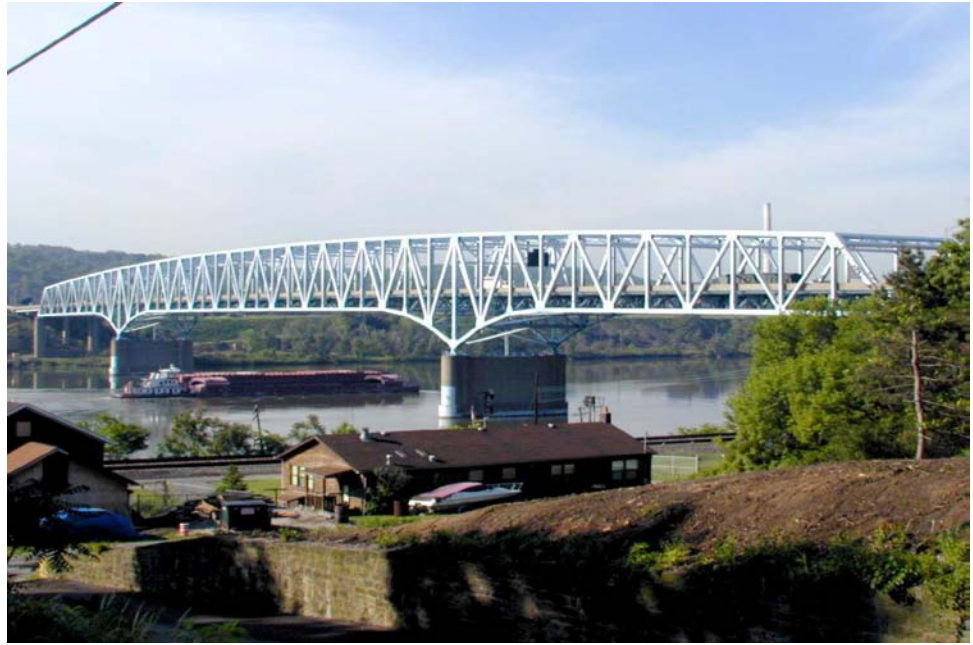
Figure 10.4.14 Continuous Through Truss
