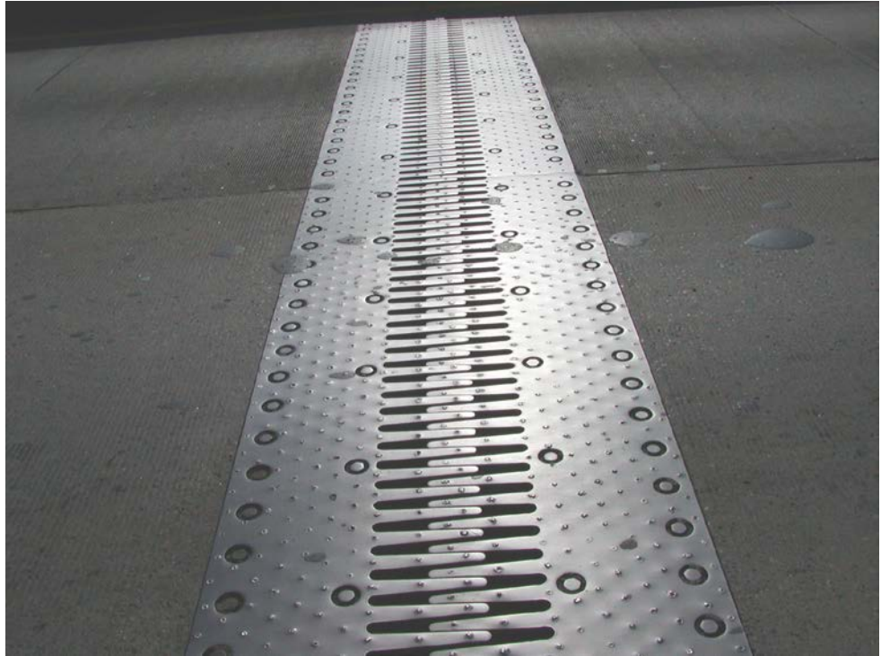
Figure 7.5.14 Finger Plate Joint
