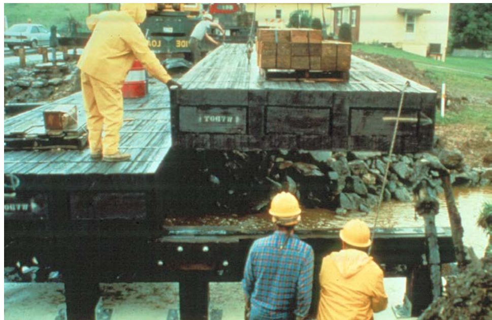
Figure 6.1.28 Coal-Tar Creosote Treated Timber Beams (Source: Barry Dickson, West Virginia University)
