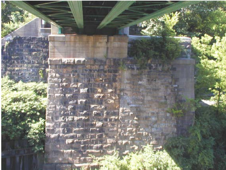
Photo No.6 Pier 1 - North Face (Looking South)
