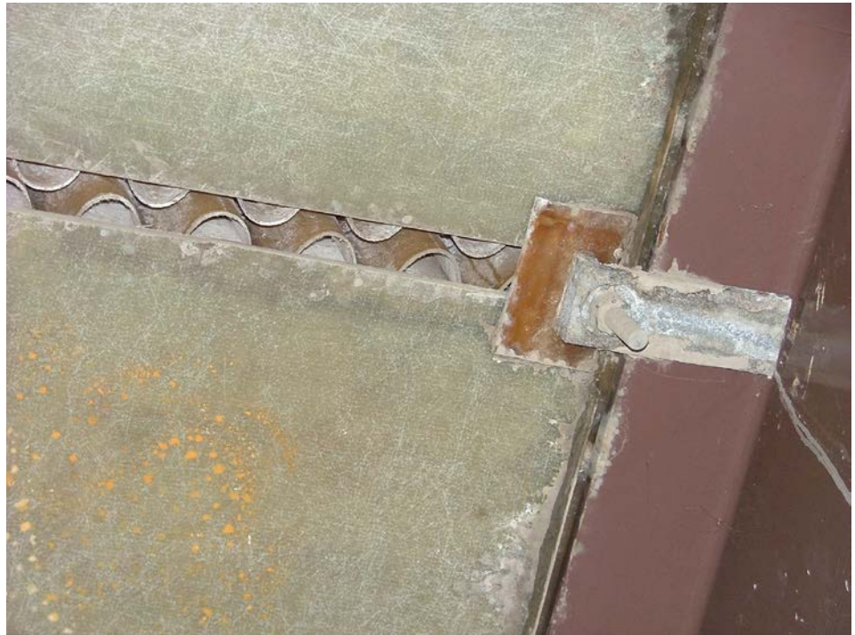
Figure 3.1.35 Fiber Reinforced Polymer (FRP) Deck
