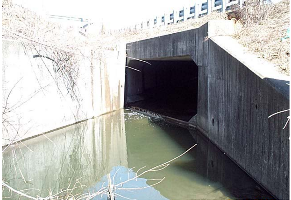
Figure 14.1.20 Culvert Skewed End
