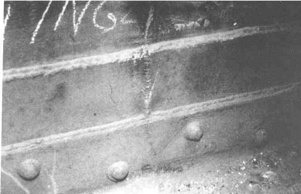
Figure 6.4.8 Patch Plate Welded on Riveted Girder Web along Flange Angle
