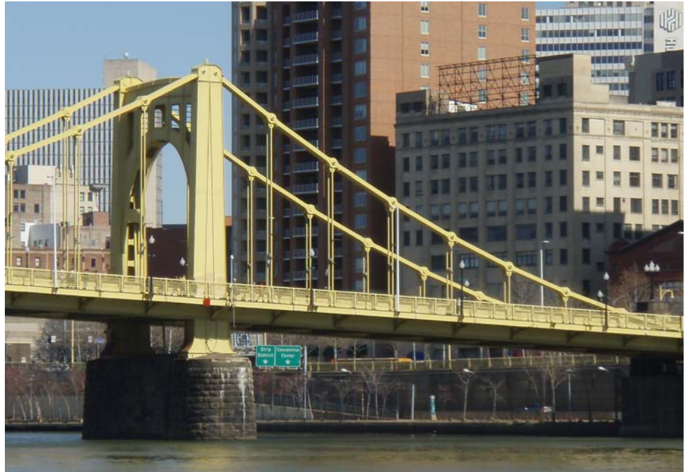
Figure 10.9.3 Eyebar Chain Suspension Bridge
