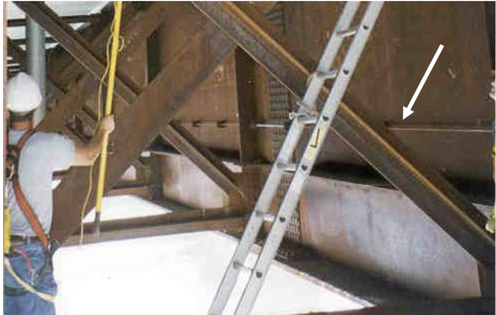
Figure 2.5.13 Handrail on Girder Bridge
