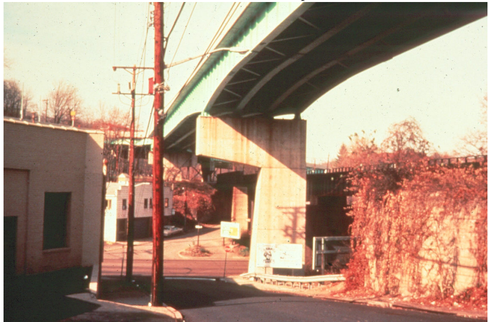
Figure 3.1.6 Unusual Concrete Shapes
