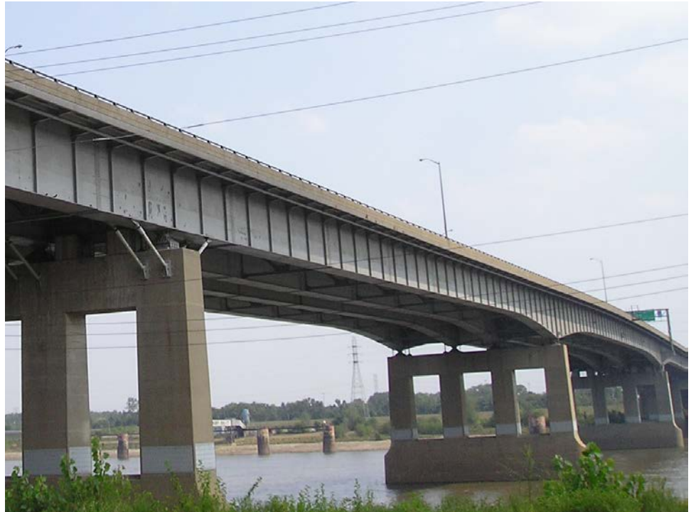
Figure 10.1.7 Continuous Span Fabricated Multi-girder Bridge
