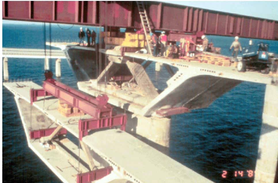
Figure 9.11.20 Balanced Cantilever Construction Using An Overhead Launching Gantry
