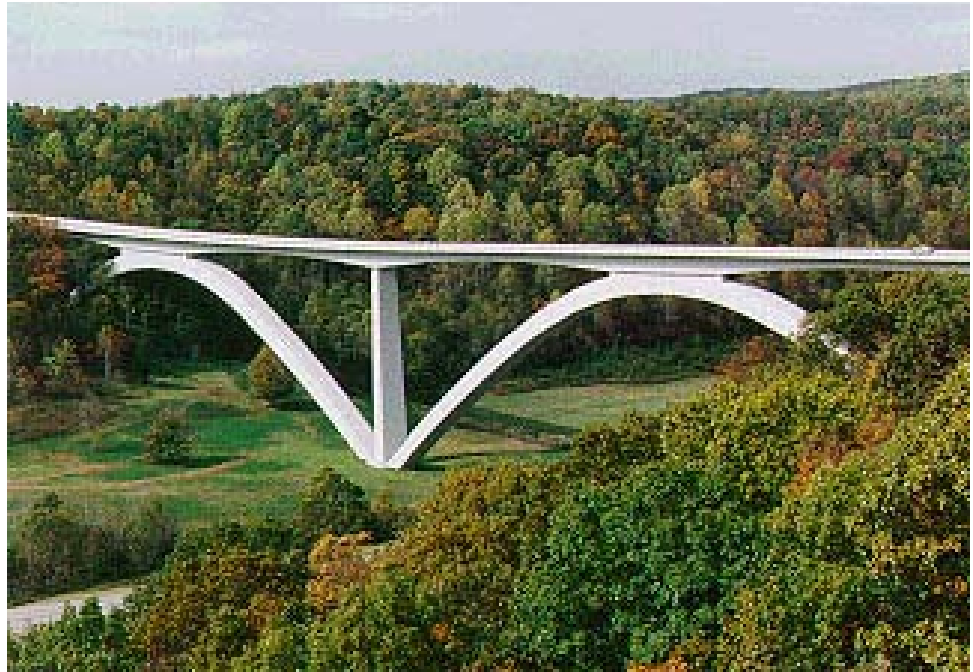
Figure 9.5.6 Precast Post-tensioned Concrete Arch without Spandrel Columns
