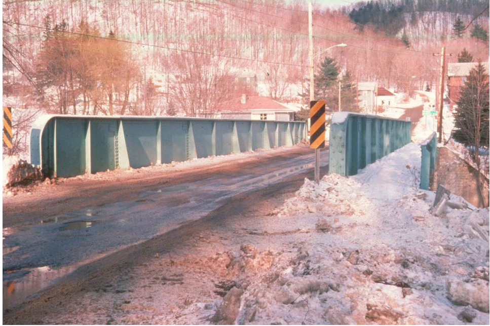
Figure 10.2.2 Through Girder Bridge
