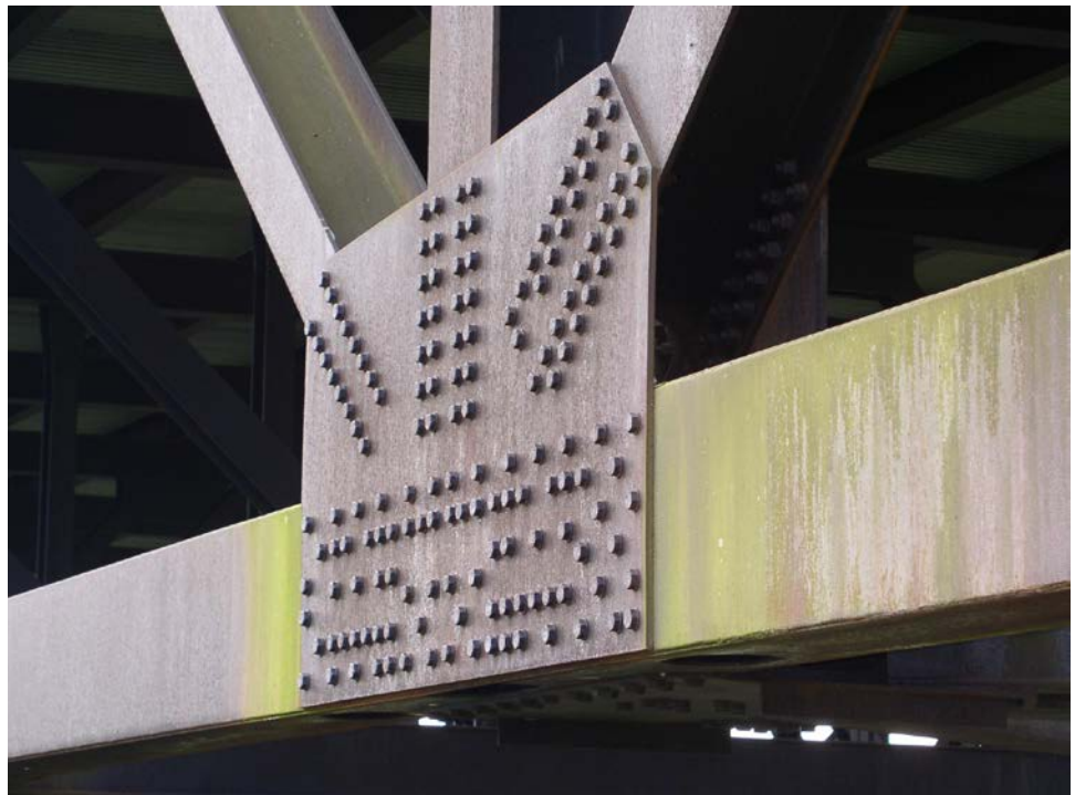
Figure 10.8.8 Gusset Plate Connecting Primary Load-Carrying Truss Members
