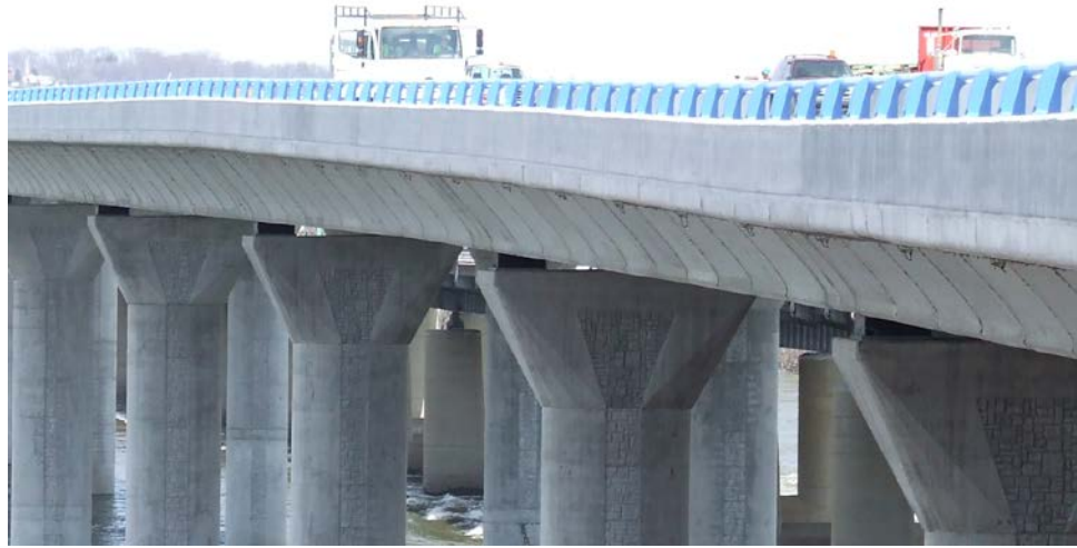
Figure 9.11.14 Segmental Concrete Bridge
