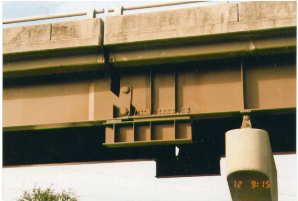
Figure 10.7.25 Underslung Catcher Retrofit
