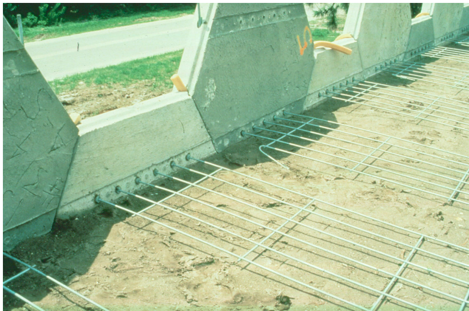
Figure 12.1.10 Mechanically Stabilized Earth Wall Under Construction
