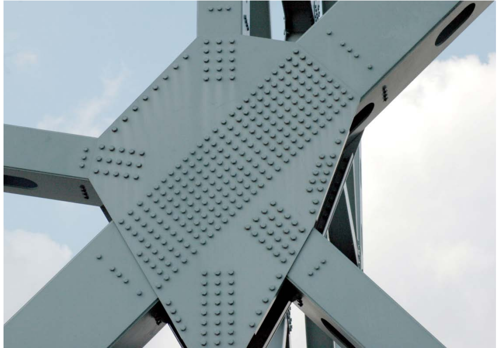
Figure 10.8.7 Odd-Shaped Gusset Plate Connecting Primary Load-Carrying Truss Members
