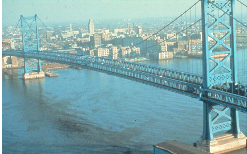
Figure 10.4.6 Suspension Bridge with Stiffening Truss
