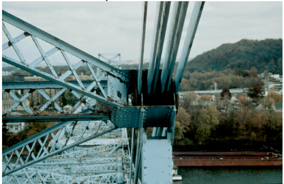
Figure 10.9.32 Fracture Critical Top Chord Truss Member: Internally Redundant Eyebar
