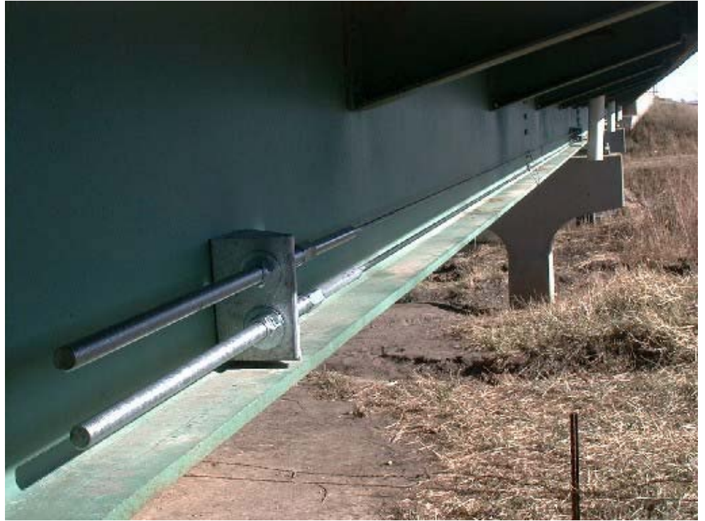
Figure 6.6.3 CFRP Post-tensioned Steel Girder
