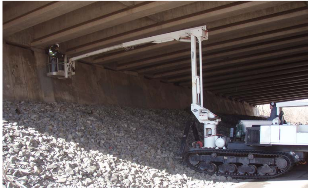
Figure 2.5.19 Track-mounted Man-lift on a Slope
