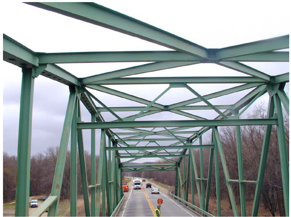
Figure 3.1.67 Top Lateral Bracing and Sway Bracing
