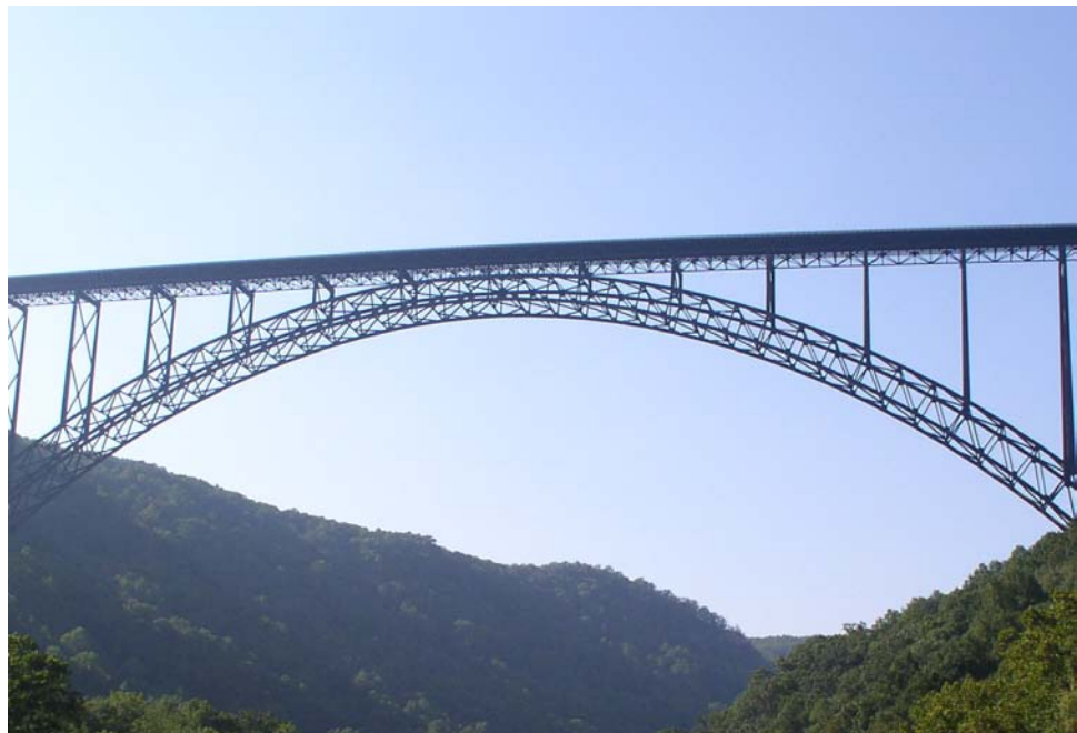
Figure 10.4.7 Deck Arch Bridge with Stiffening Truss
