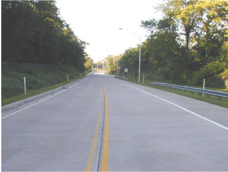
Photo No.3 North Approach (far)
