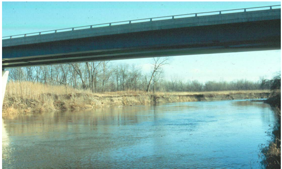
Figure 10.3.1 Simple Span Box Girder Bridge
