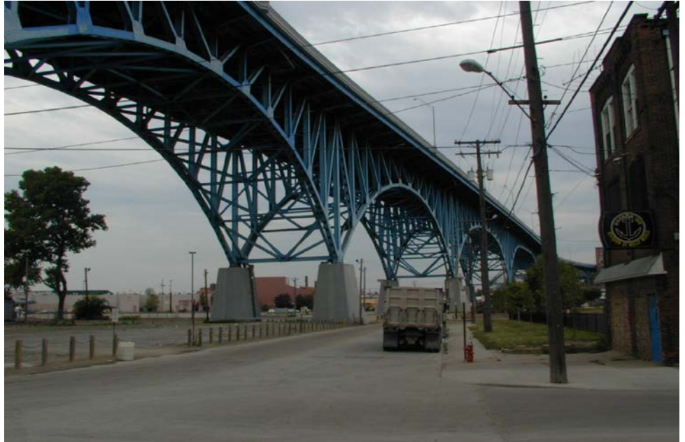
Figure 3.1.52 Deck Truss Bridge
