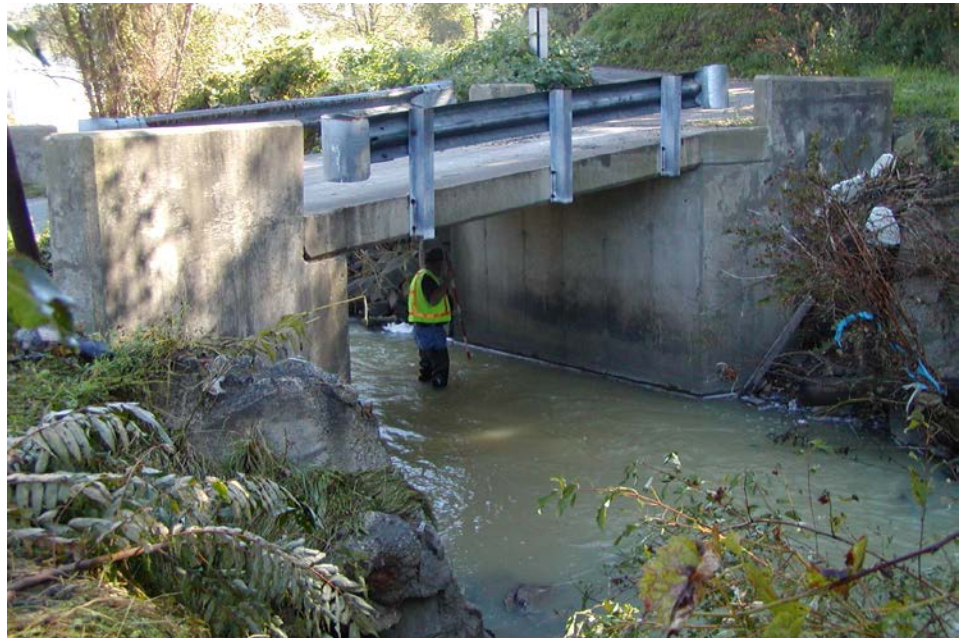
Figure 12.1.51 Inspector Checking for Scour
