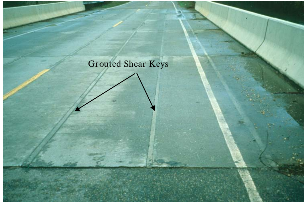
Figure 9.4.6 Top of Deck View of Precast Channel Beam Bridge
