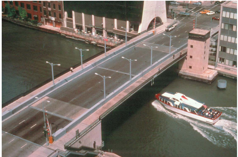
Figure 16.2.11 Double-Leaf Trunnion Bascule Bridge
