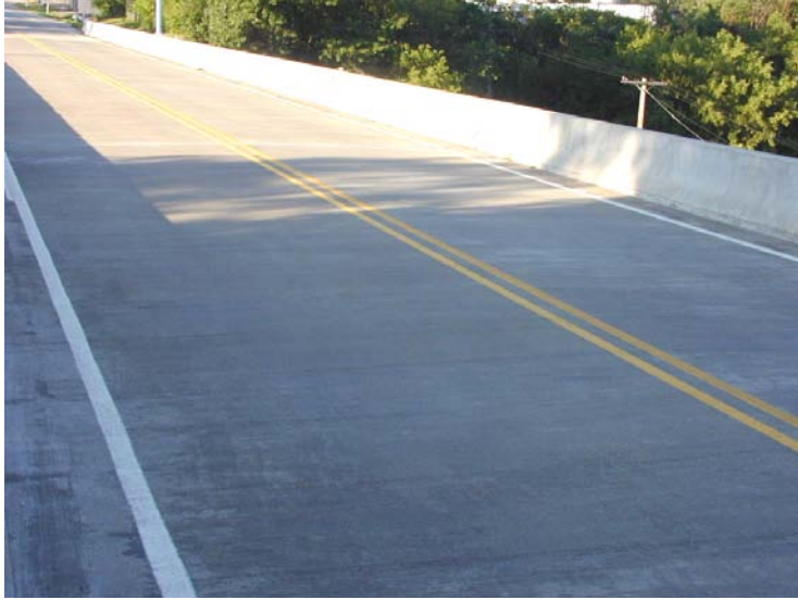
Photo No. 11 General Deck View
