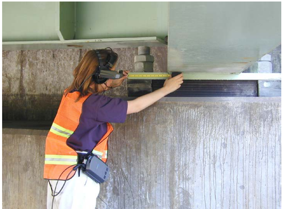
Figure 4.1.9 Inspector Using Wearable Computer
