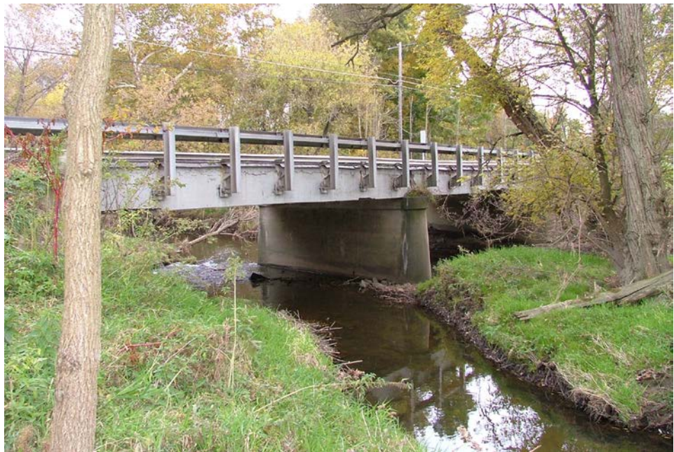
Figure 13.2.44 Sediment Accumulation Redirecting Streamflow
