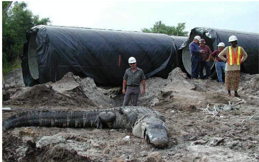
Figure 14.2.5 Concrete Pipe Culvert
