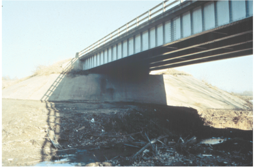
Figure 13.2.42 Approach Roadway Built in the Floodplain
