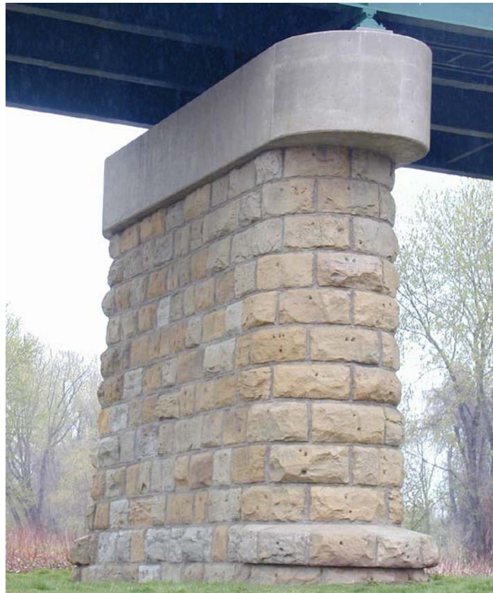
Figure 3.1.76 Solid Shaft Pier
