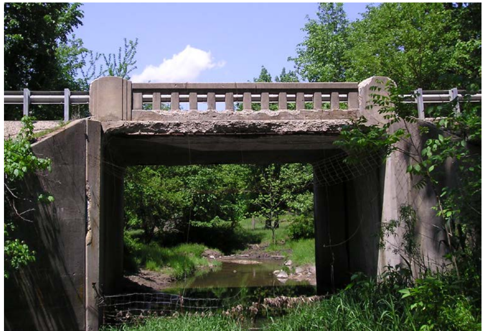
Figure 9.1.1 Typical Simple Span Cast-in-Place Slab Bridge
