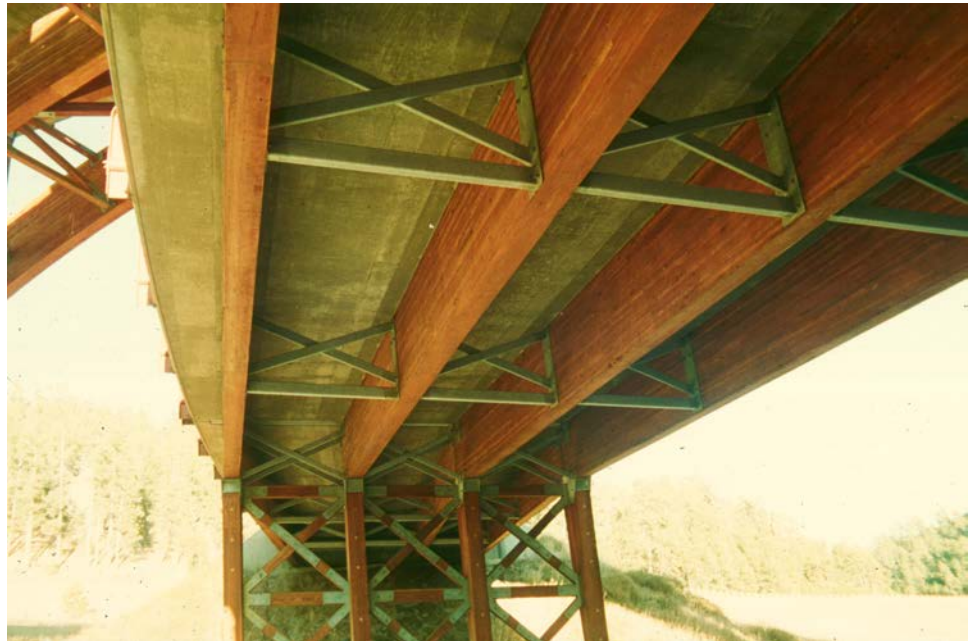
Figure 8.2.14 Glulam Beams with Numerous Fastener Locations
