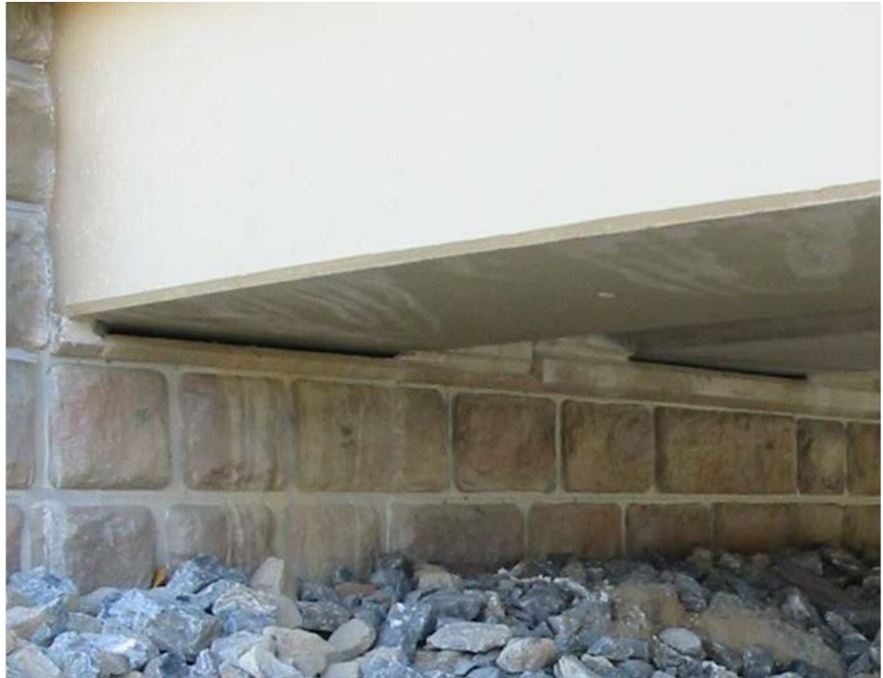
Figure 11.1.18 Enclosed or Concealed Bearing
