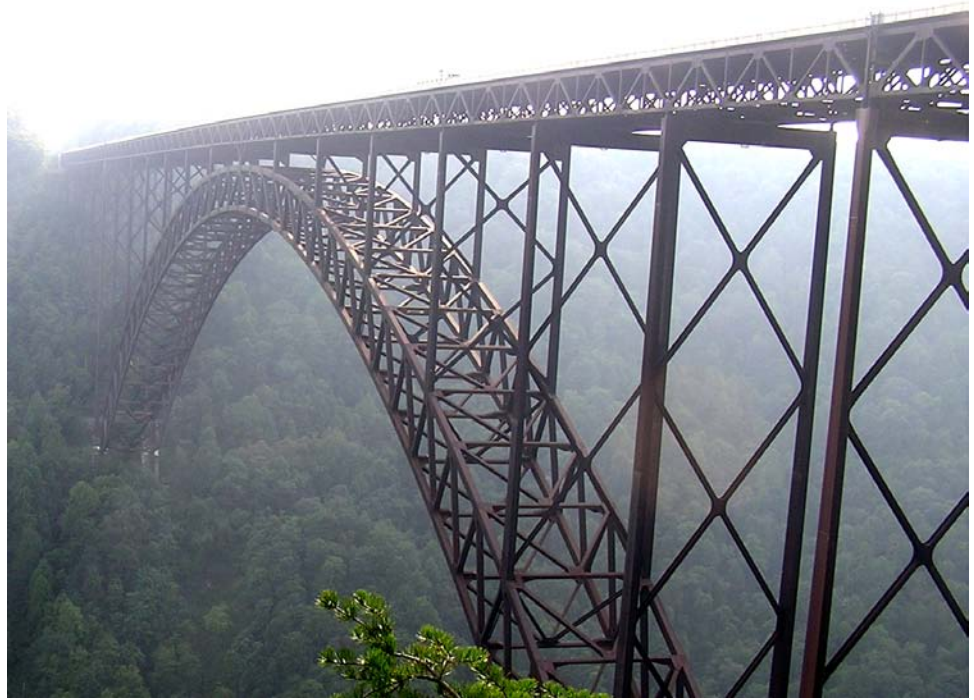
Figure 10.5.6 Braced Rib Deck Arch, New River Gorge, WV
