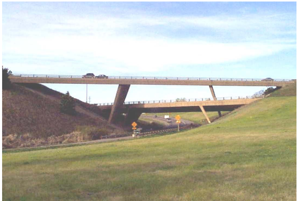
Figure 9.6.1 Multi-span Concrete Rigid Frame Bridges
