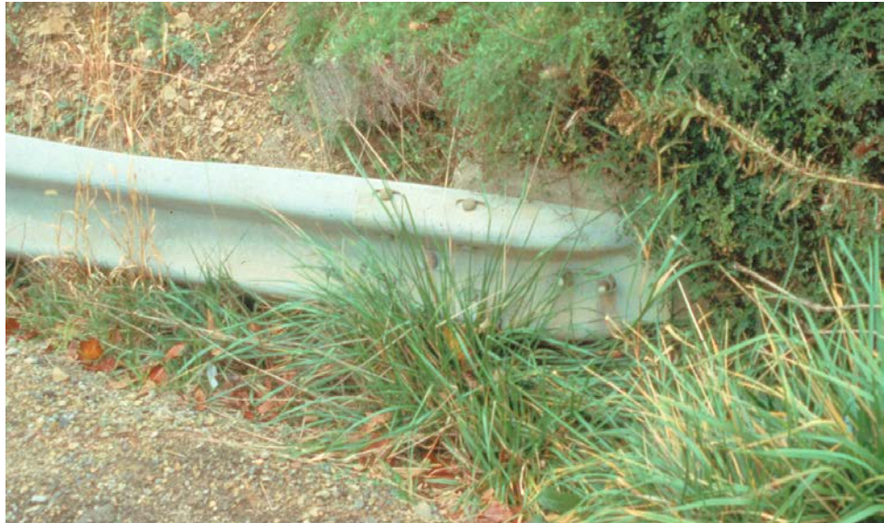
Figure 7.6.10 W-Shaped Guardrail End Flared and Buried into an Embankment
