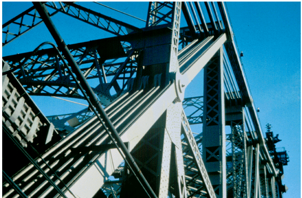
Figure 10.9.2 Eyebare Cantilevered Truss Bridge (Queensboro Bridge, NYC)
