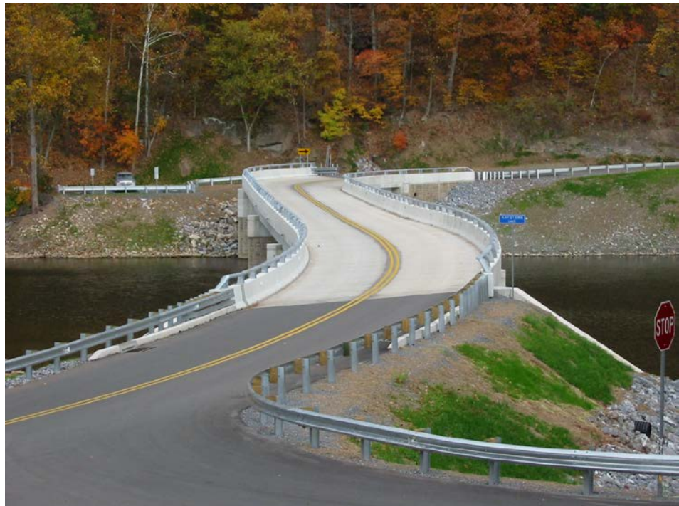
Figure 3.1.28 Bridge Deck with a Smooth Riding Surface
