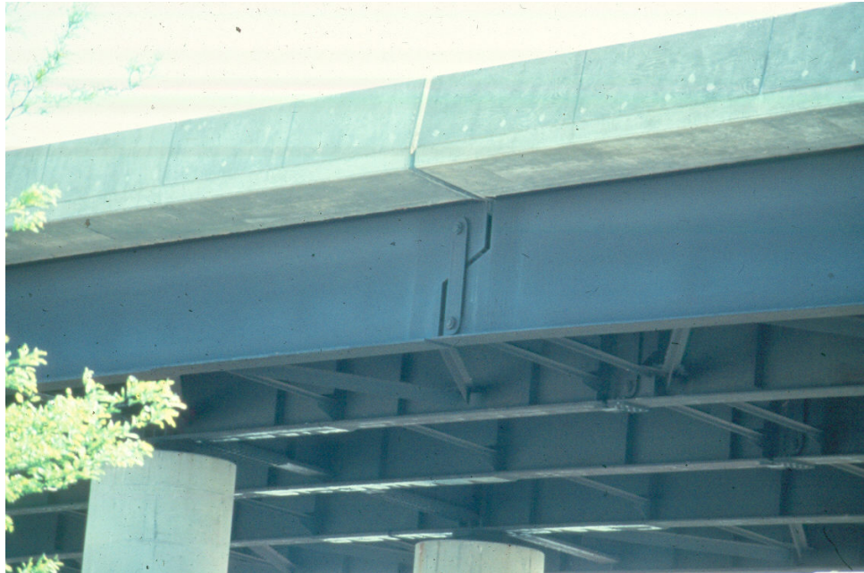
Figure 10.1.9 Fabricated Multi-girder Bridge with Pin & Hanger Connection
