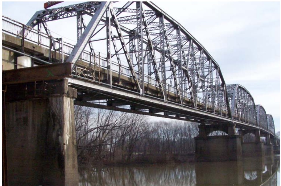
Figure 10.4.13 Multiple Span Through Truss
