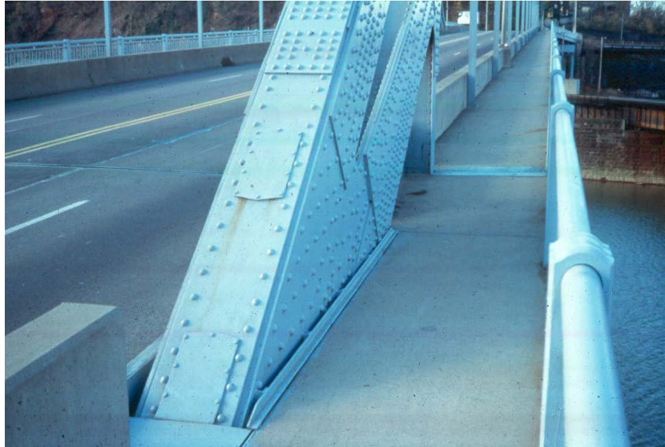
Figure 10.5.24 Through Arch Member Exposed to Traffic
