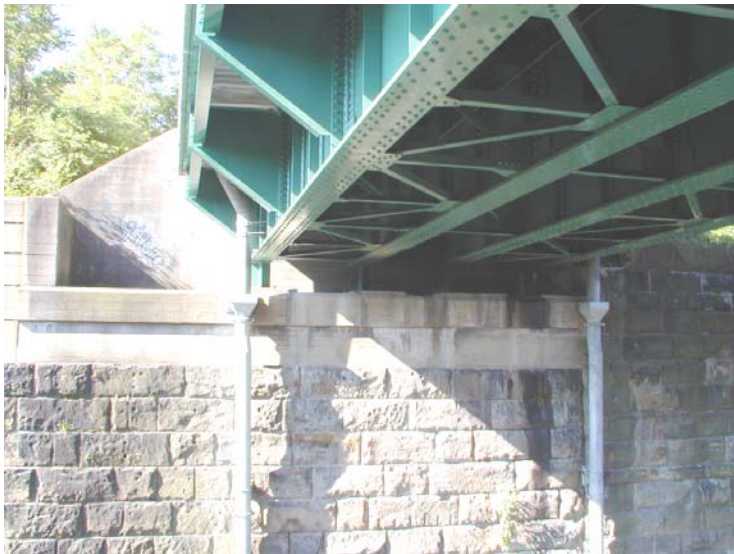
Photo No.4 South Abutment (near) - Elevation
