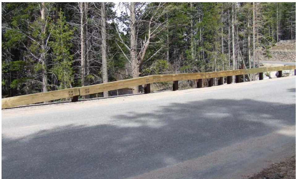
Figure 7.6.17 Timber Traffic Safety Features, Rocky Mountain National Park
