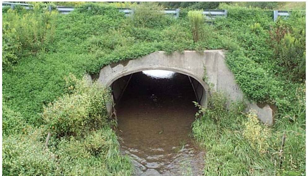
Figure 14.2.7 Concrete Arch Culvert
