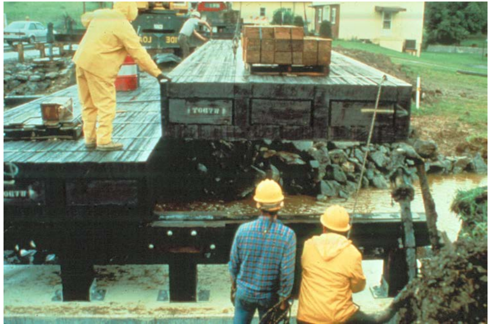
Figure 8.3.8 Stress-Laminated Timber Box Beam Bridge Being Erected
