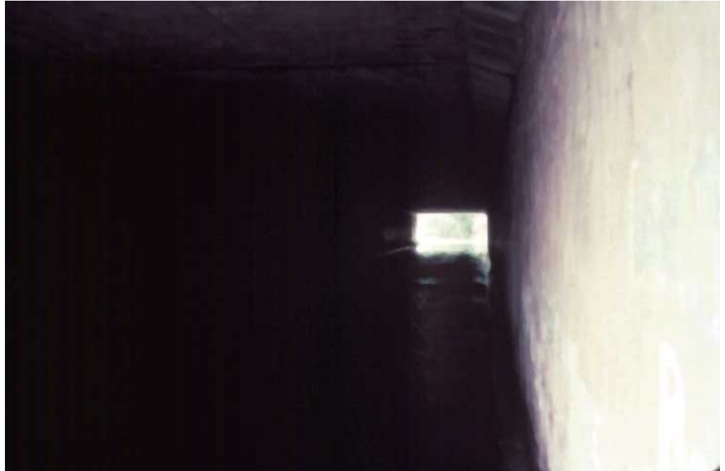
Figure 14.2.16 Sighting Along Culvert Sidewall to Check Horizontal Alignment
