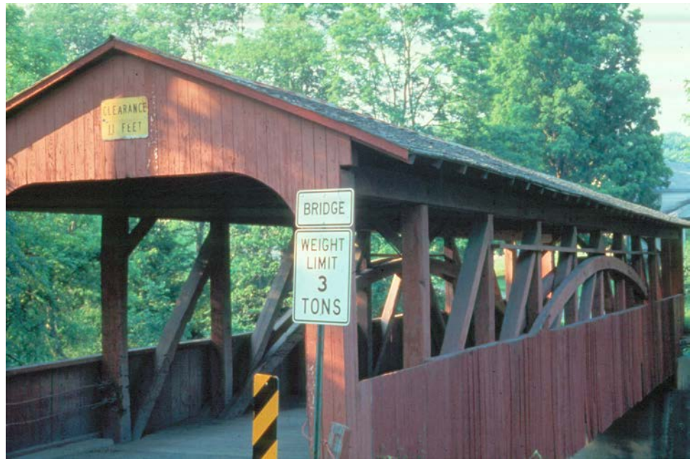
Figure 8.1.8 Burr Arch-truss Covered Bridge
