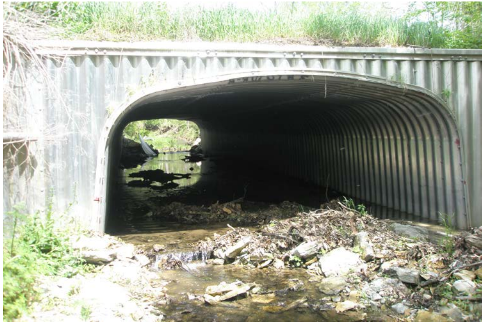
Figure 14.1.14 Large Structural Plate Box Culvert
