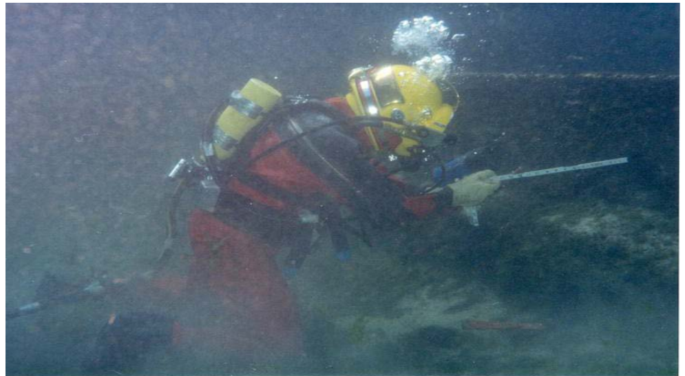
Figure 13.3.35 Surface-Supplied Diving Inspection
