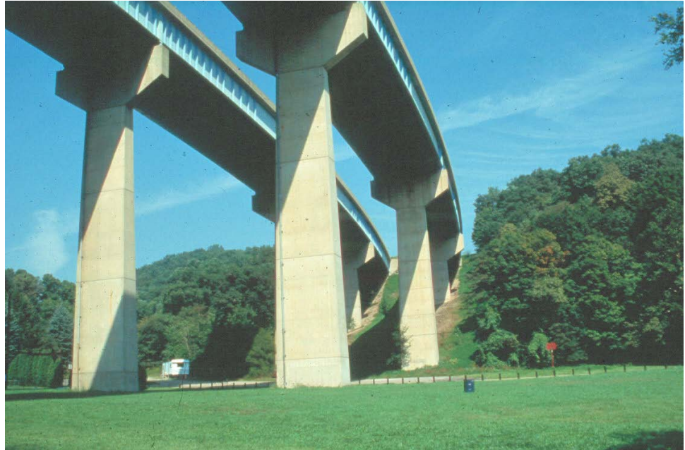
Figure 12.2.1 Example of Piers as Intermediate Supports for a Bridge
