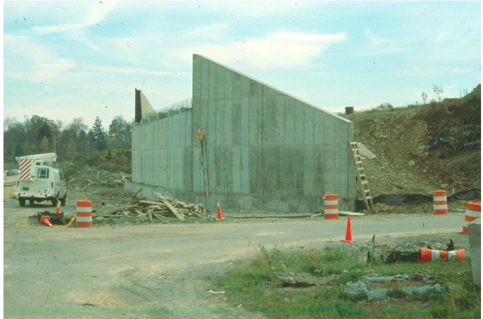
Figure 12.1.14 Reinforced Concrete Cantilever Abutment
