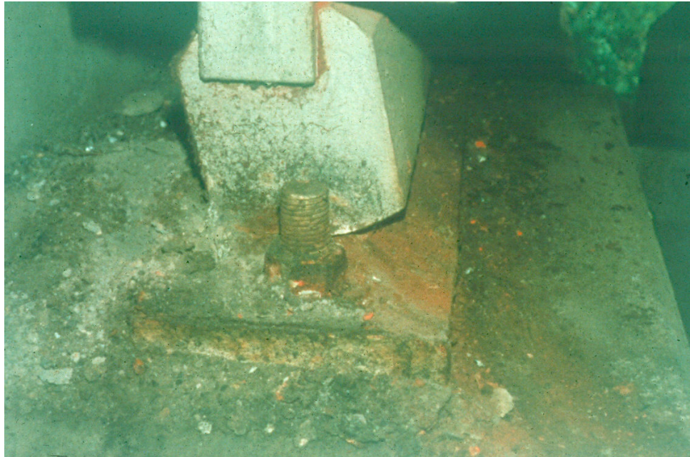
Figure 11.1.10 Segmental Rocker Bearing
