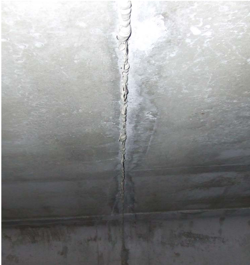
Figure 9.11.46 Close-up View of Box Girder Joint
