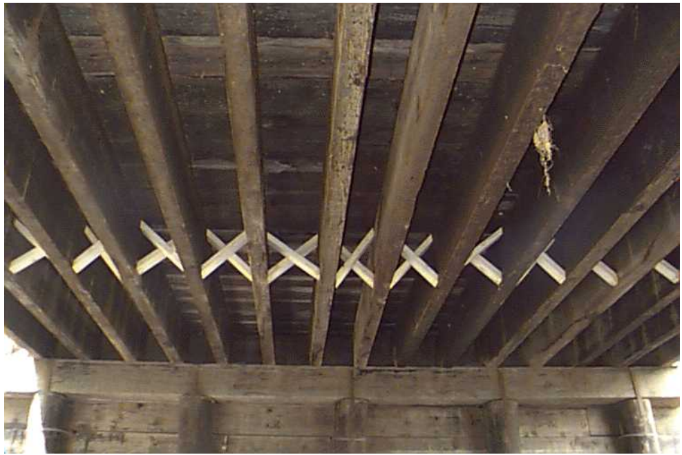
Figure 8.1.2 Underside View of a Solid Sawn Multi-Beam Bridge
