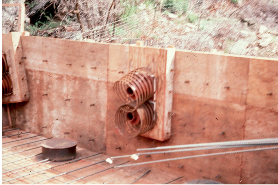
Figure 9.11.11 Post-tensioning Spiral Anchorage Reinforcement Prior to Concrete Placement
