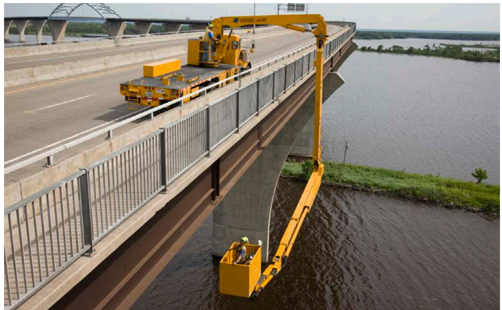
Figure 2.5.20 Under Bridge Inspection Vehicle with Bucket
