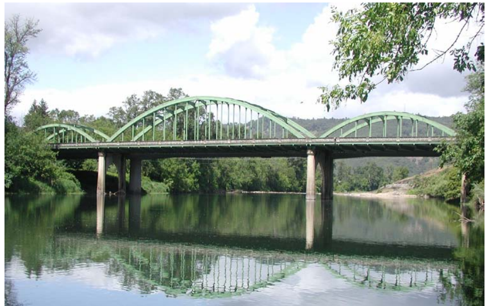
Figure 10.5.14 Three-Span Tied Arch Bridge
