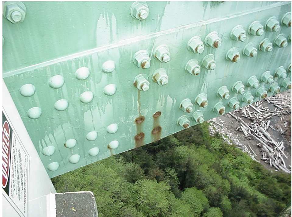
Figure 3.1.24 Shop Rivets and Field Bolts
