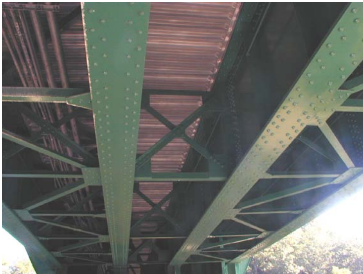
Photo No.8 General Underside View - Span 1
