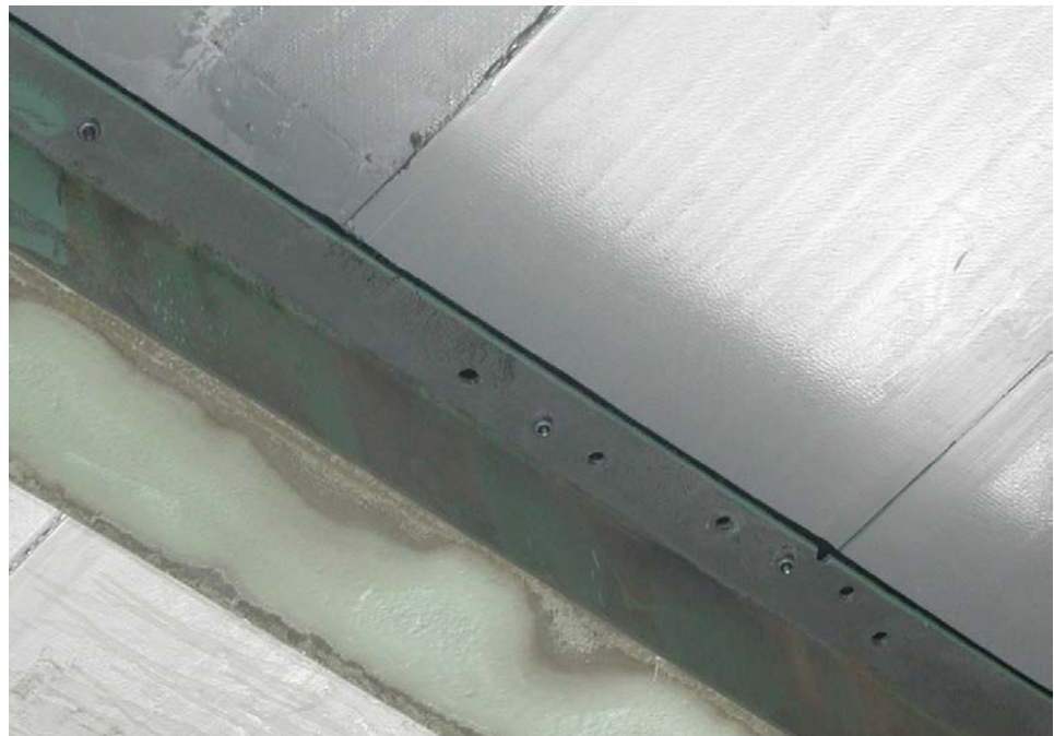
Figure 7.3.8 FRP Deck underside near superstructure beam
