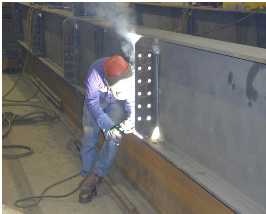
Figure 6.3.3 Steel Plate Welded to Girder
