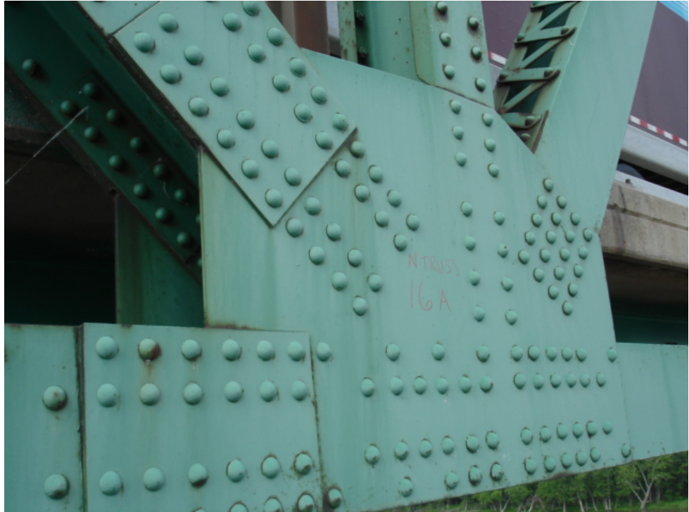
Figure 6.4.44 Riveted Gusset Plate Connection
