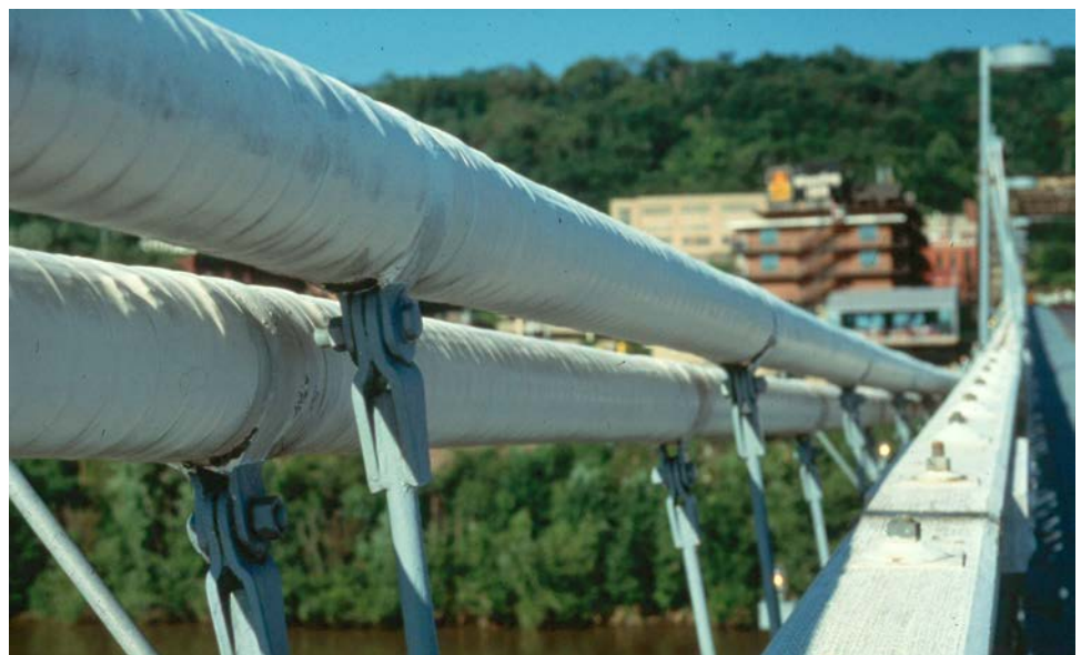
Figure 16.1.12 Cable Wrapping on the Wheeling Suspension Bridge
