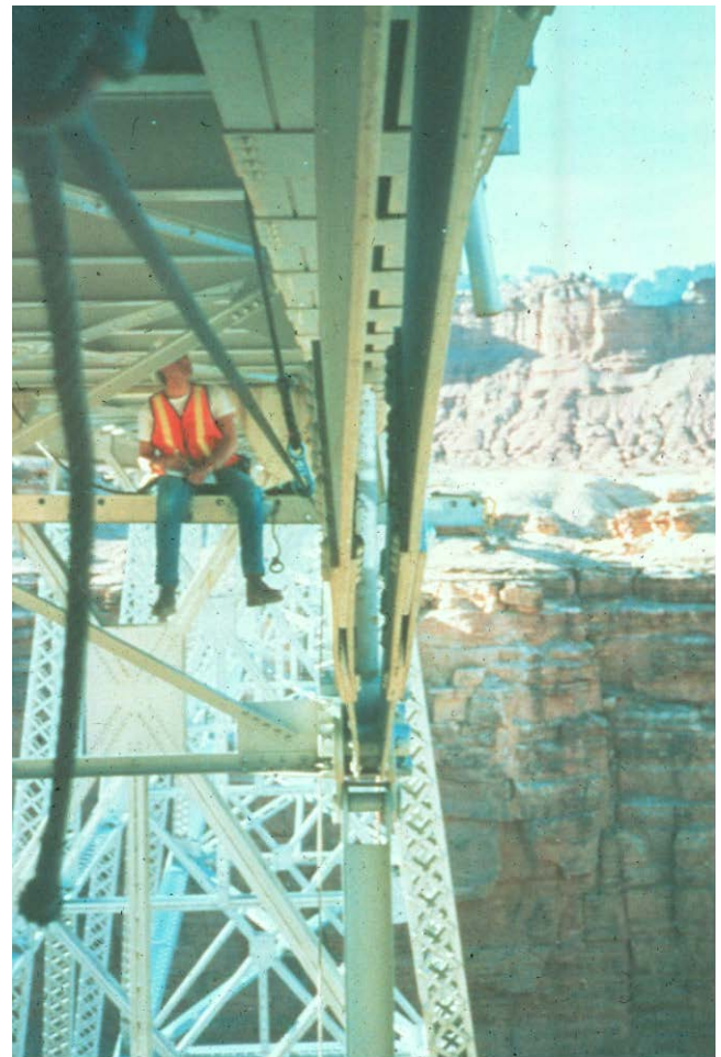
Figure 2.5.4 Rigging for Superstructure Inspection
