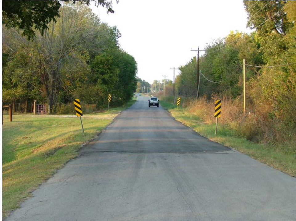
Figure 14.1.30 Repaired Roadway Over a Culvert
