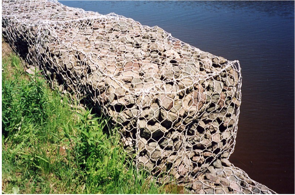
Figure 13.1.12 Gabion Basket Serving as Slope Protection
