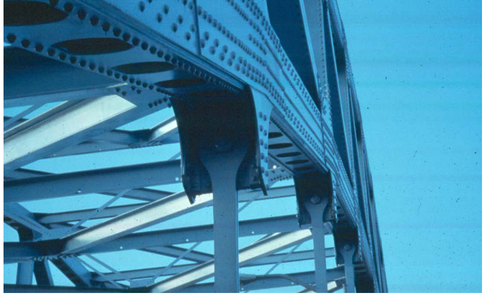
Figure 10.5.21 Hanger Connection on a Through Arch
