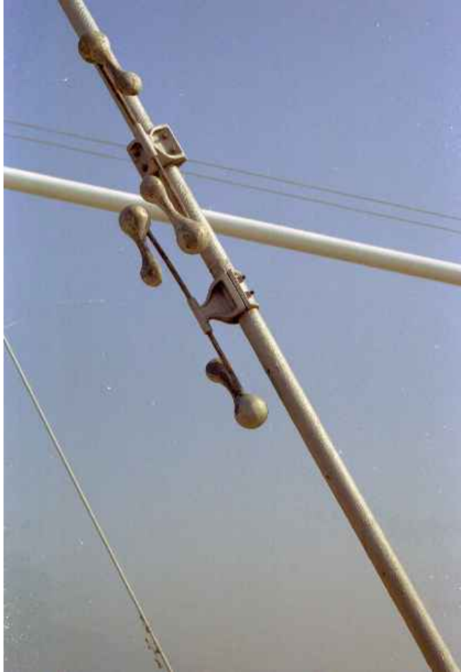
Figure 16.1.51 Tuned Mass Damper System
