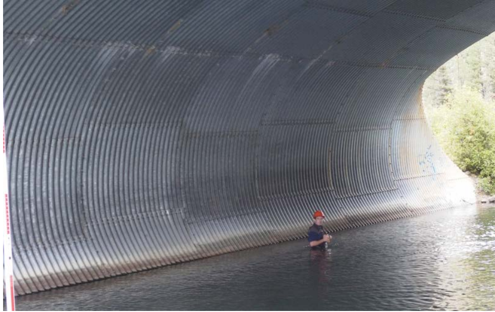
Figure 14.1.13 Large Structural Plate Pipe Arch Culvert
