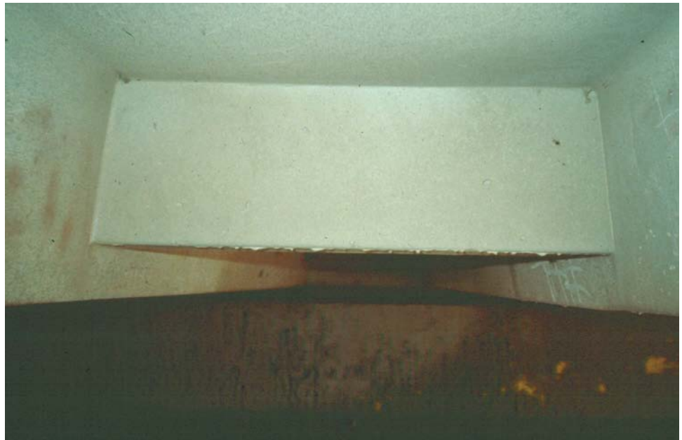
Figure 9.4.9 Close-up of Intermediate Diaphragm
