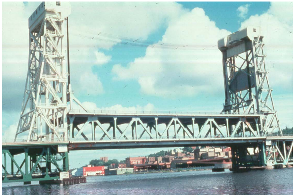
Figure 16.2.33 Concrete Counterweight on a Vertical Lift Bridge
