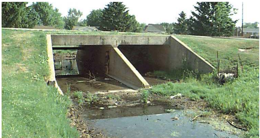
Figure 14.2.3 Multi-Cell Concrete Box Culvert
