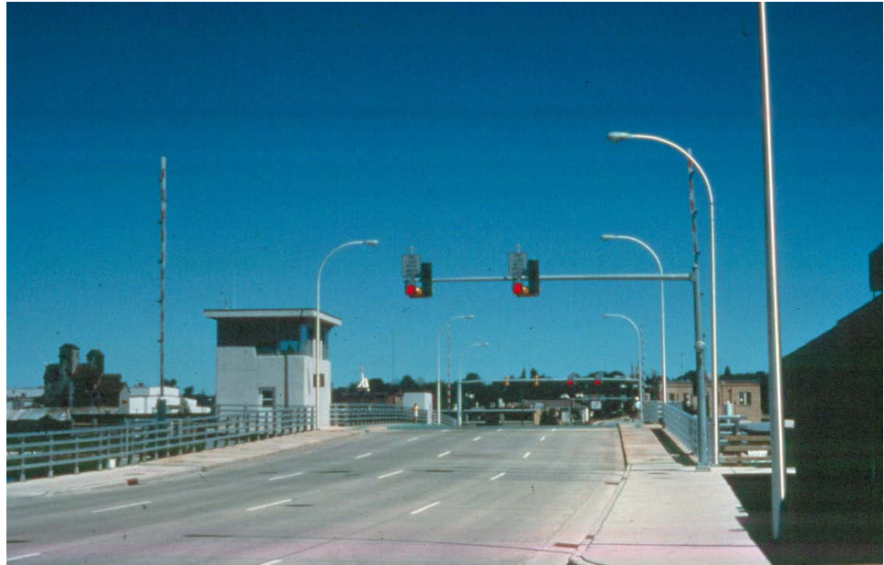
Figure 16.2.53 Operator's House with Clear View of Traffic Signals and Lane Gates
