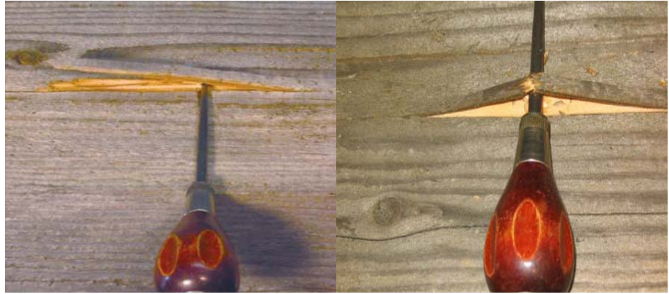
Figure 15.1.8 Pick Test: Sound Wood, Decayed Wood
