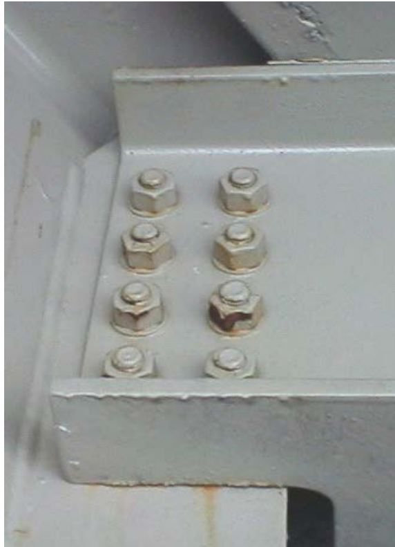
Figure 6.4.67 Blocked Floorbeam Flange
