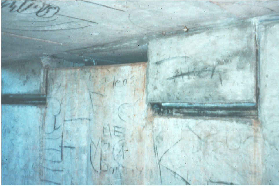
Figure 9.11.28 Bearing Area of a Box Girder Bridge
