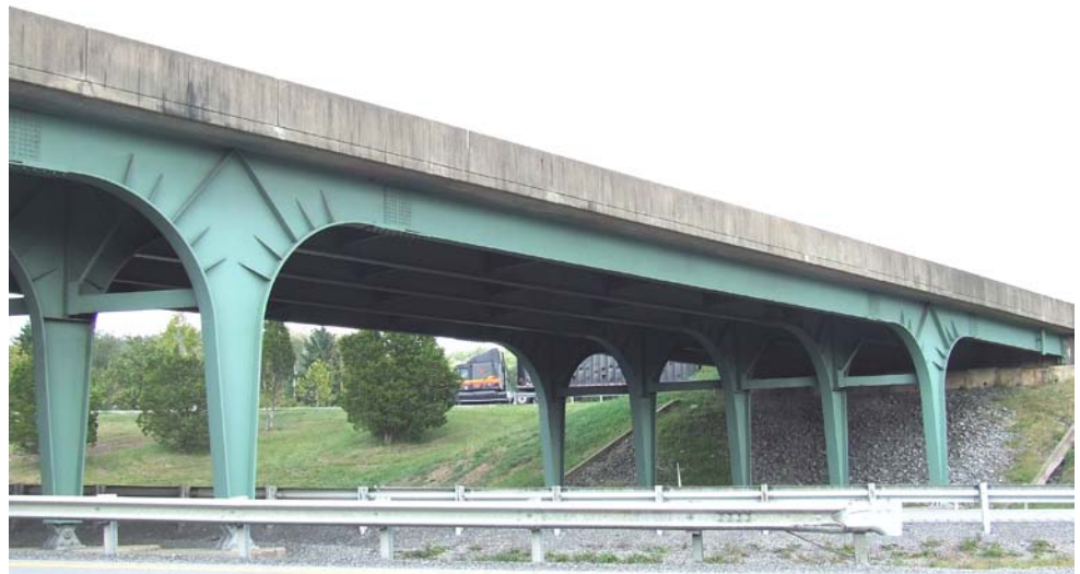
Figure 10.6.12 Multiple Frame Rigid Frame – Not a Fracture Critical Structure
