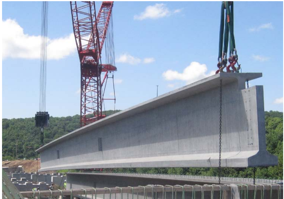
Figure 9.9.5 Placement of an AASHTO-PCI Bulb-Tee Beam
