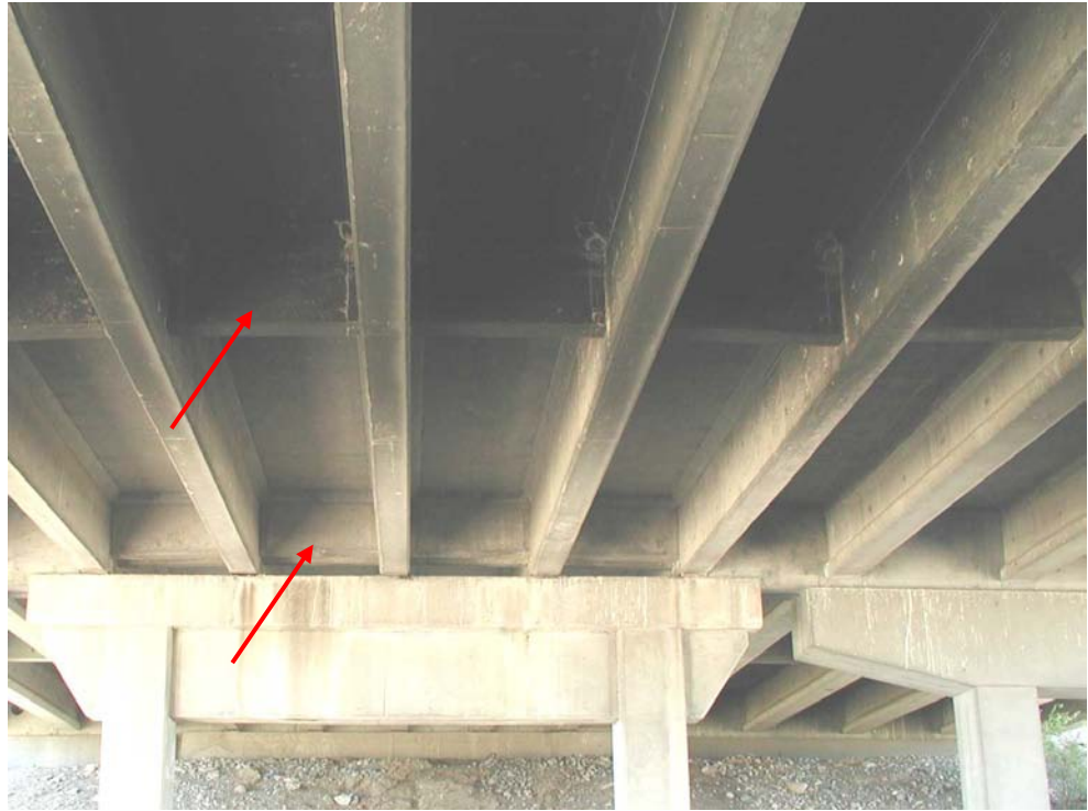
Figure 9.9.12 Concrete Intermediate and End Diaphragms
