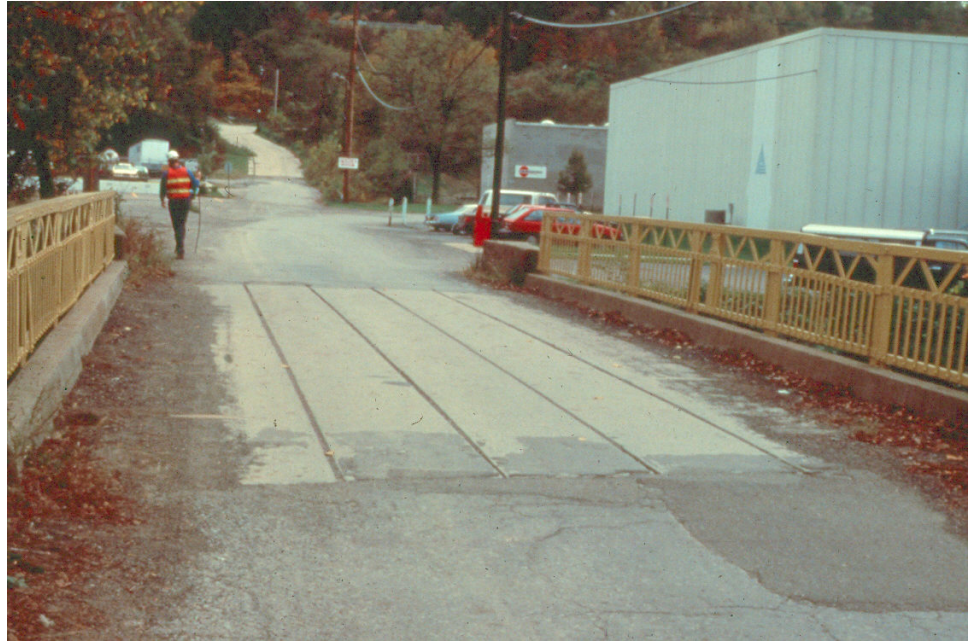
Figure 9.10.5 Adjacent Box Beams: Top Flanges Acting as the Deck
