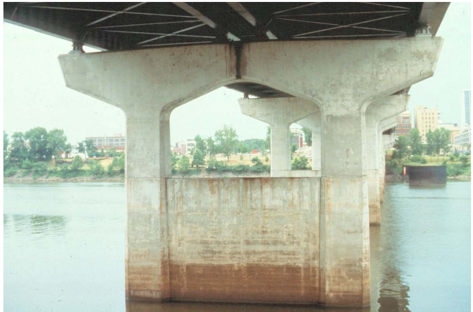
Figure 12.2.22 Cantilevered Piers Joined by a Web Wall
