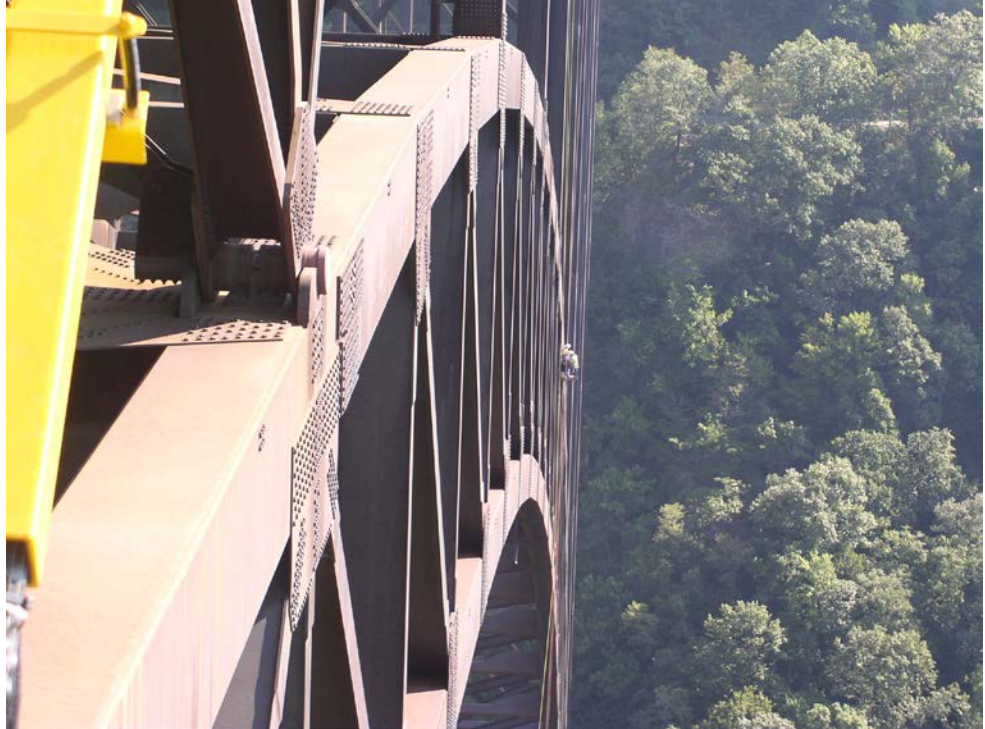
Figure 10.8.2 Steel Deck Arch Superstructure with Stiffening Truss and Gusset Plates
