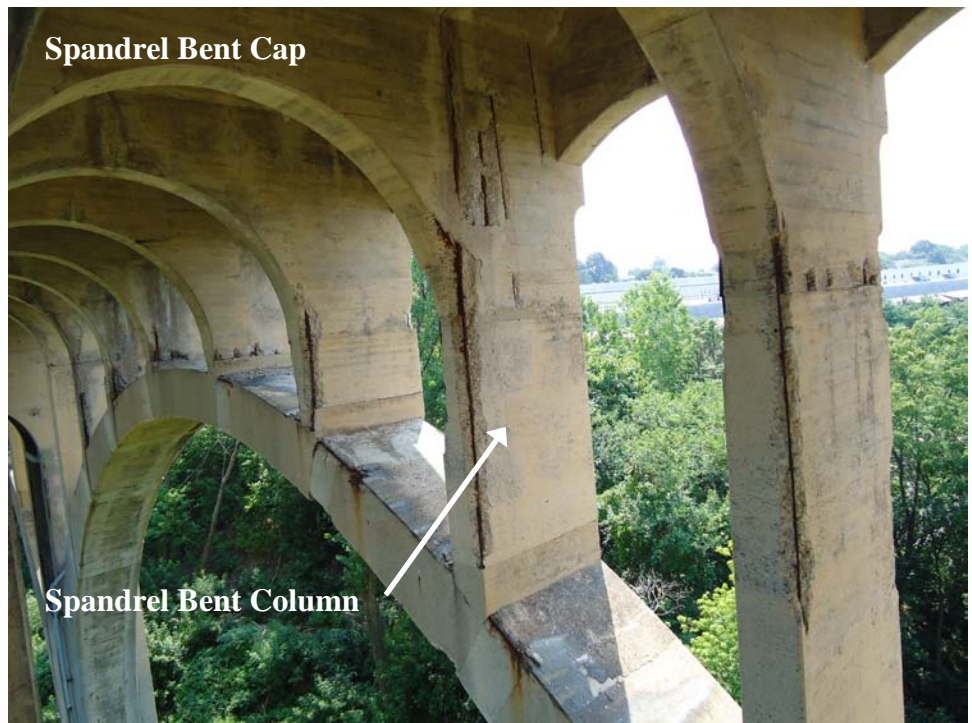
Figure 9.5.13 Spandrel Column Bent Cap Interface
