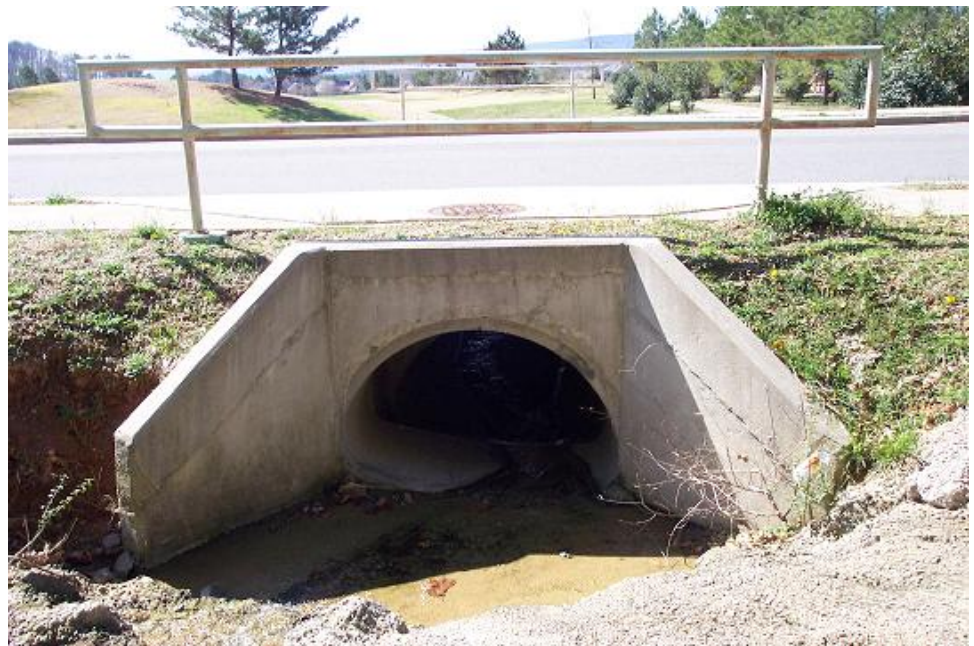
Figure 14.1.21 Culvert Headwall and Wingwalls
