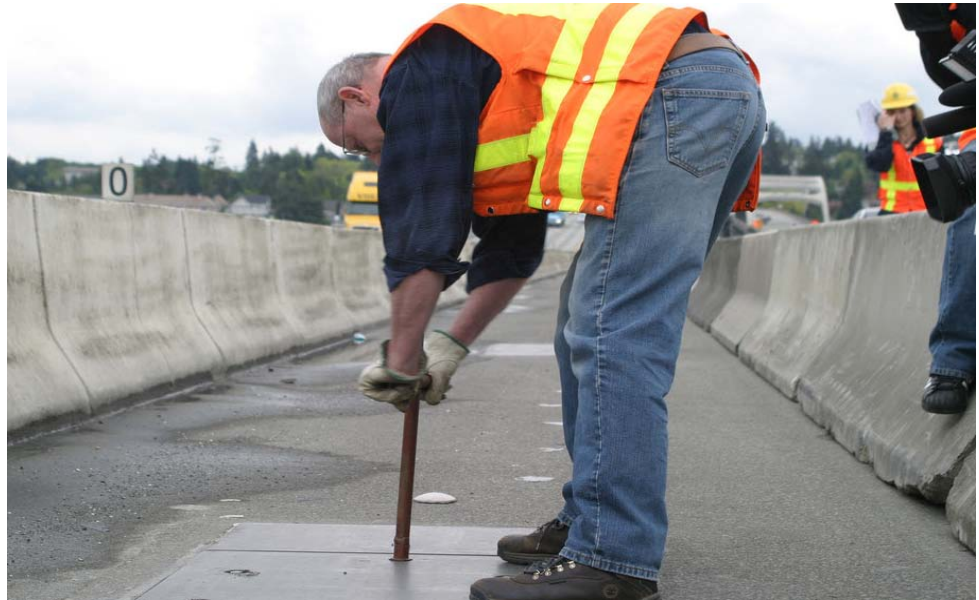
Figure 16.3.16 Inspector Opening Pontoon Access Hatch
