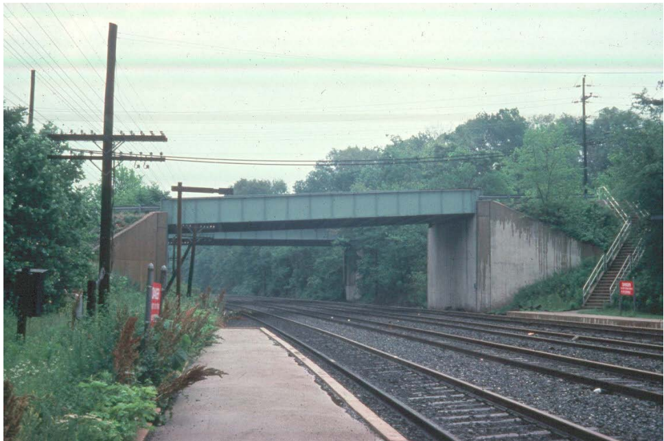
Figure 10.2.3 Through Girder Bridge with Limited Underclearance
