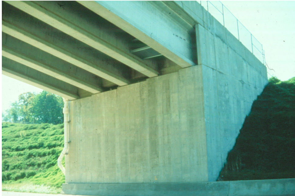
Figure 12.1.4 Full Height Abutment
