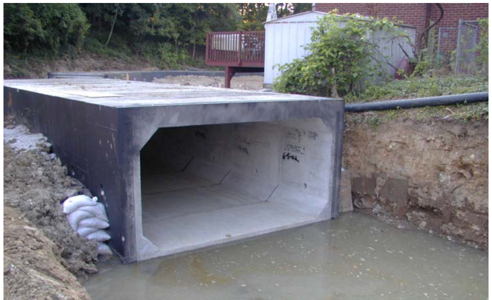
Figure 14.2.4 Precast Concrete Box Culvert
