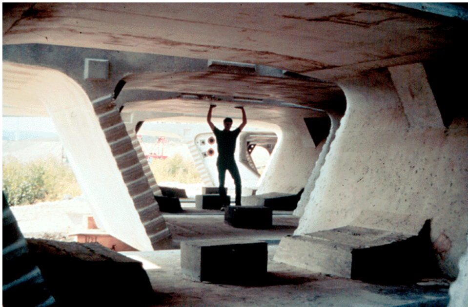
Figure 9.11.16 Box Girder Segment
