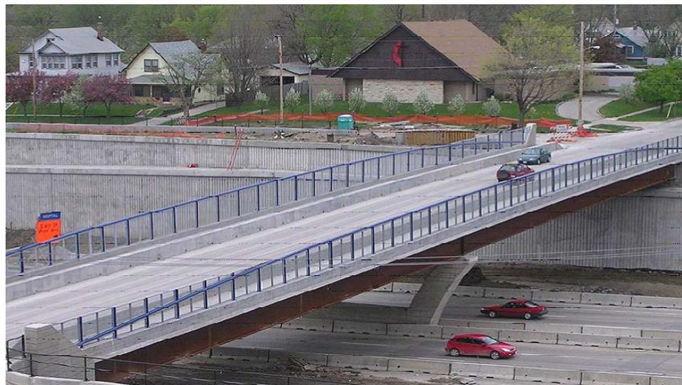
Figure 6.3.9 High Performance Steel Bridge
