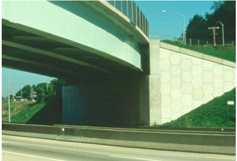
Figure 12.1.28 Independent MSE Wingwall
