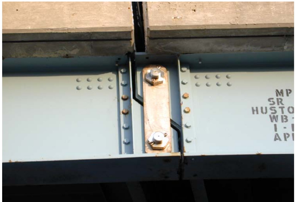
Figure 10.7.26 Stainless Steel Pin-and-Hanger Assembly
