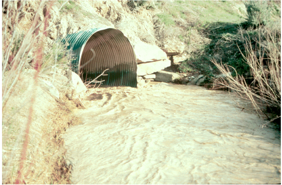
Figure 14.1.18 Culvert End Projection
