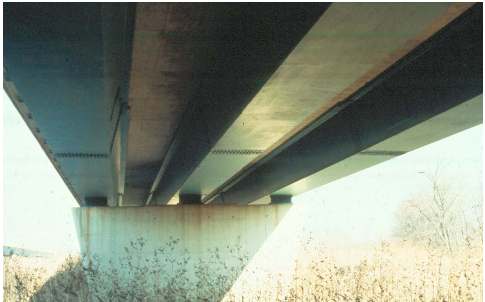
Figure 10.3.13 Redundant Box Girder Bridge
