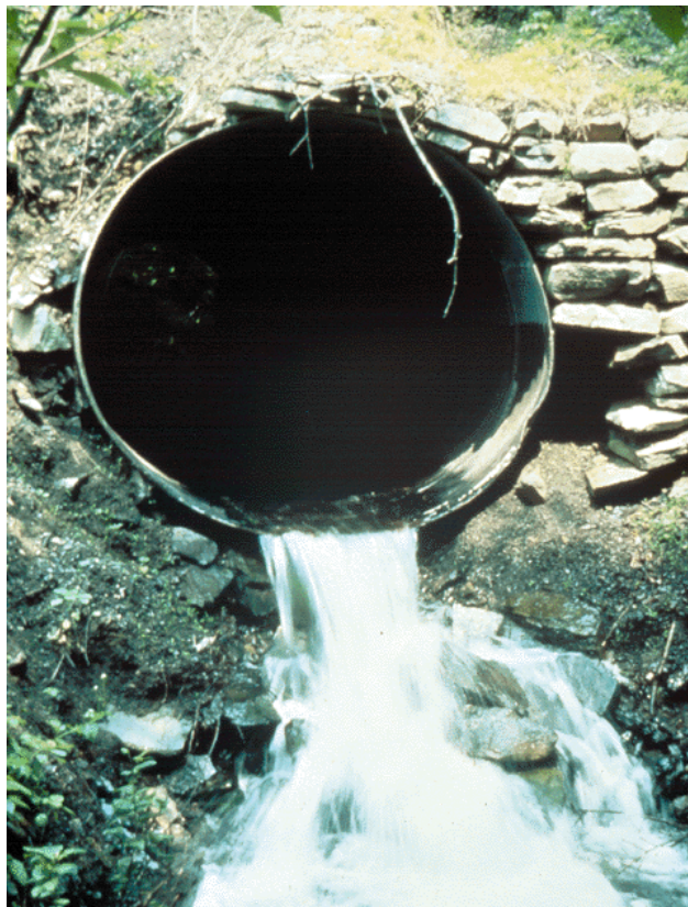
Figure 14.1.7 Circular Culvert Structure
