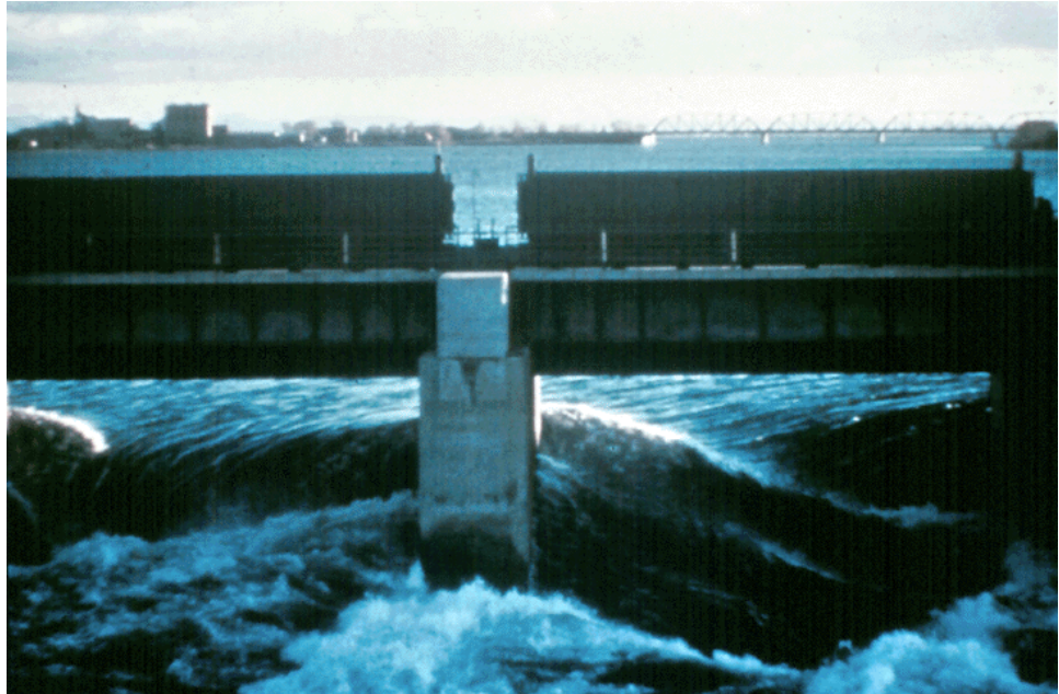
Figure 13.2.1 Flood Flow Around a Pier Showing High Streamflow Velocity
