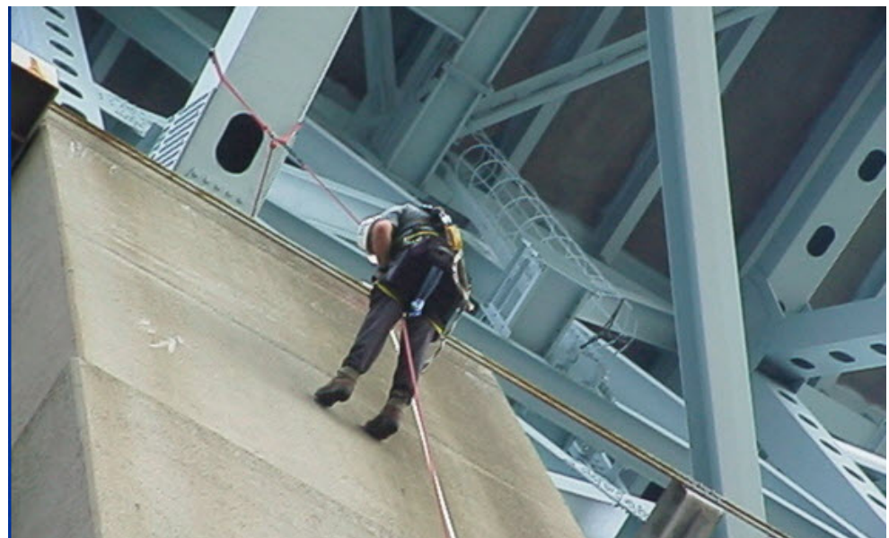
Figure 2.5.9 Inspector Rappelling Substructure Unit
