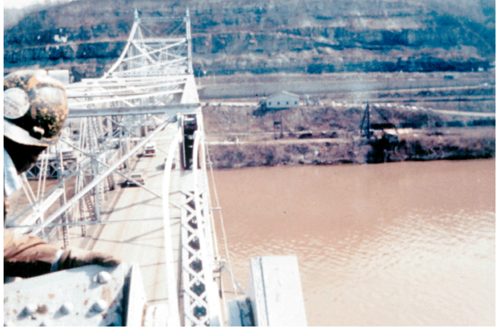
Figure 10.9.6 Inspection of Eyebars
