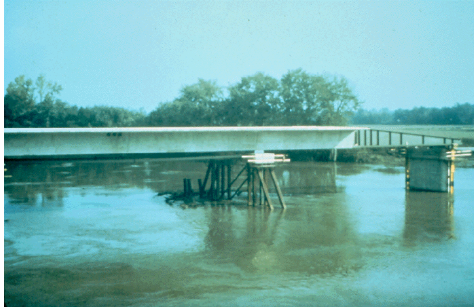
Figure 9.11.27 Incremental Launching Overview (Note Temporary Pile Bent)
