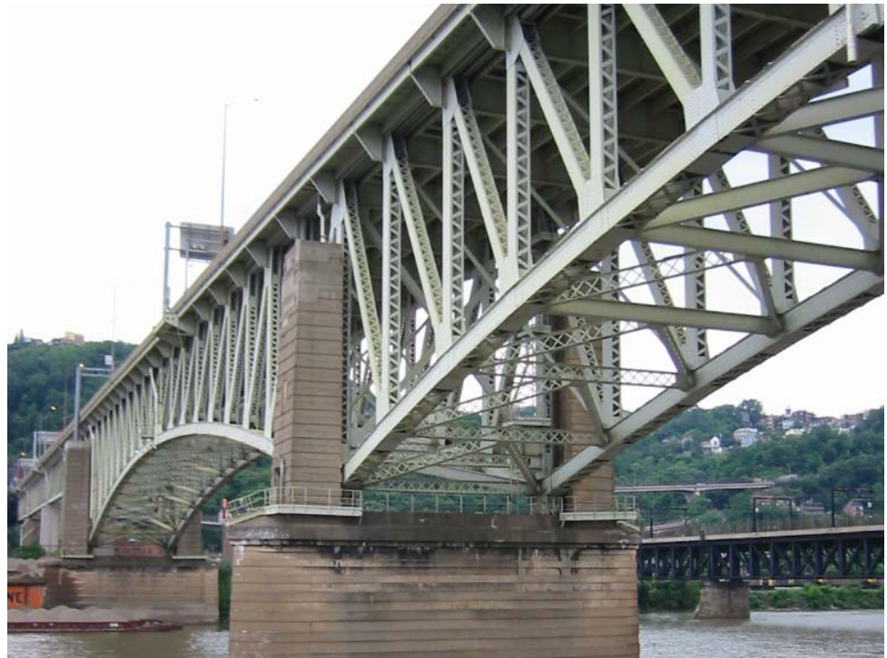
Figure 10.5.23 Bracing Members in Deck Arch Bridge
