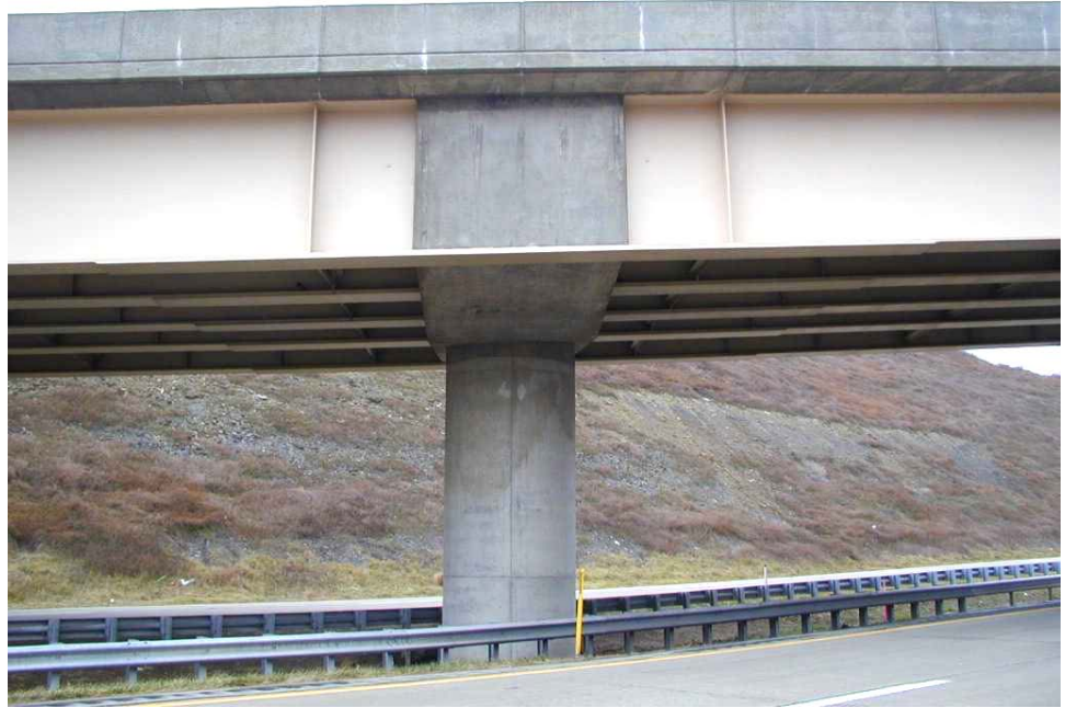
Figure 12.2.11 Integral Concrete Pier and Pier Cap
