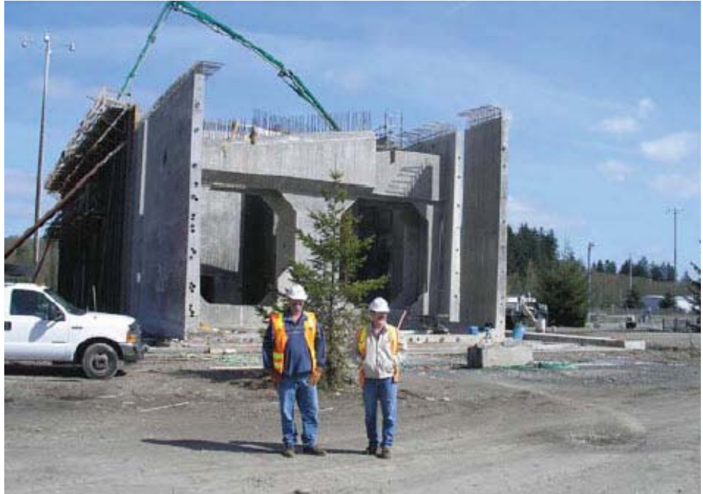
Figure 16.3.5 Concrete Pontoons Under Construction
