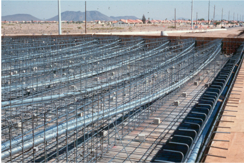
Figure 9.11.6 At-grade Formwork with Post-tensioning Ducts
