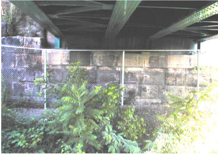
Photo No.5 North Abutment (far) - Elevation
