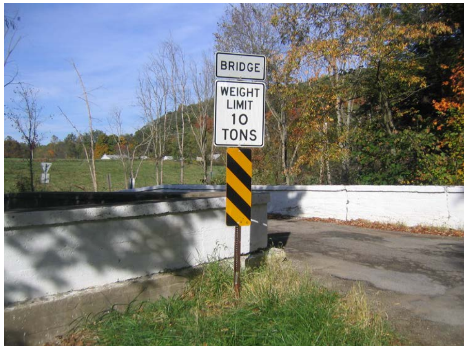
Figure 5.1.19 Bridge Weight Limit Posting
