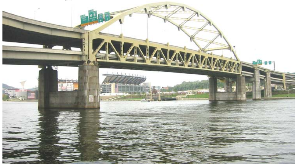
Figure 10.5.3 Tied Arch Bridge
