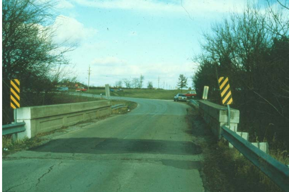
Figure 9.3.2 Concrete Through Two-Girder Bridge
