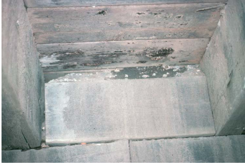
Figure 8.1.14 Typical Timber End Diaphragm
