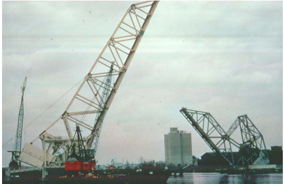
Figure 16.2.32 Concrete Counterweight on a Single-Leaf Bascule Bridge
