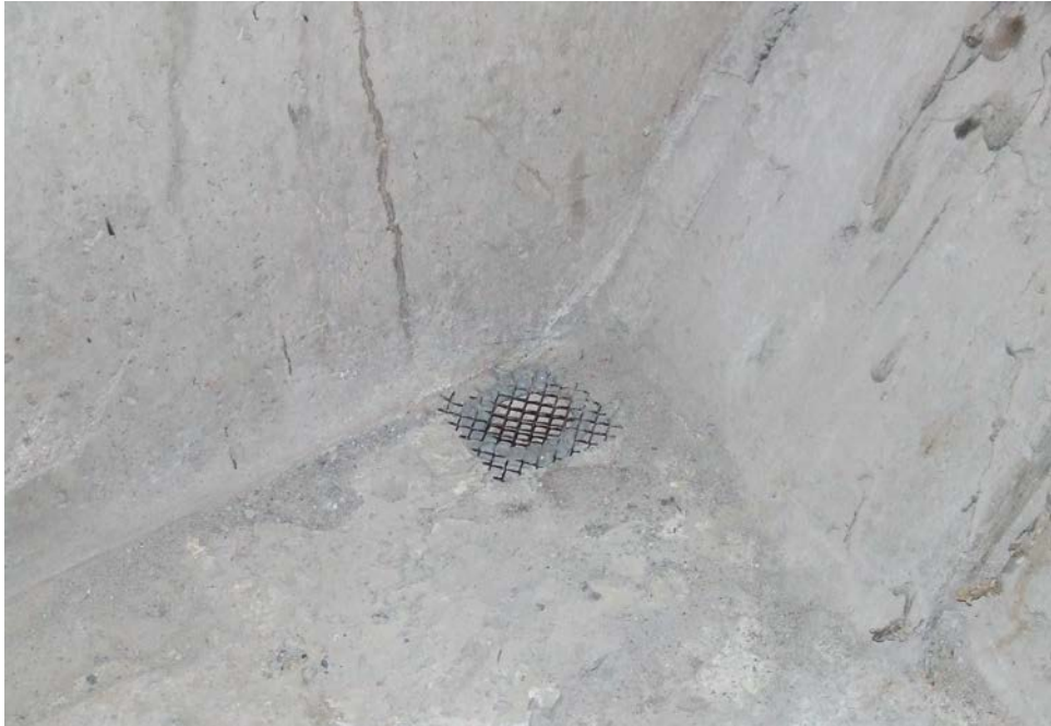
Figure 9.11.37 Concrete Box Girder Drain Hole with Screen
