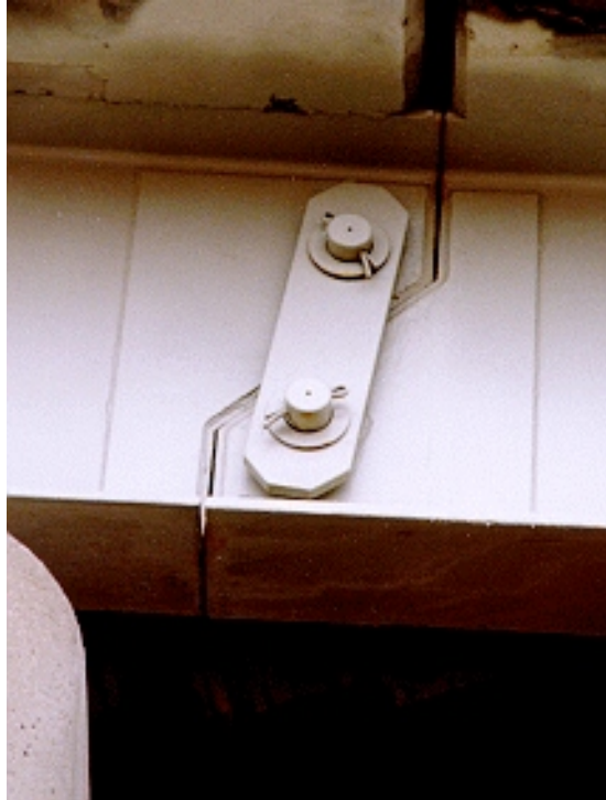
Figure 3.1.26 Pin and Hanger Assembly
