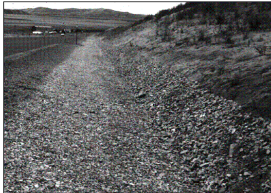
Figure 5.3. Riprap channel lining.
