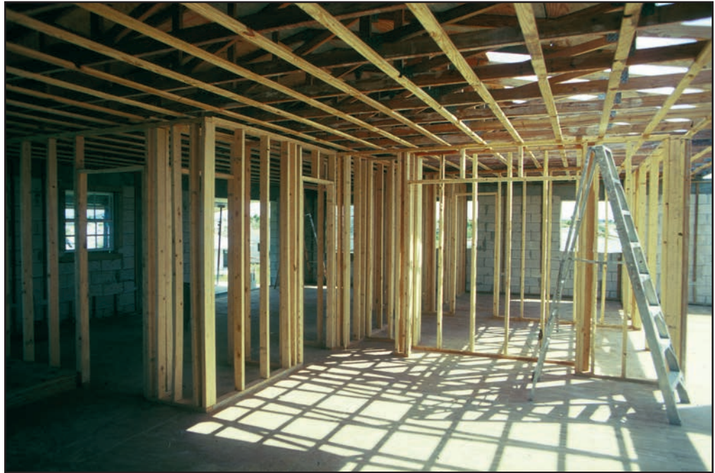
Figure 48 Wood 2 by 4 studs were used to frame the interior walls of the second story.
