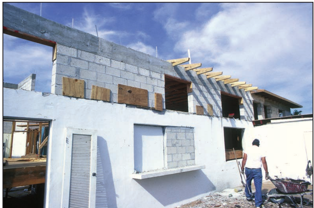
Figure 67 The extended first-story walls.
