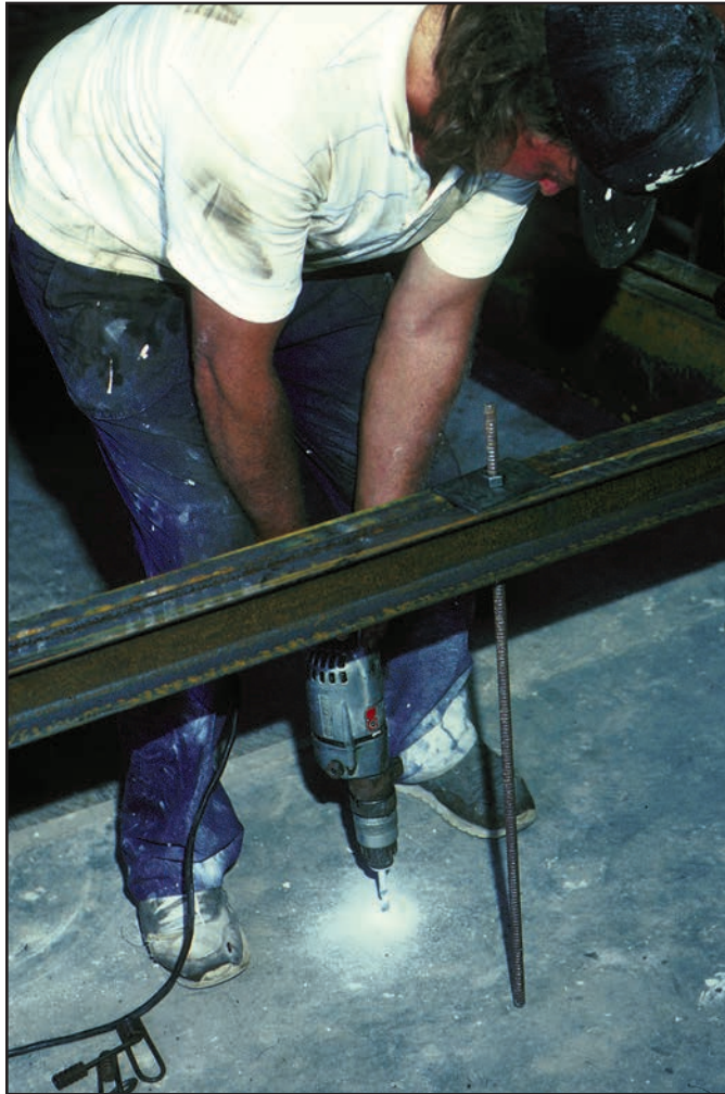
Figure 77 ... install anchors ...
