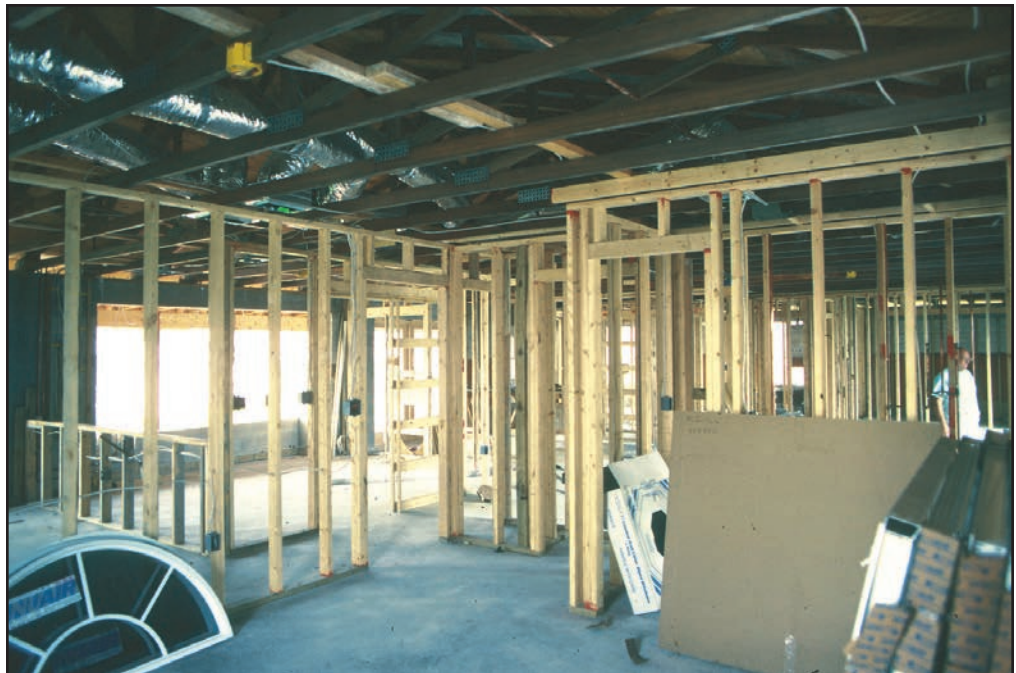
Figure 30 Interior partition walls and utilities are added.
