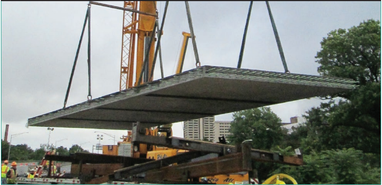
Figure 18. Transport and rigging of precast deck panel.
