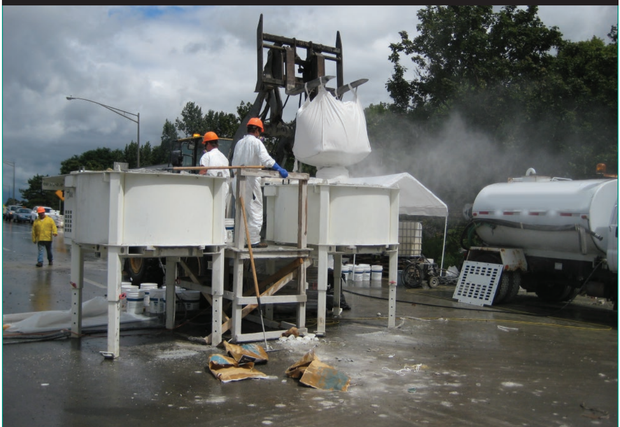
Figure 25. Mixing operation for the field-cast UHPC.
