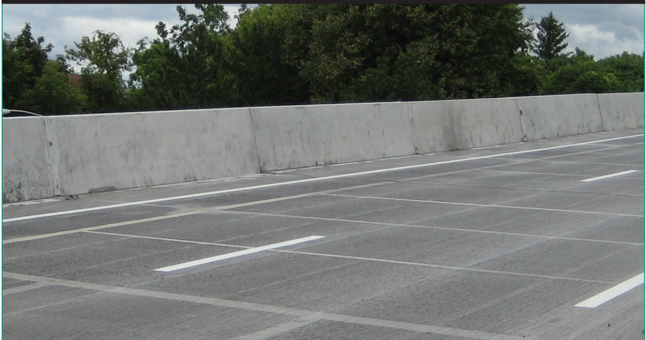
Figure 27. Bridge deck after grinding, grooving, and opening to traffic.
