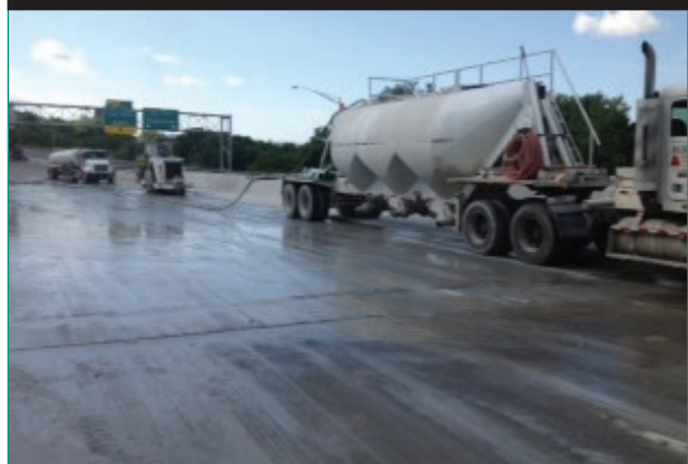
Figure 16. Surface profiling of a bridge deck on I-81 near Syracuse, NY.
