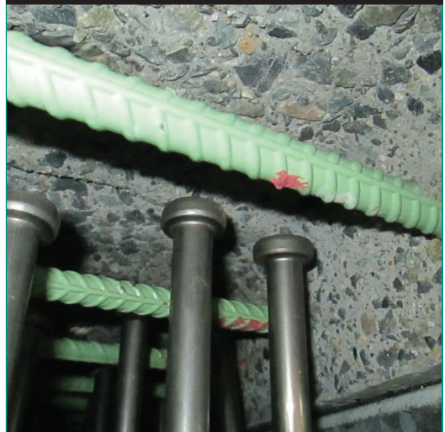
Figure 23. Hidden pocked connection detail with shear studs extending above the bottom mat of rebar to allow use with non-UHPC grouts or concretes.
