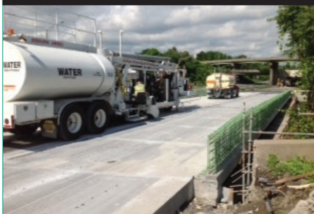
Figure 15. Surface profiling of a bridge deck on I-690 near Syracuse, NY.
