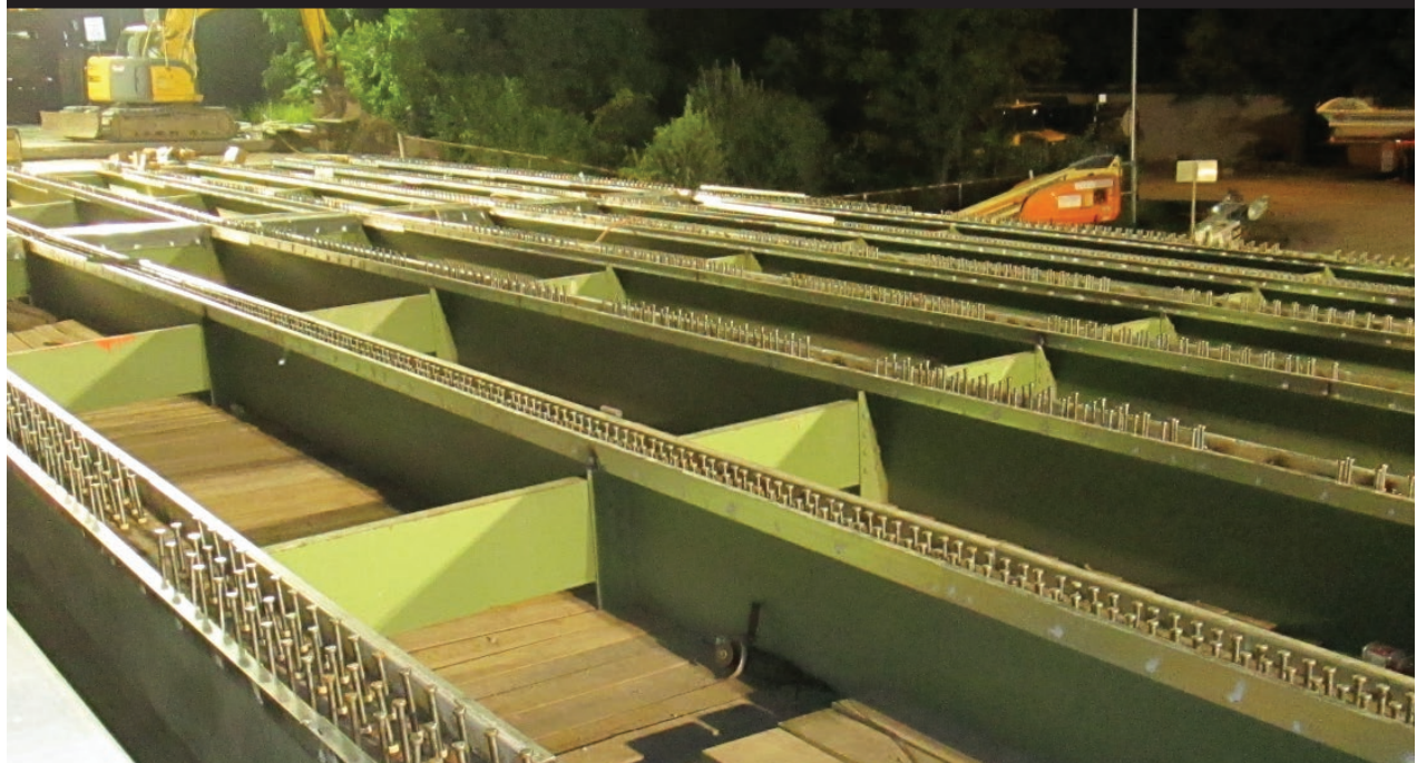
Figure 17. Superstructure prepared for precast panel installation.
