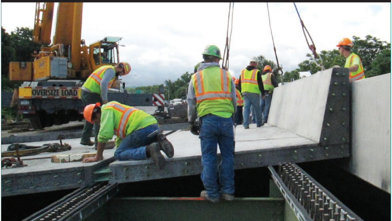
Figure 19. Installation of precast panel with integral barrier.
