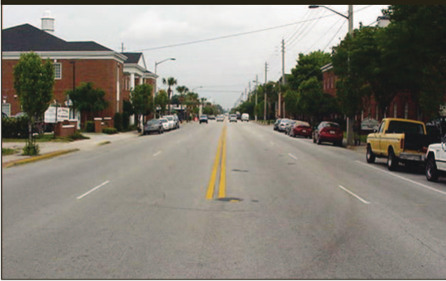
Figure 1. Photo. Four-lane configuration before road diet.
