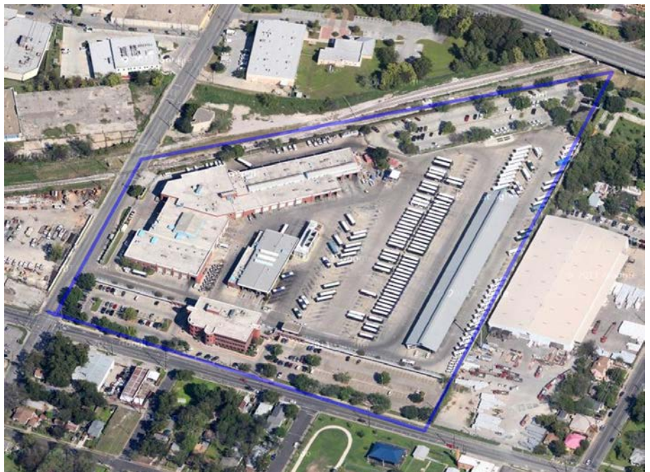
Capital Metro headquarters facility
