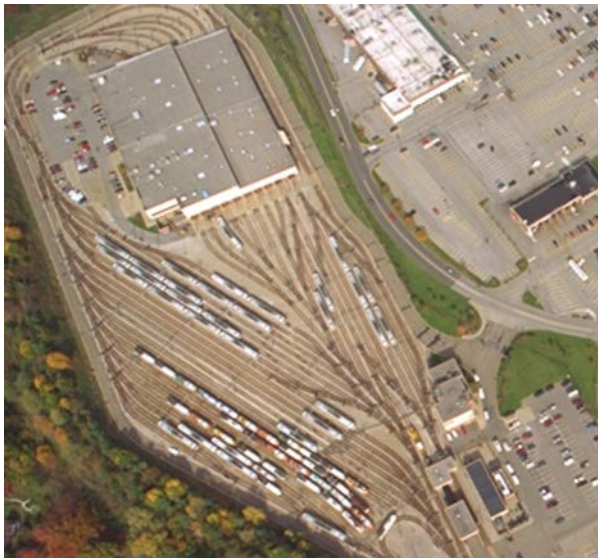
South Hills Village Rail Center
