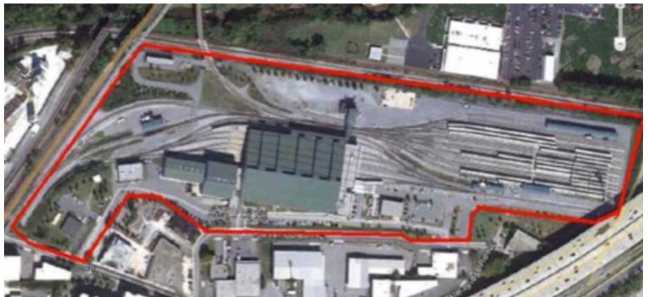
Armour Yard Vehicle Maintenance Facility (EMS scope outlined)
