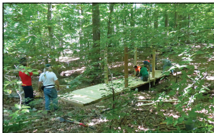
Colonel Dave Peeler (USMC Ret), Dennis Mitchell and others "supervise" as the treads get secured to a boardwalk on Beaver Pond Trail.
