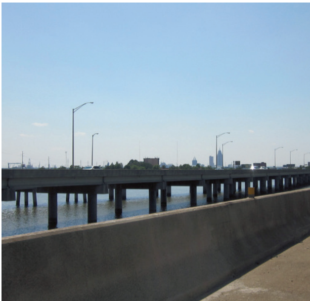
Figure 2: Highway asset in the study area. Photo credit: Infrogmation
