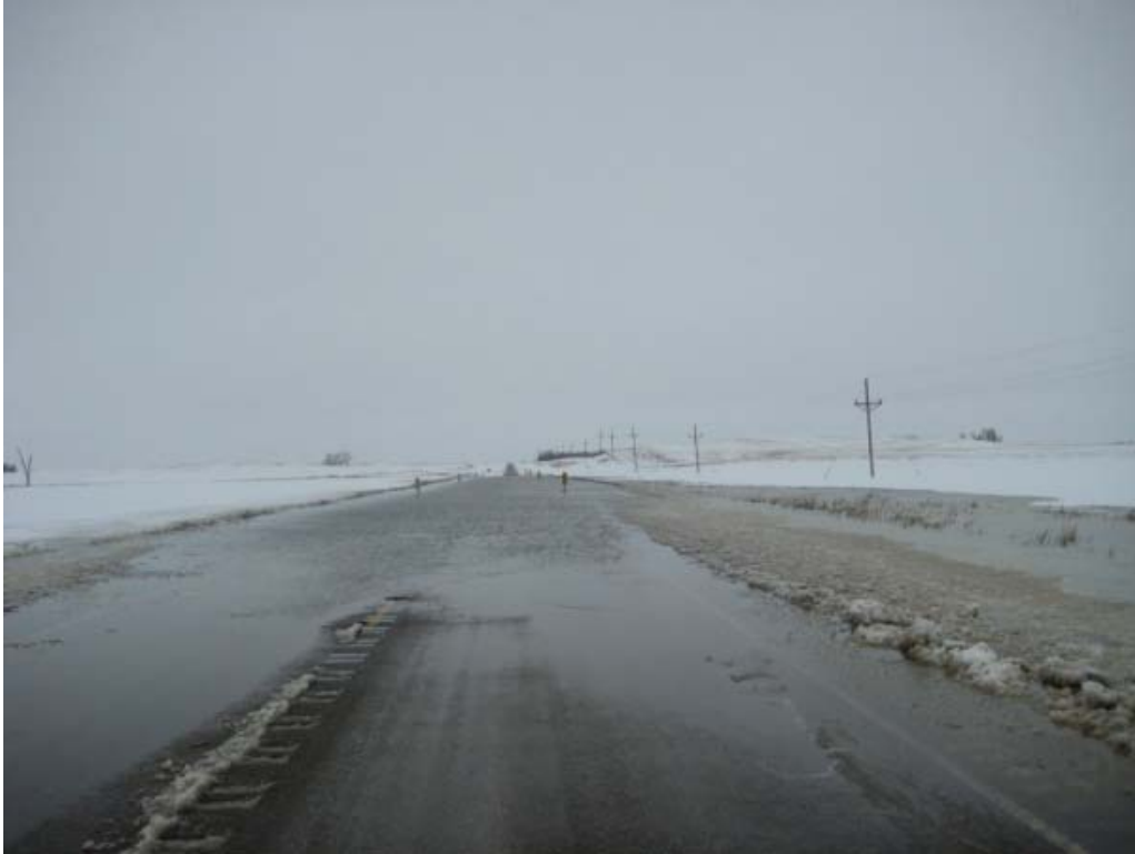
Photo: f F4 site roadway conditions. Source: FHWA ND Division Office.
