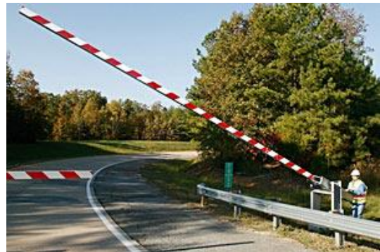
Figure 9. Gates at freeway entrances/exits are a key element in managing evacuations in Virginia.
