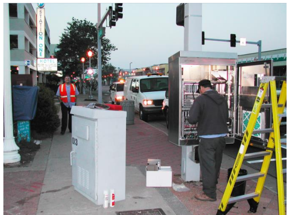
Figure 16. Virginia Beach traffic signal control cabinet installation
