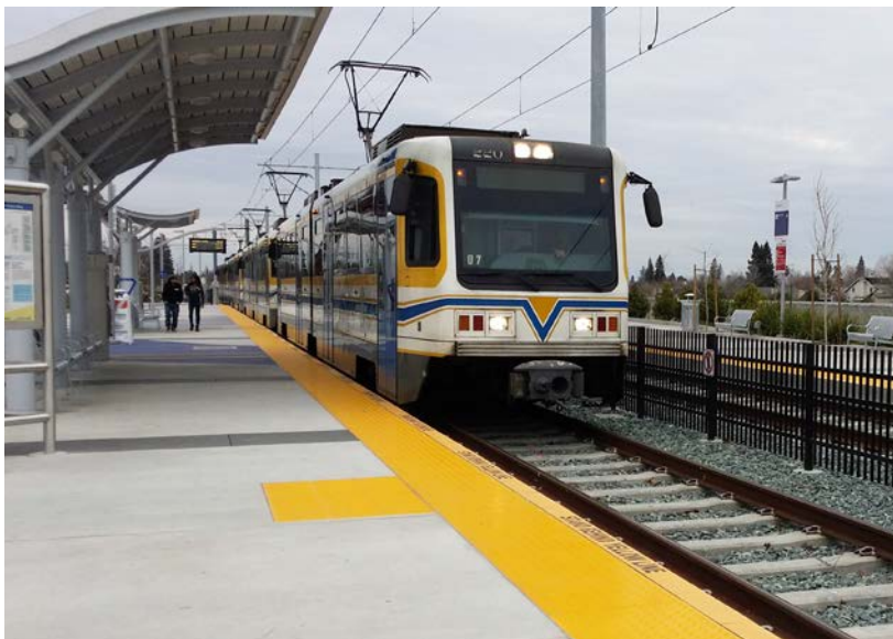
Figure 17: Light Rail Station Along the Recent Blue Line Extension
