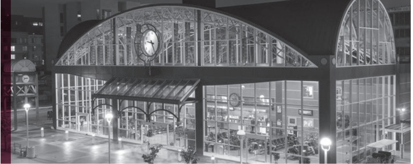
Photo: Greg Linhares, City of Oakland
