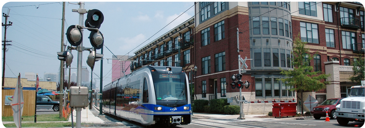
Street Crossing for LYNX Blue Line Train
