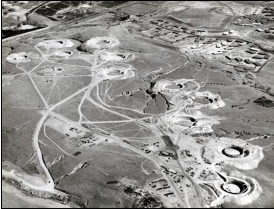
Photo 3.2-2. Installation of the USTs at the Main Terminal in 1942 (DLA 2008)
