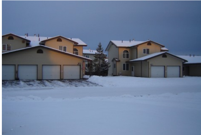
Figure 12. Eielson AFB French Creek Section 801 Housing Units
