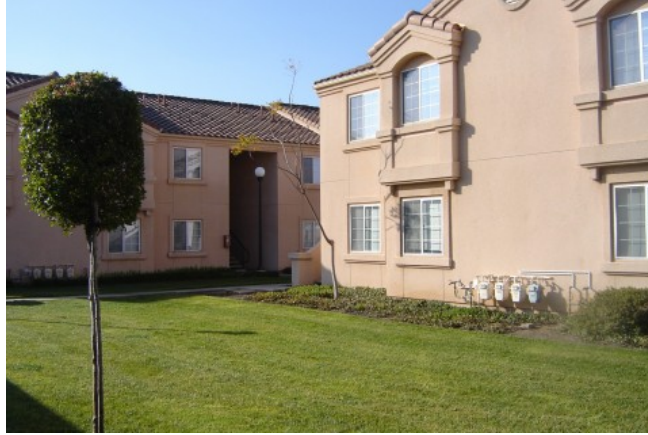
Figure 10. NBVC Section 801 Housing Units
