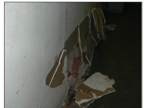
Figure 2: Leaking Pipes and Cracked Walls at a Damaged Warehouse Facility at Fort Sam Houston
