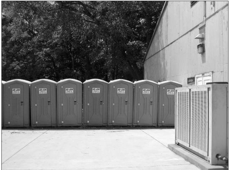
Figure 11: Outdoor Portable Facilities Used to Supplement Inadequate Indoor Facilities at Quantico Marine Corps Base, Virginia
