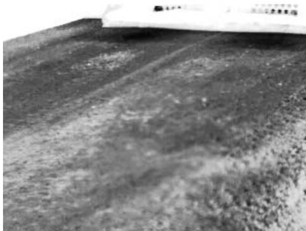
Figure 19. Photo. Thermal image of hot mix placement from the back of the paver.
