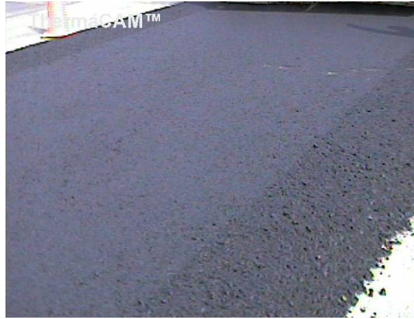
Figure 18. Photo. Conventional photo of hot mix placement from the back of the paver.
