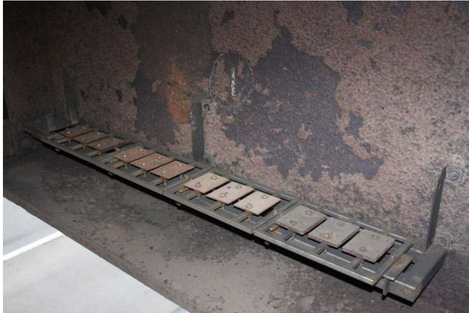
Figure 36. Photo. Corrosion coupons on Moore Drive Bridge on rack 1 just prior to removal after 1-year exposure.
