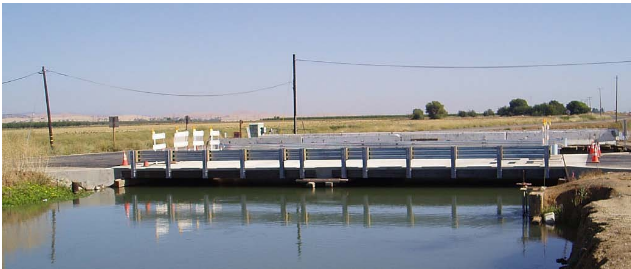
Figure 1. Photo. Fairview Road Bridge over the Glen-Colusa Canal in Colusa, CA.
