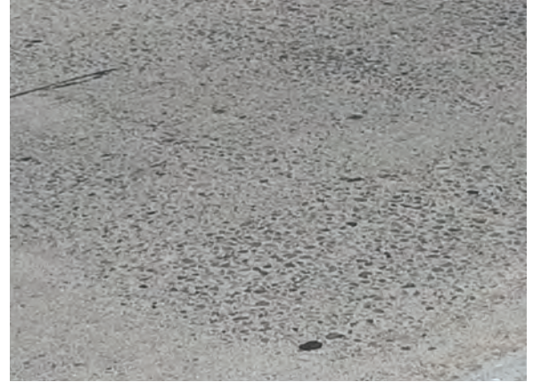
Figure 9. A close-up view of the Route 60E/71N interchange in the Los Angeles, CA, area shows good performance after 17 years of continual heavy traffic loads. (Surface wear and perhaps early grinding for rideability is apparent.)
