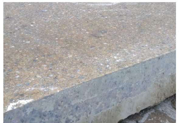
Figure 3. Cast surface of the slab section in Dublin, GA.
