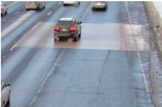
Figure 15. Repaired pavement on northbound I-90 in Chicago, IL, shows good performance of the CAC concrete after 5 years.
