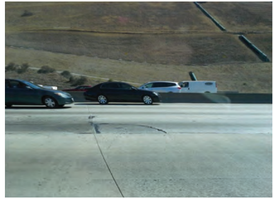
Figure 13. An example of pavement slabs cracking and spalling at joints after 1 year of use on Route 60W near Los Angeles, CA.
