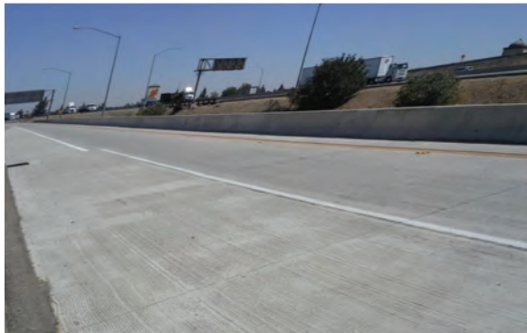
Figure 4. The Route 60W/71S interchange in the Los Angeles, CA, area shows good performance after 17 years of continual heavy traffic loads.
