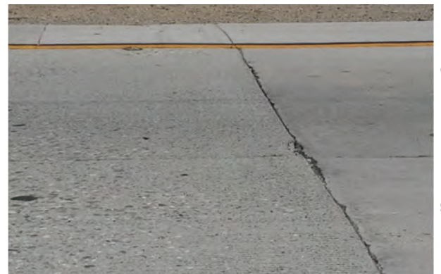
Figure 7. Surface wear and minor joint spalling on the Route 60W/71S interchange in the Los Angeles, CA, area.
