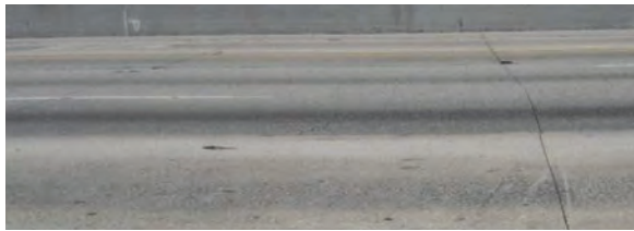
Figure 10. A close-up view of pavement slabs on I-10E near Los Angeles, CA, shows deterioration after 15 years.
