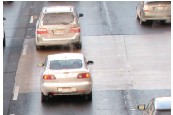
Figure 16. Vehicles travel over the repaired pavement on northbound I-90 in Chicago, IL, which shows good performance of the CAC concrete after 5 years.
