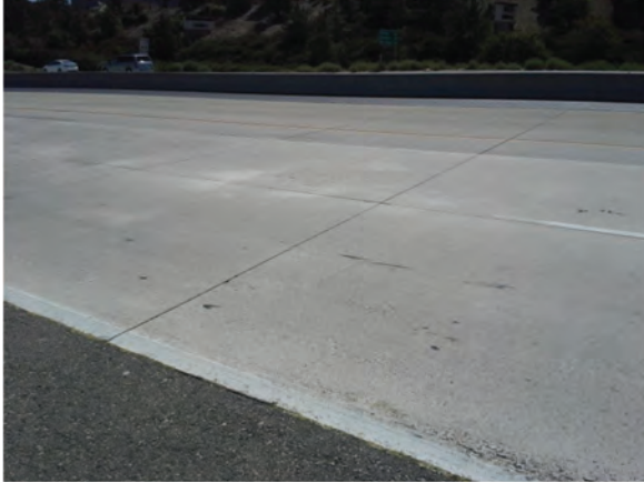
Figure 8. The Route 60E/71N interchange in the Los Angeles, CA, area shows good performance after 17 years of continual heavy traffic loads.
