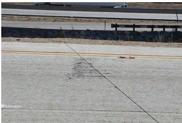
Figure 6. The Route 60W/71S interchange in the Los Angeles, CA, area. (A defect, perhaps caused by a placing or finishing issue, is apparent in the passing lane.)
