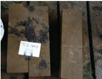
Figure 18. CSA cement concrete beams after 1 year of exposure at Treat Island.
