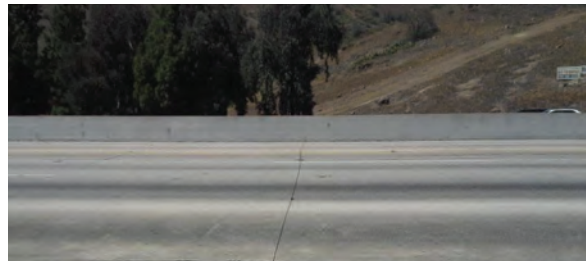
Figure 11. Pavement slabs on I-10E near Los Angeles, CA, shows deterioration after 15 years.
