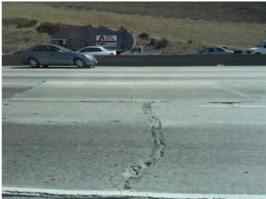
Figure 12. Pavement slabs on Route 60W in Los Angeles, CA, show some cracking and spalling at joints after 1 year of use.
