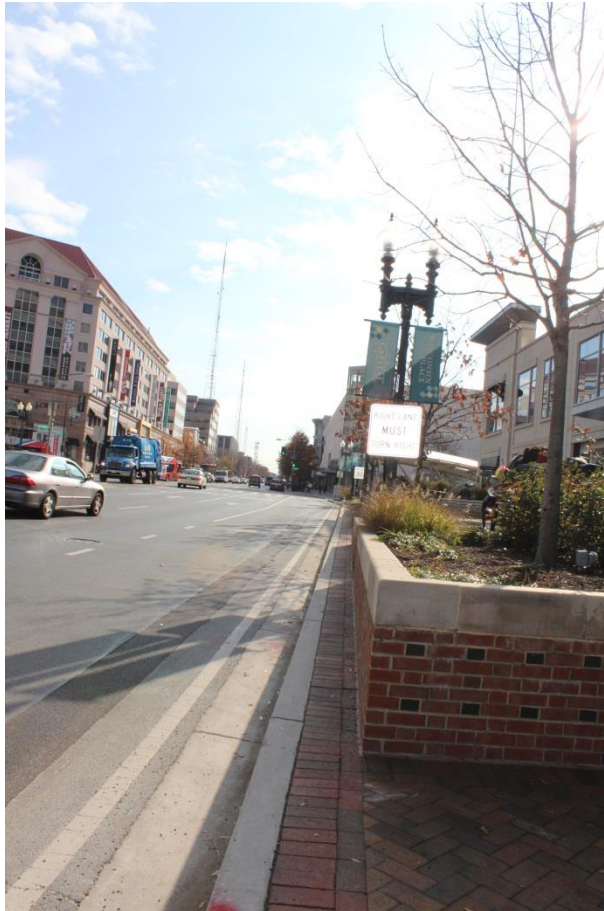
Figure 56. Photo. View of the planters located between the southbound lanes of traffic and the adjacent sidewalk along Wisconsin Avenue.
