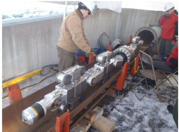
Workers ready a robot for a field test of its ability to inspect the interior of pipelines for faults and cracks.
