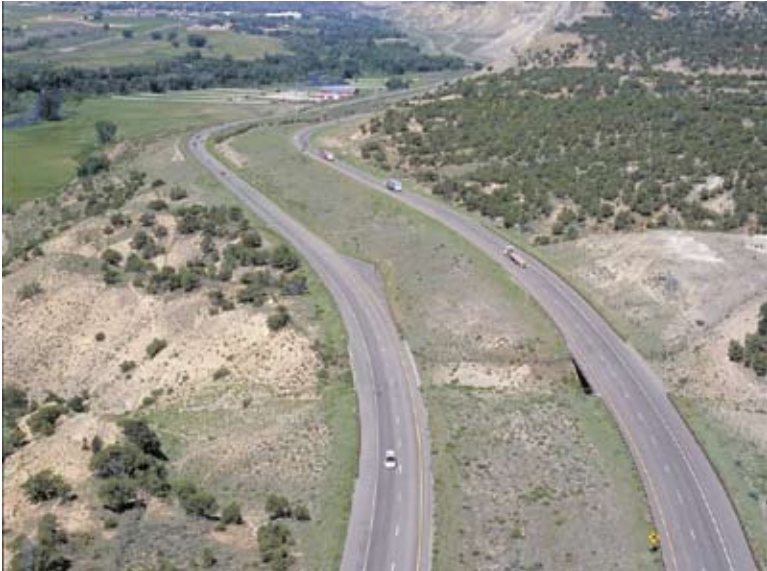
Aerial photo of I-70 near Gypsum.
