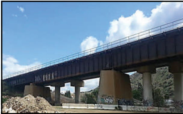
BSNF Railroad Bridge
