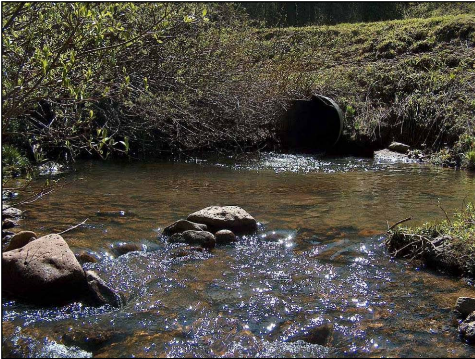
Figure H.2b. North Thompson Creek Culvert Outlet.
