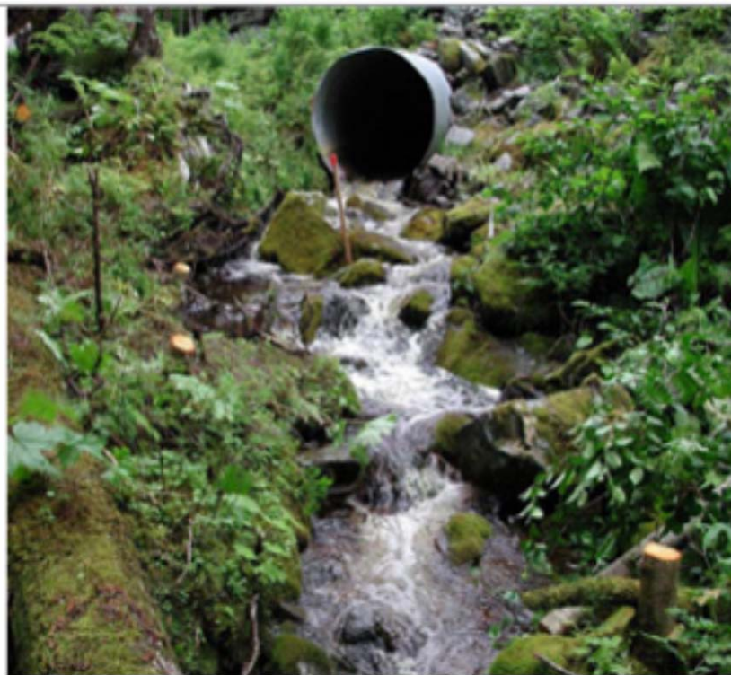
Figure I.1. Tributary to Bear Creek Culvert Outlet.
