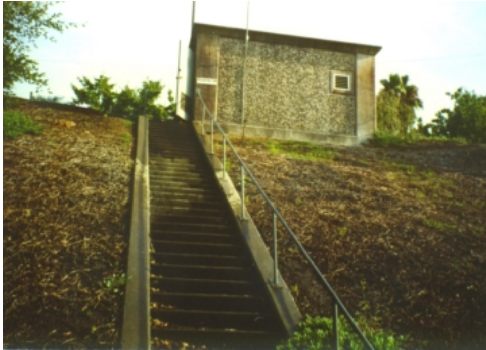
Figure 5-2. Pump station for a depressed section
