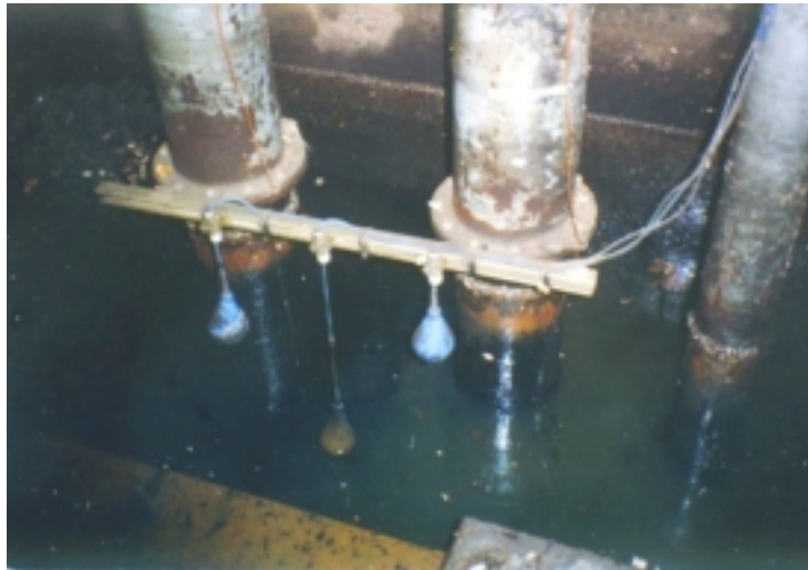
Figure 11-6. Tilting bulb switch
