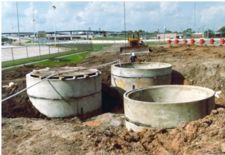
Figure 3-14. Circular caisson wet wells under construction.
