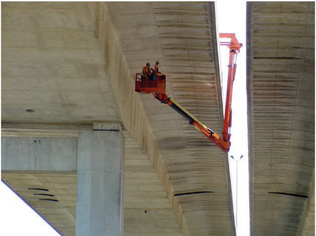
Bridge Inspection, Michigan DOT
