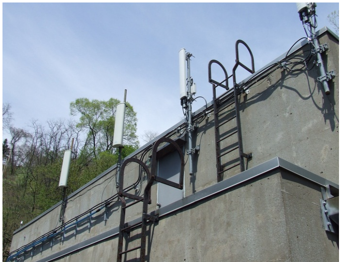
Figure 4.42 – Ancillary building: with metal ladders to roof.
