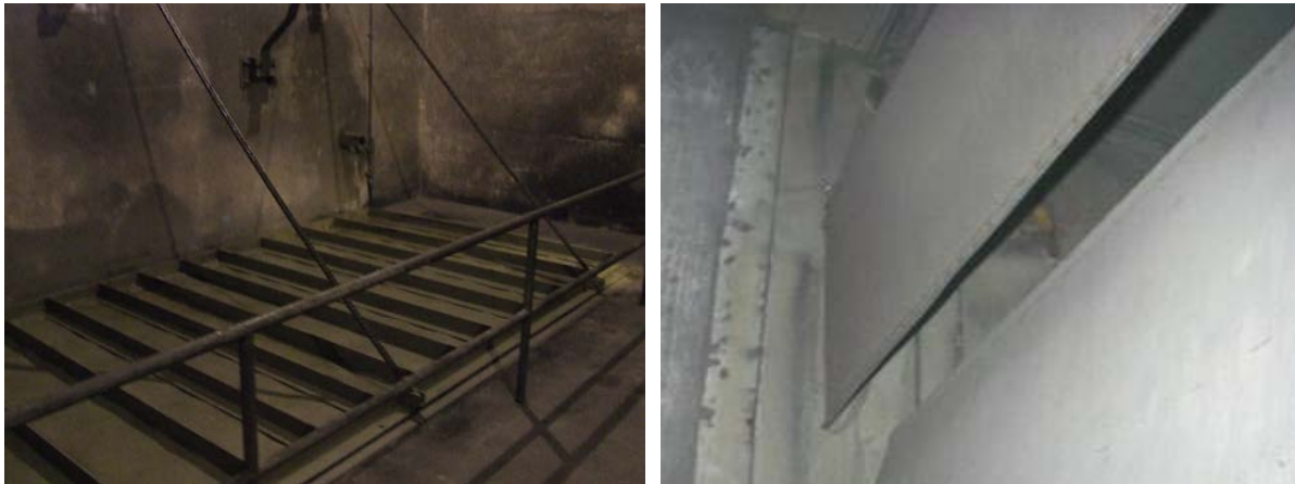
Figure 4.57 – Louvers in closed position, left; louver with large gap when closed, right.
