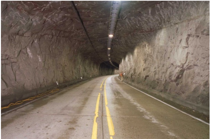
Figure 1.7 – Unlined rock tunnel.
