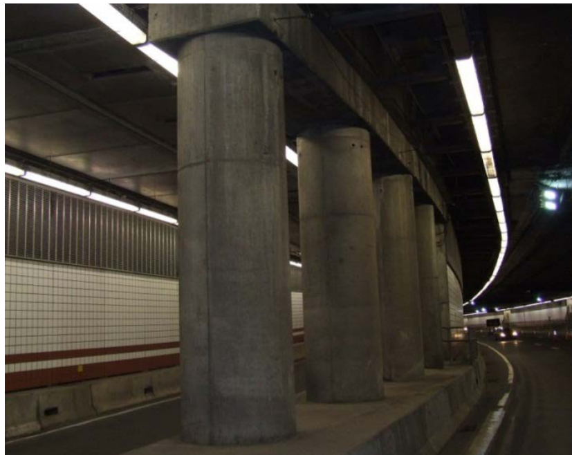
Figure 4.30 – Columns with bent cap.
