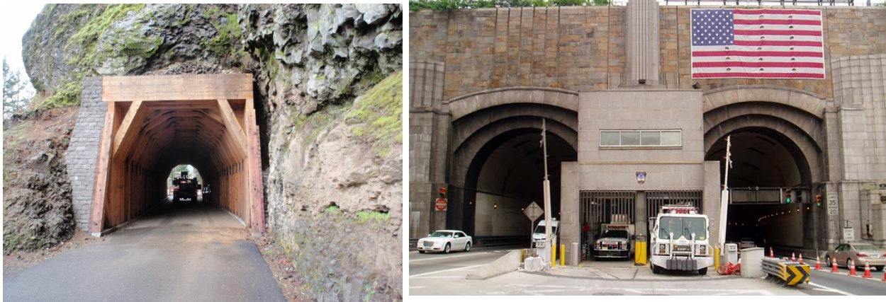
Figure 4.34 – Tunnel portals range from simple (left) to complex (right) structures.
