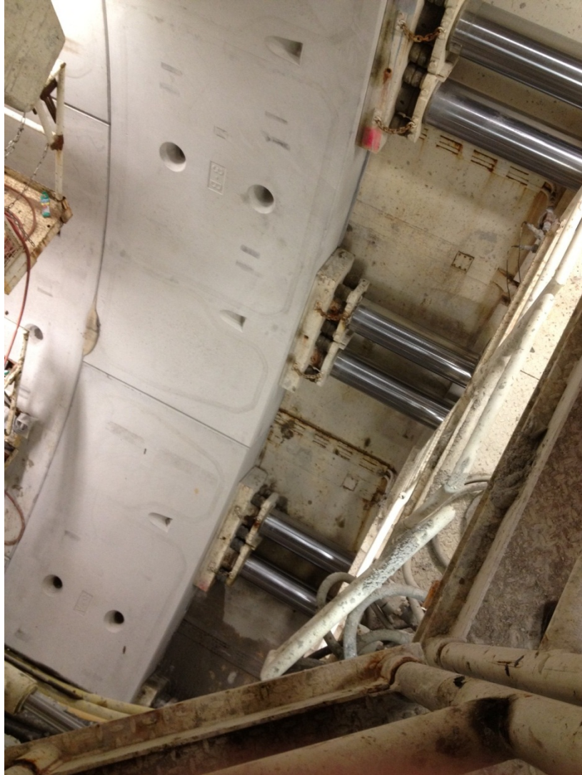
Figure 1.2 – TBM using large hydraulic jacks to advance against assembled segment ring.
