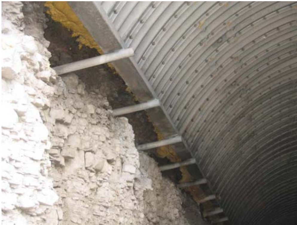
Figure 4.19 – Steel liner plate above the springline.
