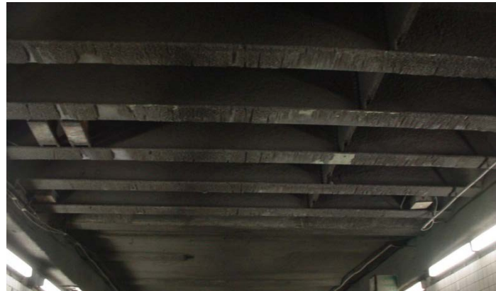
Figure 4.29 – Exposed roof girders.
