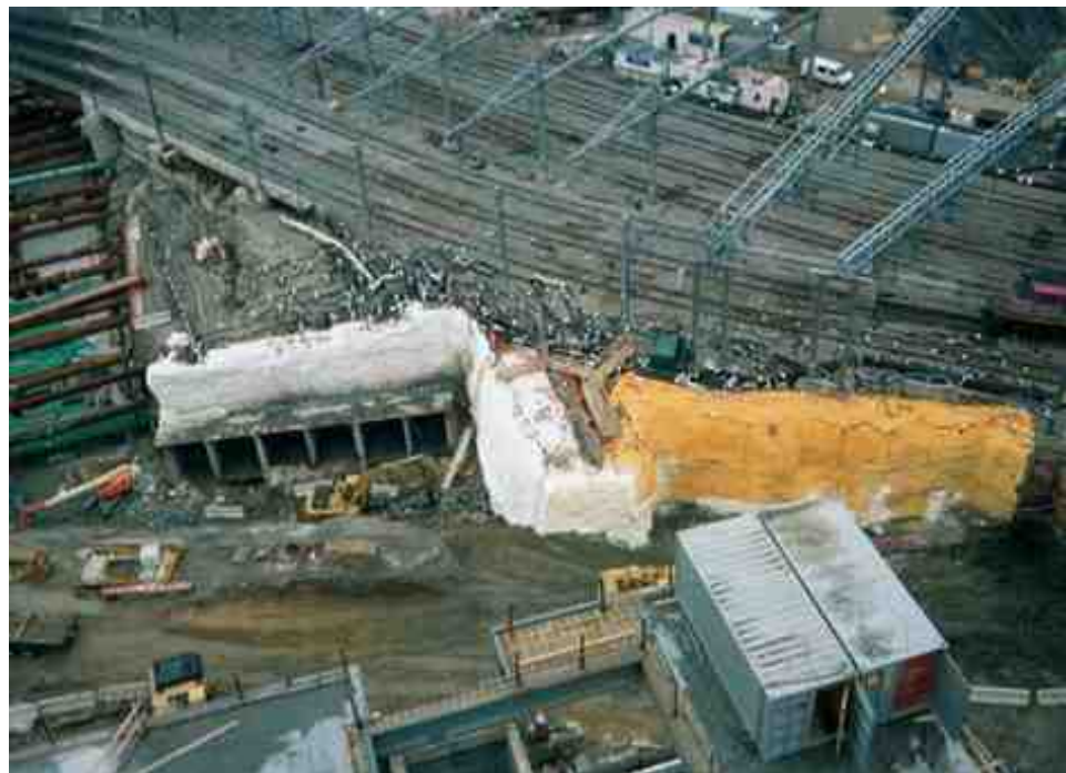
Figure 1.3 – Jacked tunnel advancing under rail corridor.
